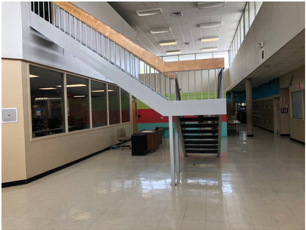
Figure 8 – North Stair in Building 3 Painted
