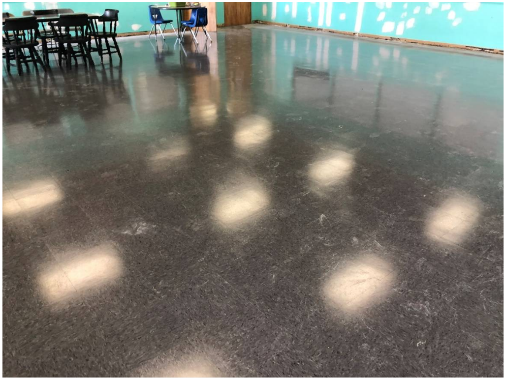
Figure 5 – Lobby A Flooring
