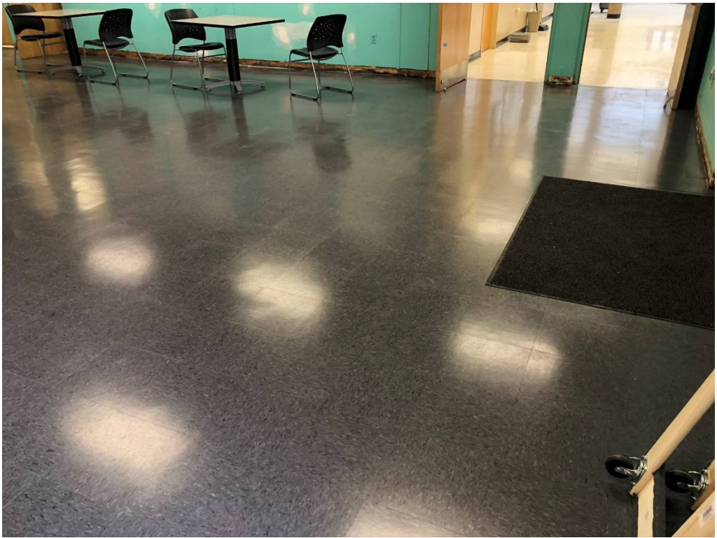
Figure 1 – Lobby B Flooring
