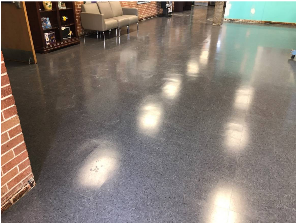
Figure 2 – Lobby B Flooring
