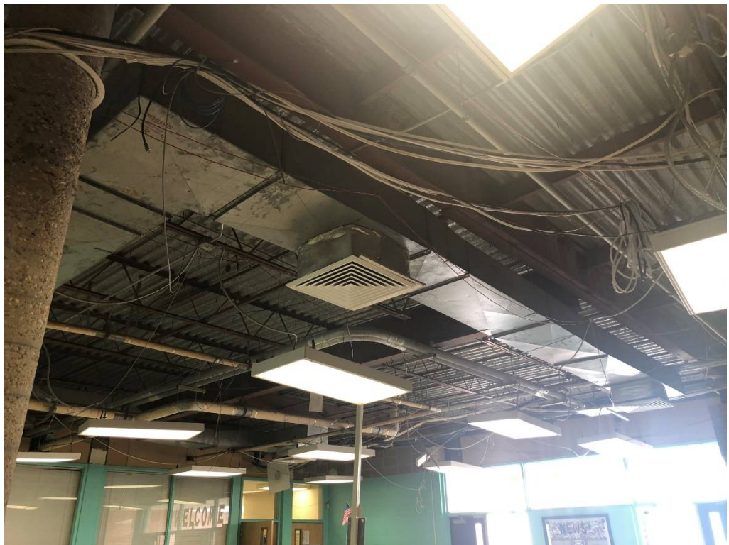
Figure 4 – Entry Lobby Ceiling Removed
