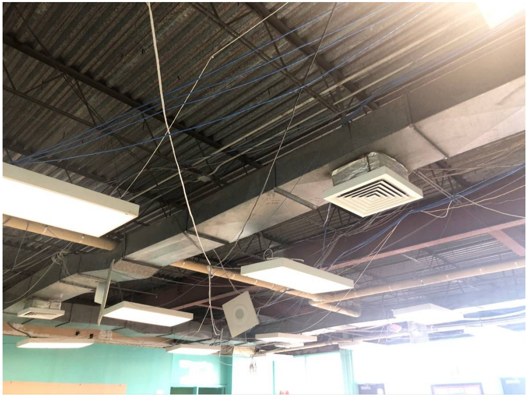
Figure 11 – Lobby @ Building 1 Ceiling Demoed
