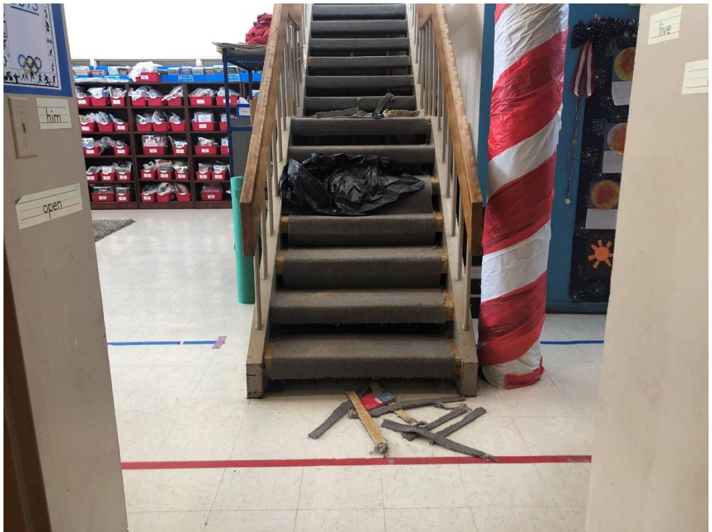
Figure 12 – Building 1 Stair Work
