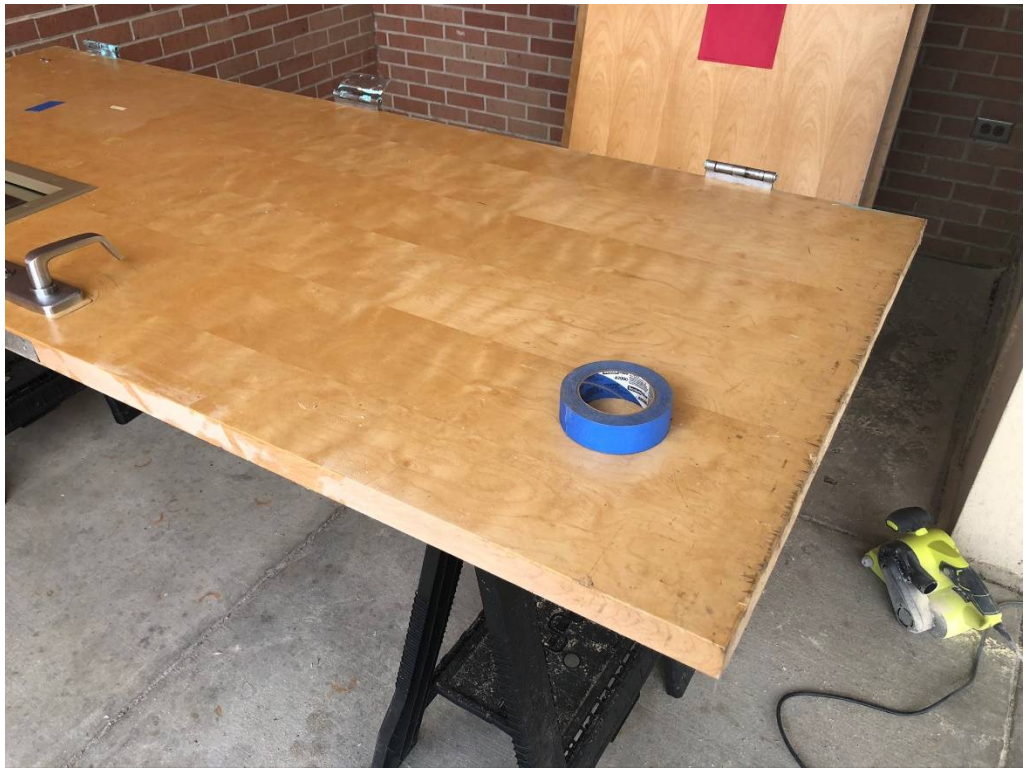
Figure 1 – Door Cut for Floor Overlay
