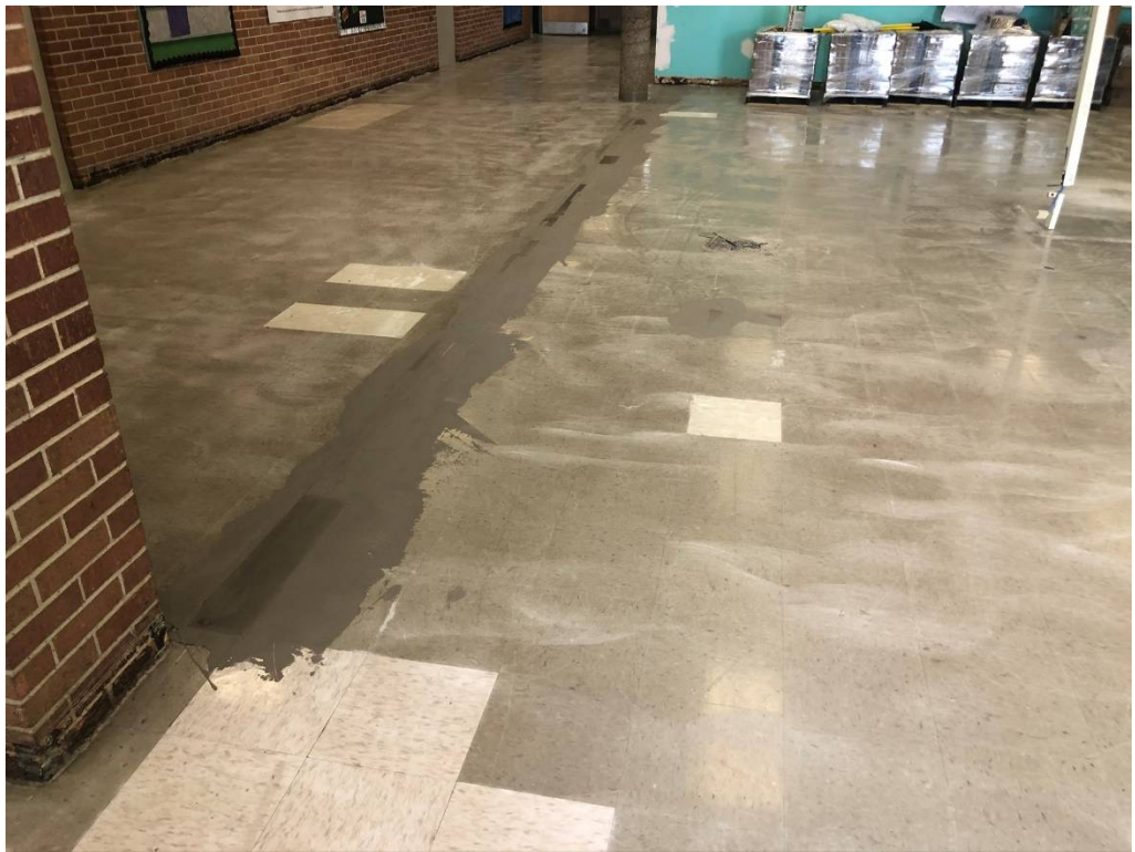
Figure 2 – Floor Prep at Entry (vct sanded and leveling compound added)
