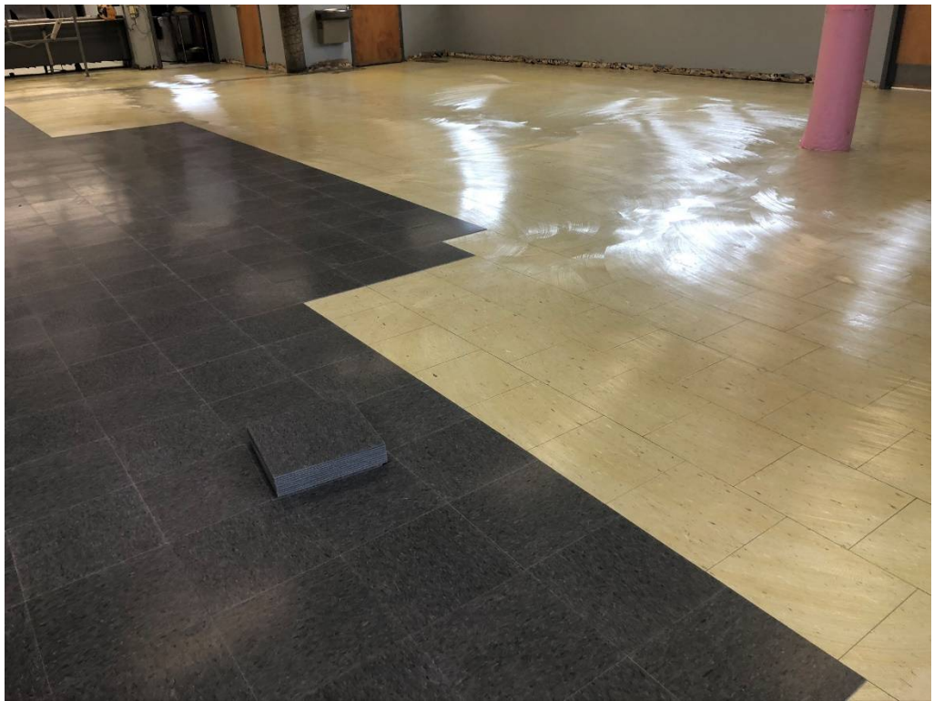
Figure 6 – New VCT Install Ongoing in Building 3 Cafeteria
