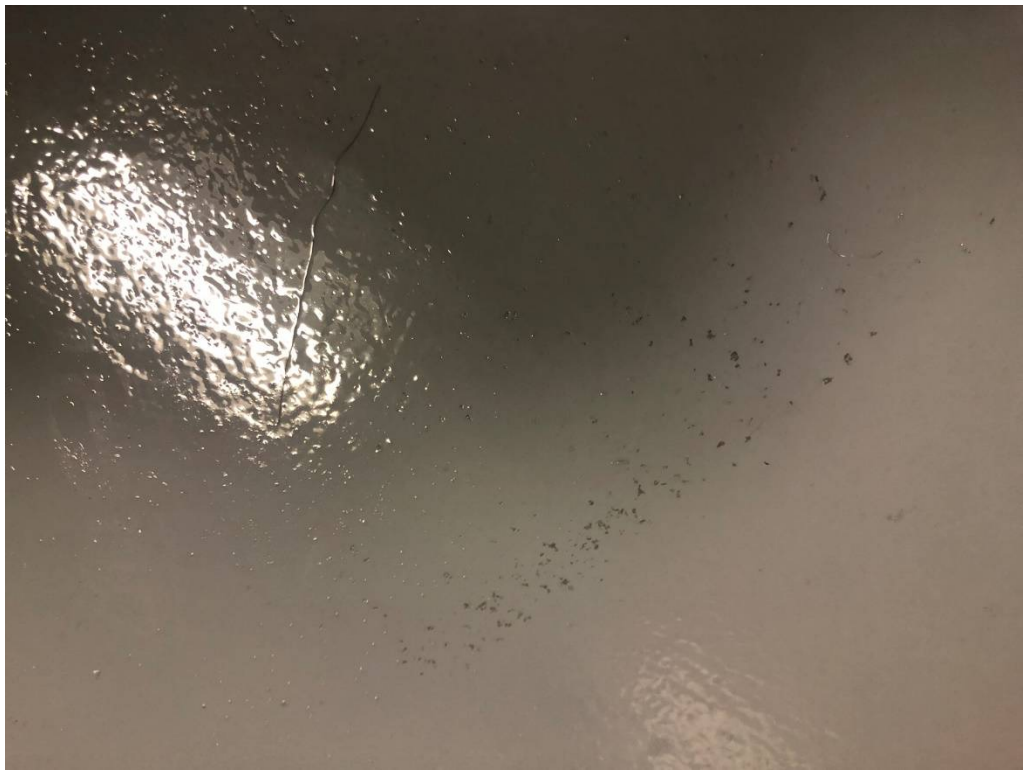
Figure 10 – Additional Coat Required in T06 for Full Coverage
