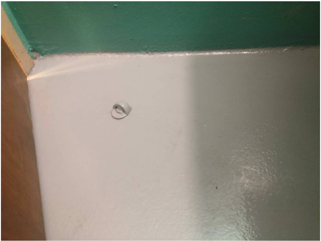
Figure 3 – Paint Over Door Stop (typical)
