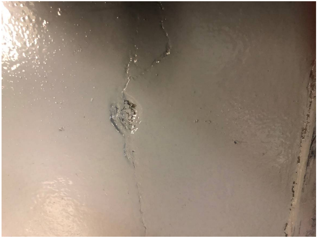
Figure 9 – Additional Coat Required in T06 for Full Coverage
