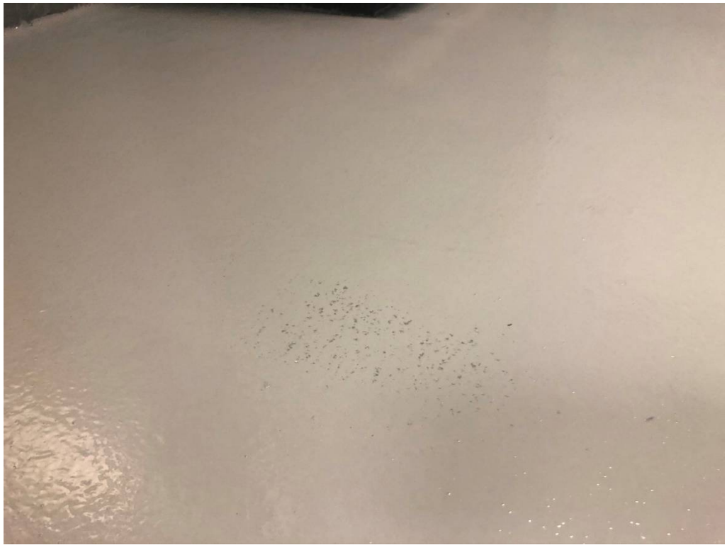
Figure 11 – Additional Coat Required in T06 for Full Coverage
