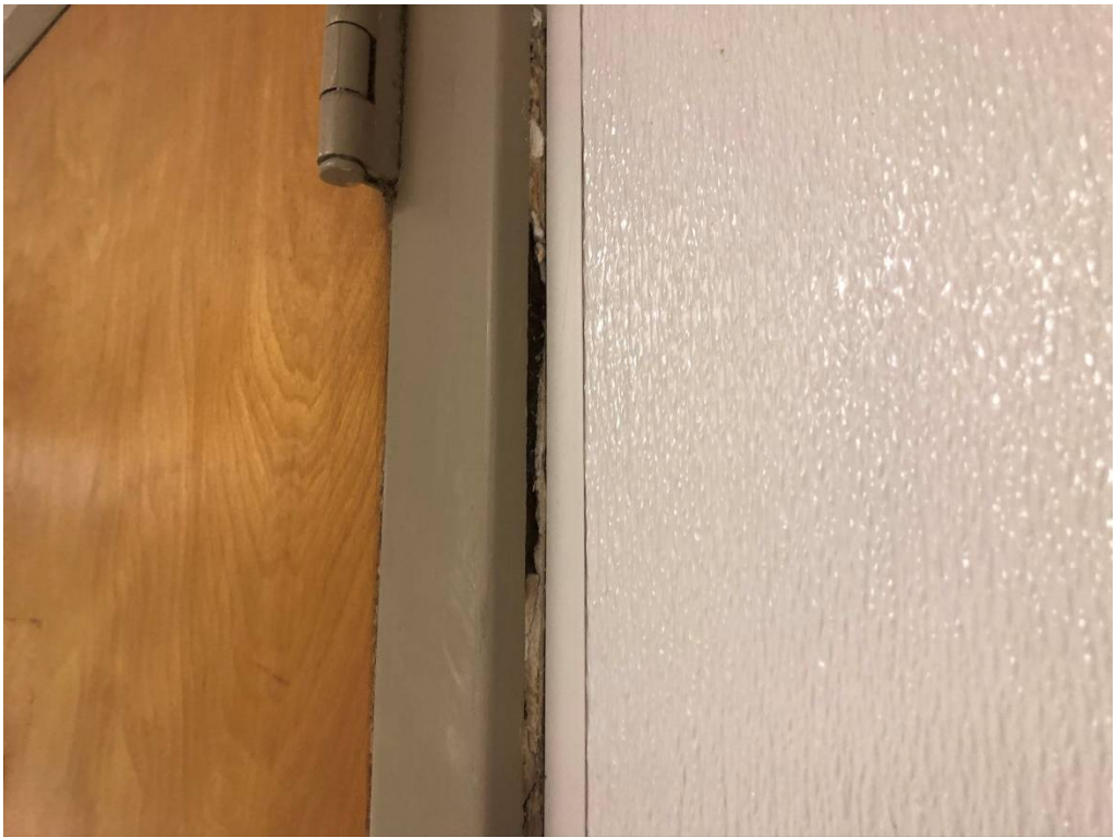
Figure 7 – Exposure at Door Jamb in Building 1 Vestibule
