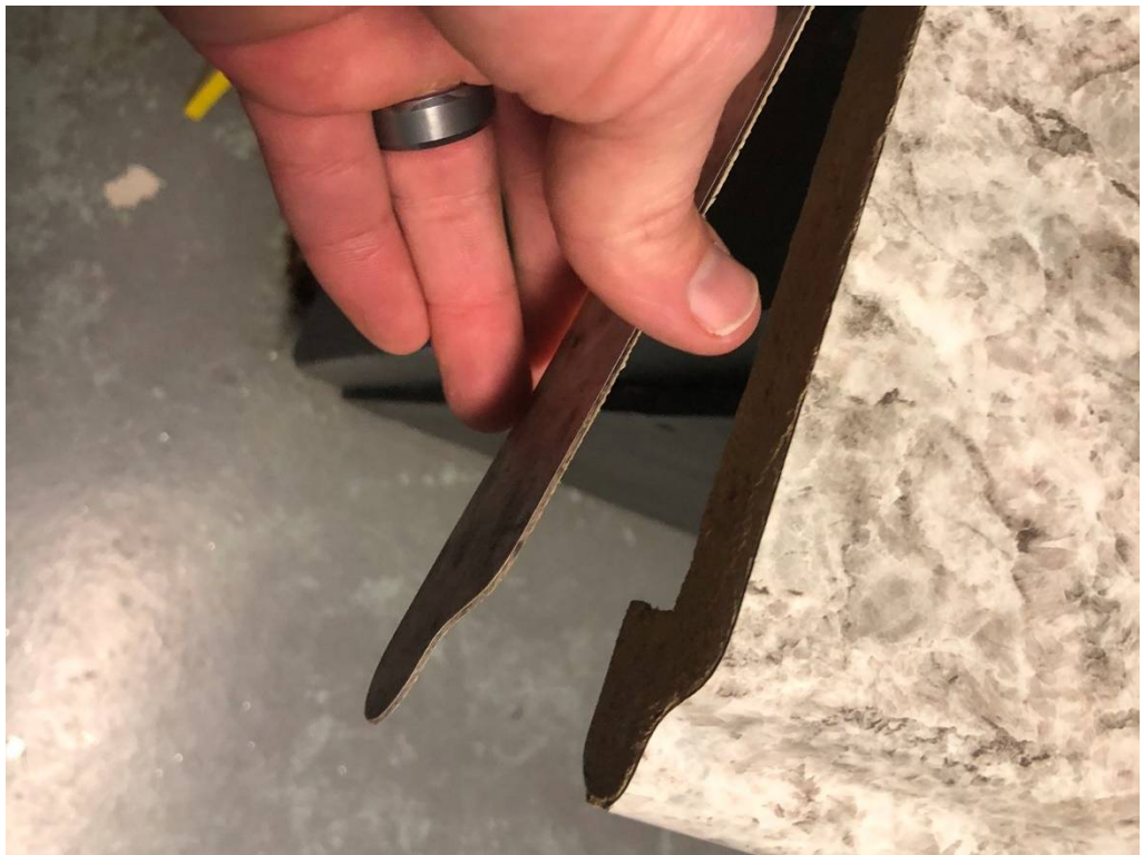
Figure 6 – Damage to New Laminate Counter
