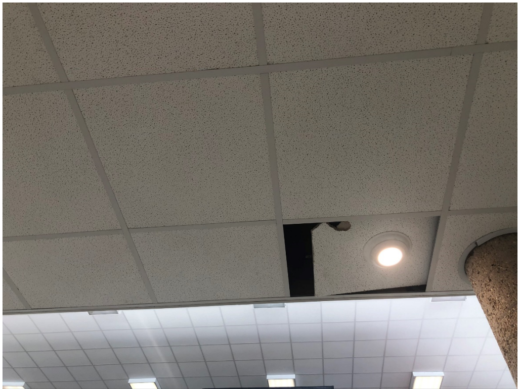
Figure 2 – Corridor in Building 1
