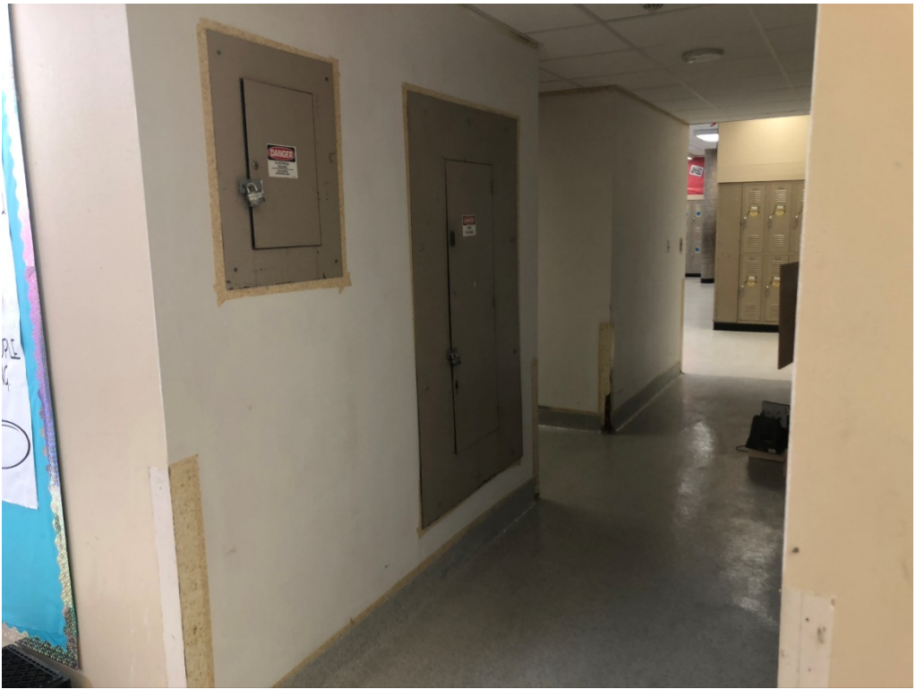
Figure 1 – Corner Guards Removed Building 3
