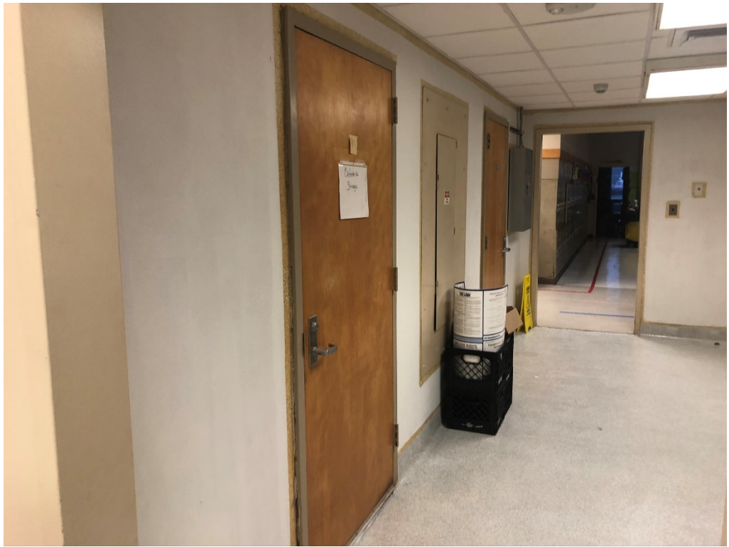
Figure 3 – Primed Panels to Received FRP @ Building 1 Vestibule
