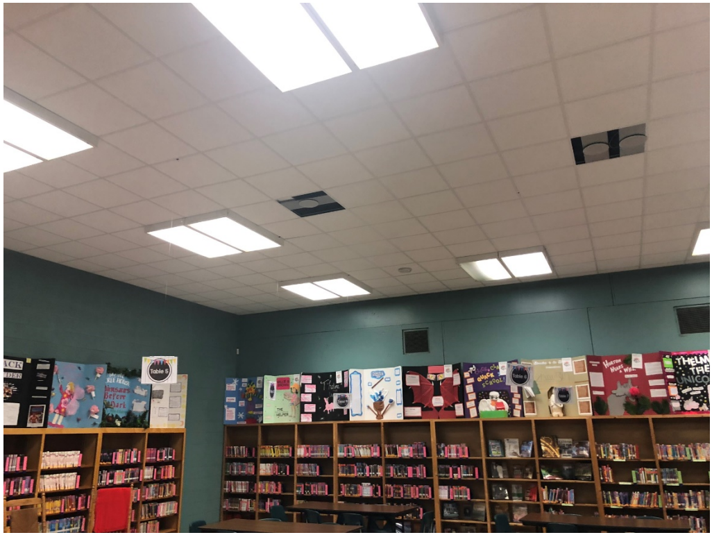
Figure 1 – Library Ceiling Installed
