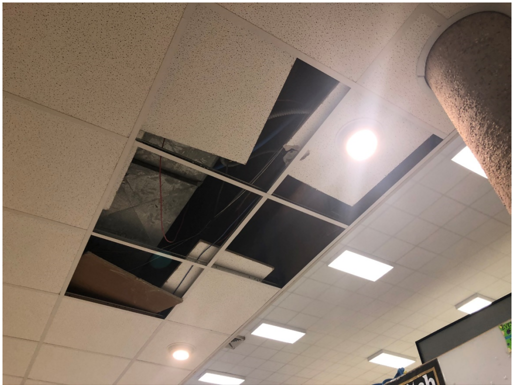
Figure 6 – Corridor in Building 1
