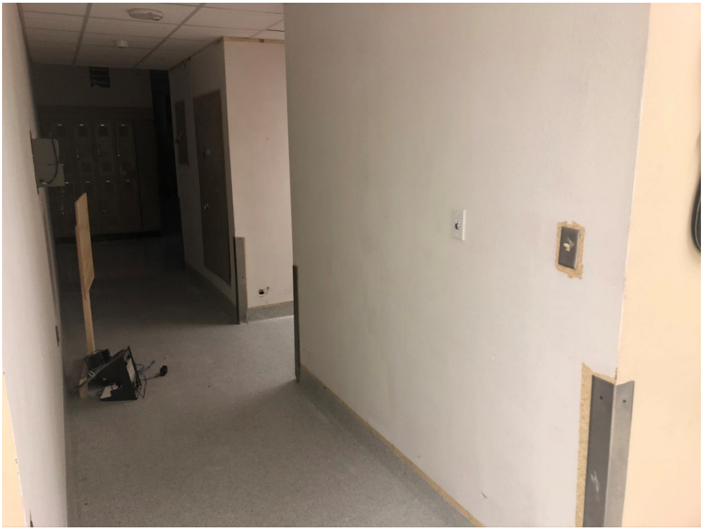
Figure 7 – Primed Panels to Received FRP @ Building 3 Vestibule
