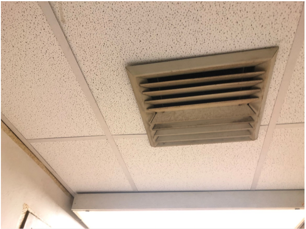
Figure 9 – Some Vents still to Paint
