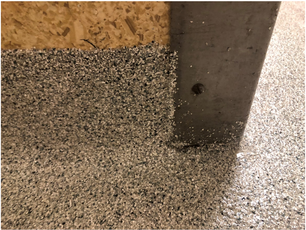
Figure 5 – Clean Required @ vertical Wall Components (typical)
