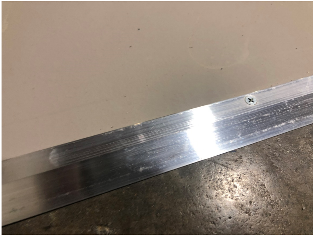
Figure 3 – Gym Floor Aluminum Threshold
