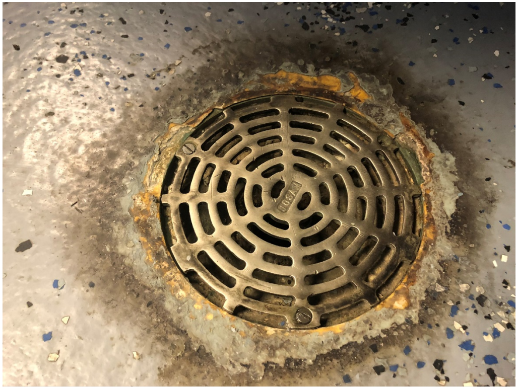
Figure 13 – Drain Grates Installed
