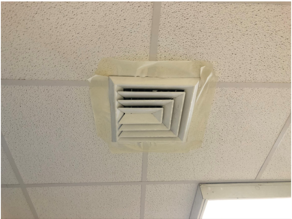
Figure 6 – Vents in the Process of RePainting
