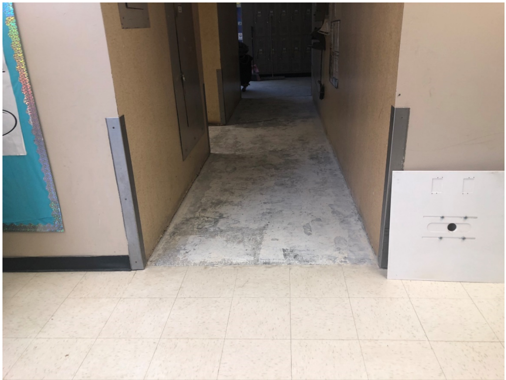
Figure 14 – Building 3 Floor Prepped for New Install
