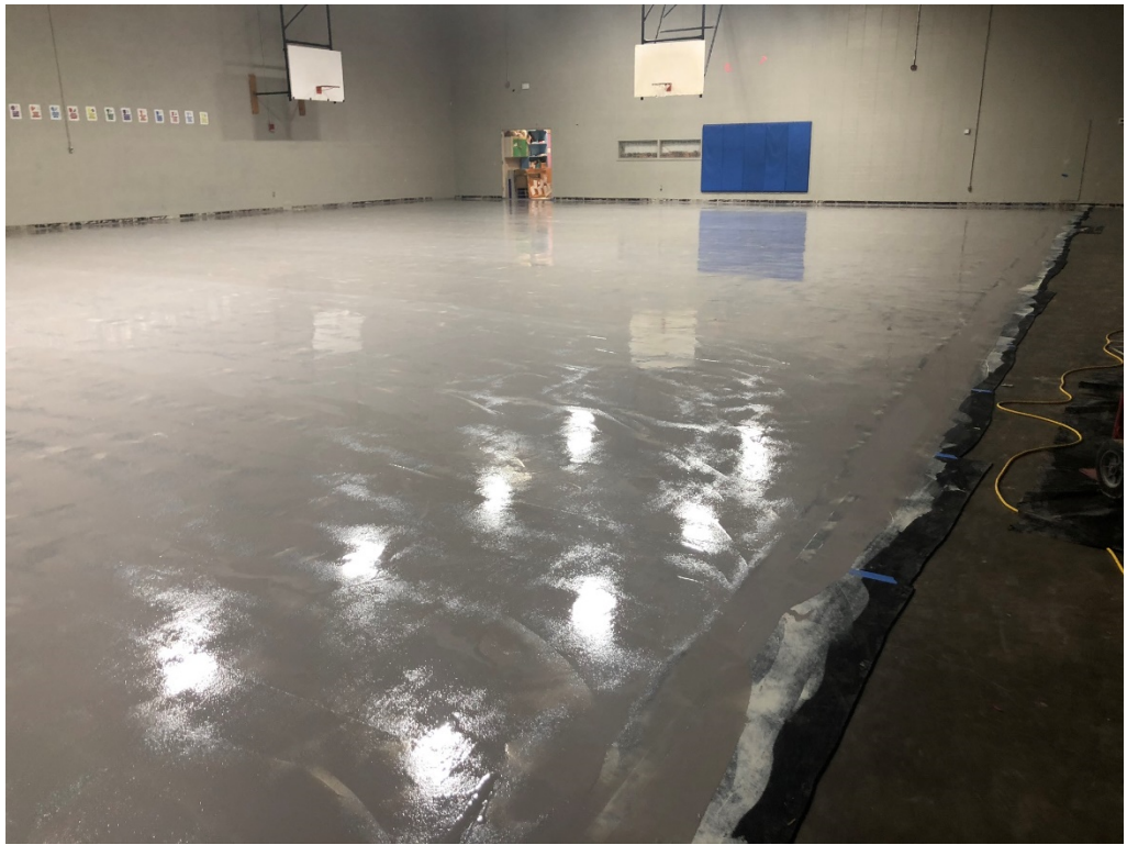
Figure 11 – Gym Floor Prime Coat
