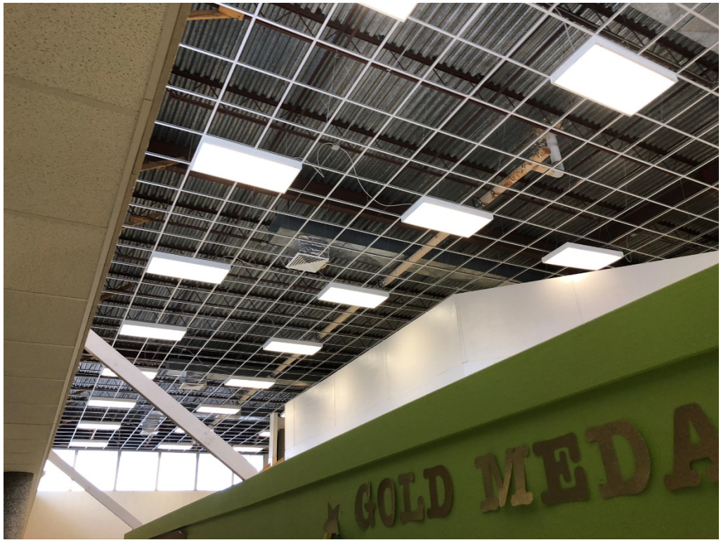
Figure 3 – Building 3 High Ceilings
