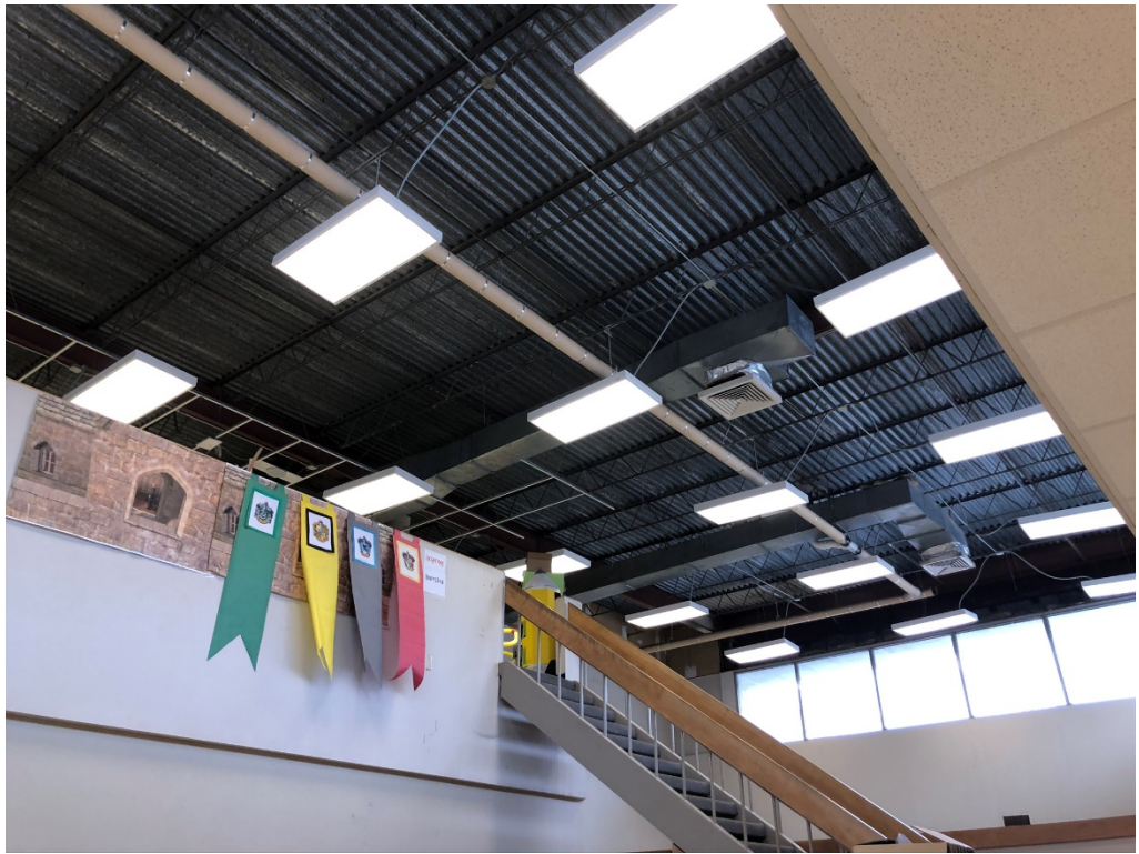
Figure 5 – Building 1 High Ceilings
