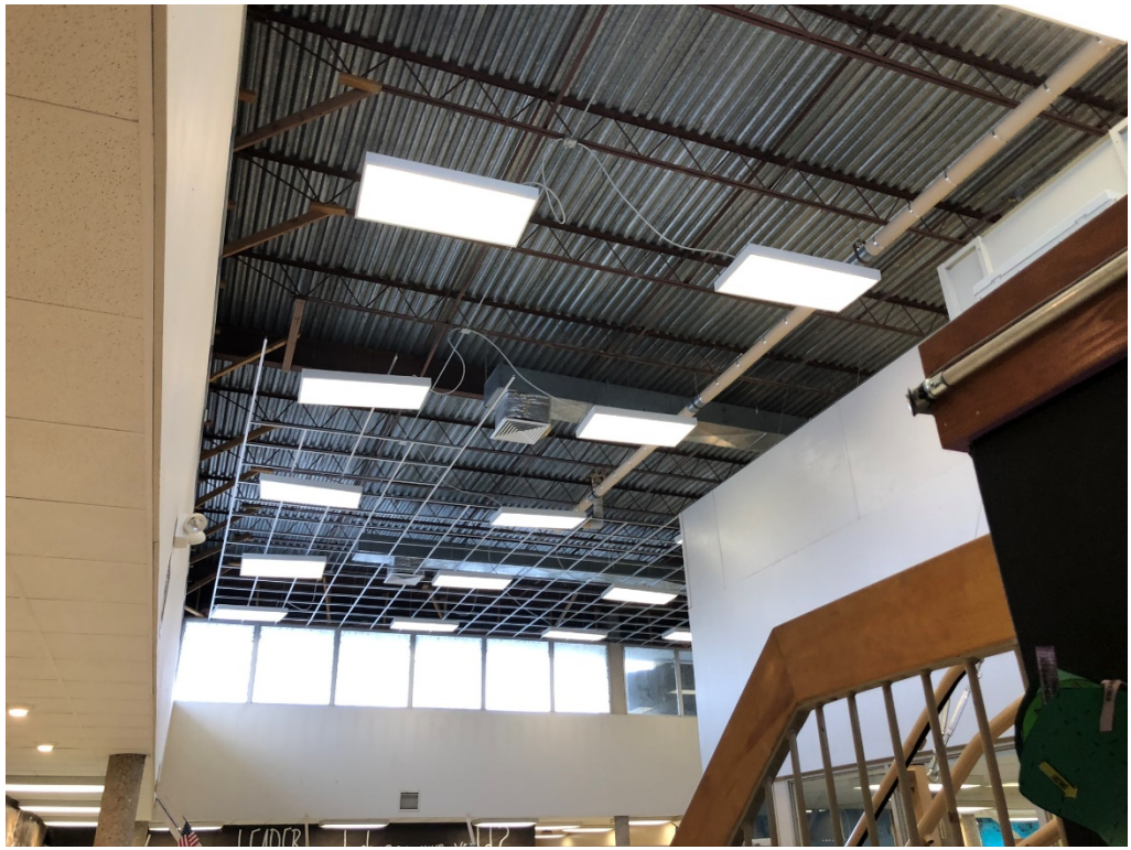
Figure 1 – Building 3 High Ceilings
