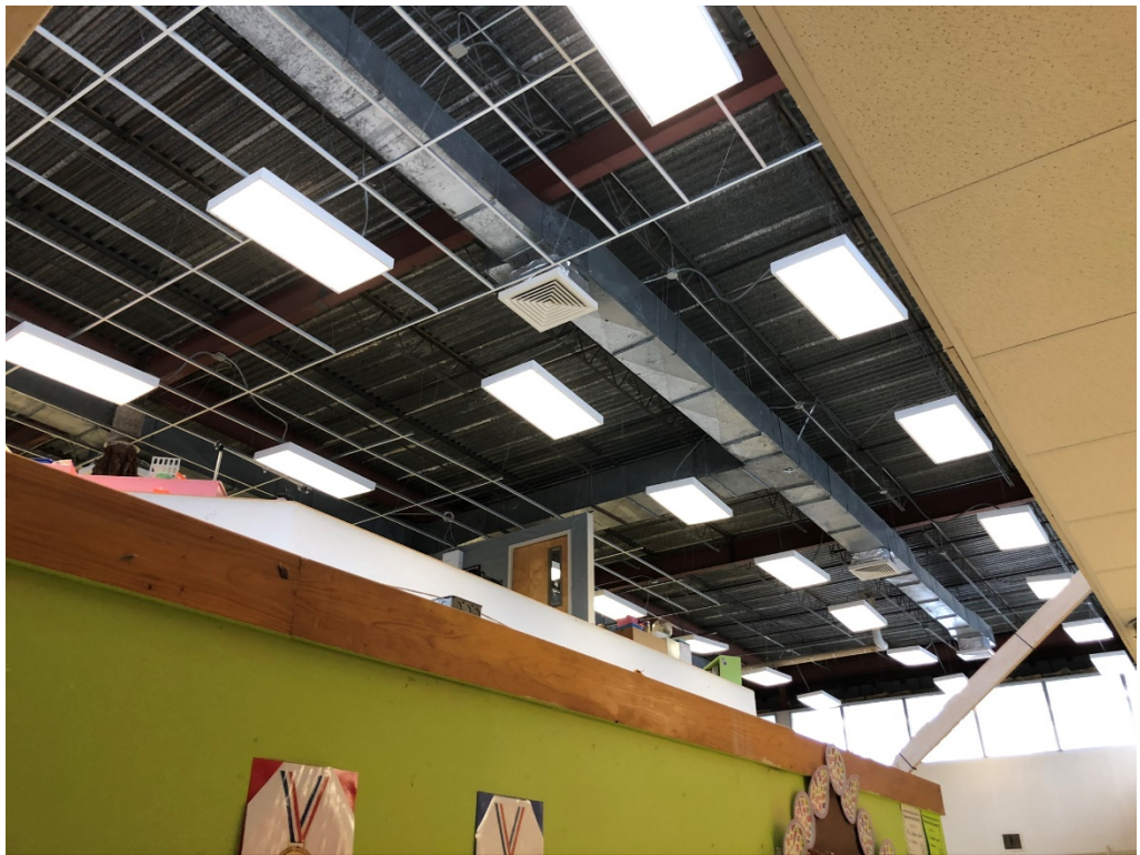
Figure 4 – Building 1 High Ceilings
