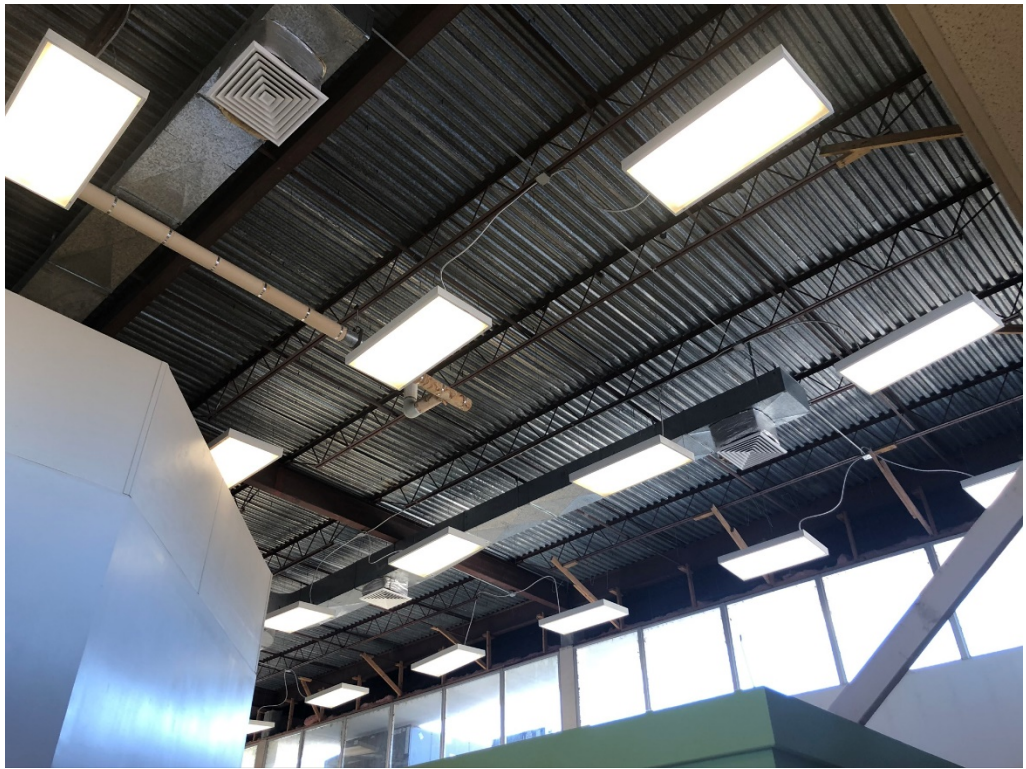
Figure 7 – Building 3 (grid removed)
