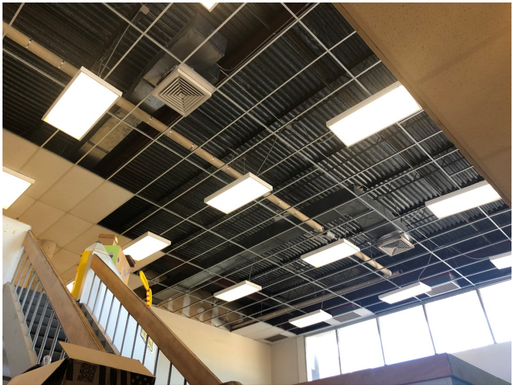
Figure 4 – Building 1 Tile Removed
