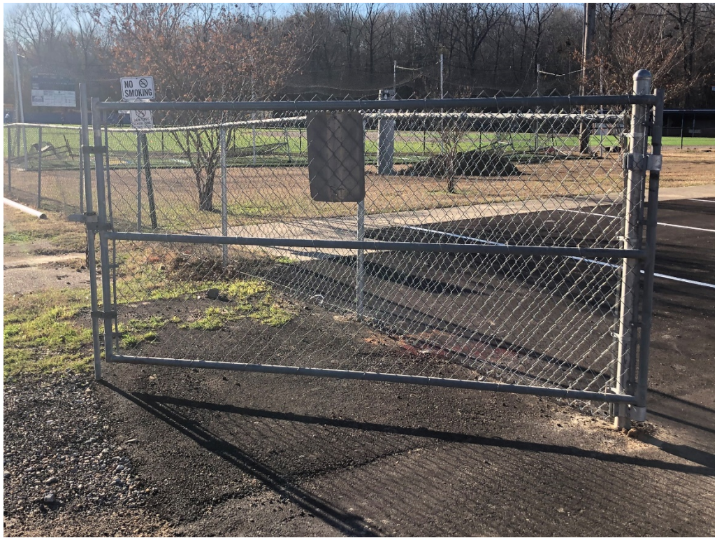
Figure 9 – Double Gate Re-Installed
