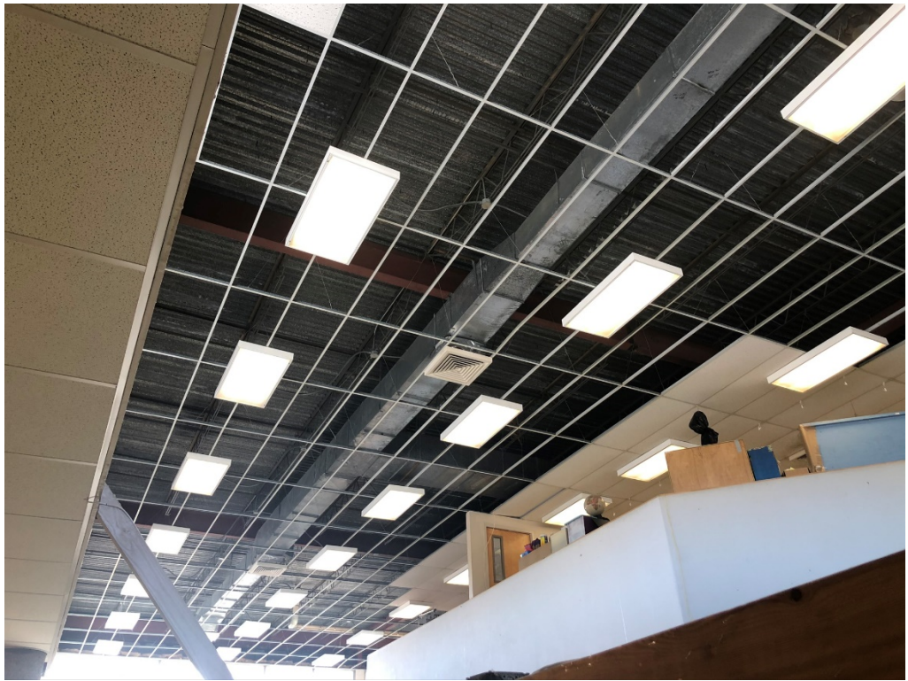
Figure 5 – Building 1 Tile Removed
