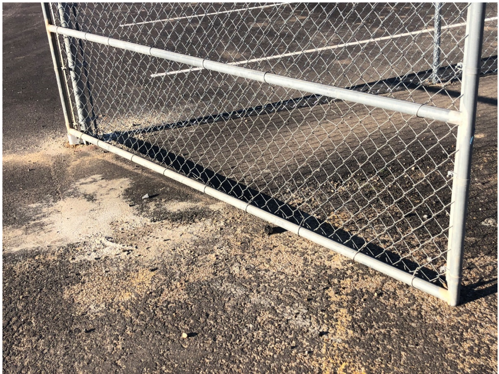
Figure 10 – Double Gate Re-Installed
