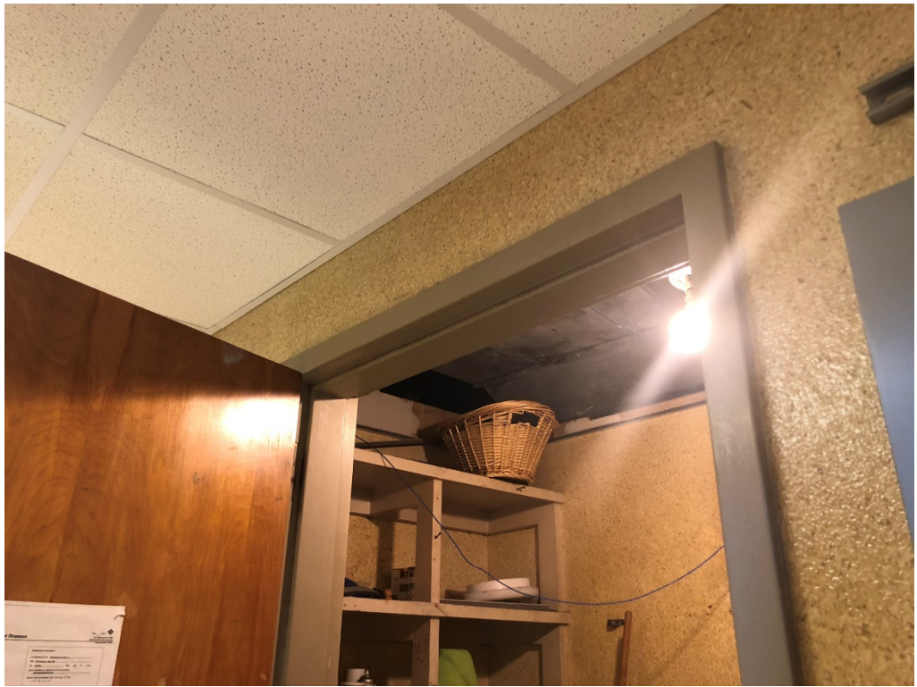
Figure 3 – Janitor Room @ 100D in building 1 (no ACT)
