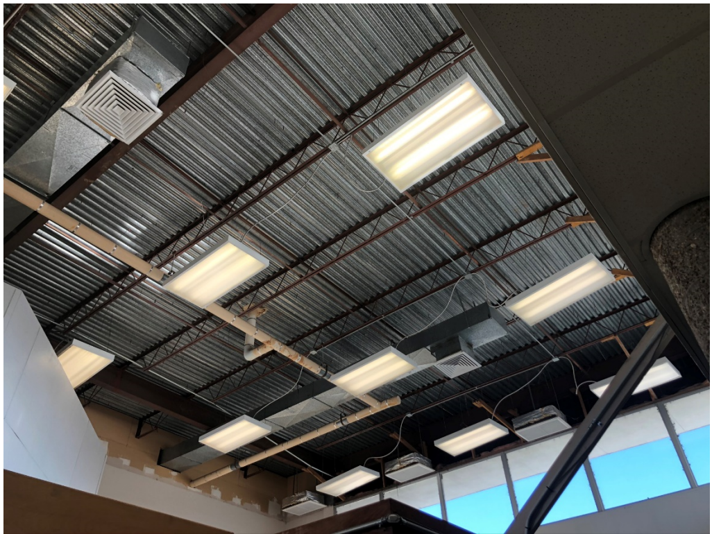
Figure 8 – Building 3 (grid removed)
