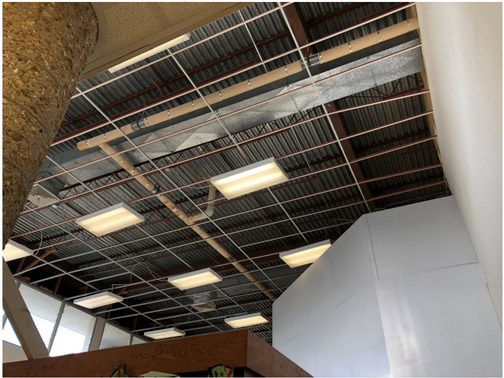
Figure 1 – Building 3 Corridor Demo
