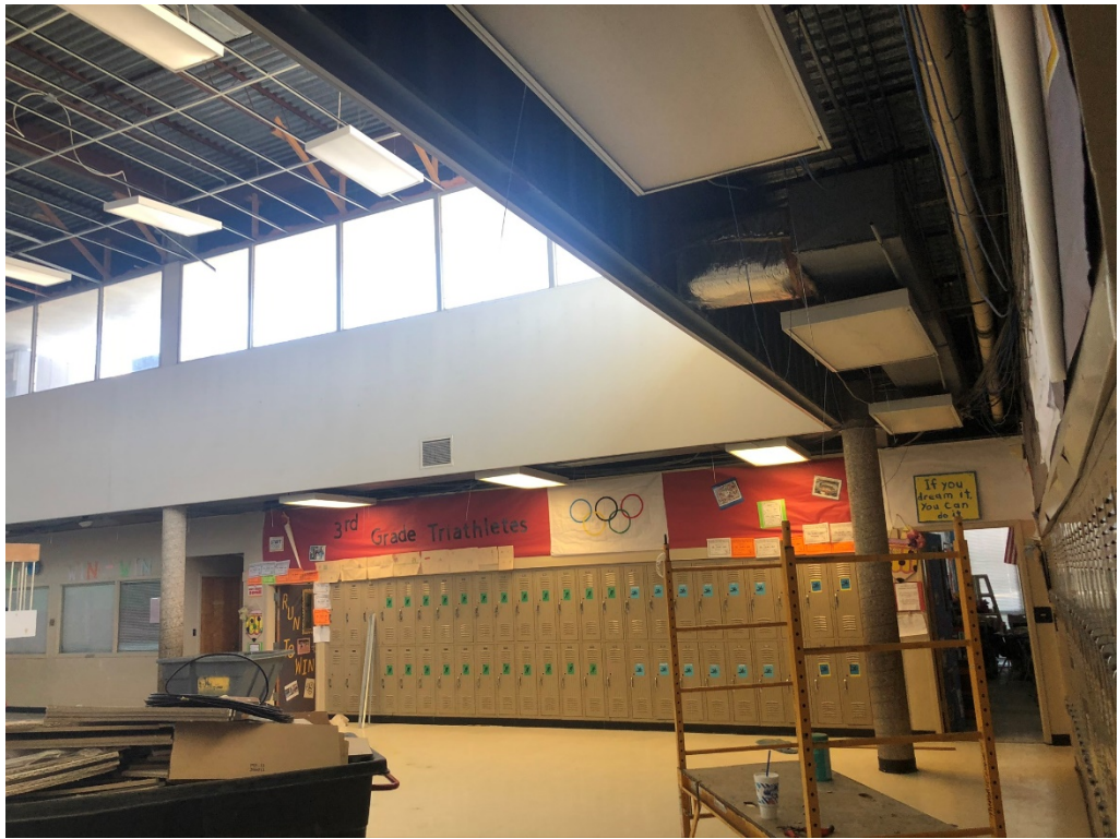
Figure 1 – Building 3 Corridor Demo
