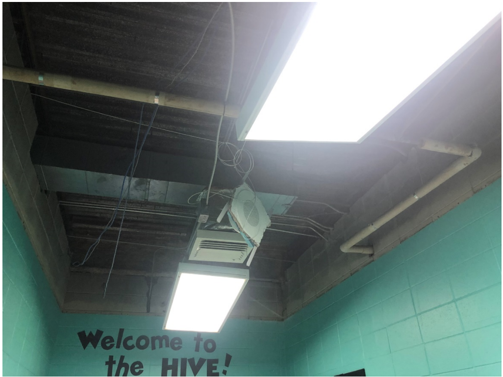
Figure 5 – Building 2 Ceiling Demo
