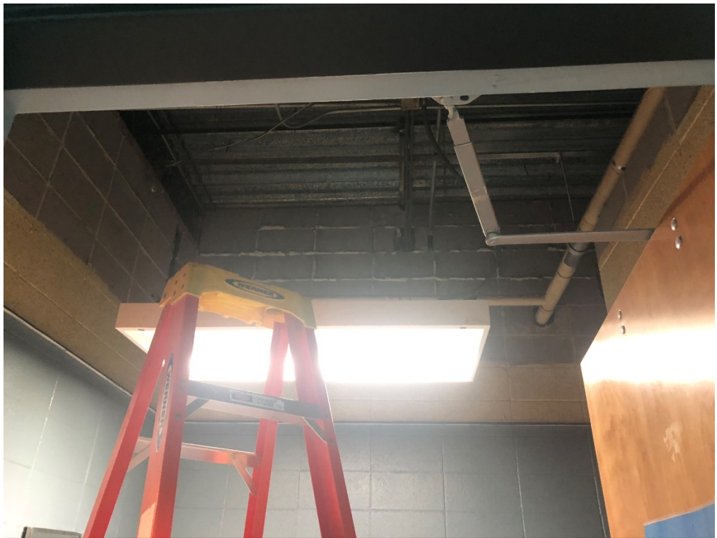
Figure 6 – Building 2 Ceiling Demo
