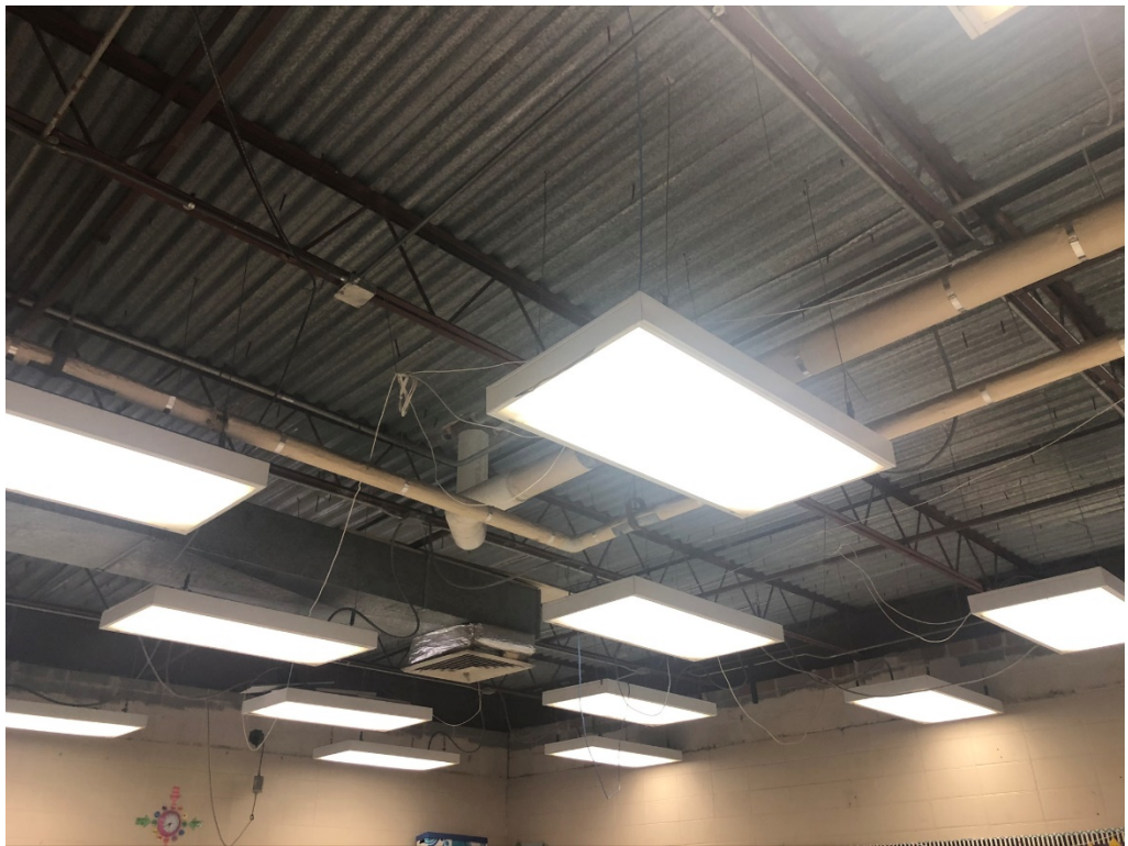
Figure 8 – Typical Demo in Building 3
