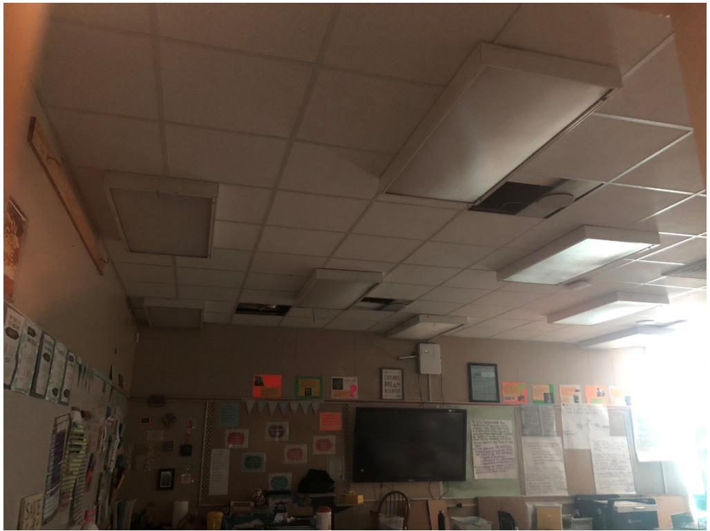
Figure 9 – Typical Finished Ceiling in Building 3
