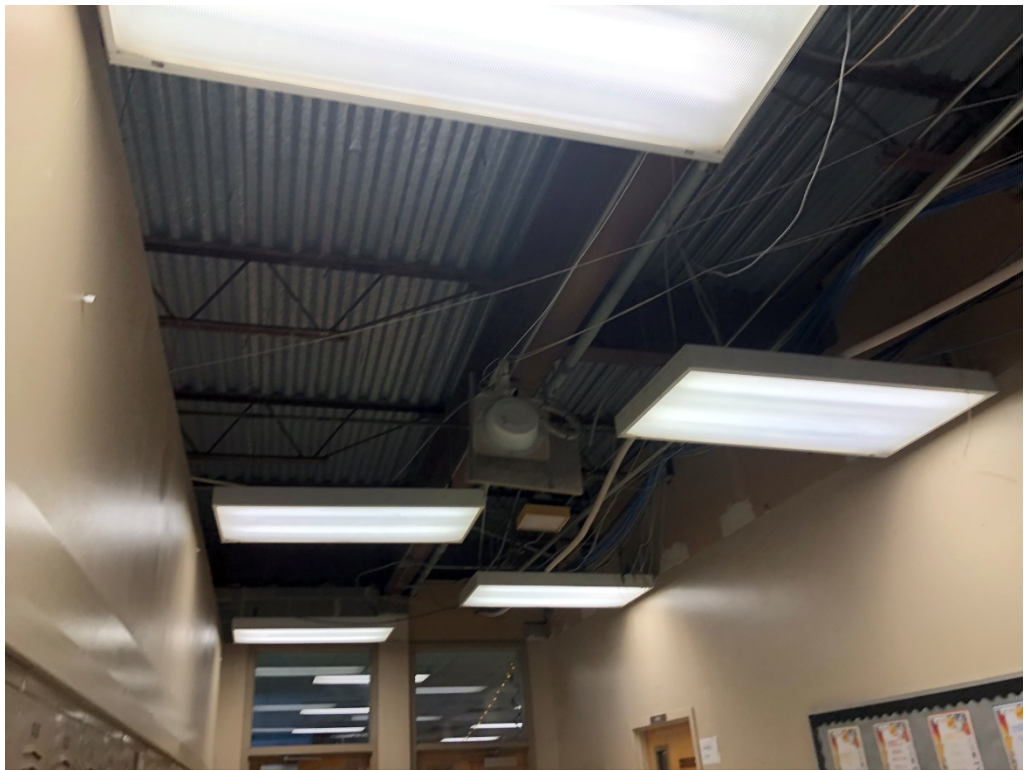
Figure 6 – Building 3 Corridor Demolition
