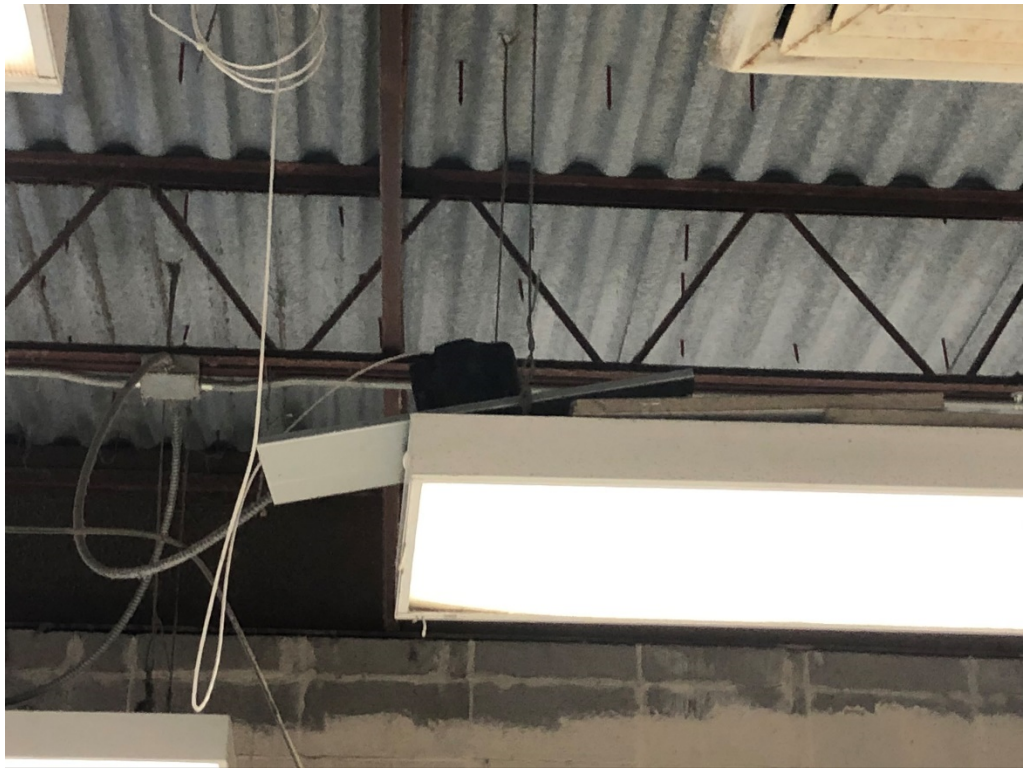
Figure 5 – Speakers Exist Prior to Reinstallation of Grid & Tile
