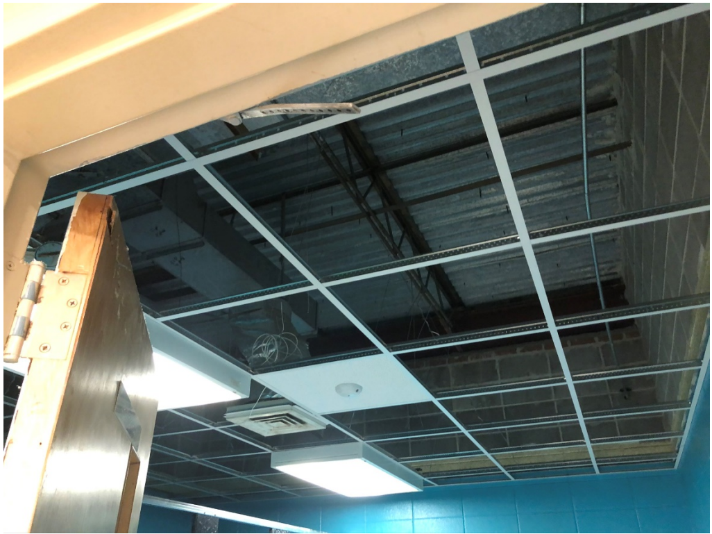
Figure 1 – Grid in Restrooms
