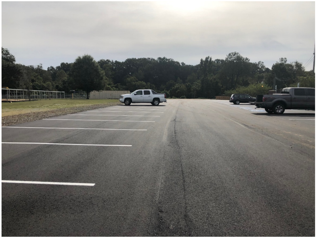
Figure 3 – Center Parking Looking SE
