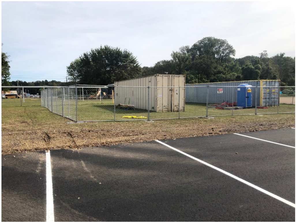
Figure 5 – Temp Fencing is Up
