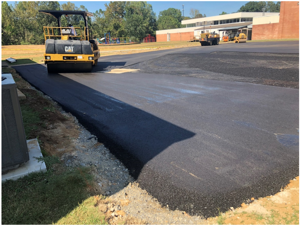
Figure 7 – Top Layer at West Corner
