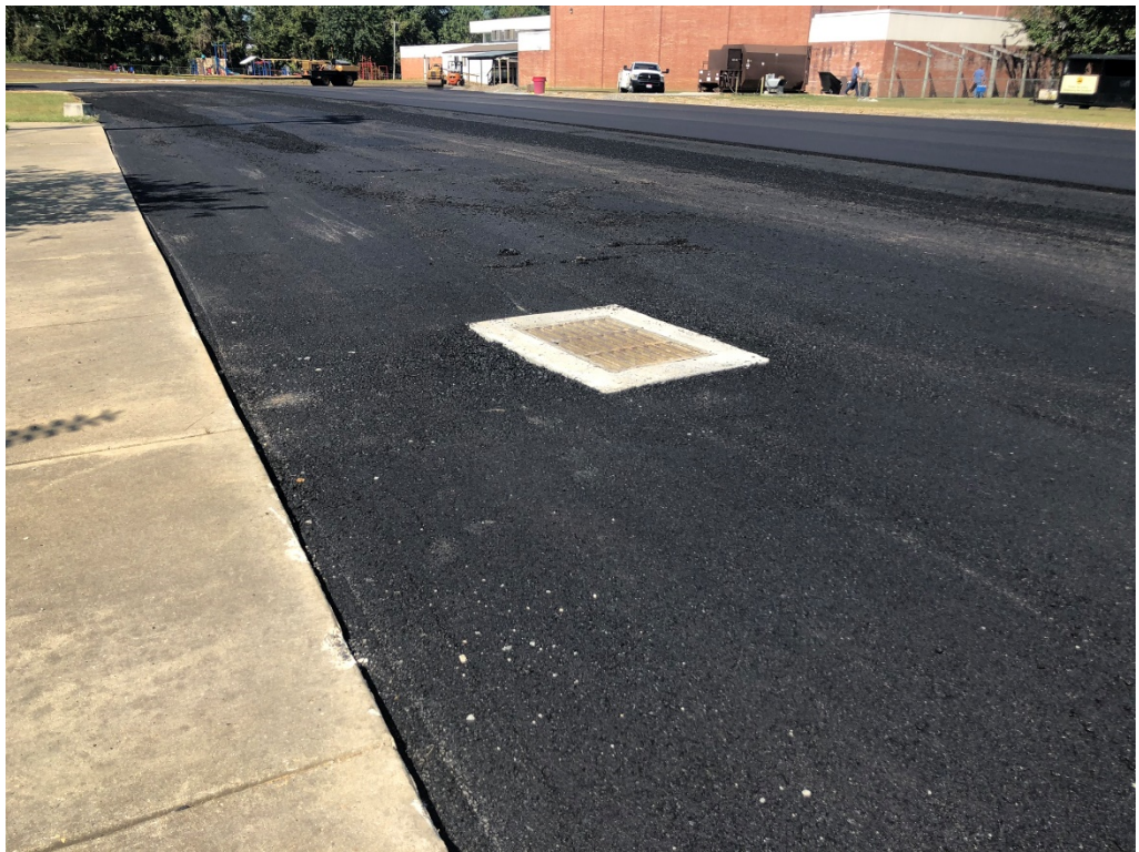
Figure 6 – Base Layer Even with Concrete Drain
