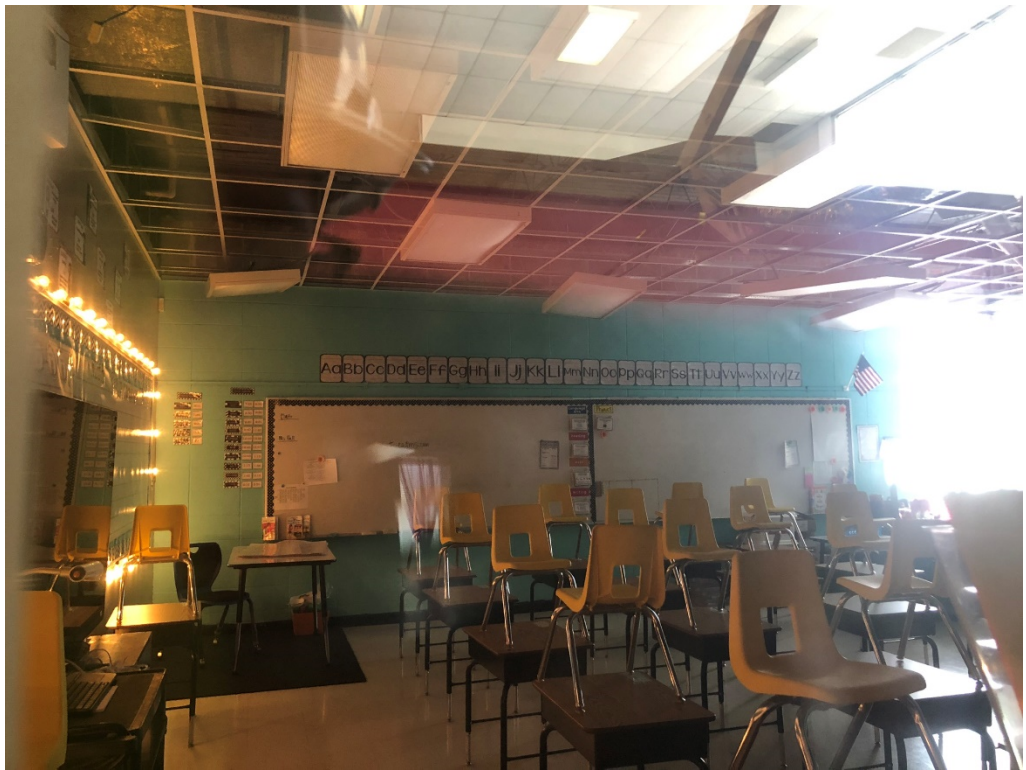
Figure 16 – West Corner of Building 1 – 3 rd Class
