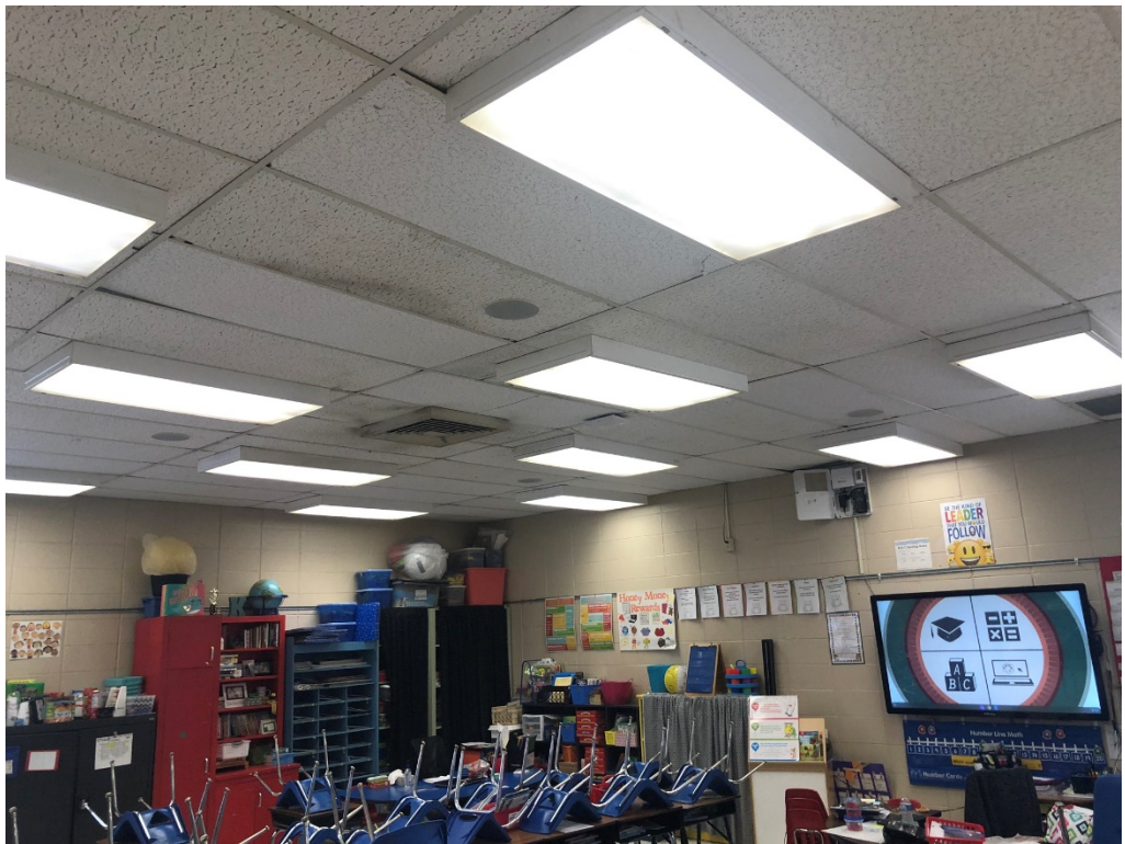
Figure 26 – North Corner of Building 1 – 11 th Class
