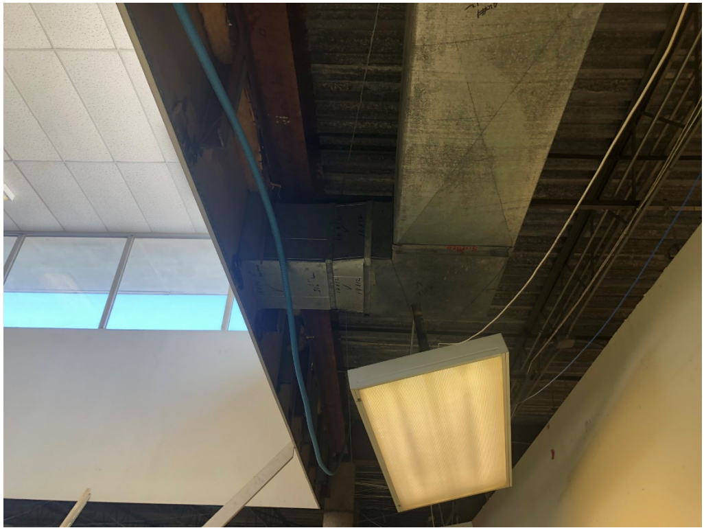
Figure 21 – East Corner of Building 1 Hall Area
