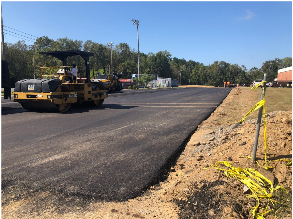
Figure 2 – East Corner Looking West
