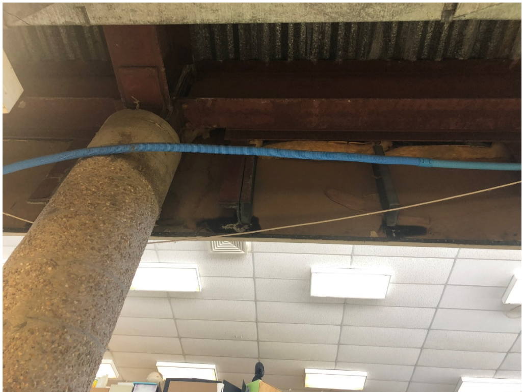
Figure 22 – Existing Furr Down Structure (Typical)
