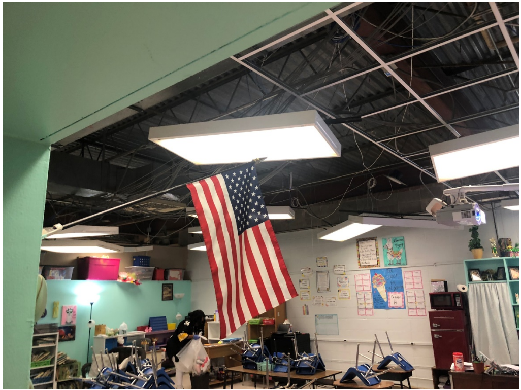
Figure 27 – North Corner of Building 1 – 12 th Class
