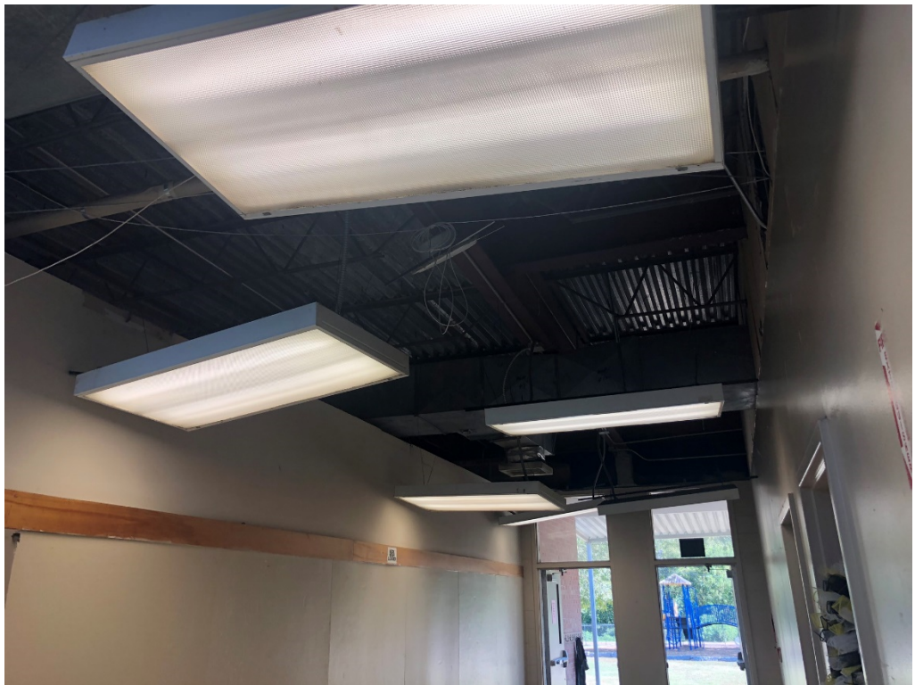
Figure 20 – Entry from Southeast Side of Building 1
