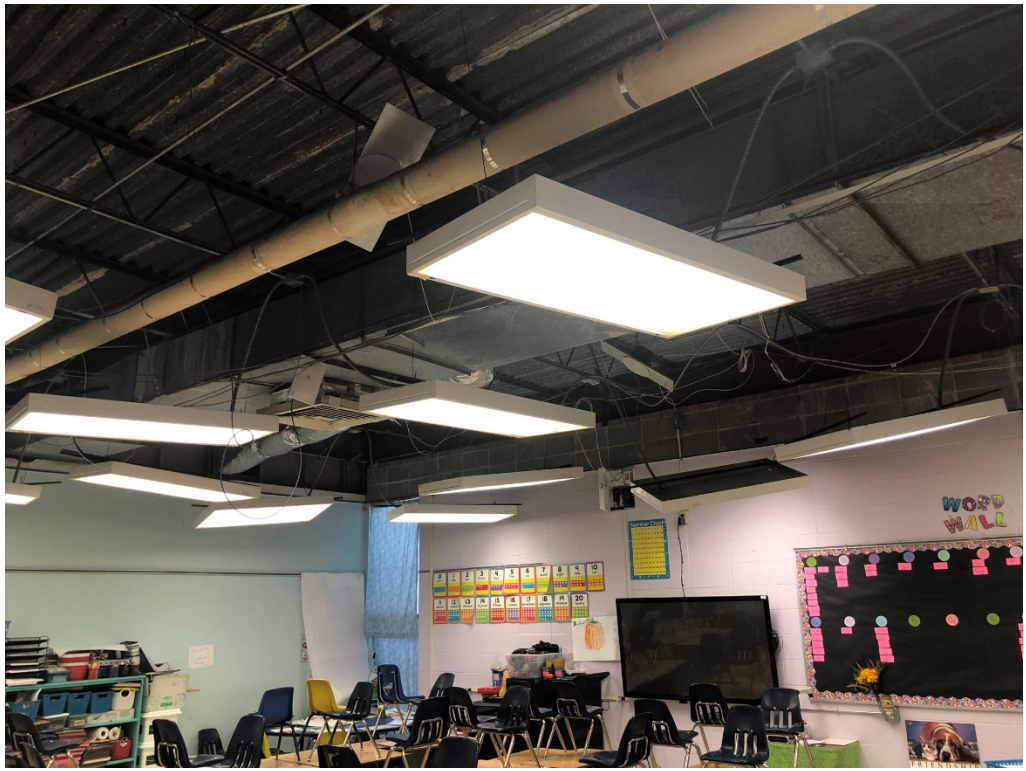
Figure 25 – North Corner of Building 1 – 10 th Class
