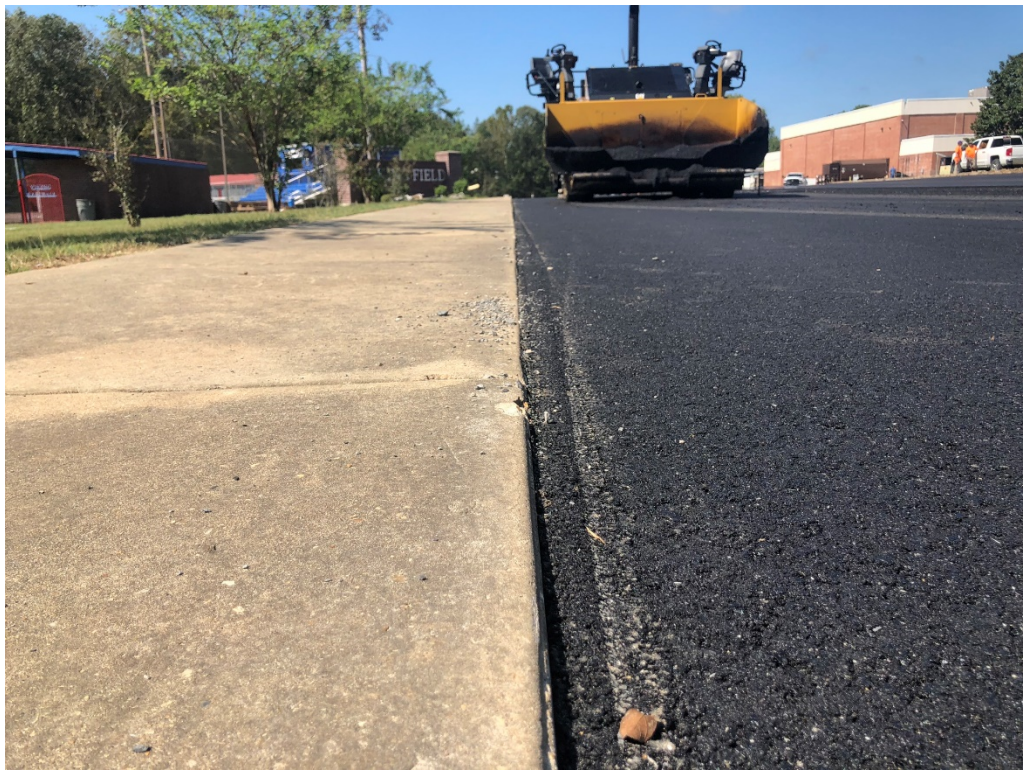
Figure 4 – Base Asphalt Paving Layer
