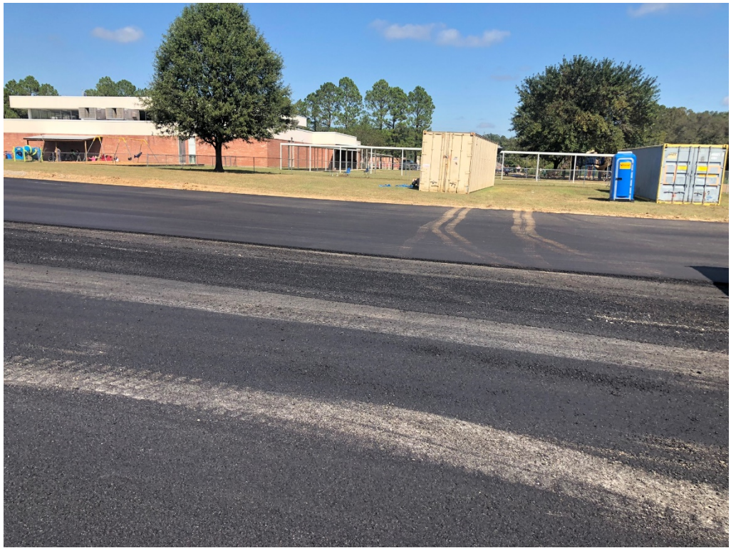
Figure 5 – Top Layer and Base Layer Asphalt
