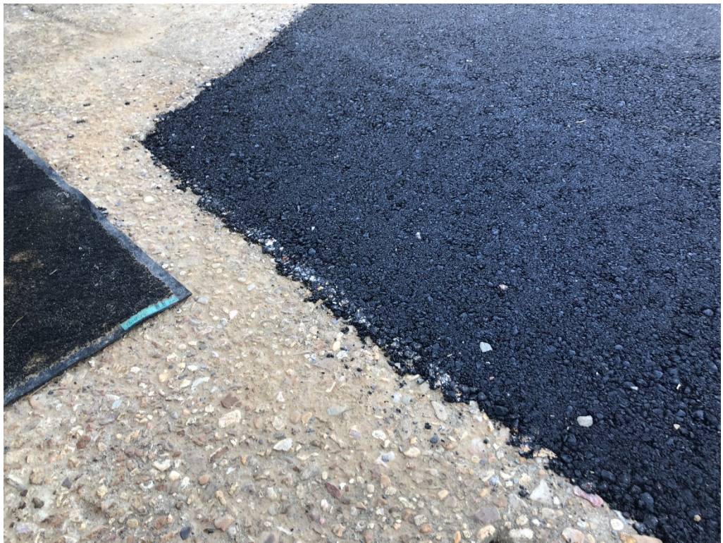
Figure 8 – Top Layer Even with Sidewalk
