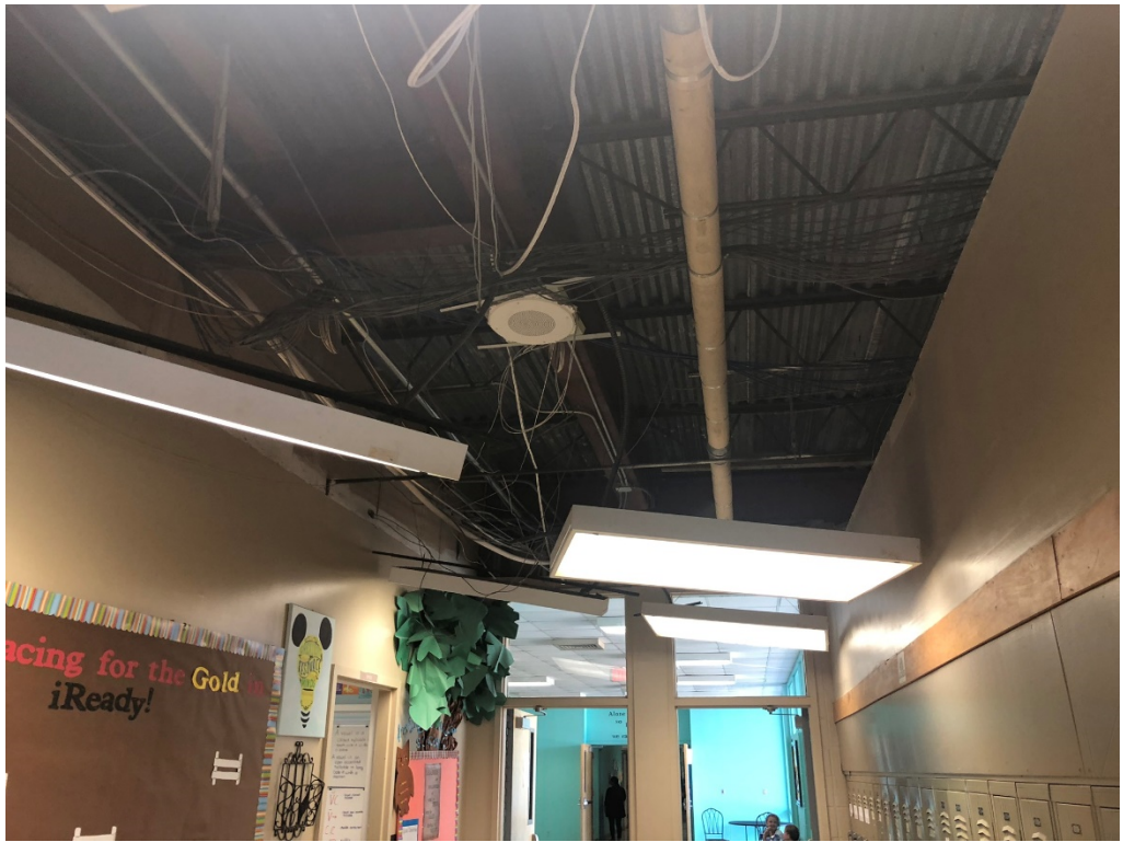
Figure 29 – North Corner of Building 1 – Entry Hall from Interior
