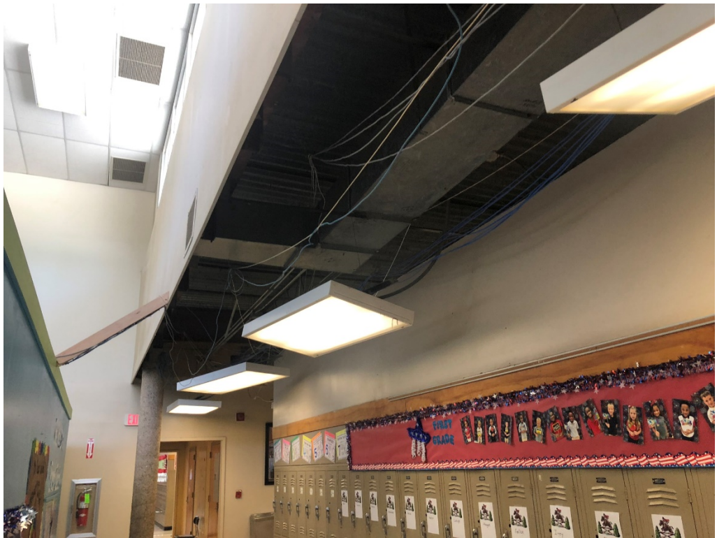
Figure 28 – North Corner of Building 1 – Hall Area
