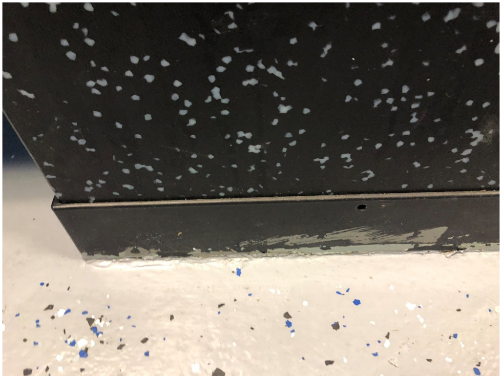
Figure 24 – Paint on Partitions
