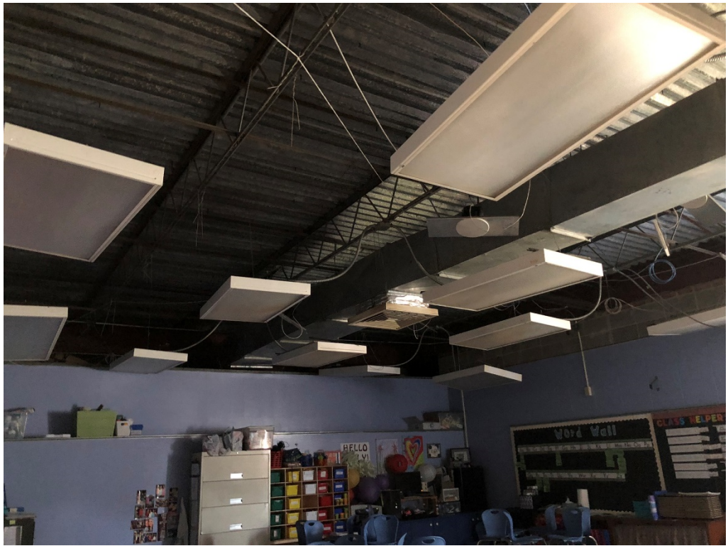
Figure 19 – Classroom Ceiling Demo
