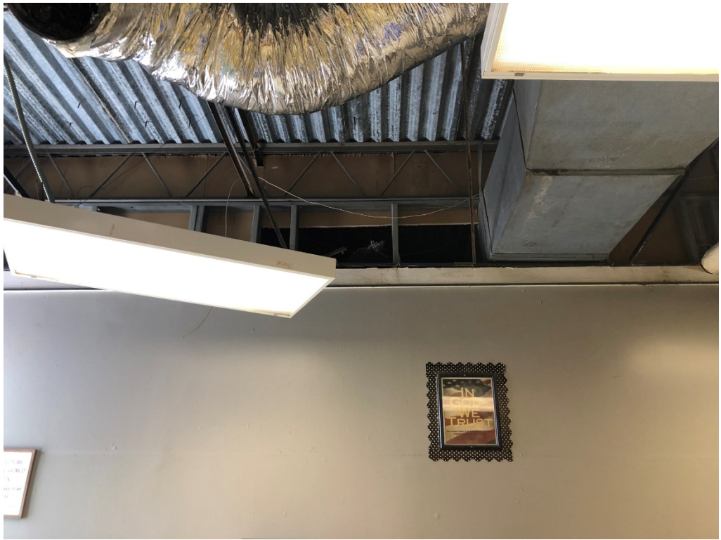
Figure 13 – Example of Opening in Upper Walls
