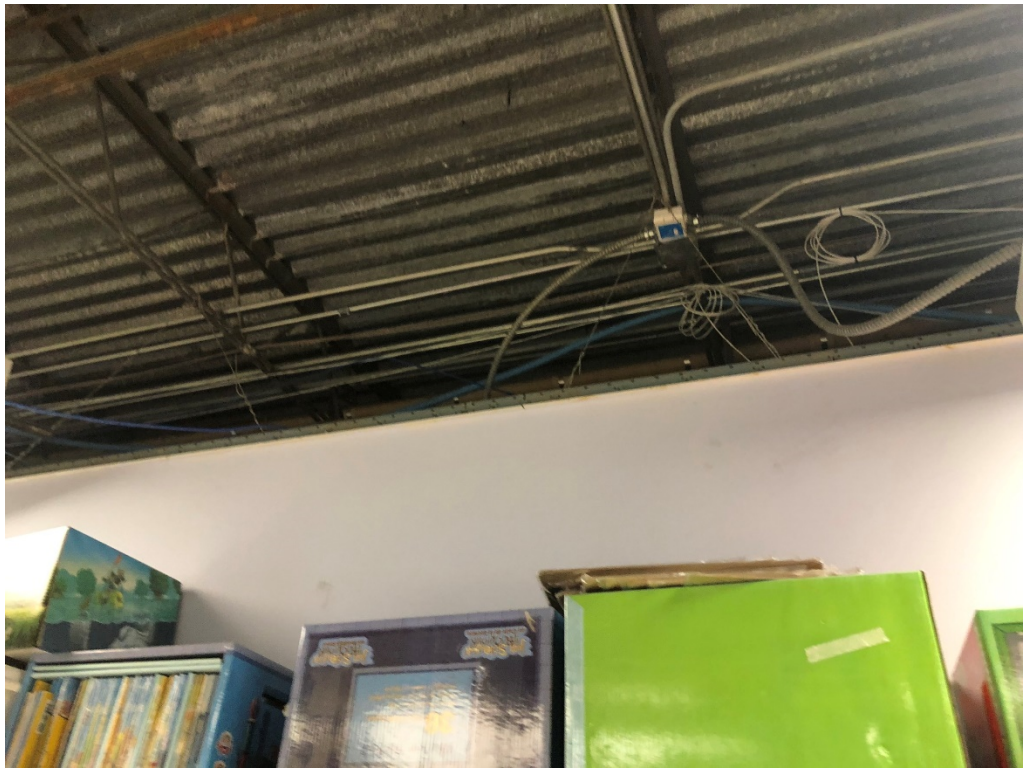
Figure 21 – Example of Typical Short Wall Opening to Furr Down in Main Space
