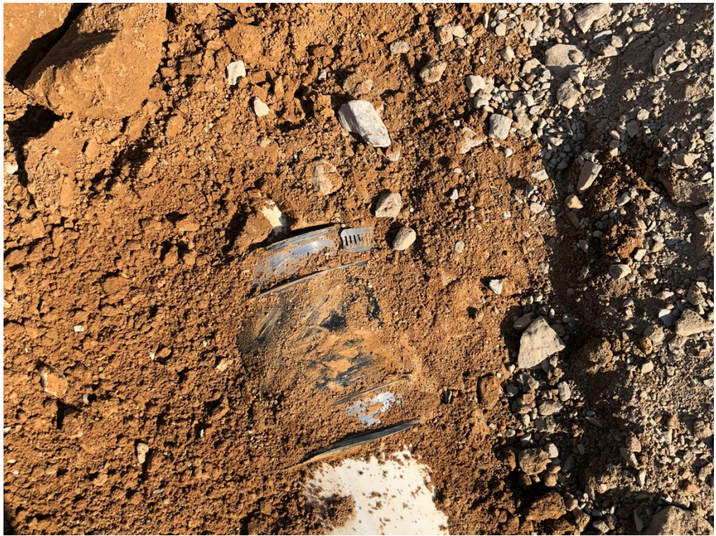
Figure 29 – Example of Repair between Thin Wall Pipe to SHC 40 PVC
