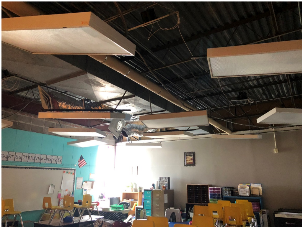
Figure 10 – Example of Demoad Ceiling
