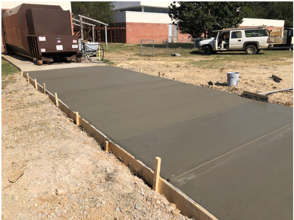
Figure 8 – Dumpster Pad Installed with Control Joints
