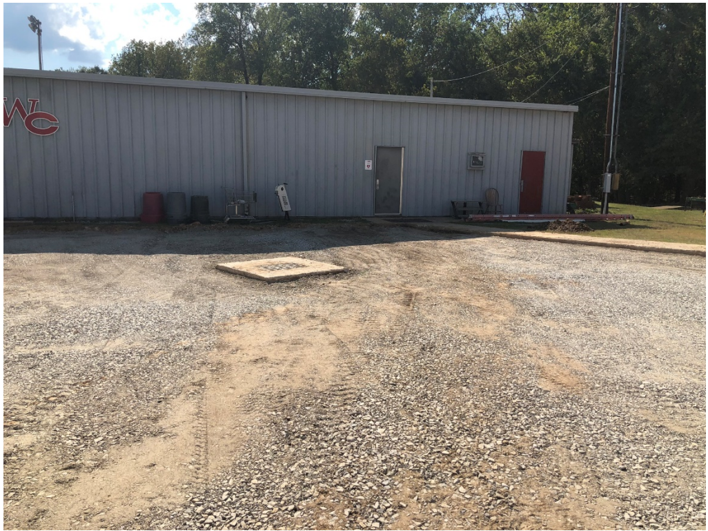
Figure 7 – Area that Sewer was Damaged and Replaced
