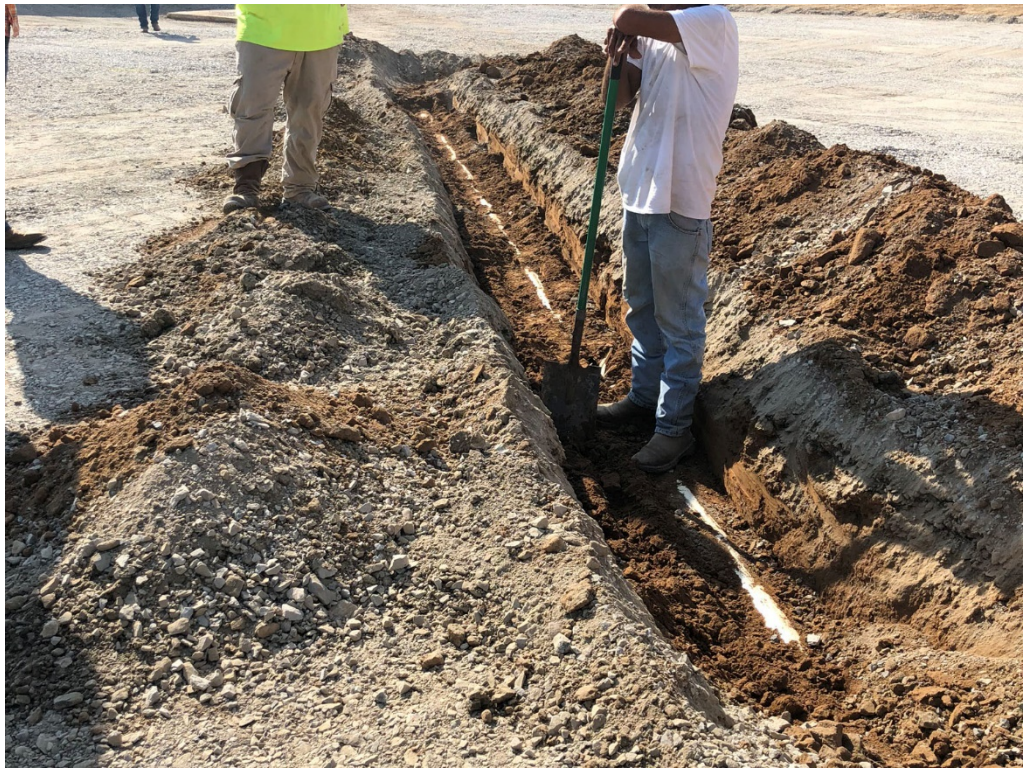
Figure 27 – Excavation of Thin Wall Pipe
