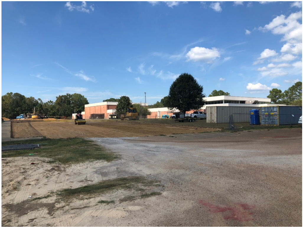
Figure 1 – Parking Area Compaction Work
