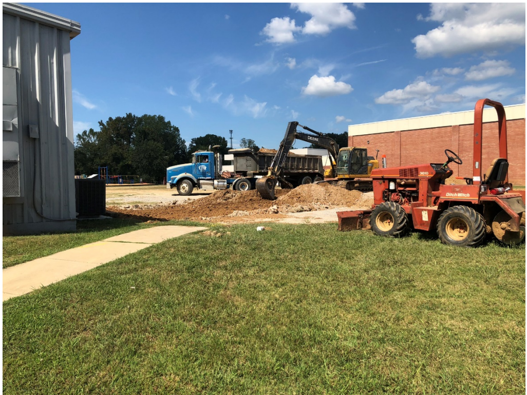
Figure 2 – Parking Area Digging Work
