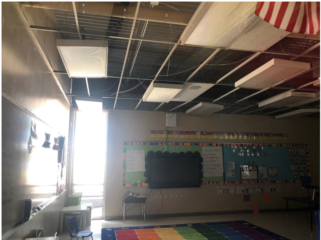
Figure 4 – Removed Ceiling Tile, Typical Demo Performed in 5 Rooms
