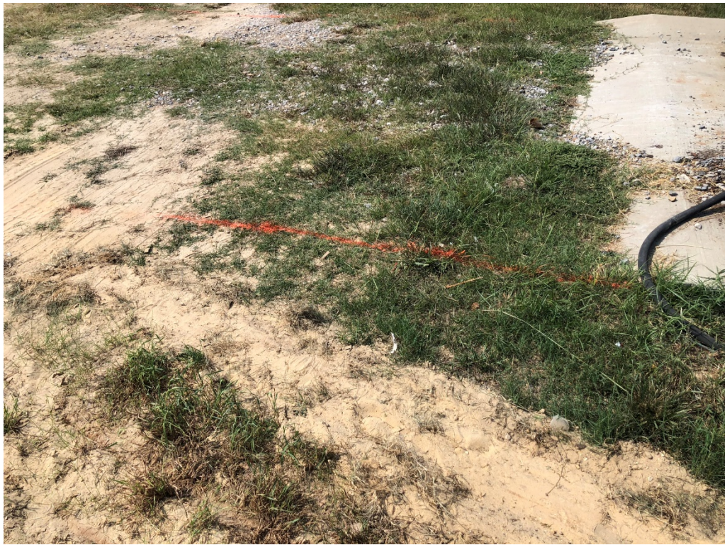
Figure 3 – Area Lined Out For Compacter Concrete Slab
