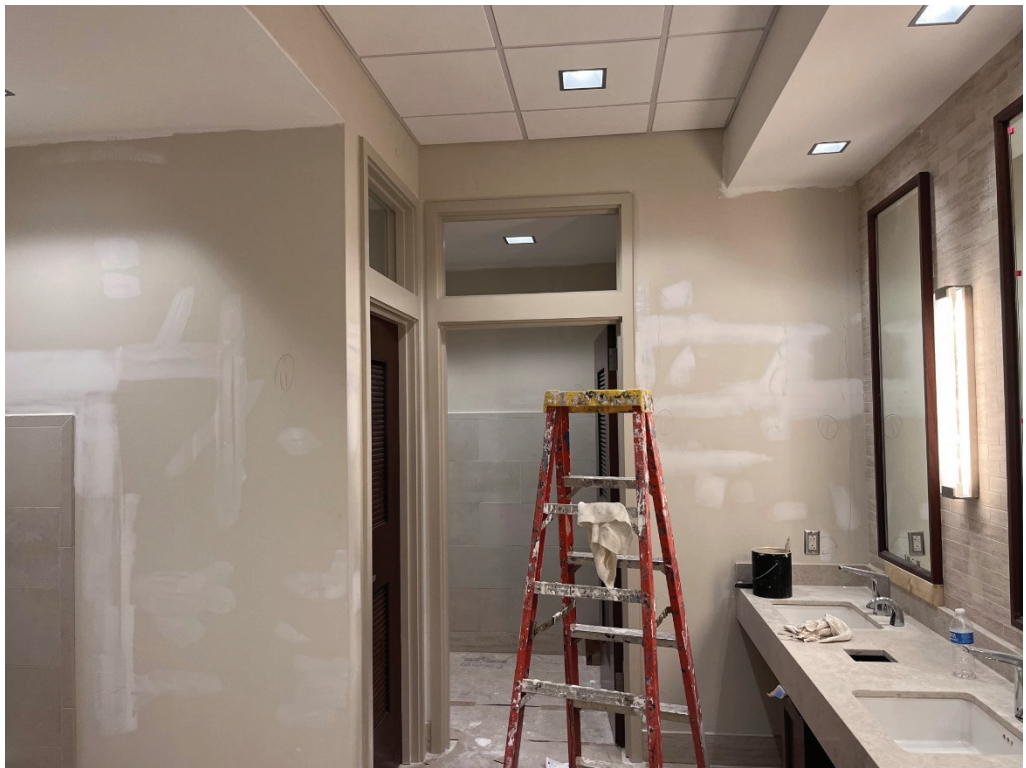
Figure 12 – Progress in First Floor Toilet Rooms
