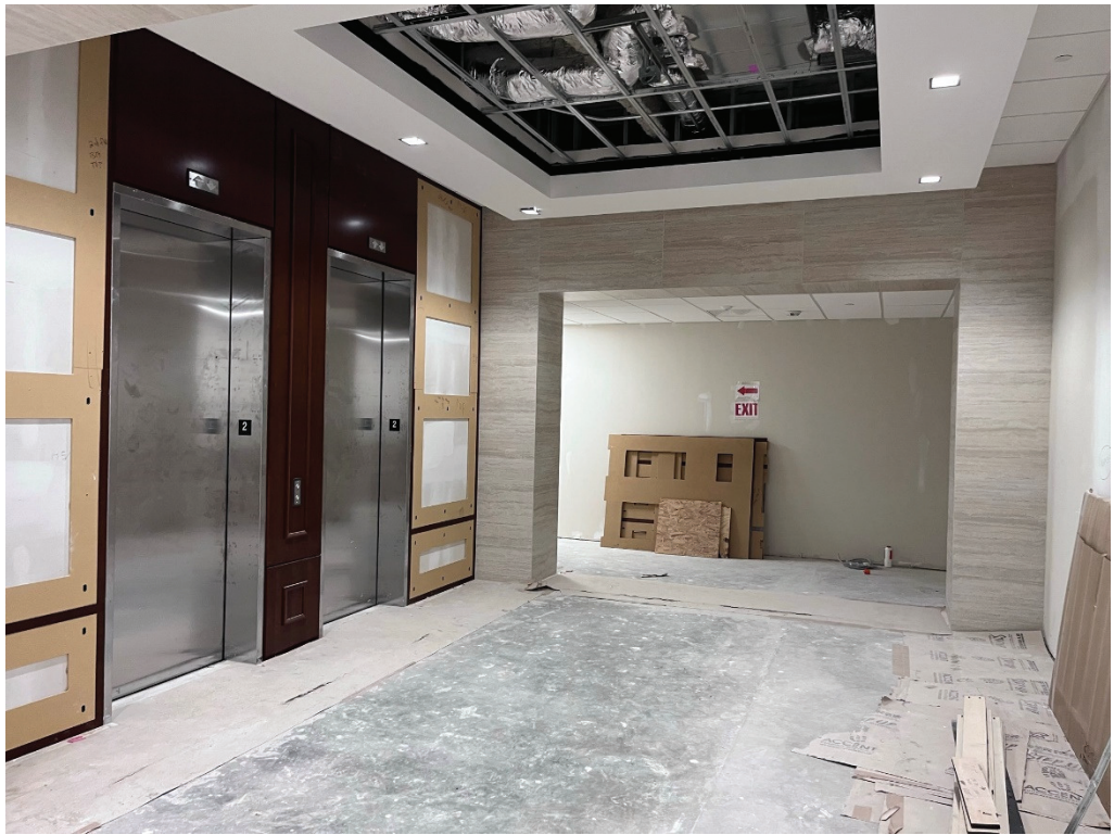
Figure 15 – 2 nd Floor Shared Space Ceilings Installed
