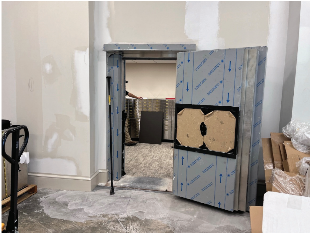
Figure 11 – Workers were present at Vault
