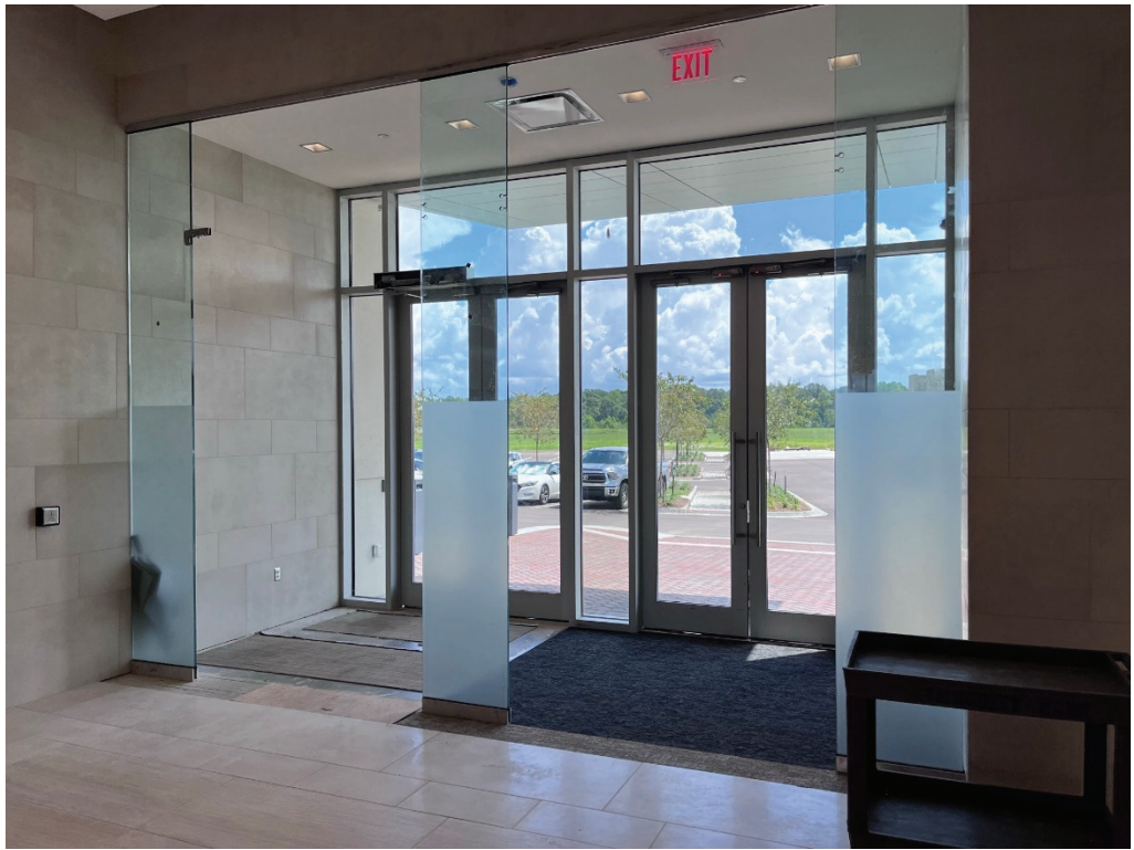
Figure 1 – 1 st Floor Entry Progress
