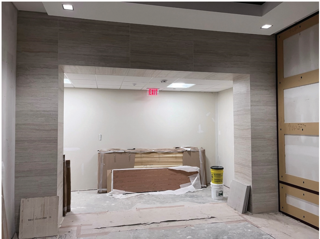
Figure 14 – 2 nd Floor Shared Space Ceilings Installed
