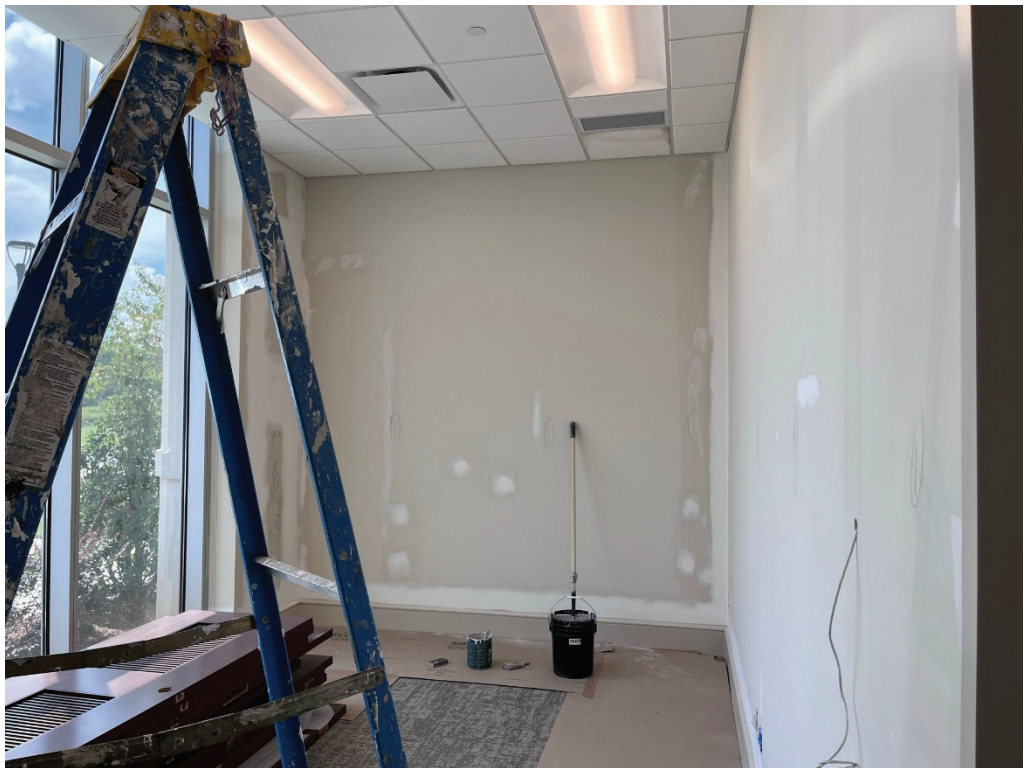
Figure 4 – 1 st Floor East Offices prepared for Wall Coverings
