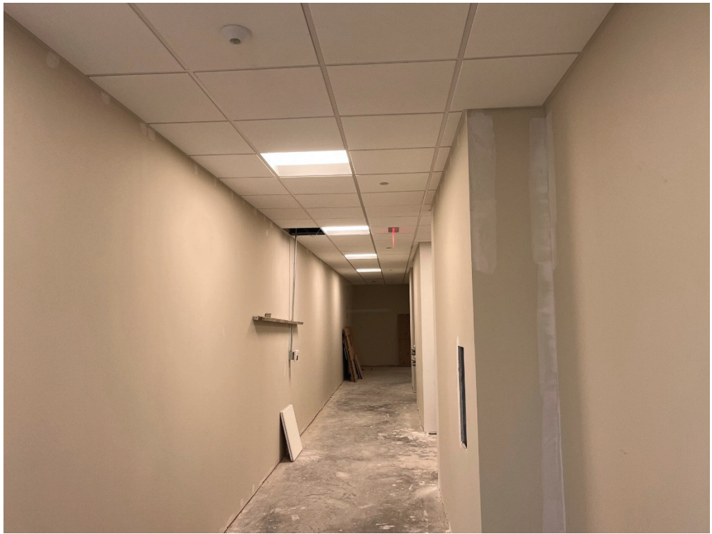
Figure 13 – 2 nd Floor Shared Space Ceilings Installed
