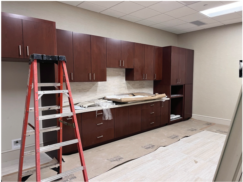
Figure 7 – 1 st Floor Break Progress
