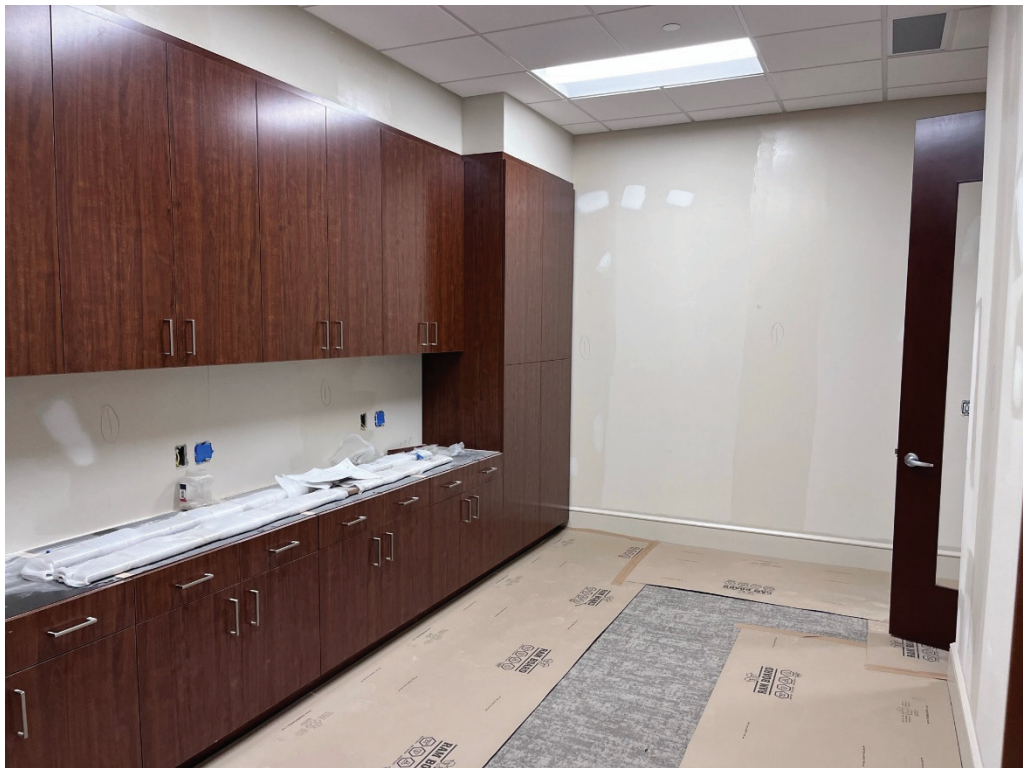
Figure 8 – Carpet Installed in Many Rooms at 1st
