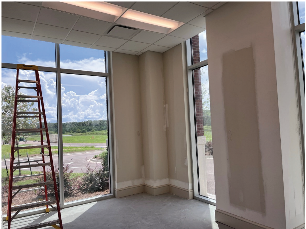
Figure 6 – 1 st Floor East Offices
