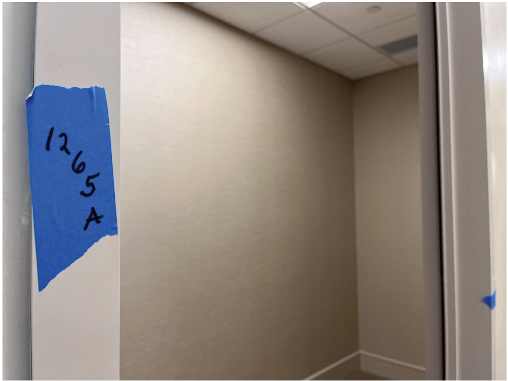
Figure 9 – 1 st Floor Wall Coverings are Ongoing
