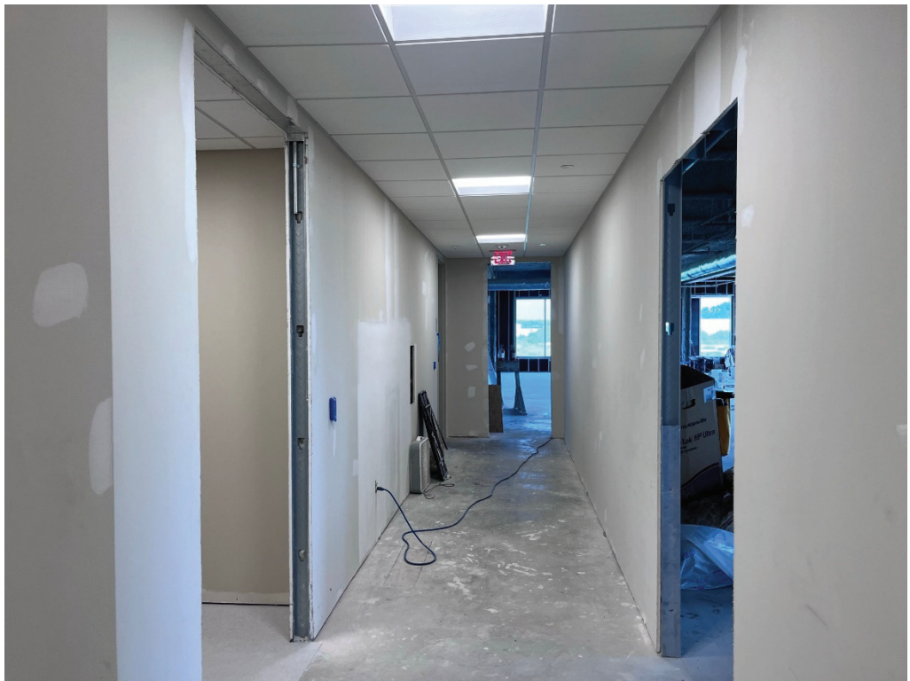
Figure 16 – 2 nd Floor Shared Space Ceilings Installed
