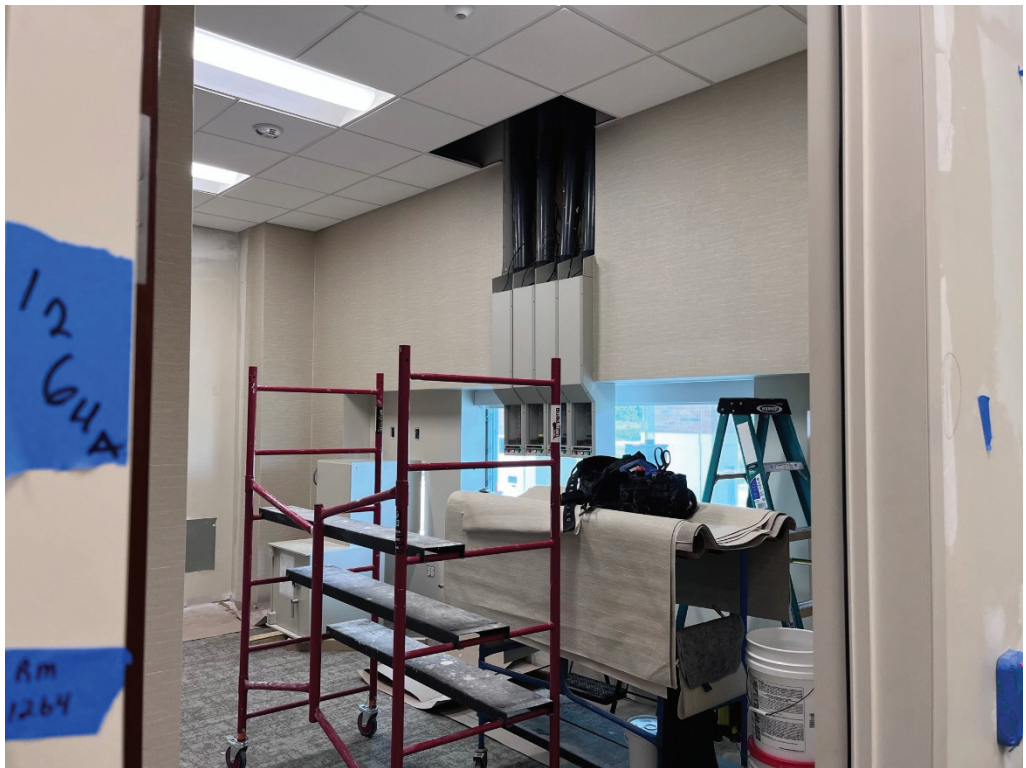
Figure 10 – Equipment Installers were at work in bank telling drive thru
