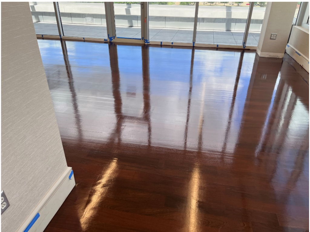
Figure 14 – Wood Floor, Drying
