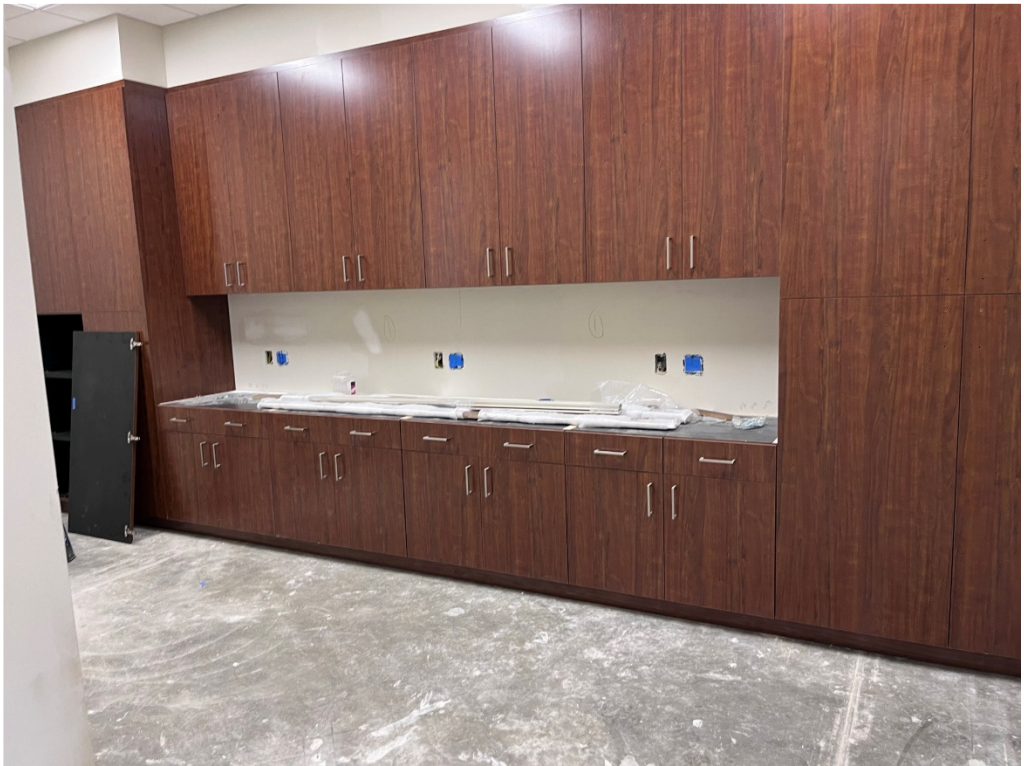
Figure 6 – 1 st Floor Workroom Progress
