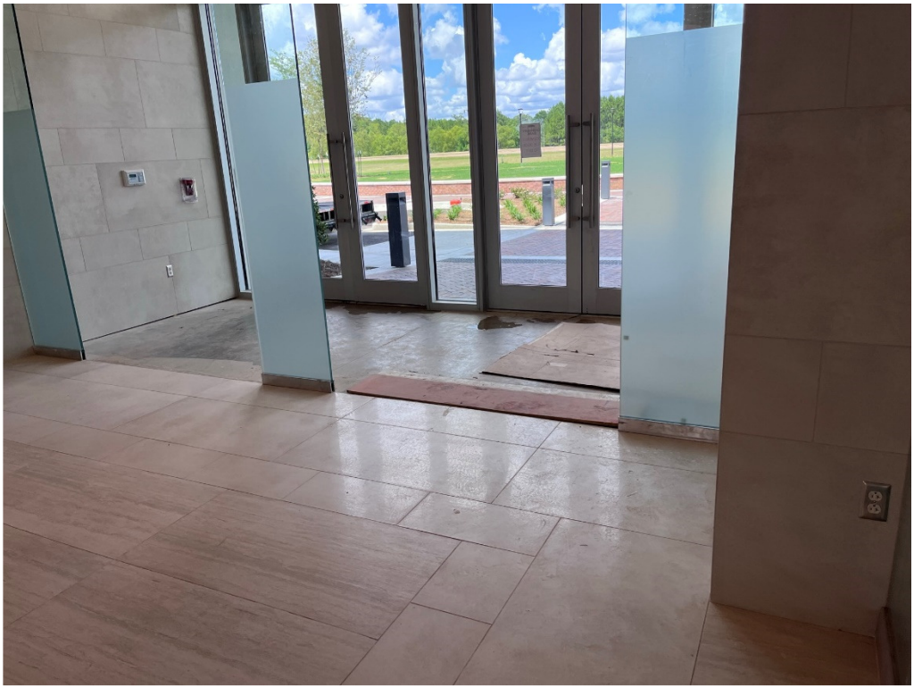
Figure 1 – 1 st Floor Entry Progressp
