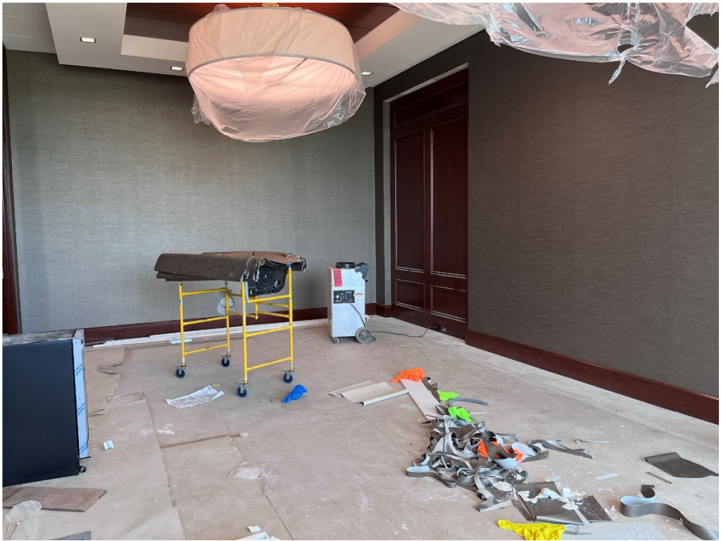
Figure 12 – Wall Covering progress
