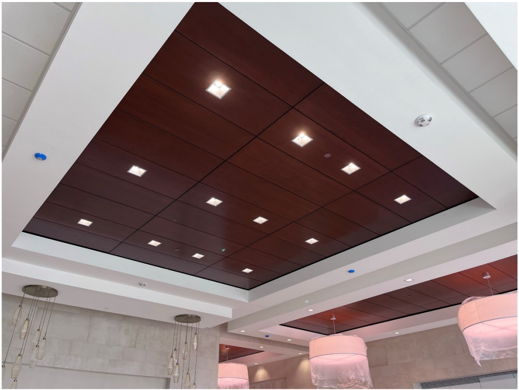
Figure 5 – 1 st Floor Lobby Ceilings
