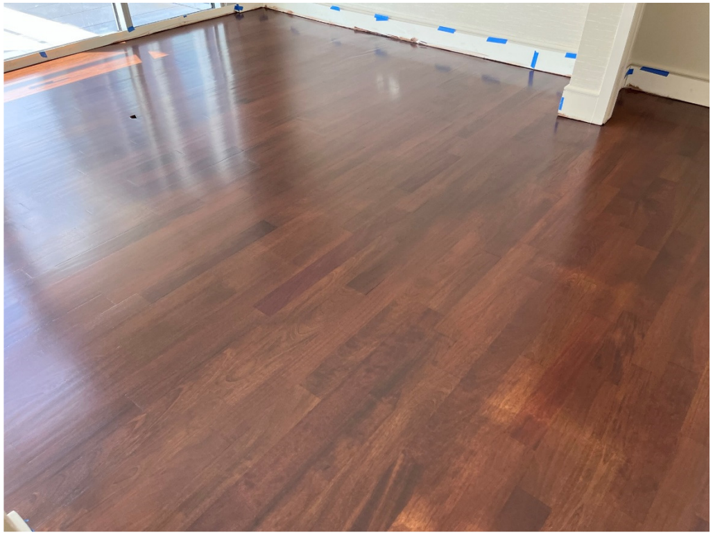
Figure 15 – Finished Wood Floor
