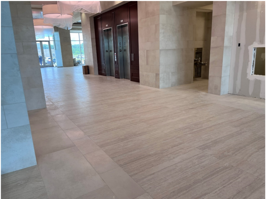
Figure 2 – 1 st Floor Clean Lobby
