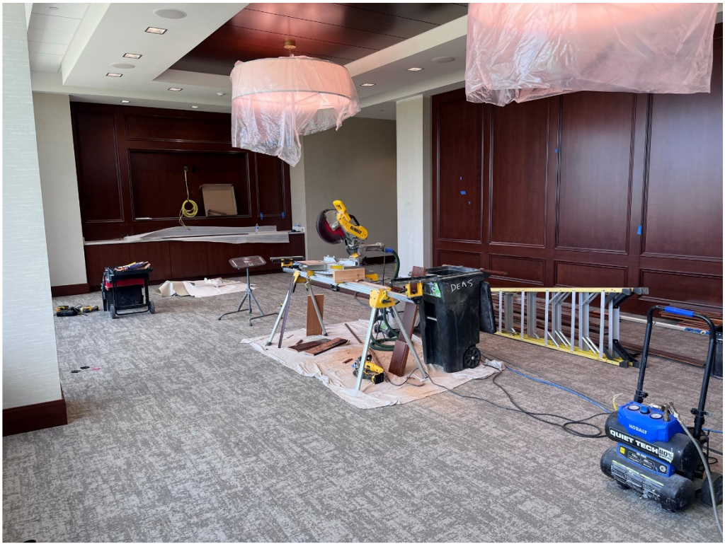
Figure 13 – Board Room Progress
