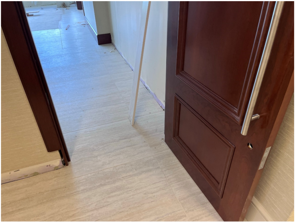
Figure 11 – Millwork is Ongoing
