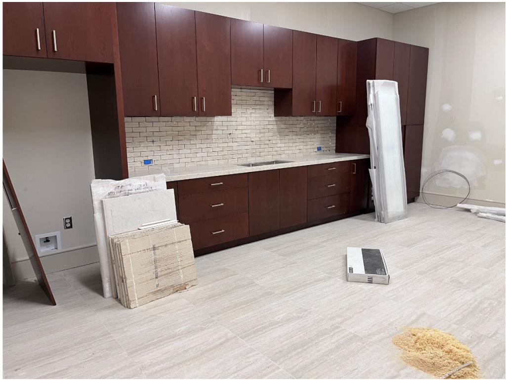
Figure 7 – 1 st Floor Break Progress
