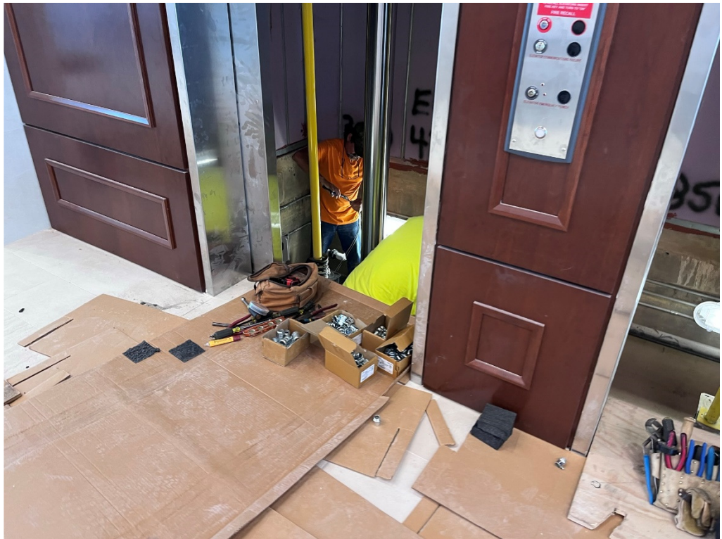
Figure 9 – Elevator work is ongoing
