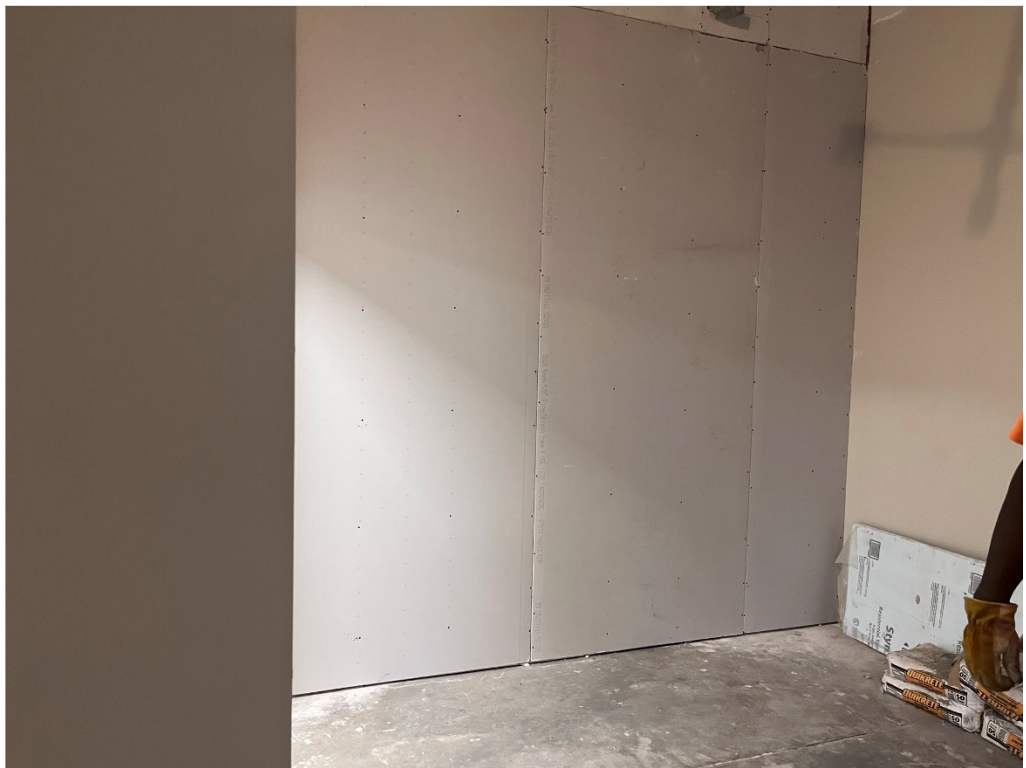
Figure 6 – Filled but still requires finishing
