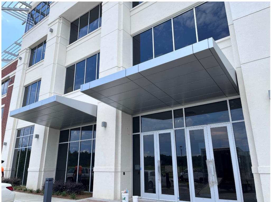
Figure 10 – Canopies are complete
