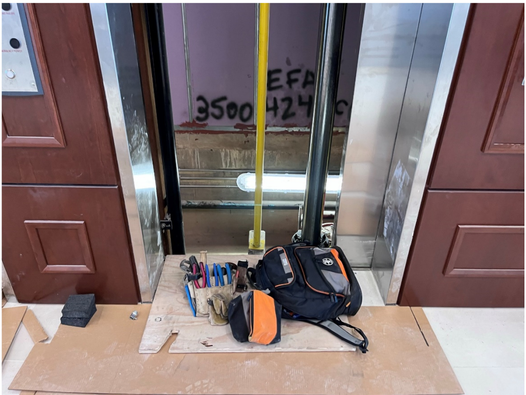
Figure 8 – Elevator work is ongoing
