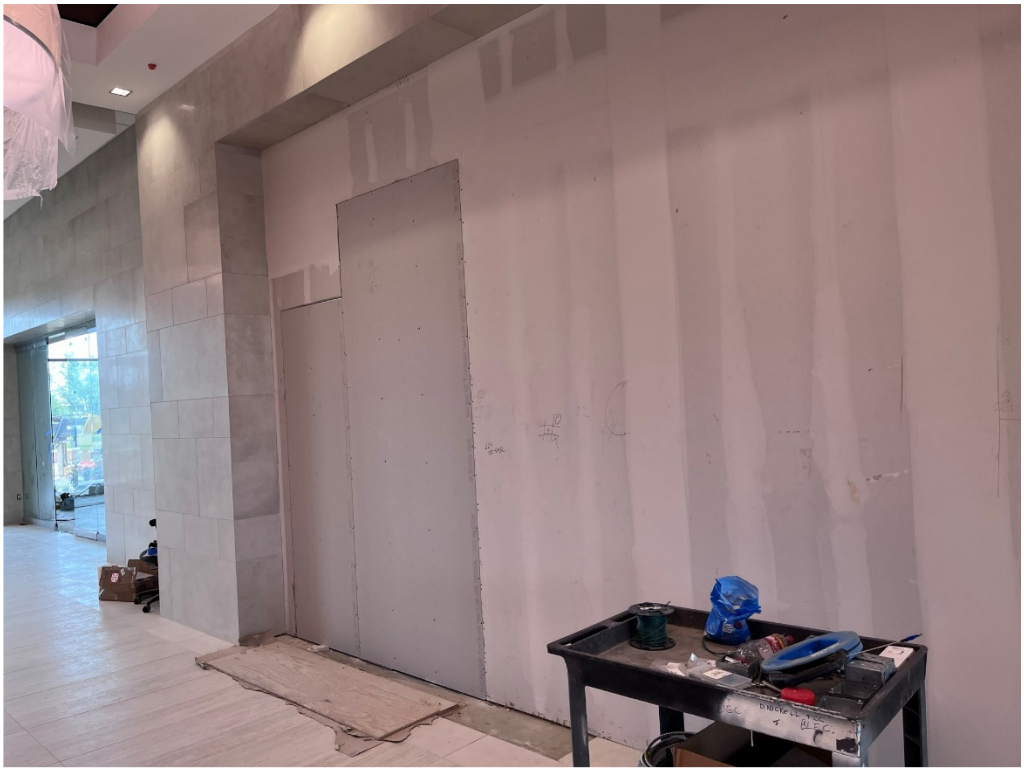
Figure 7 – Filled but still requires finishing
