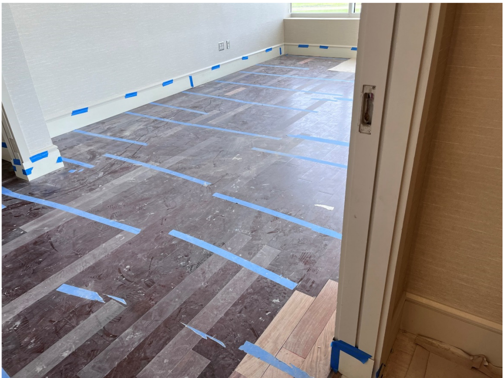
Figure 28 – No Sanding has begun
