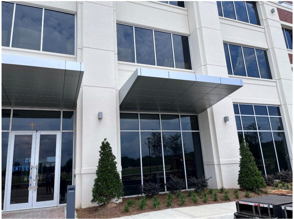
Figure 12 – Canopies are complete
