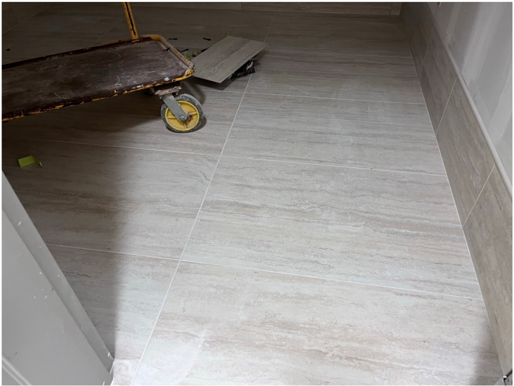
Figure 2 – Grout Installed
