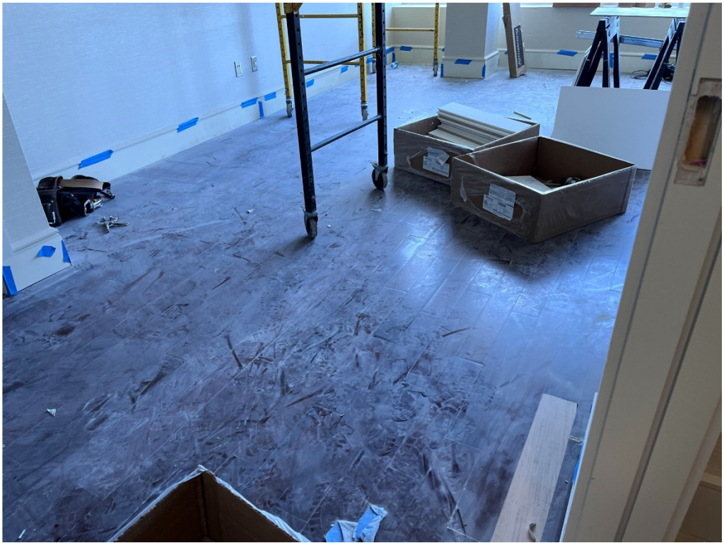
Figure 26 – No Sanding has begun
