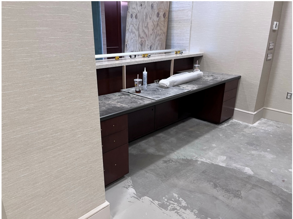
Figure 21 – Stone work is ongoing
