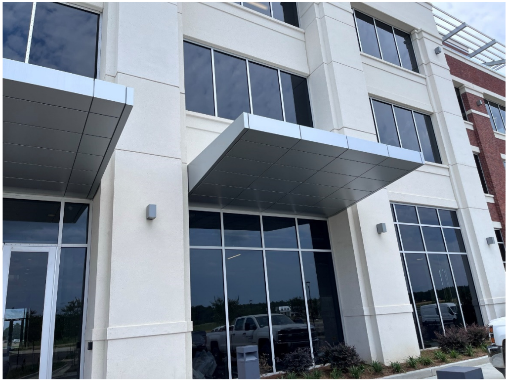
Figure 11 – Canopies are complete
