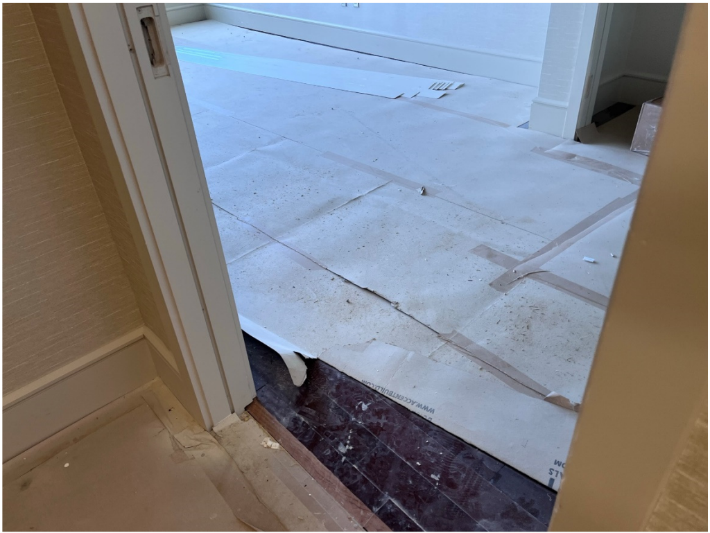
Figure 25 – No Sanding has begun
