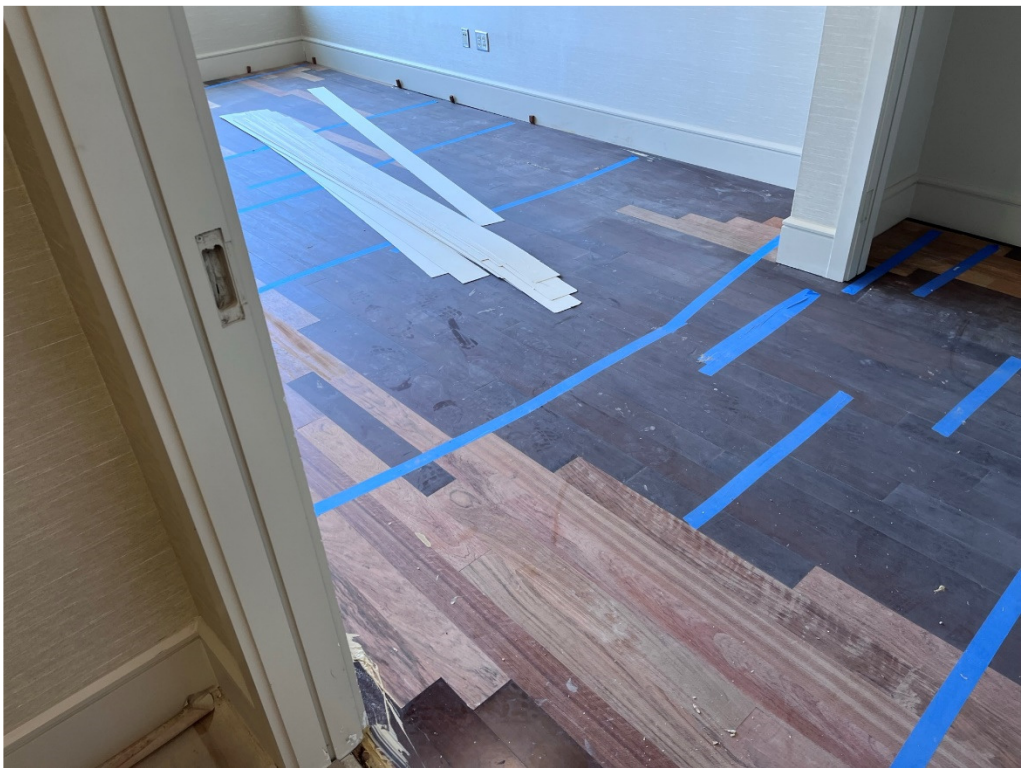
Figure 24 – No Sanding has begun
