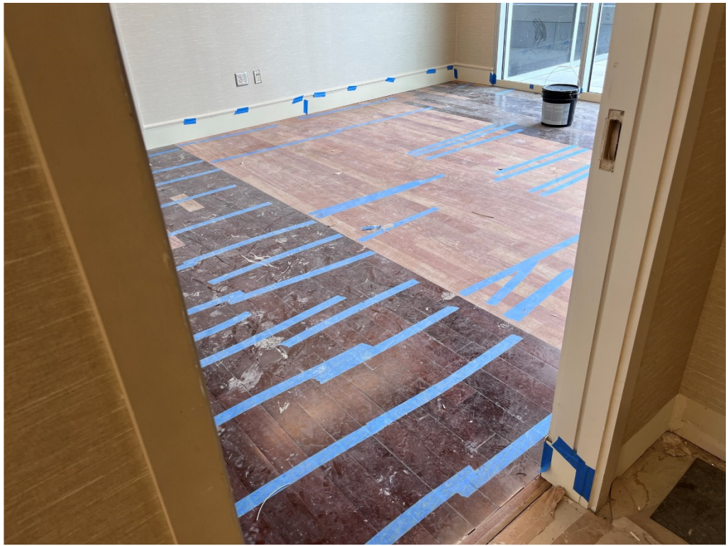
Figure 29 – No Sanding has begun
