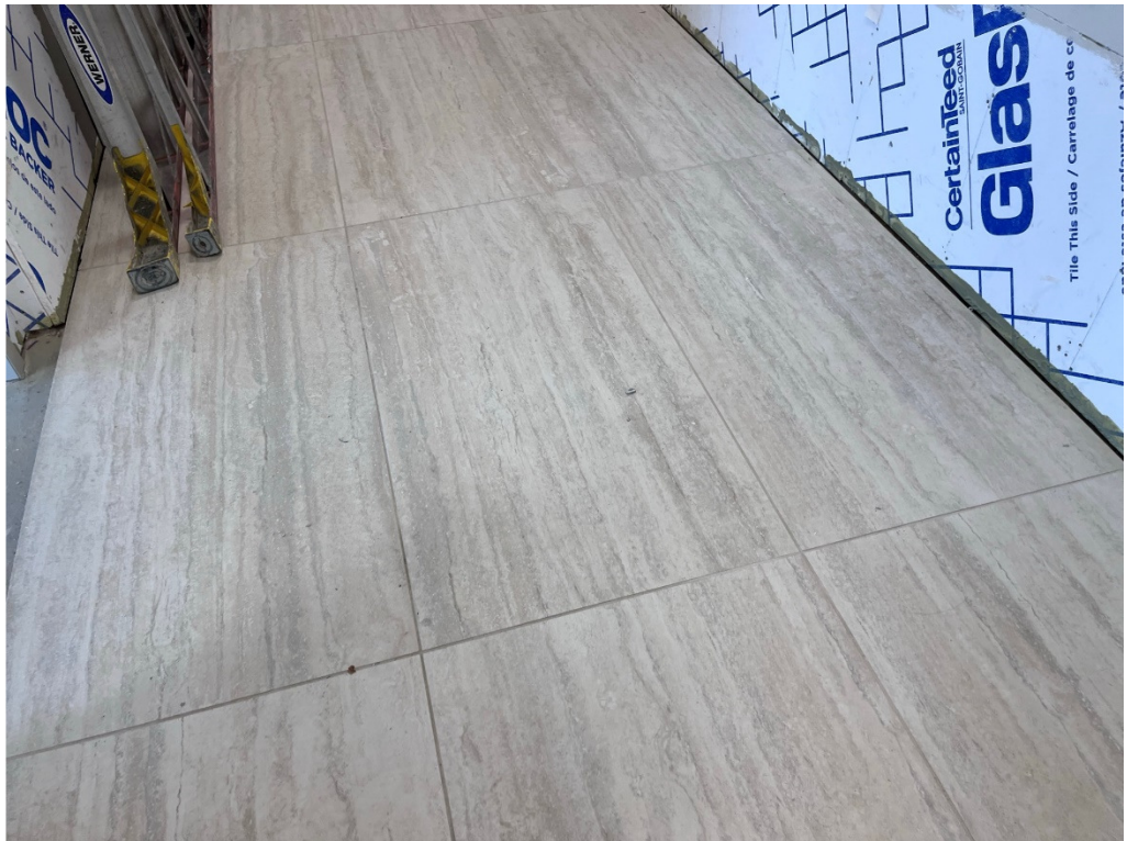
Figure 5 – Grout Installed
