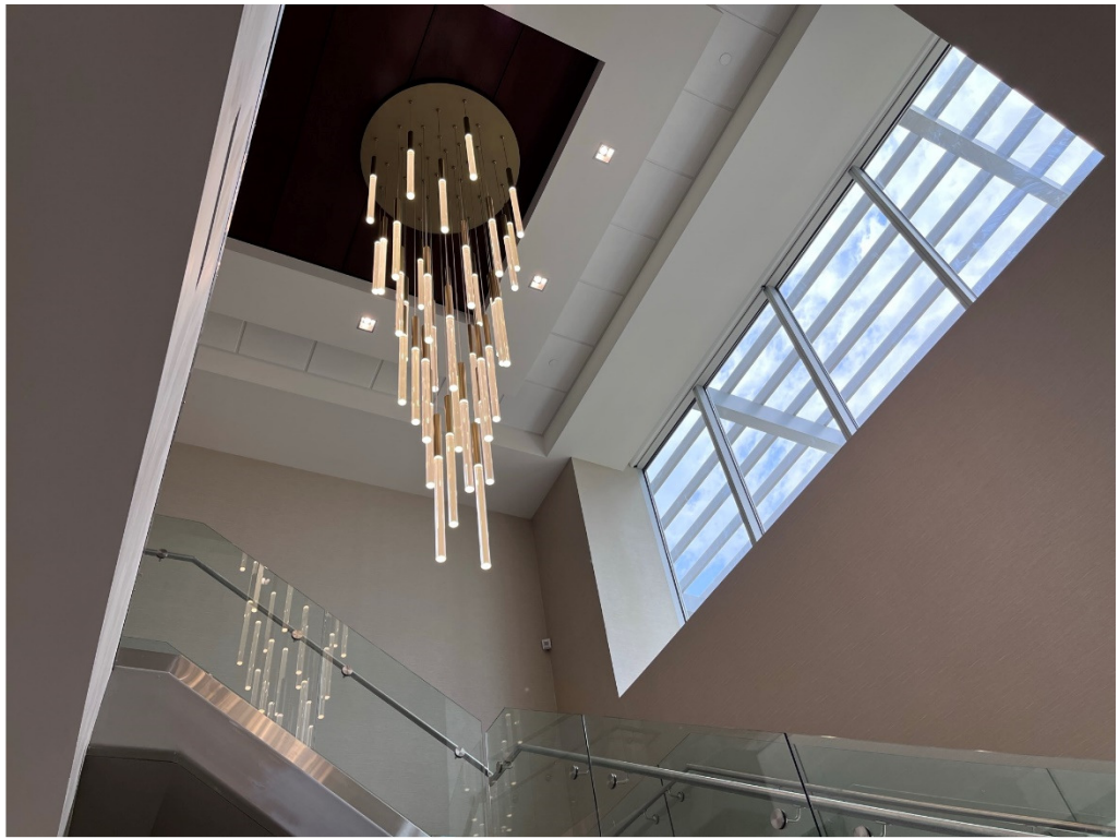
Figure 15 – Light Fixture Installed
