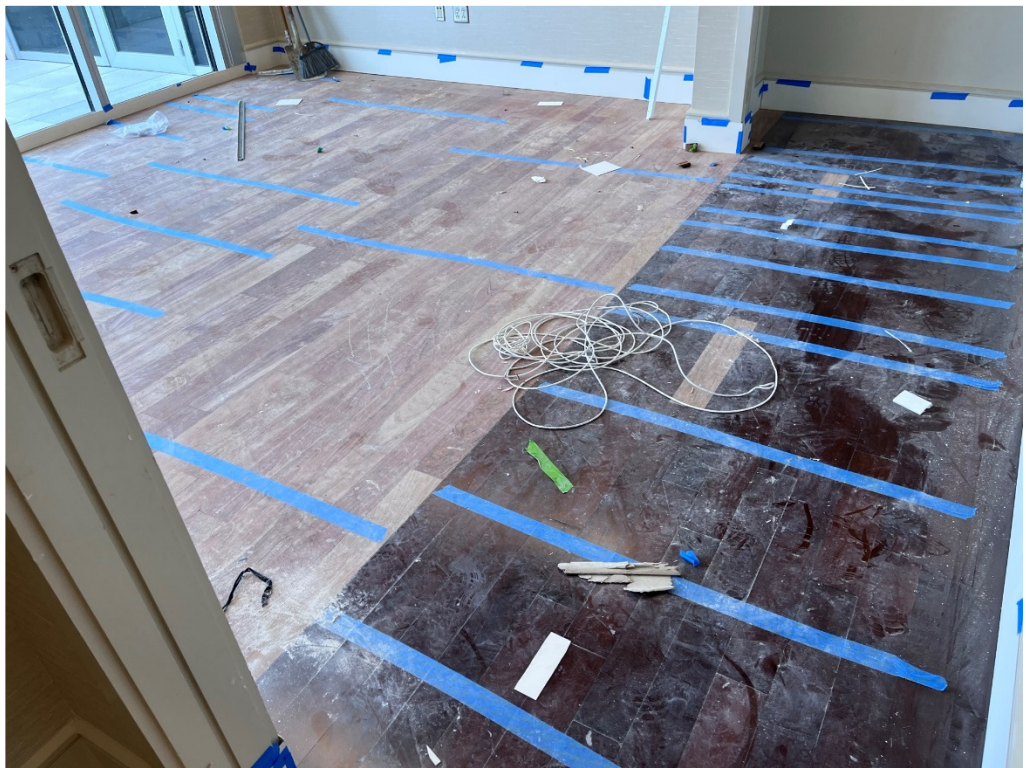
Figure 22 – No Sanding has begun
