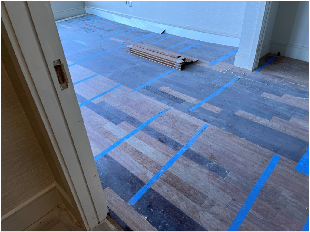
Figure 23 – No Sanding has begun
