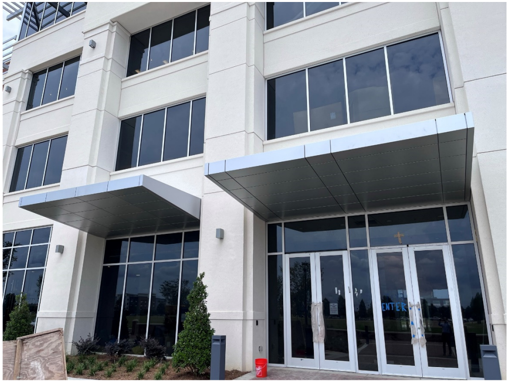
Figure 13 – Canopies are complete
