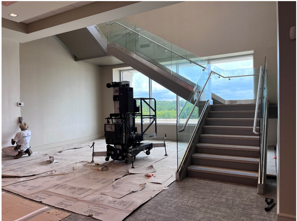
Figure 14 – Scaffolding is removed
