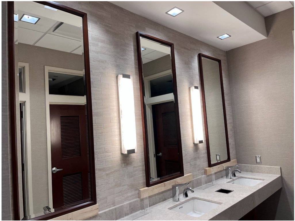
Figure 17 – Mirrors installed with temporary supports
