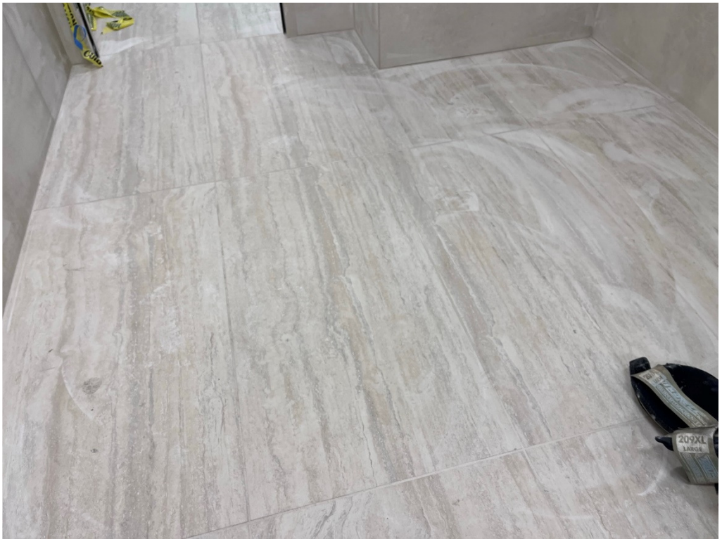
Figure 4 – Grout Installed
