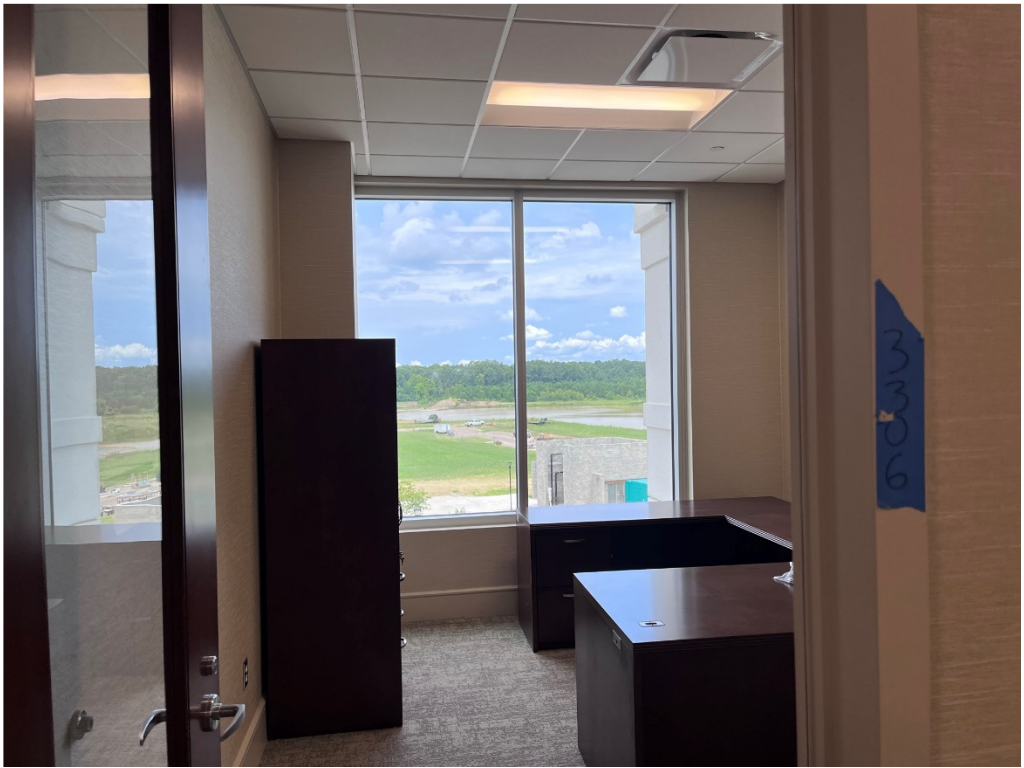
Figure 20 – Room where blinds are missing
