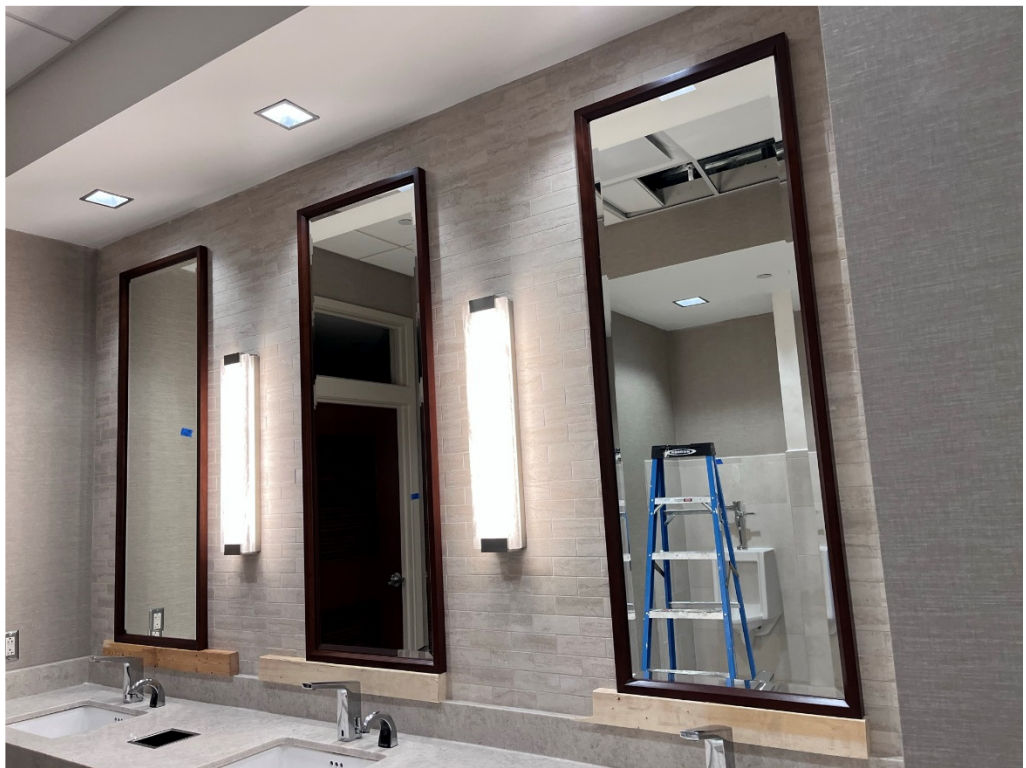
Figure 16 – Mirrors installed with temporary supports
