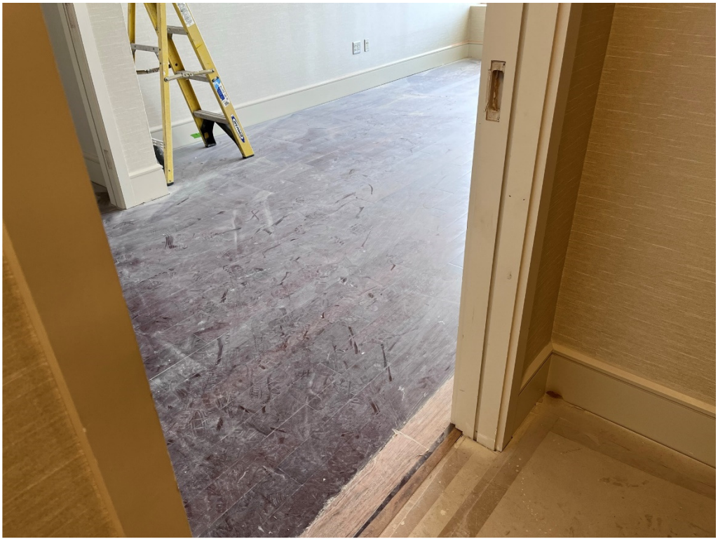
Figure 27 – No Sanding has begun
