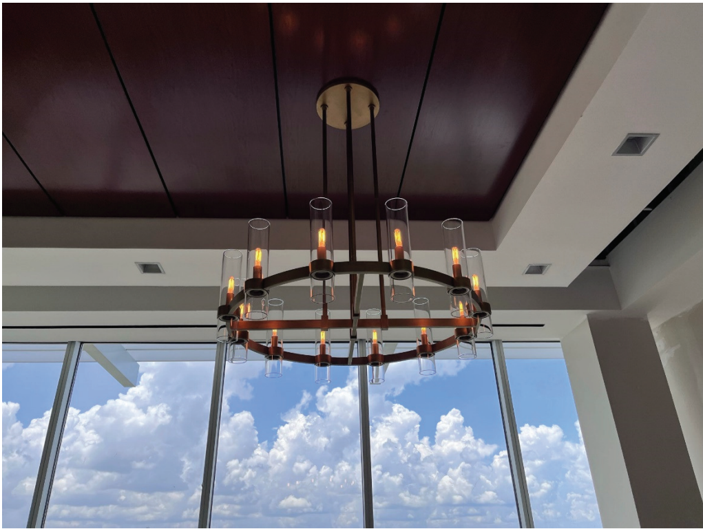
Figure 1 – Light Fixture Installation
