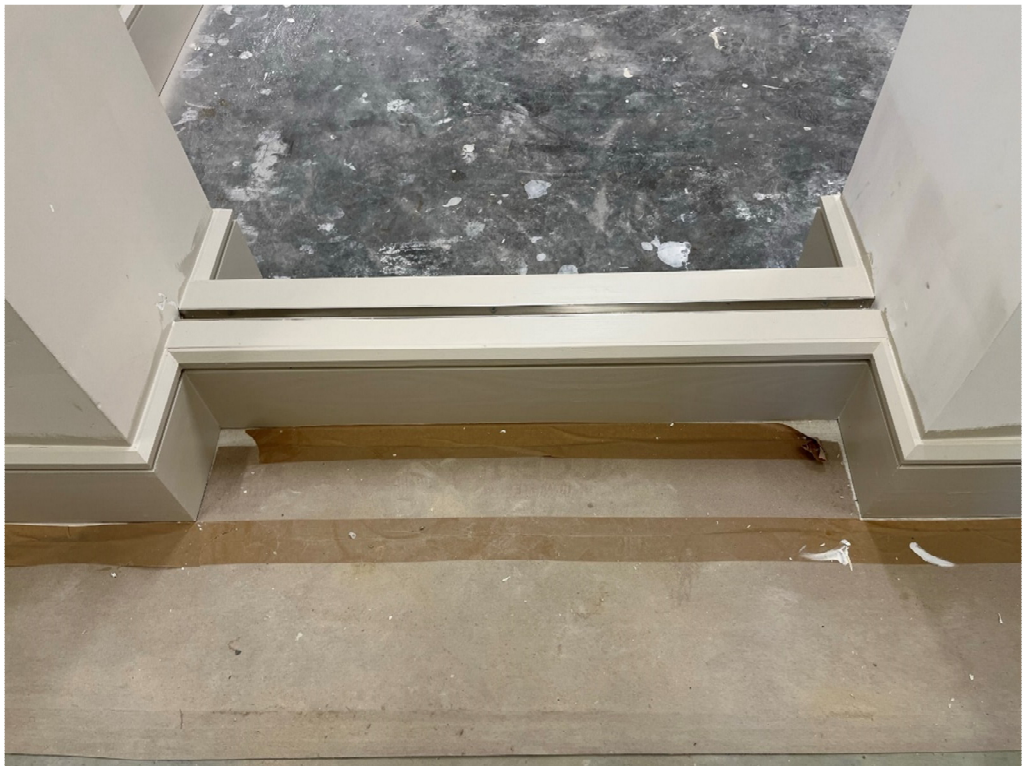
Figure 9 – Good Installation of Glass Receiver
