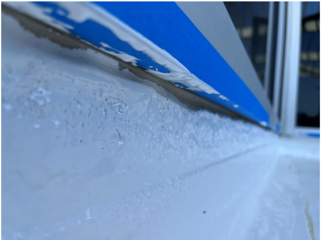
Figure 10 – Liquid Roofing Product installed to underside of AL Framing
