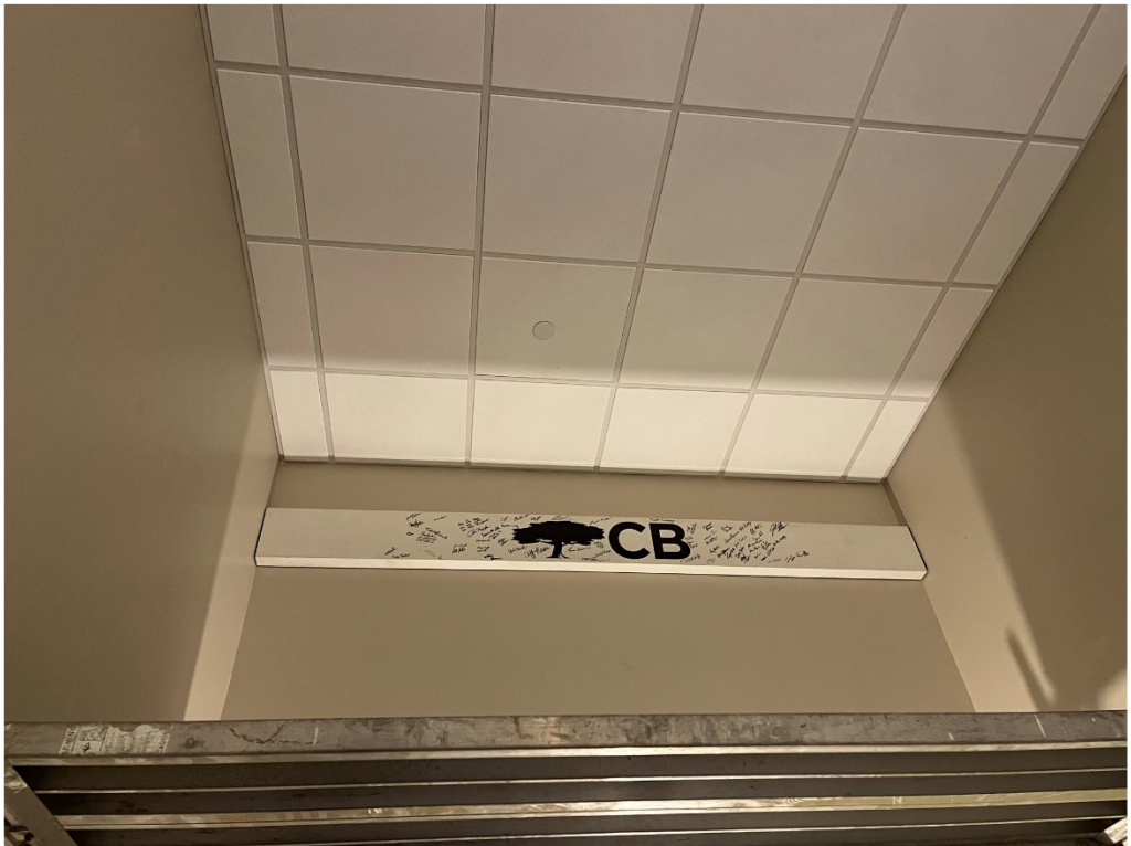
Figure 14 – South Stairwell Hanging Installed
