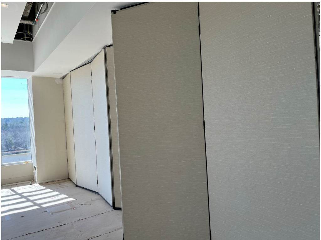
Figure 12 – Hanging Partitions Installed
