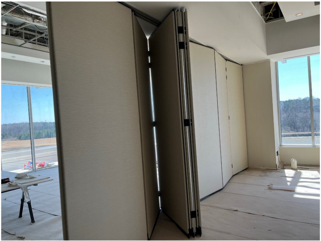
Figure 13 – Hanging Partitions Installed
