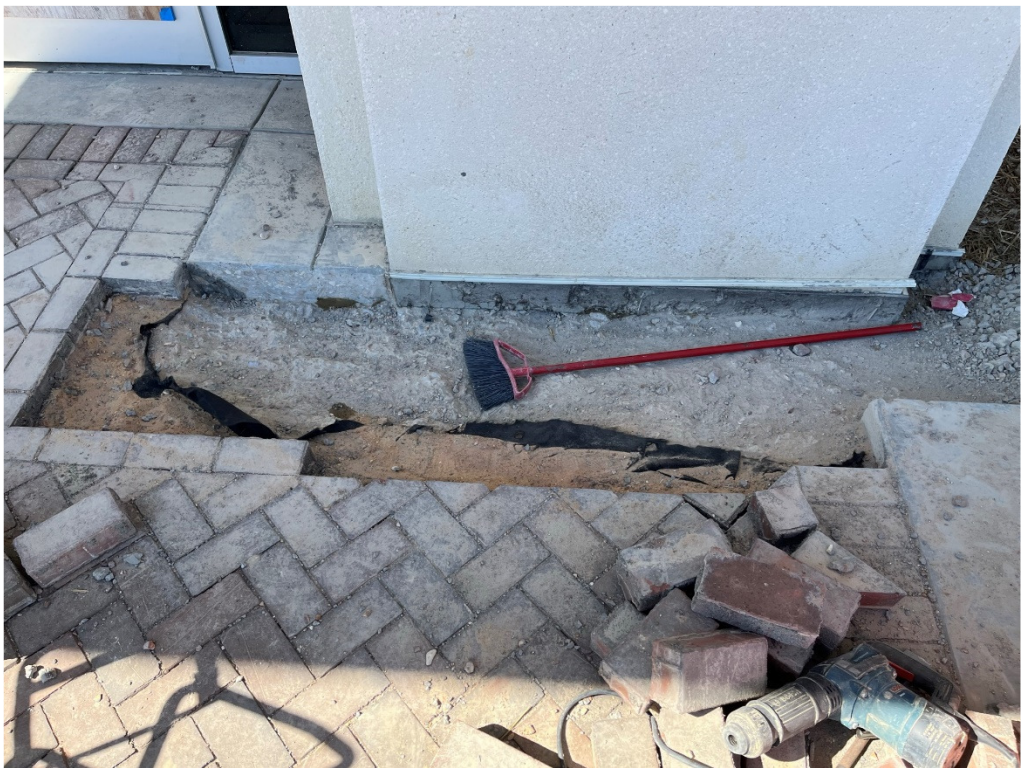
Figure 4 – Demo Work at East Entry
