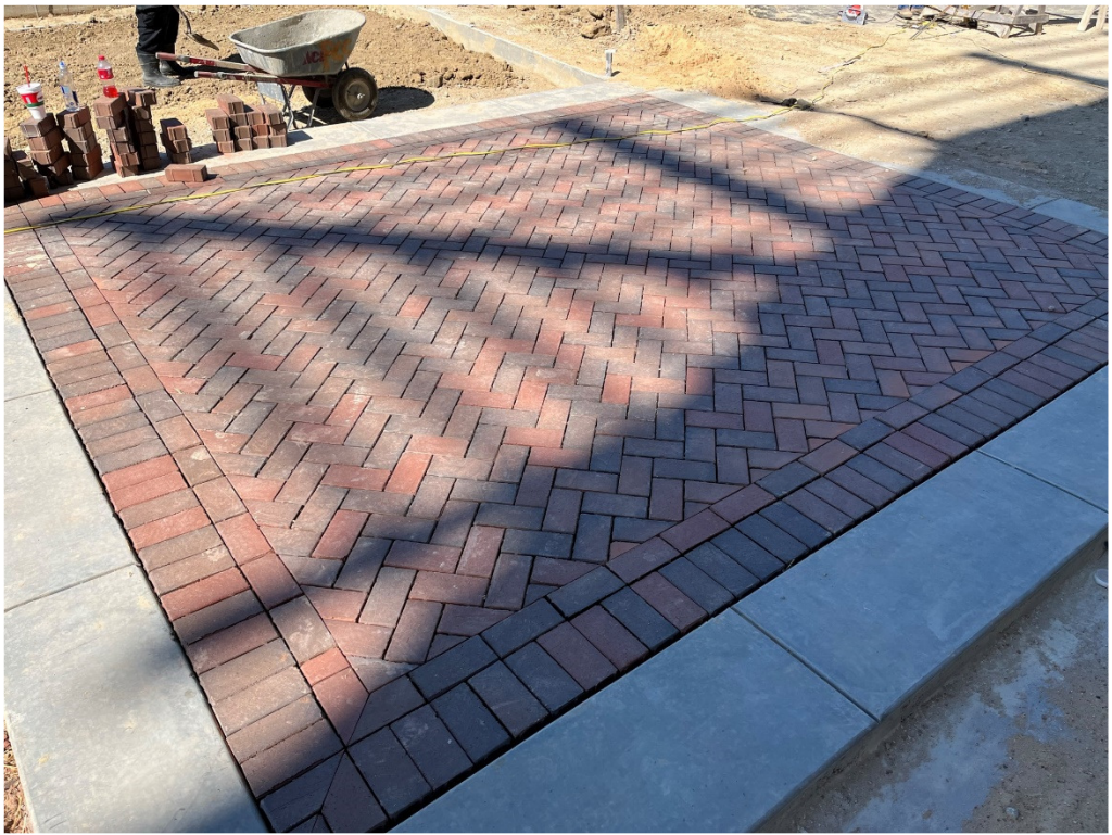
Figure 3 – Brick paver Installation looks good
