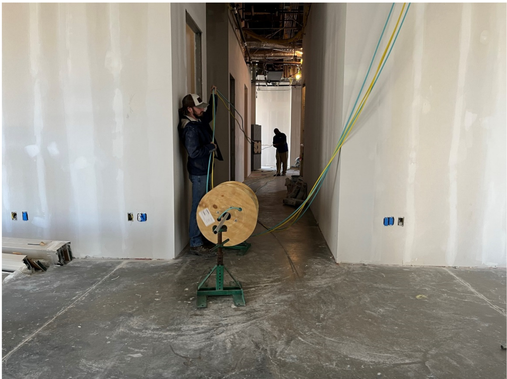
Figure 6 – Data Cable Installers on Site at 1 st Floor
