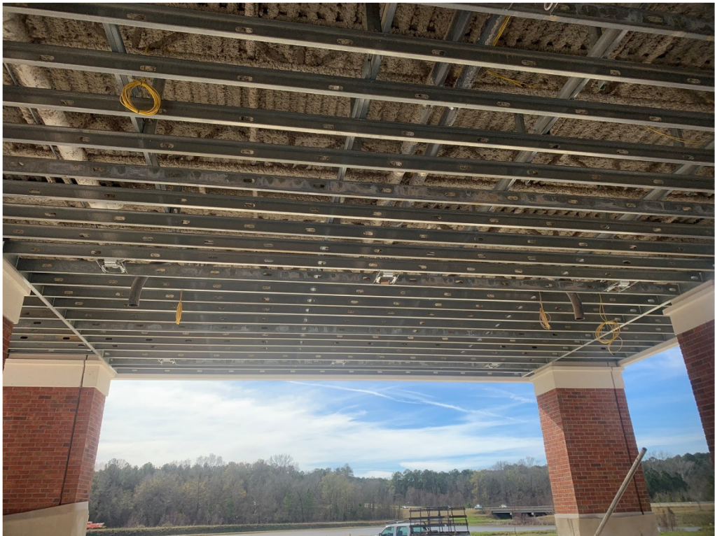
Figure 2 – Ceiling Framing @ Drive-Thru
