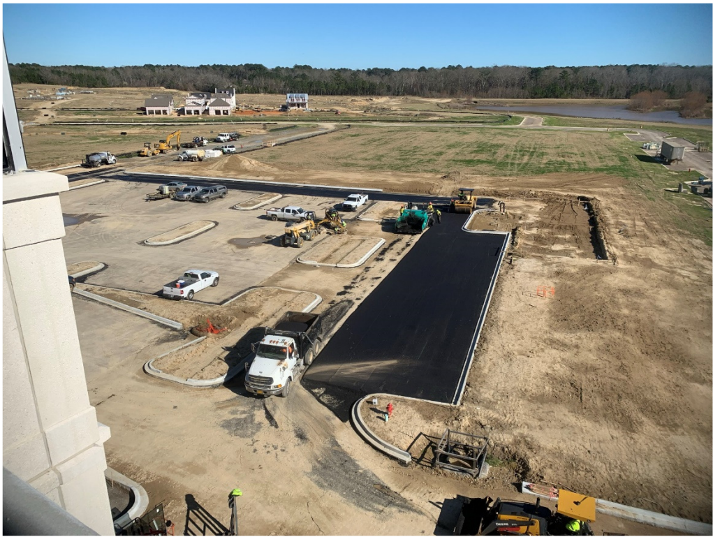
Figure 9 – Asphalt Installation
