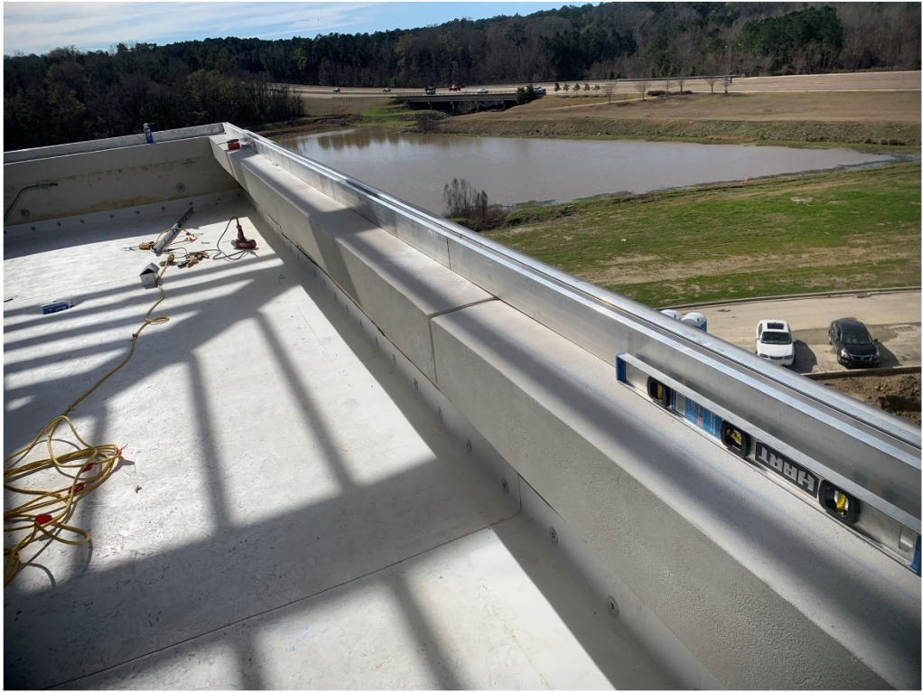
Figure 6 – Typical Glass Rail Install
