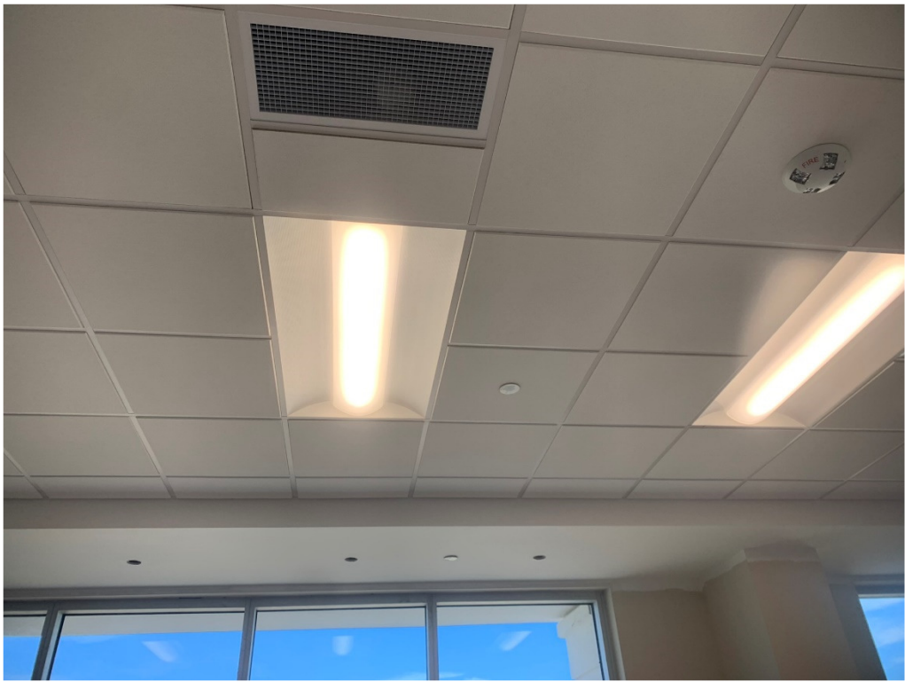
Figure 3 – ACT Install is Ongoing
