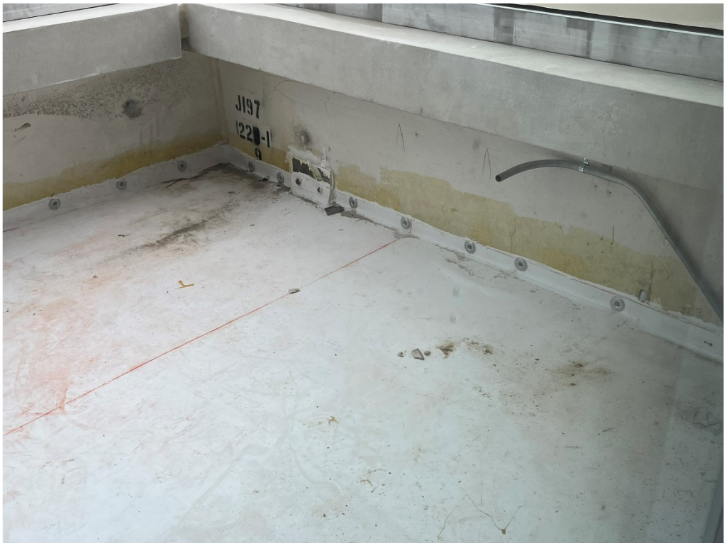
Figure 7 – TPO installation @ Balcony
