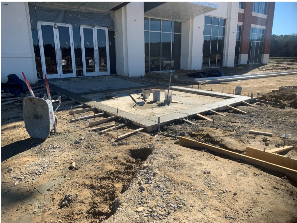
Figure 8 – Concrete is Ongoing
