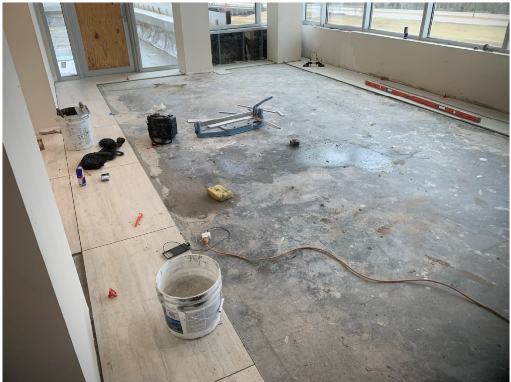
Figure 6 – Tile is ongoing throughout
