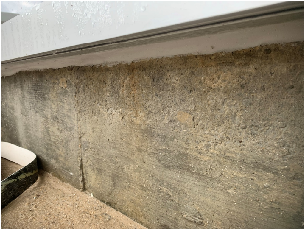
Figure 9 – Caulking below curtain walls assemblies at balconies on 4th
