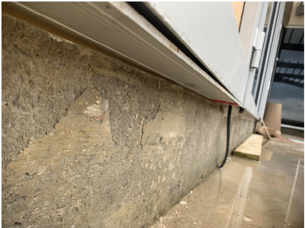
Figure 8 – No Caulking present in some locations below curtain walls assemblies at balconies on 4 th
