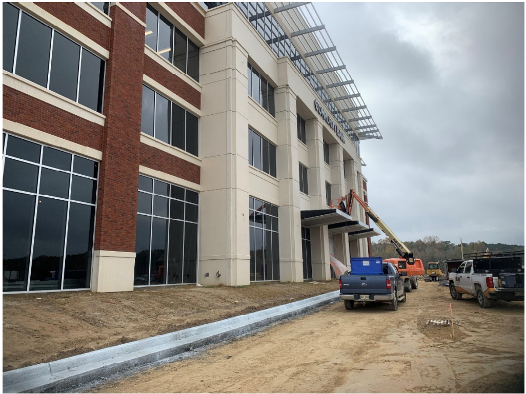
Figure 1 – West Façade; curb installed
