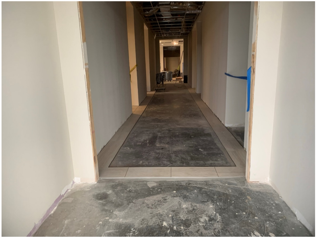
Figure 5 – Tile is ongoing throughout
