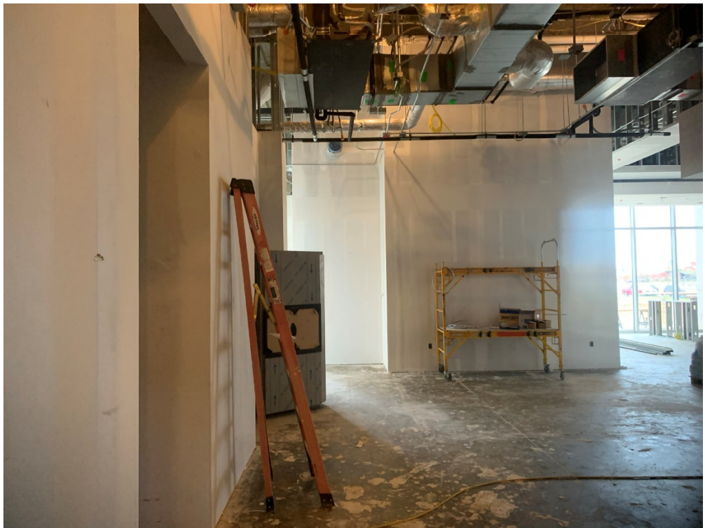
Figure 4 – Drywall is ongoing throughout
