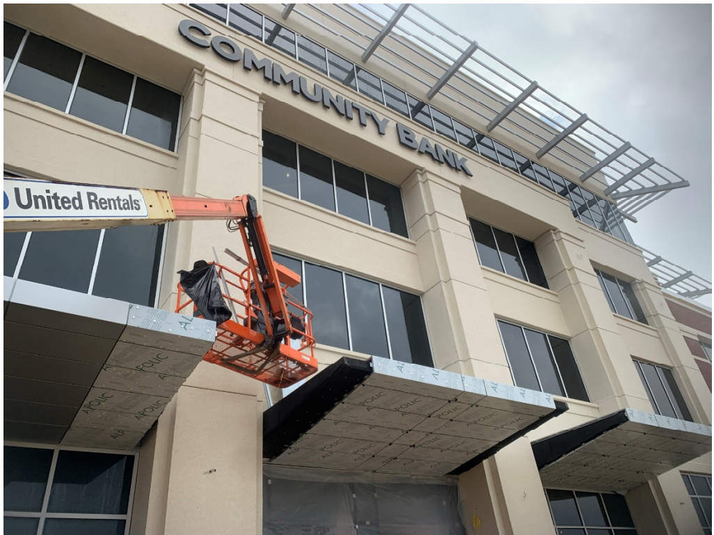
Figure 2 – Aluminum Cladding is ongoing
