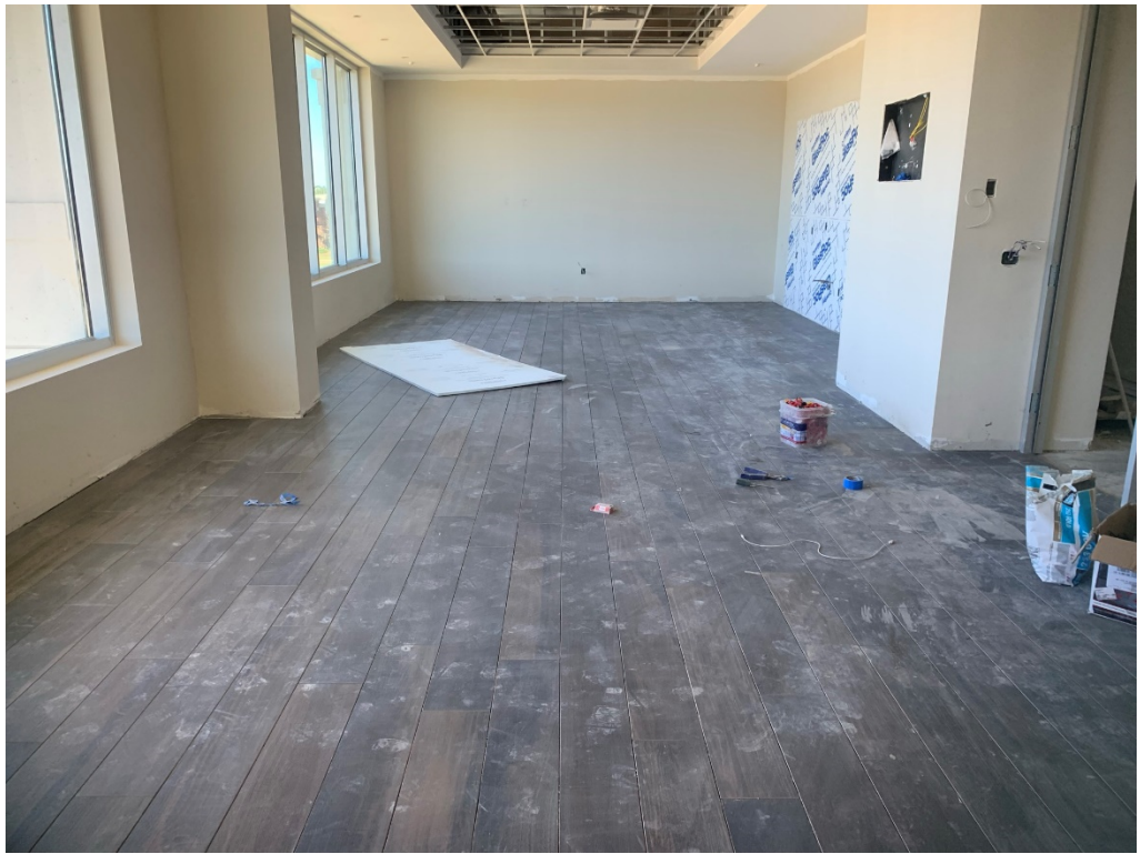
Figure 13 – Tile at Break Area Laid
