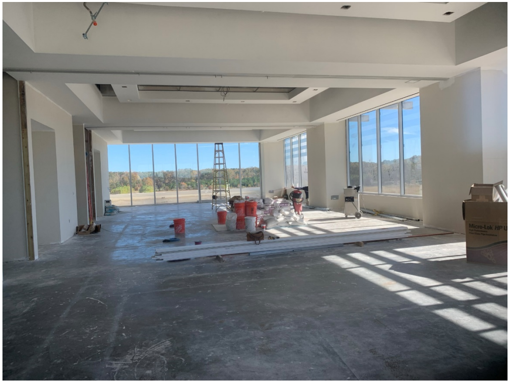
Figure 17 – Banquet Room Progress
