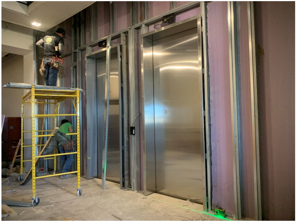
Figure 9 – Main Elevator work is ongoing
