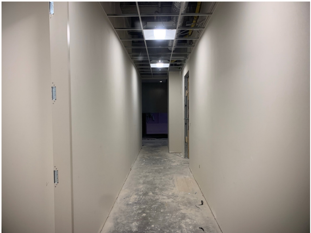
Figure 10 – Painting and Finishing is ongoing
