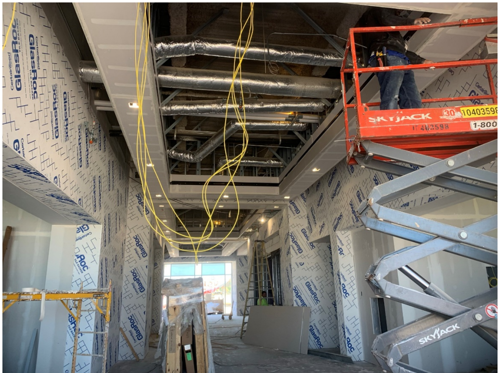
Figure 8 – First Floor Lobby Progress
