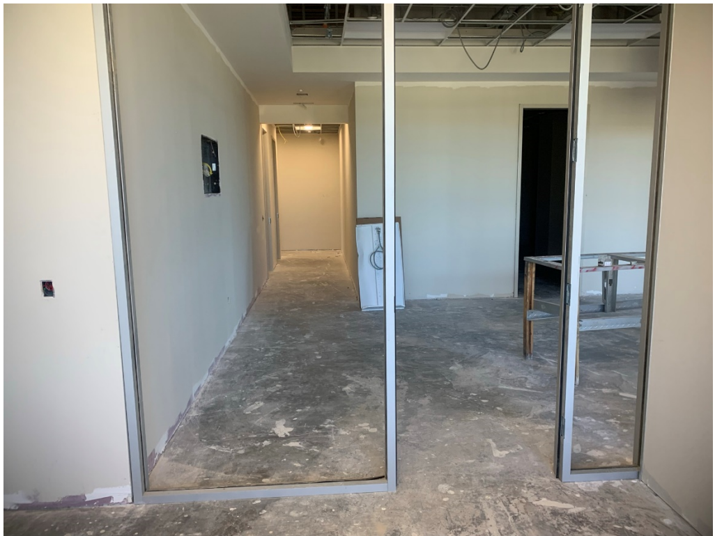
Figure 12 – Interior Frames installed throughout
