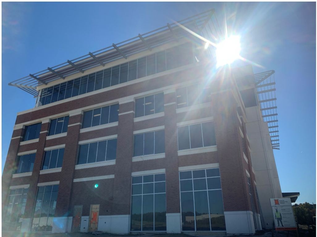
Figure 2 – North Façade Progress
