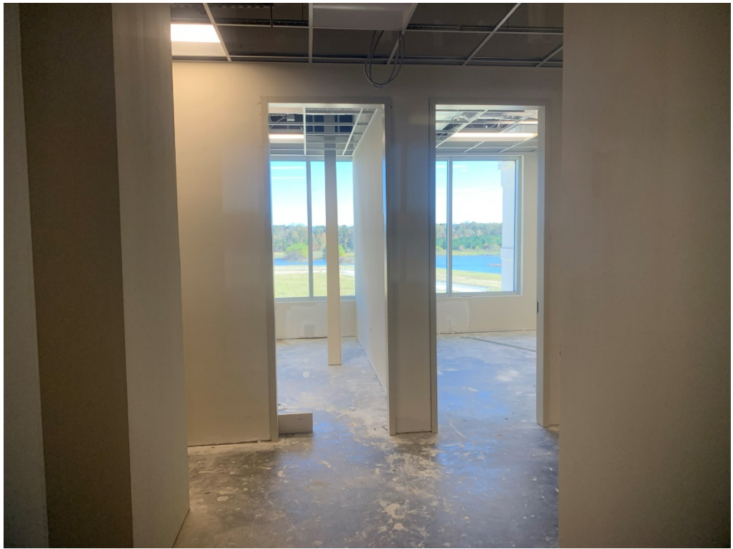
Figure 11 – Painting and Finishing is ongoing
