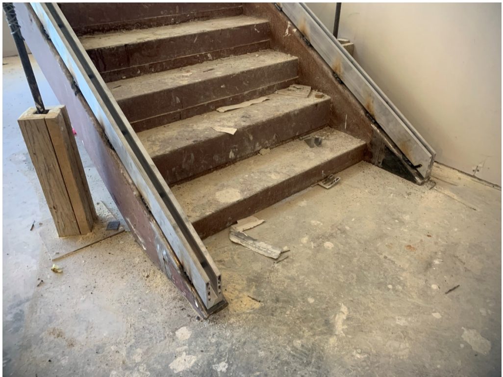
Figure 14 – Glass Handrail Base Fitted and Secured
