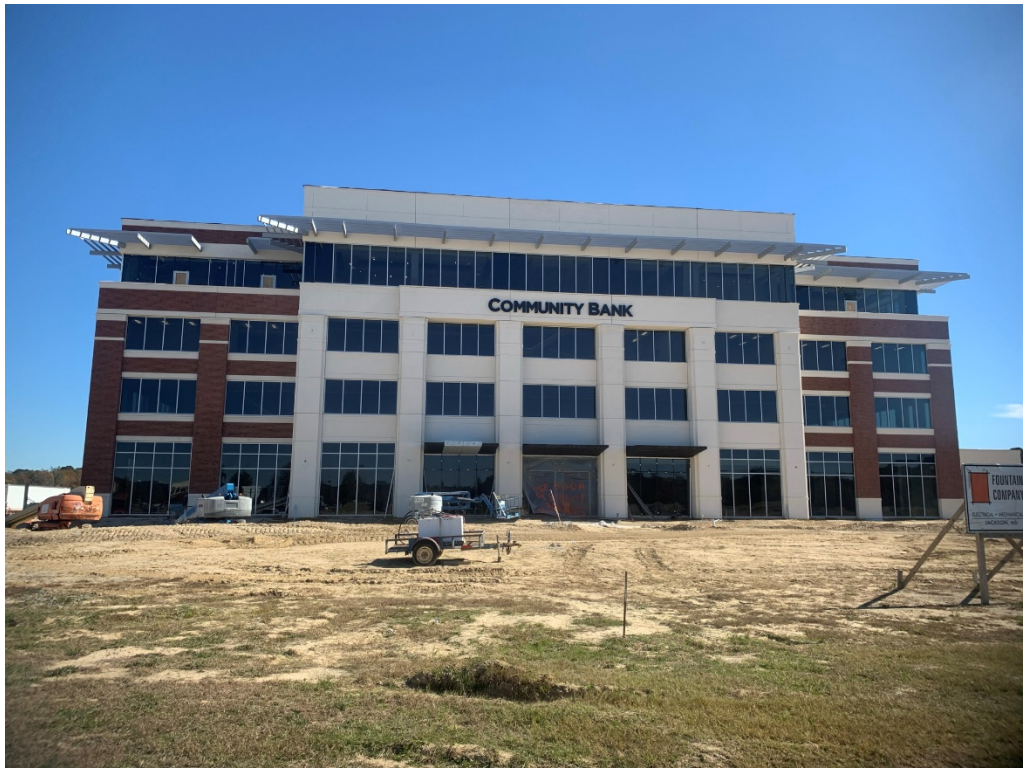
Figure 1 – West Façade Progress
