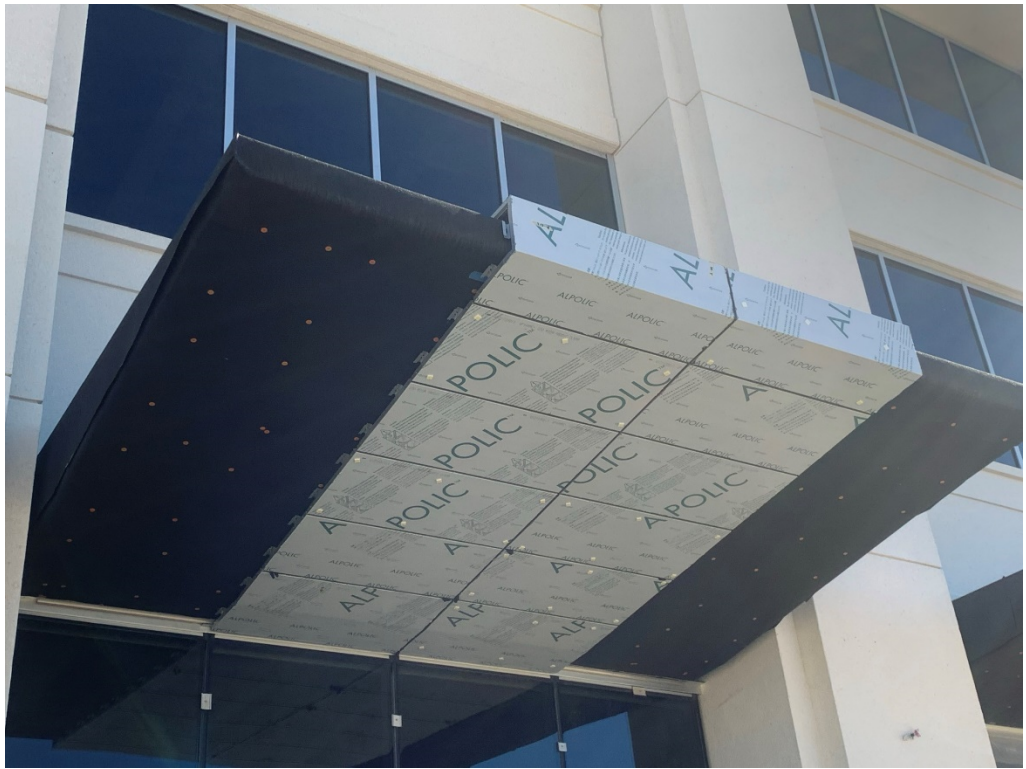
Figure 7 – Aluminum Clad Panel Installation Progress
