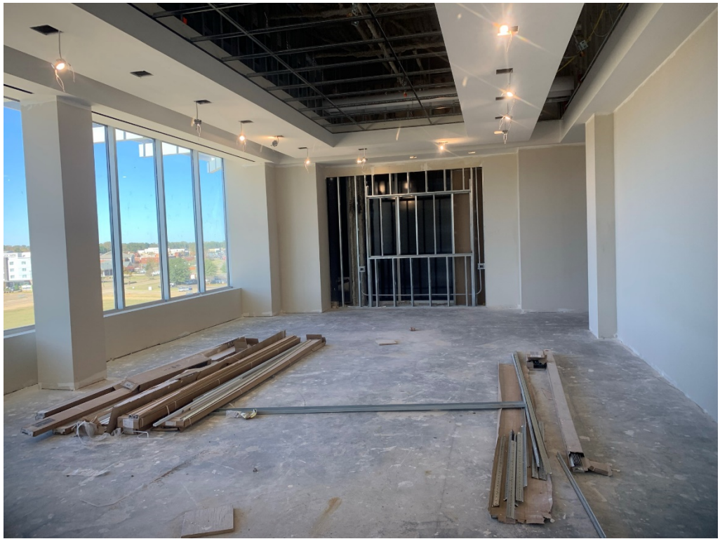
Figure 19 – Board Room Progress
