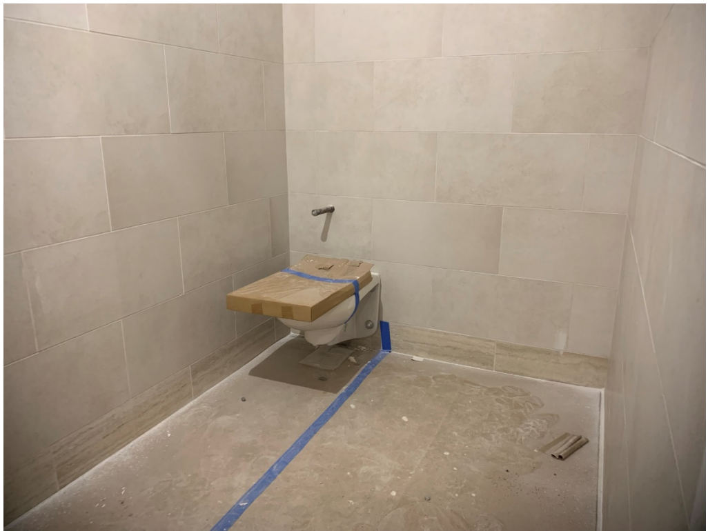
Figure 16 – Toilets are being installed Throughout
