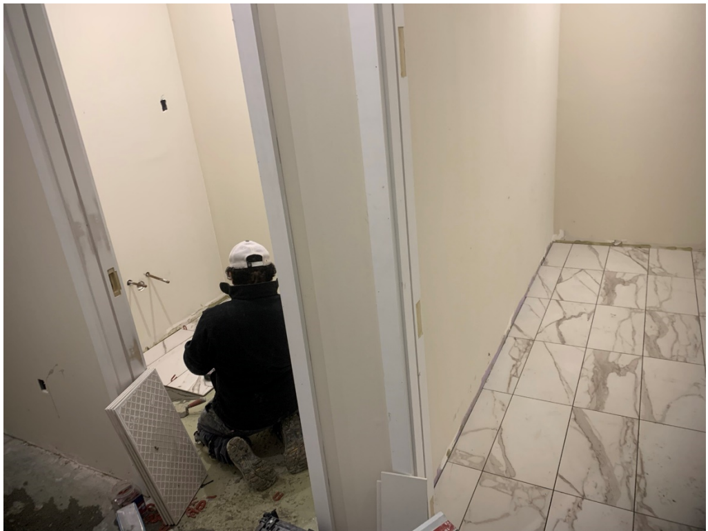
Figure 20 – Tile at fourth Floor Exec. Toilets
