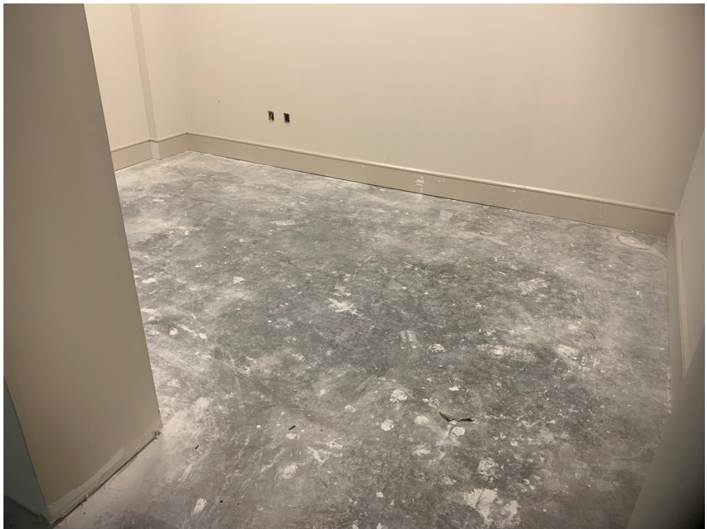
Figure 22 – Trim work at base is ongoing
