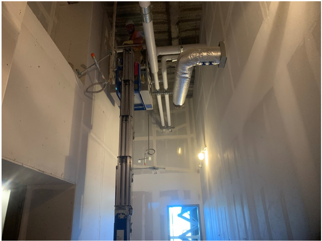
Figure 13 – Repair of fireproofing in ongoing
