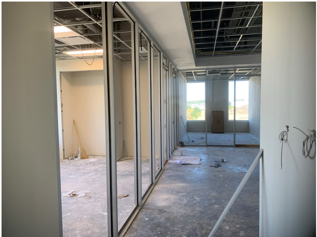
Figure 18 – 3 rd Floor Open Office Progress
