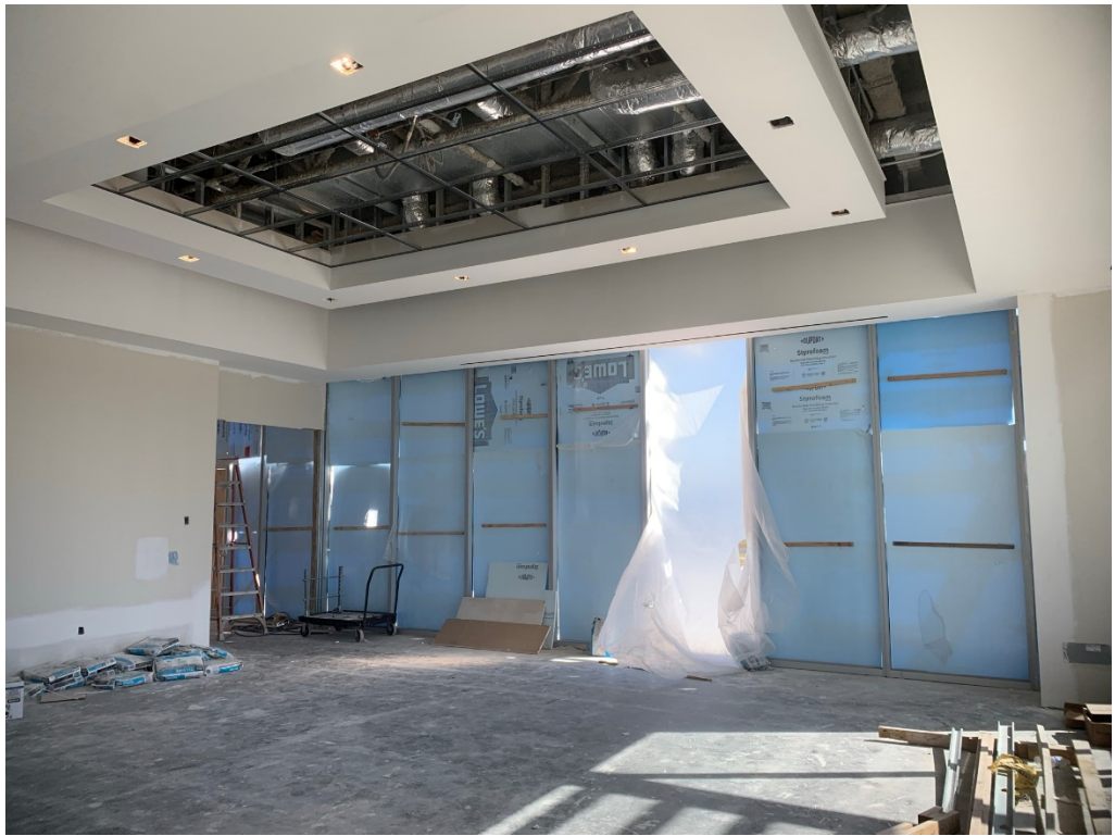
Figure 19 – Banquet room progress ( one of the last areas to receive glass)
