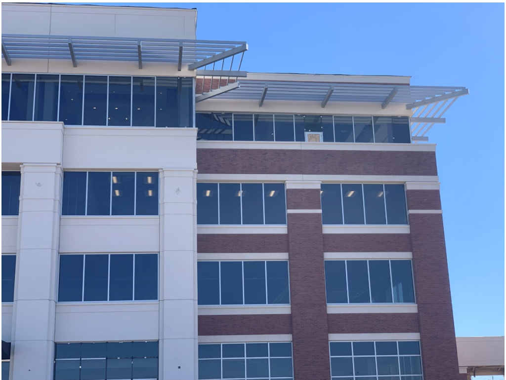
Figure 6 – Sun Shades are 80% Installed
