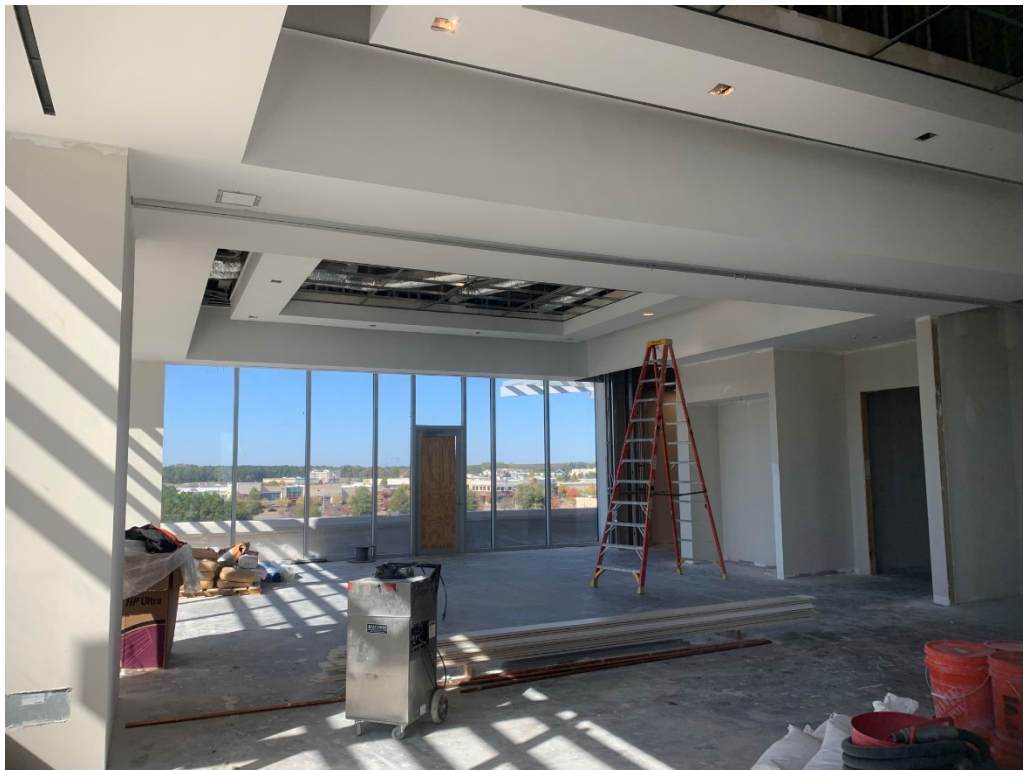
Figure 20 – Banquet room progress
