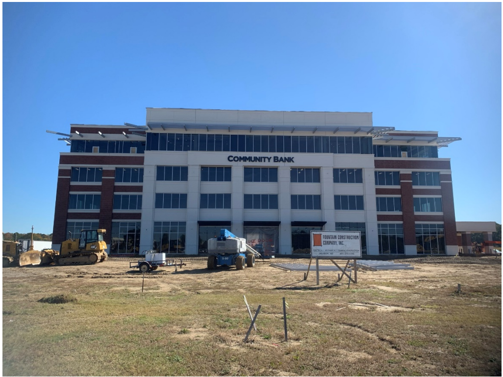
Figure 1 – West Façade Progress
