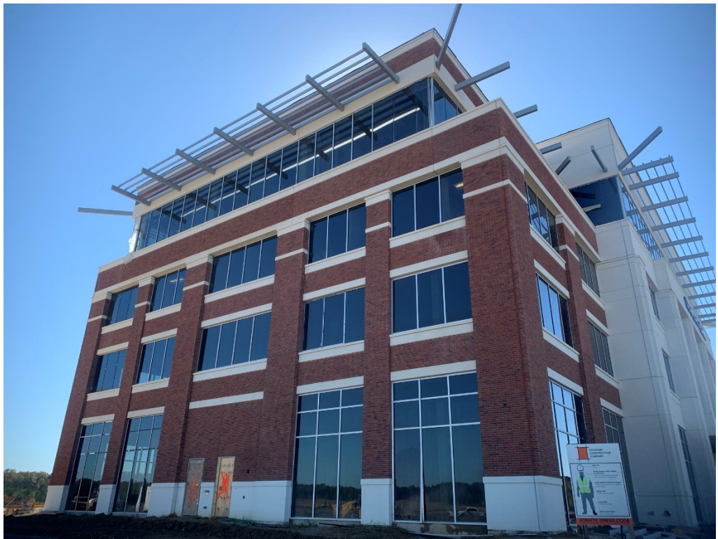
Figure 2 – North Façade Progress
