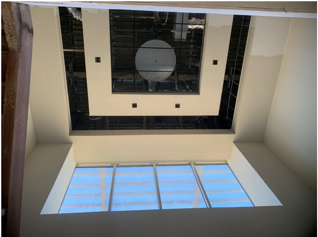
Figure 16 – Monumental stair Ceiling
