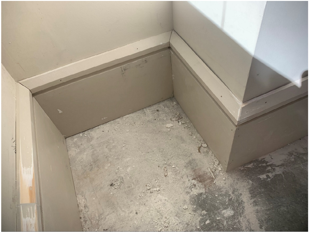
Figure 15 – Good attention to detail; trim work is moving along
