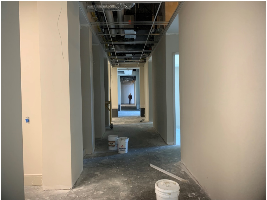
Figure 21 – 4 th floor hallway progress (typical)
