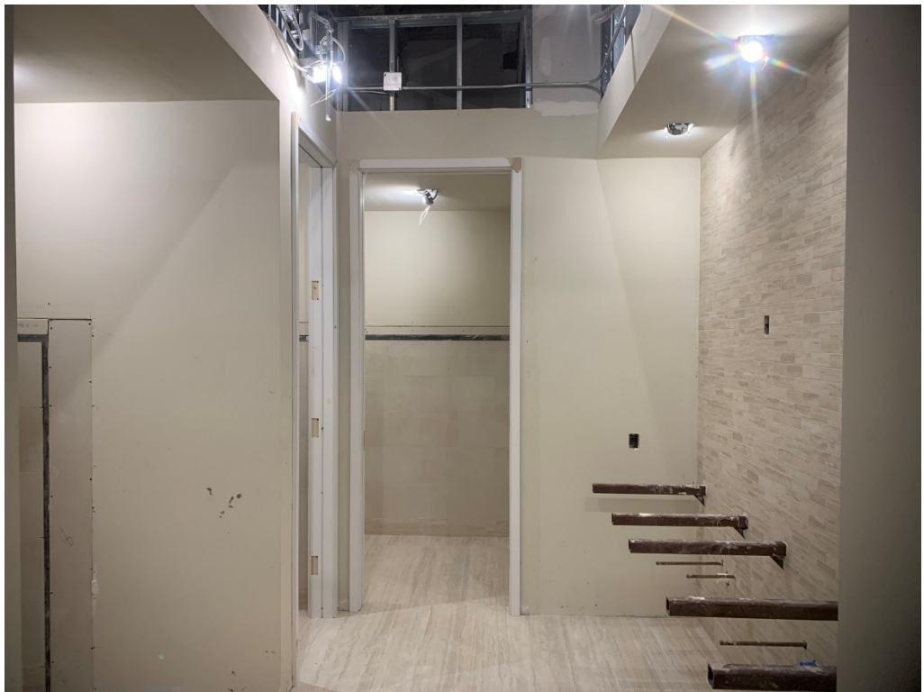
Figure 14 – Tile is ongoing at toilet rooms
