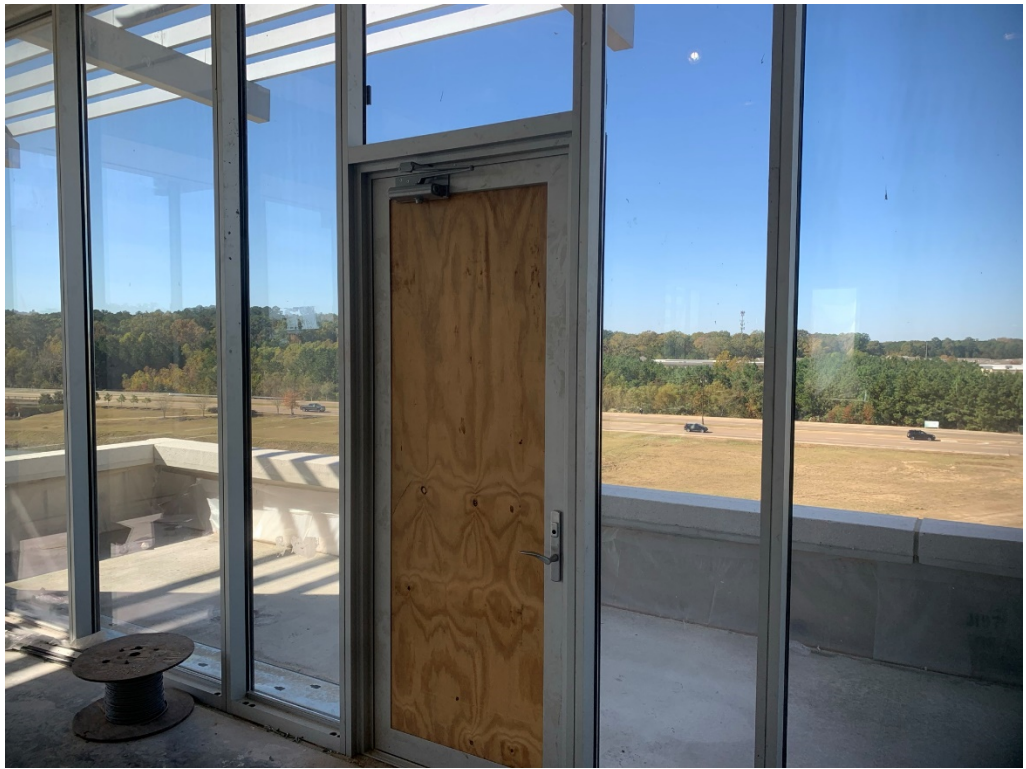
Figure 23 – Door hardware installed
