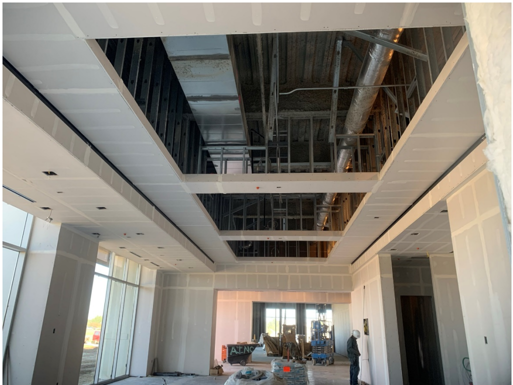
Figure 12 – Ceiling work at 1 st floor
