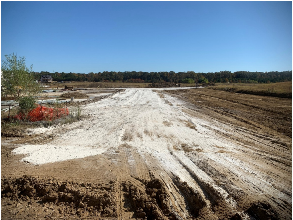
Figure 5 – Lime at sitework is ongoing
