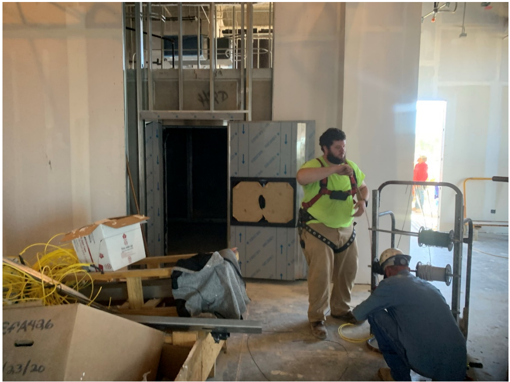
Figure 11 – Electrical is ongoing
