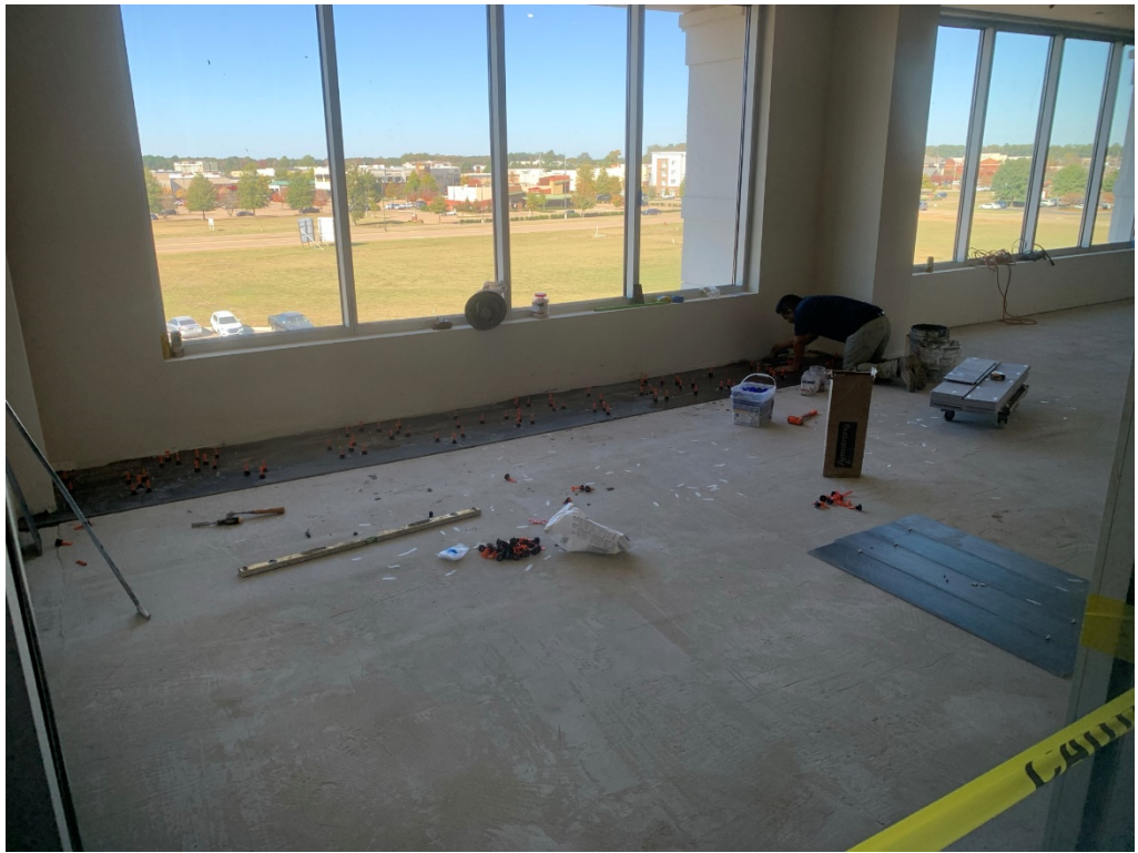
Figure 17 – Tile at break room is started and ongoing
