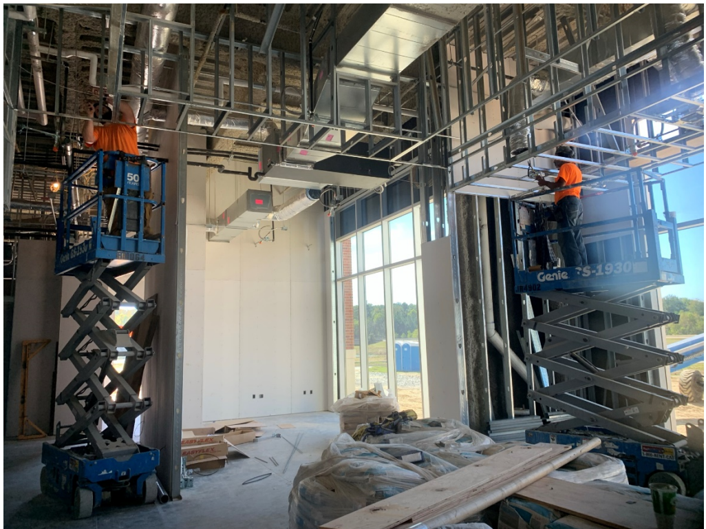
Figure 8 – Electrical is Ongoing
