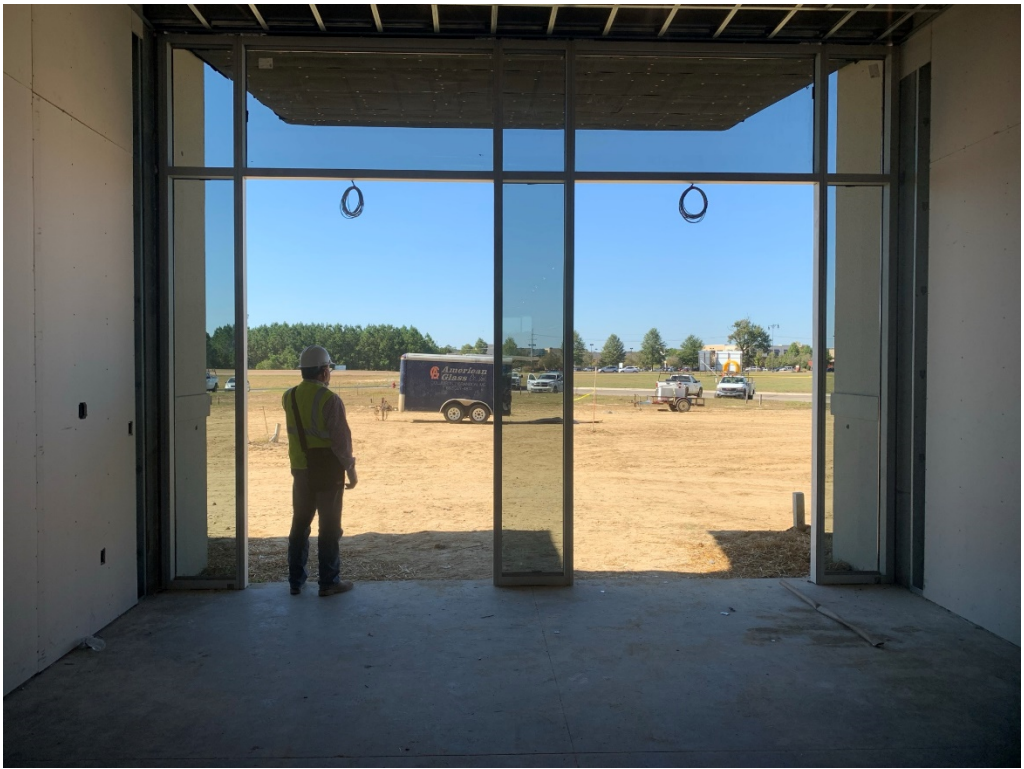
Figure 9 – Storefront install is ongoing
