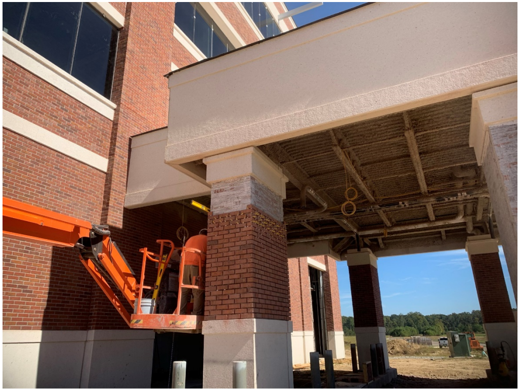
Figure 7 – Panel Rework at the drive thru is ongoing
