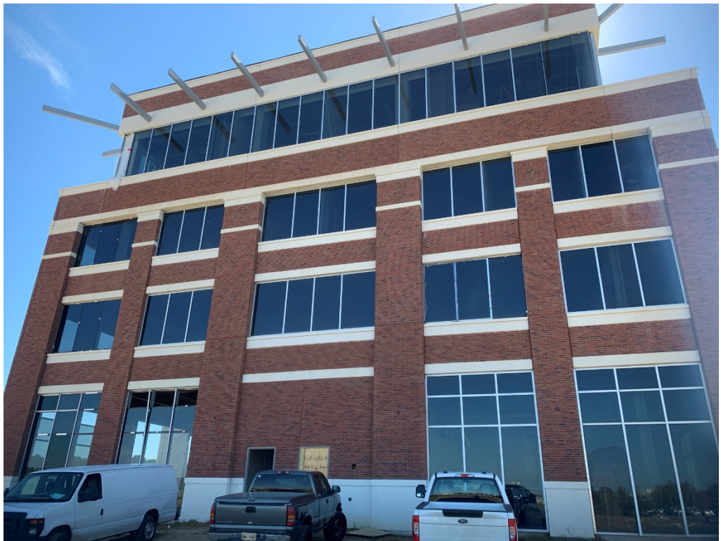
Figure 2 – North Façade Progress
