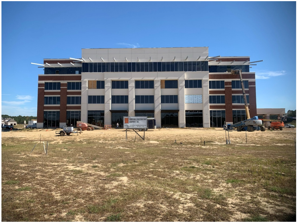
Figure 1 – West Façade Progress
