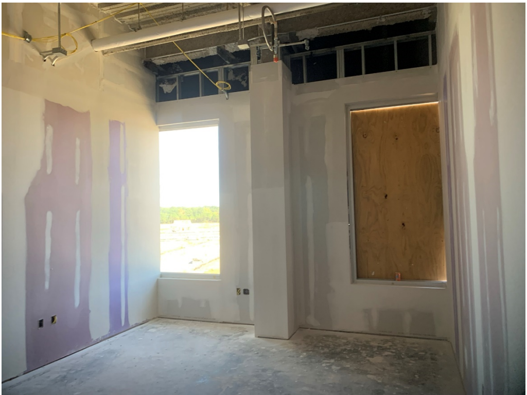
Figure 10 – Drywall is ongoing
