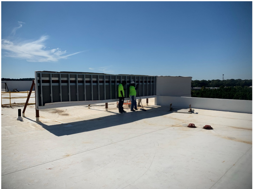
Figure 12 – Roof work in ongoing
