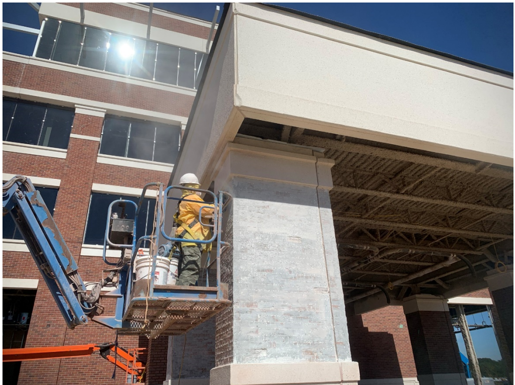
Figure 6 – Panel Rework at the drive thru is ongoing
