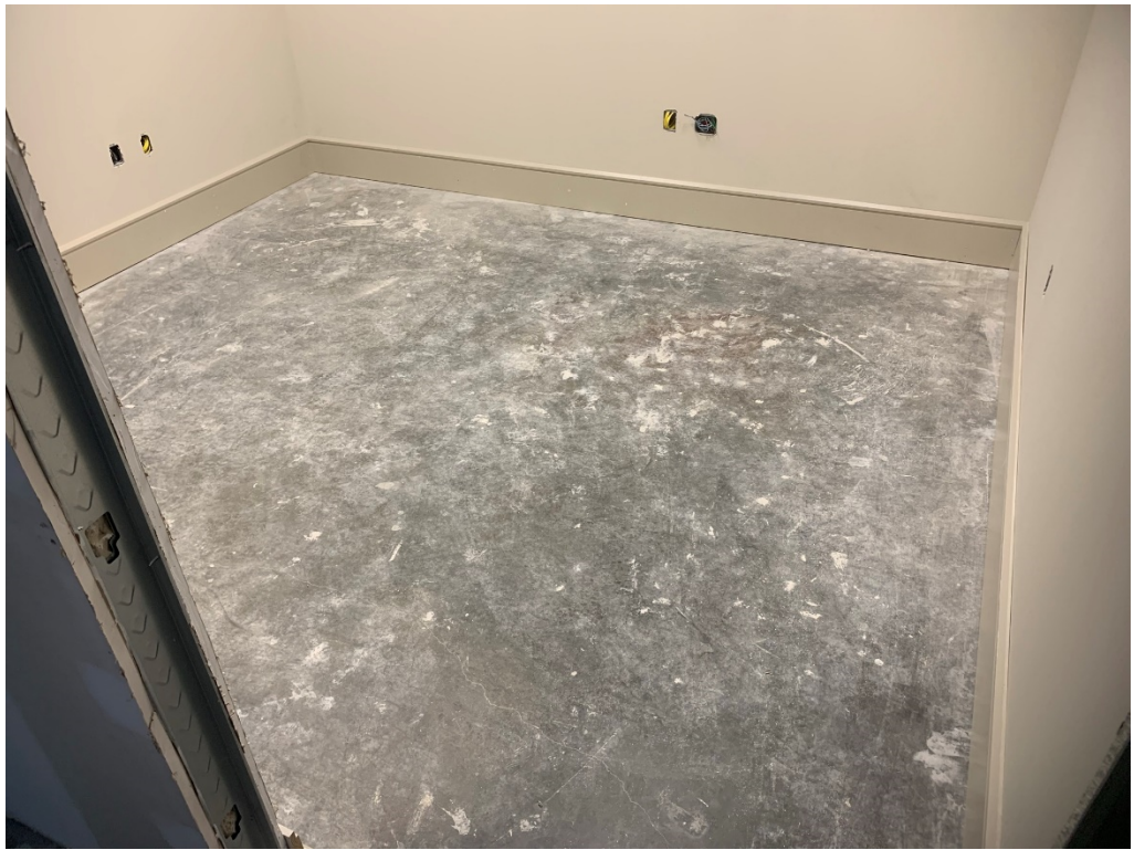
Figure 11 – Base trim install has begun
