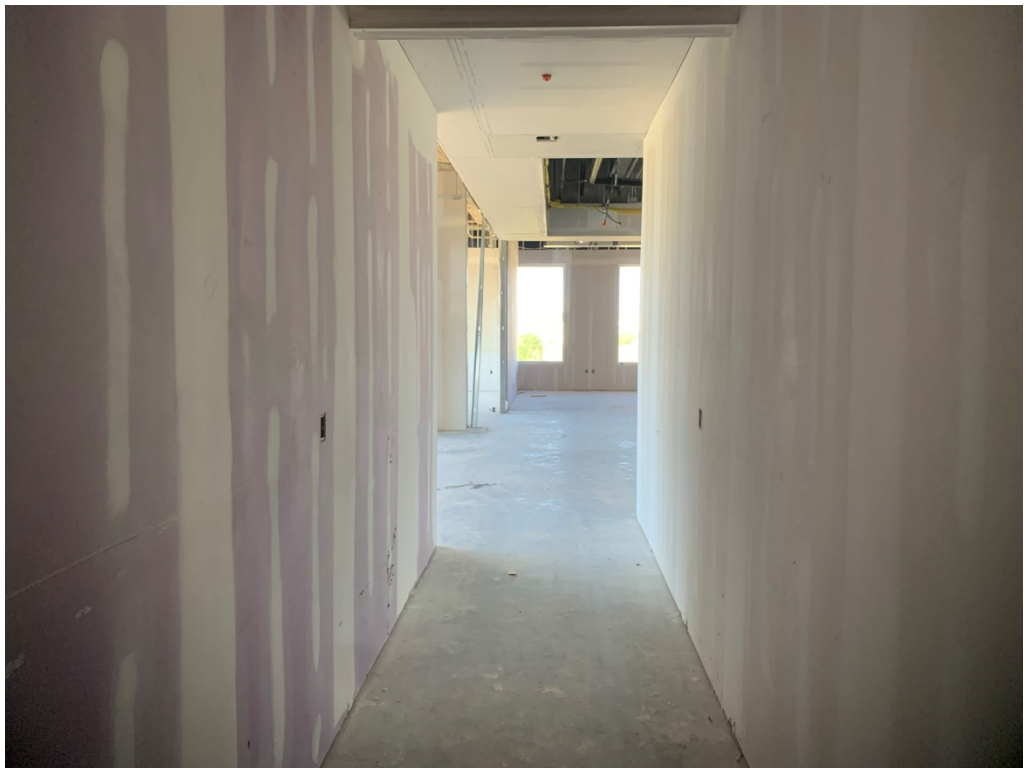
Figure 8 – Drywall finishing is on going @ 3 rd Floor
