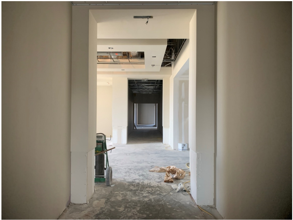
Figure 11 – A large portion of the 4 th floor has at least 1 coat
