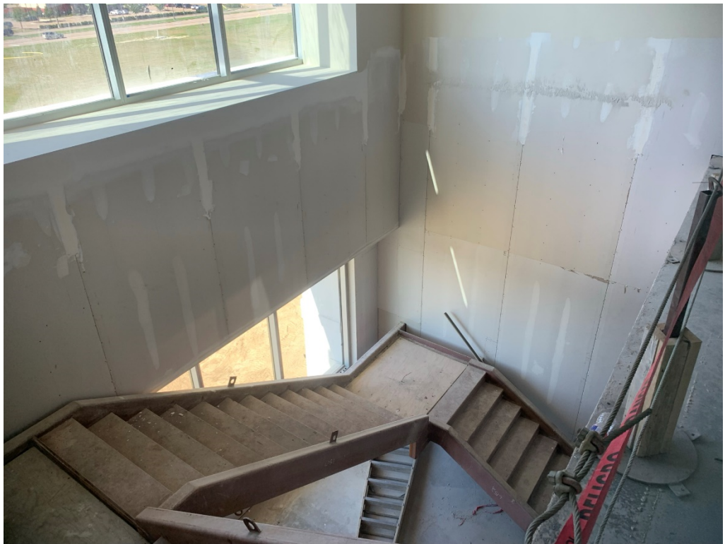
Figure 10 – Monumental Stair Progress
