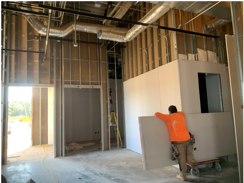
Figure 6 – Drywall at 1sr Floor is ongoing
