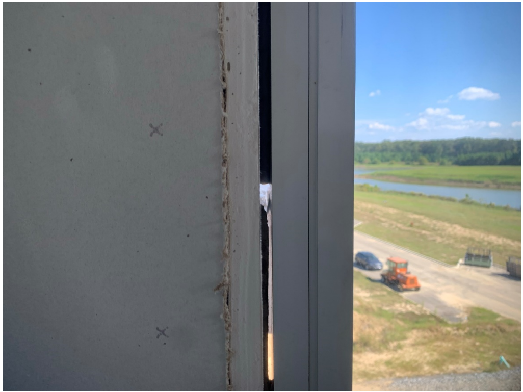
Figure 7 – Sealant at AL Storefront is ongoing
