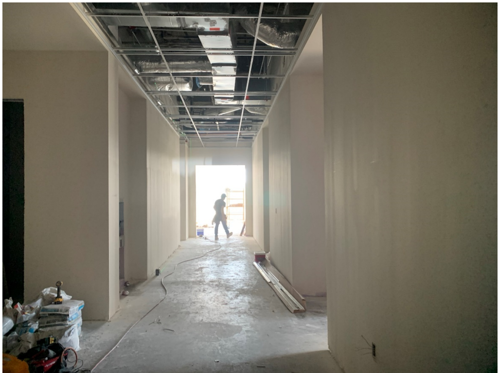
Figure 12 – Ceiling Work is Ongoing at 4 th Floor
