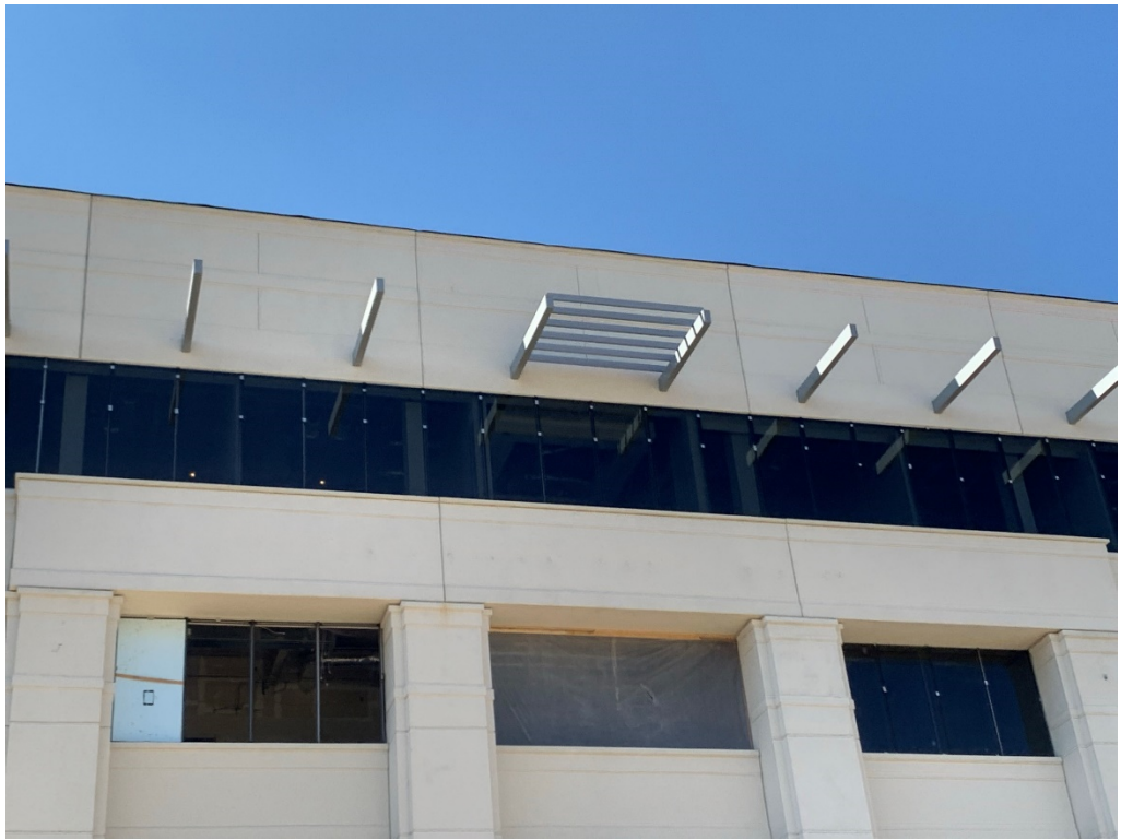
Figure 5 – Sun Shade Section Installed
