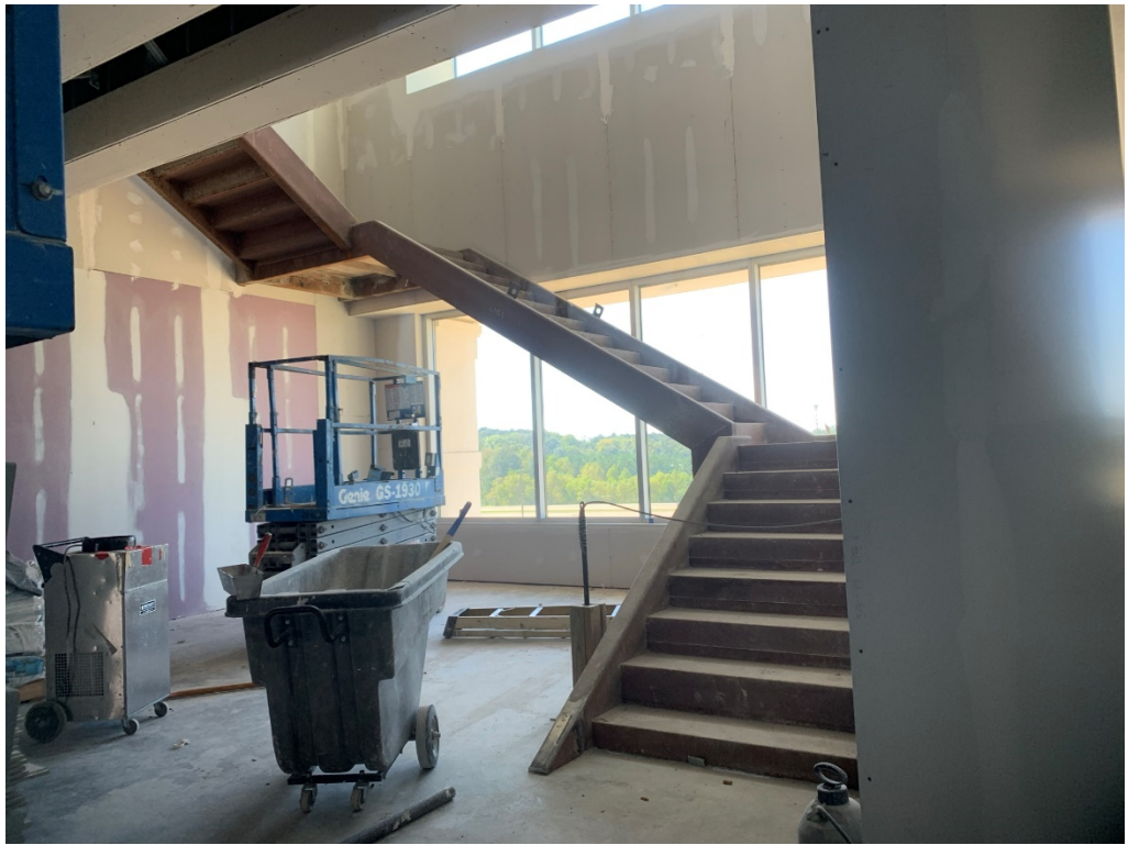
Figure 9 – Monumental Stair Progress
