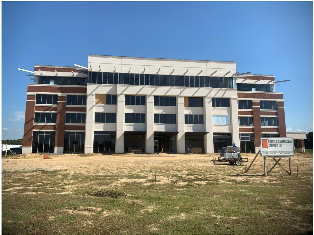
Figure 1 – West Façade Progress
