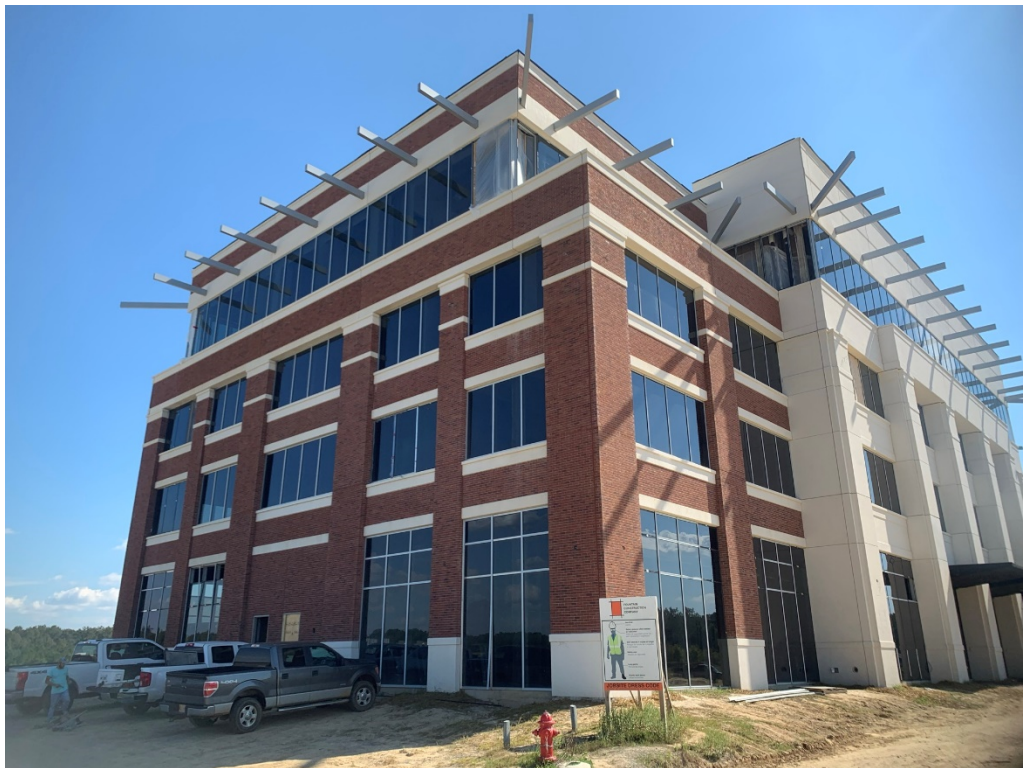
Figure 2 – North Façade Progress
