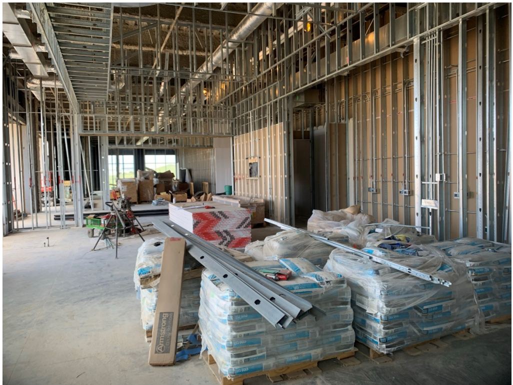
Figure 8 – 1 st Floor West Lobby
