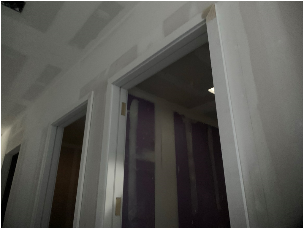
Figure 13 – Wood Jamb Installation @ Exec. Tlts
