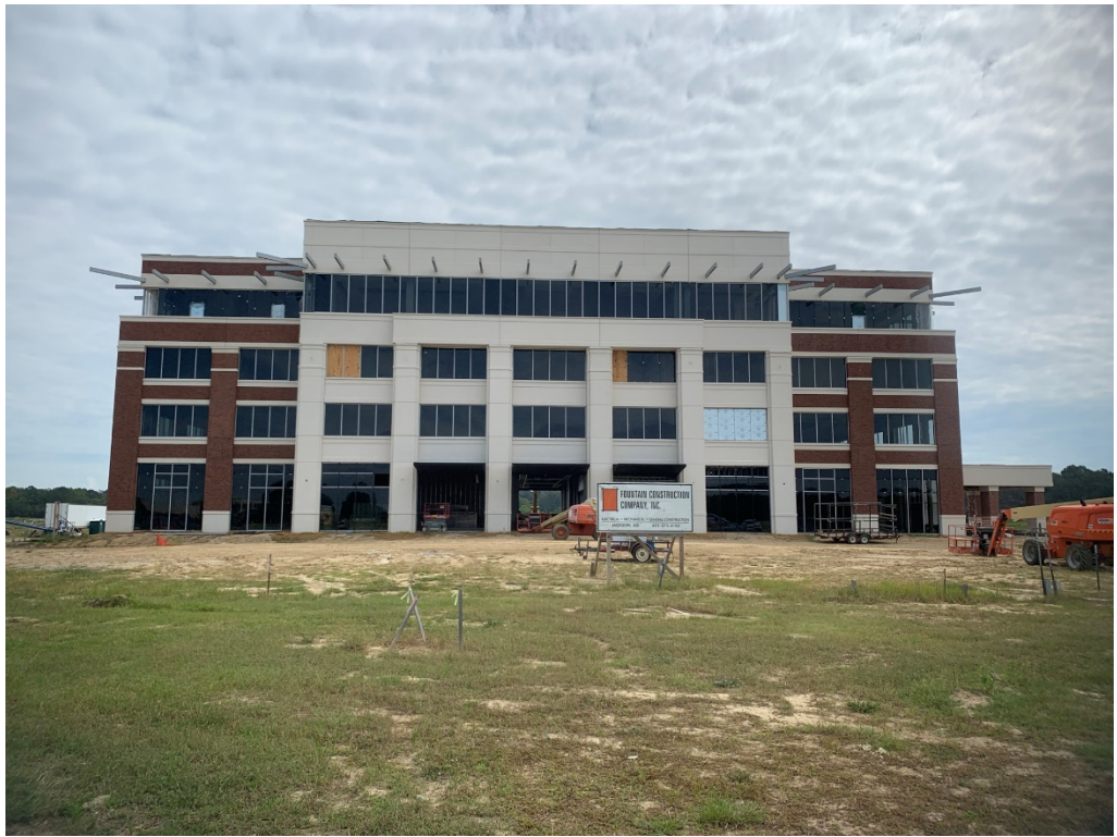
Figure 1 – West Façade Progress
