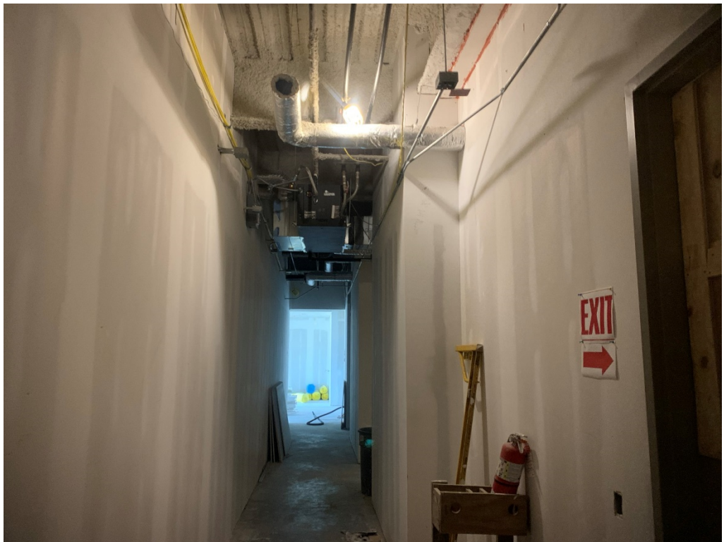
Figure 10 – Drywall is Ongoing
