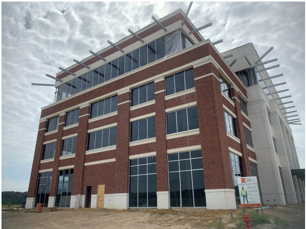
Figure 2 – North Façade Progress
