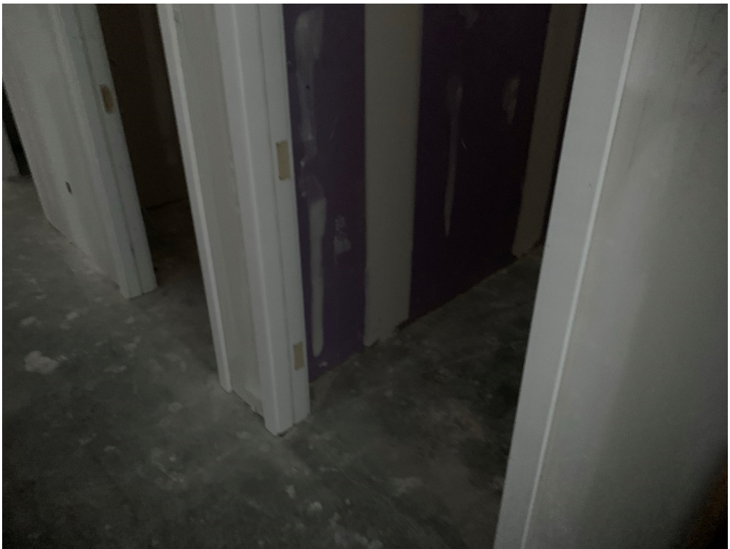
Figure 14 – Wood Jamb Installation @ Exec. Tlts
