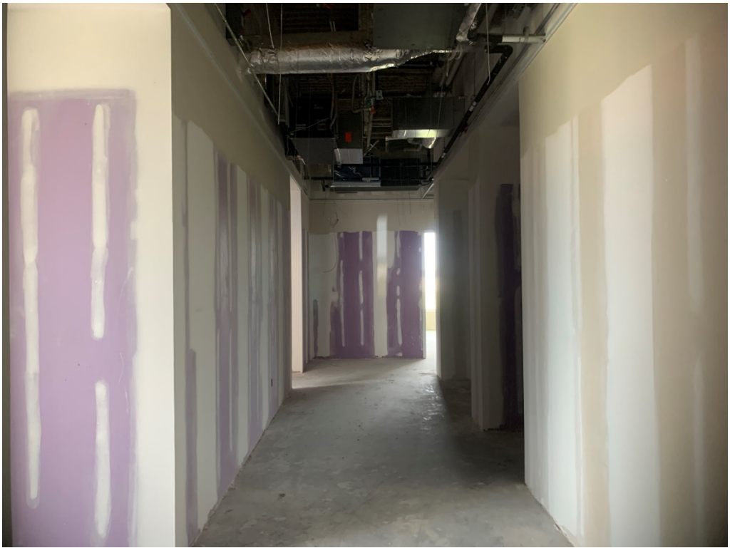
Figure 11 – Drywall is Ongoing
