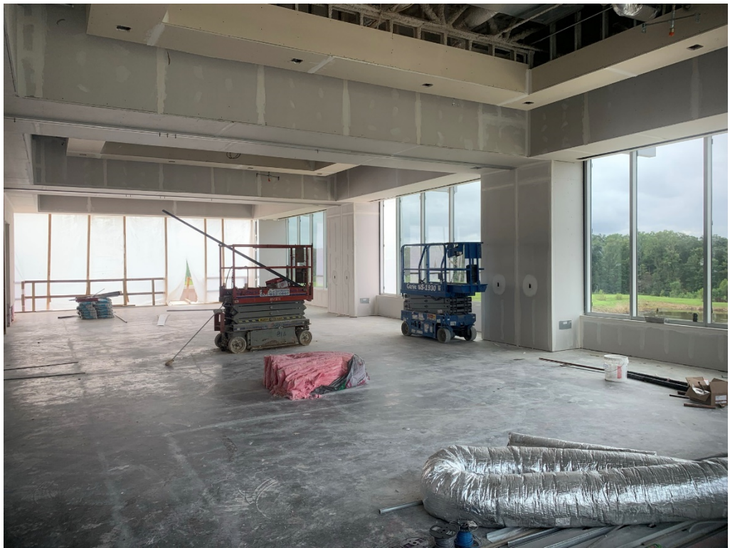
Figure 16 – Continued Drywall at Banquet 4 th Floor
