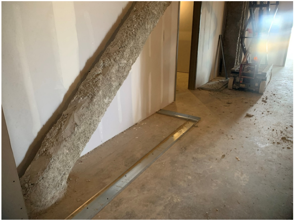
Figure 7 – Framing at the first floor is ongoing
