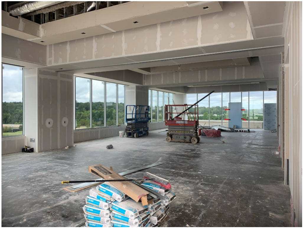
Figure 15 – Continued Drywall at Banquet 4 th Floor
