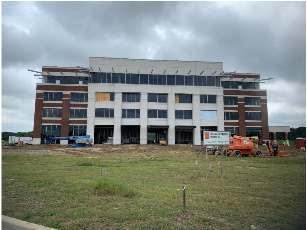
Figure 1 – West Façade Progress
