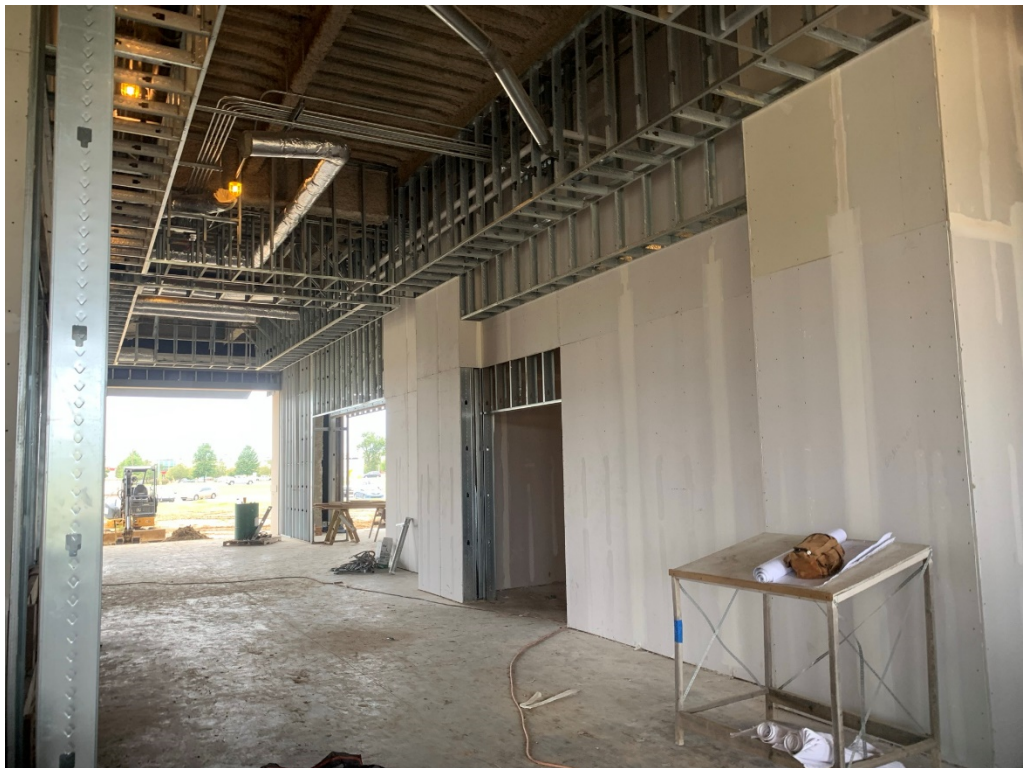
Figure 8 – Ceiling Framing at the First Floor
