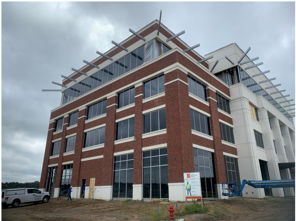
Figure 2 – North Façade Progress
