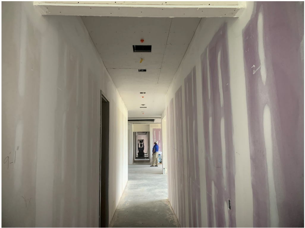
Figure 13 – Hard Ceiling Installation at the 3 rd Floor
