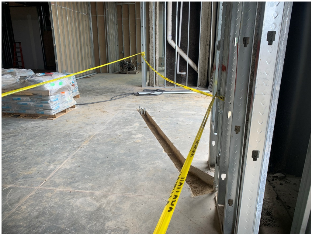
Figure 6 – Trenches for added conduit
