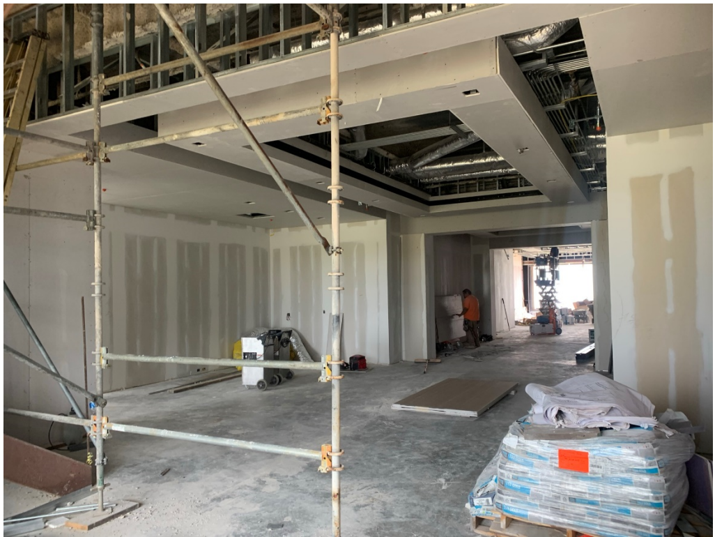
Figure 14 – Hard Ceiling Installation at the 3 rd Floor
