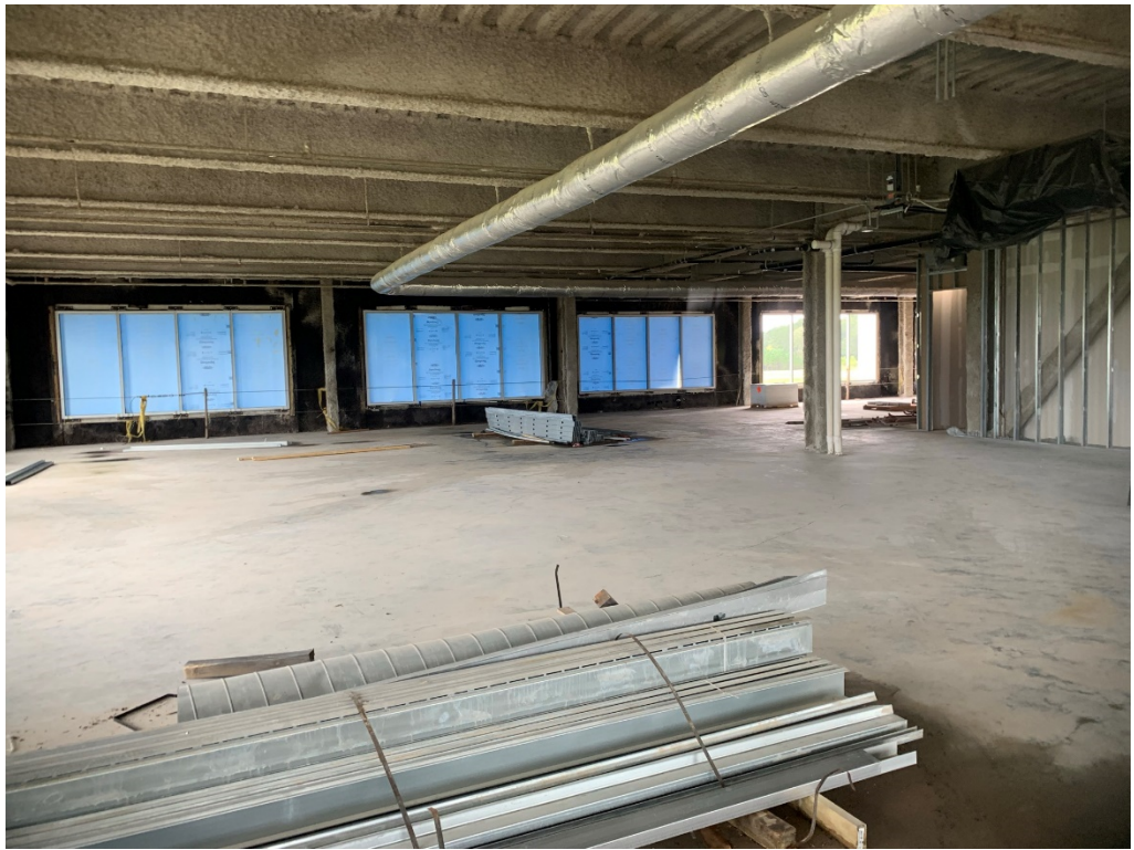
Figure 9 – rigid insulation installed at windows
