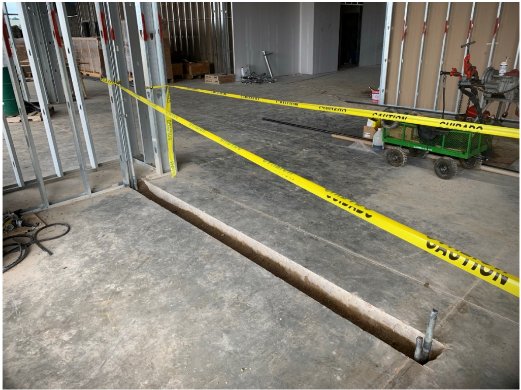
Figure 5 – Trenches for added conduit
