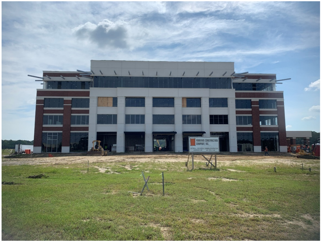
Figure 1 – West Façade Progress
