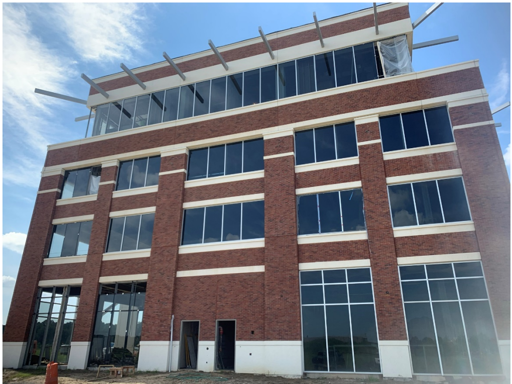
Figure 2 – North Façade Progress
