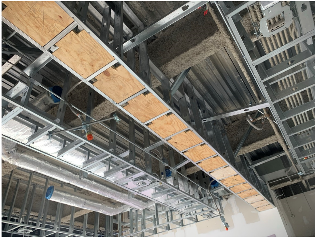
Figure 9 – Blocking and Framing are ongoing
