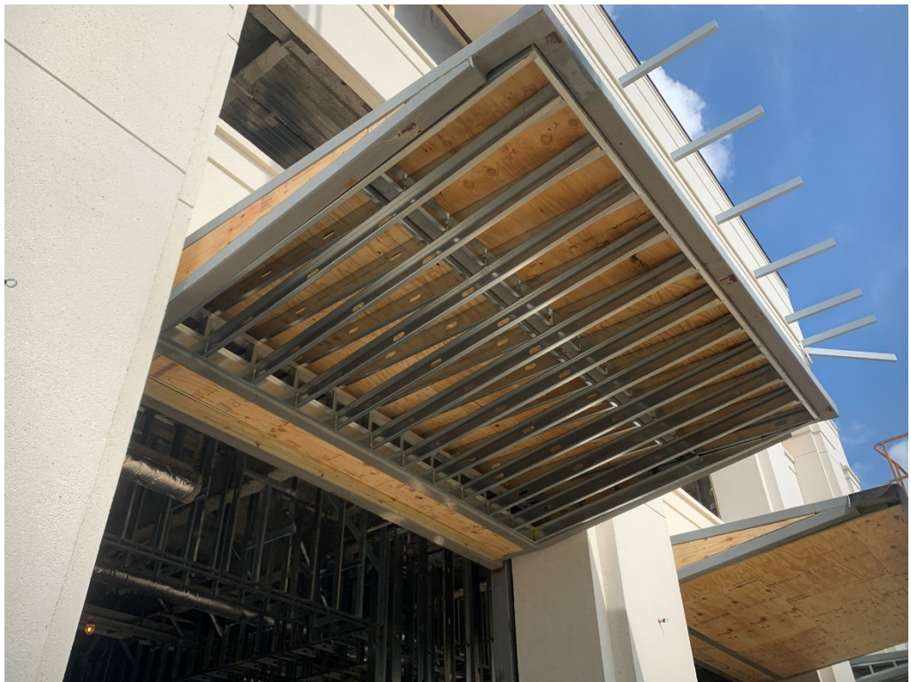
Figure 6 – Awning Decking and Roofing work
