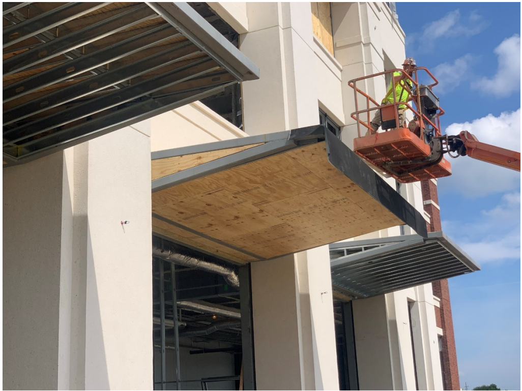
Figure 5 – Awning Decking and Roofing work
