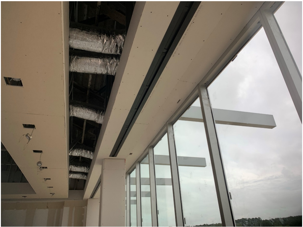
Figure 7 – Boardroom Ceiling and Glazing Progress
