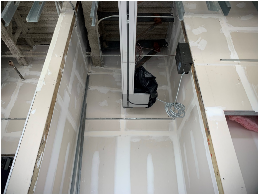
Figure 11 – Sliding Tracks Installed
