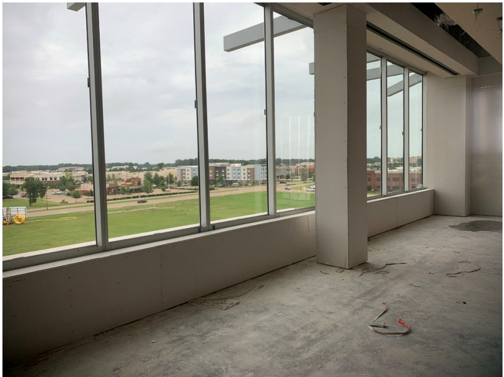
Figure 6 – Framing & Gypsum at Board Room Exterior Wall
