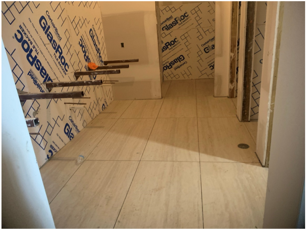
Figure 5 – Tile is installed in both 4 th floor main bathrooms
