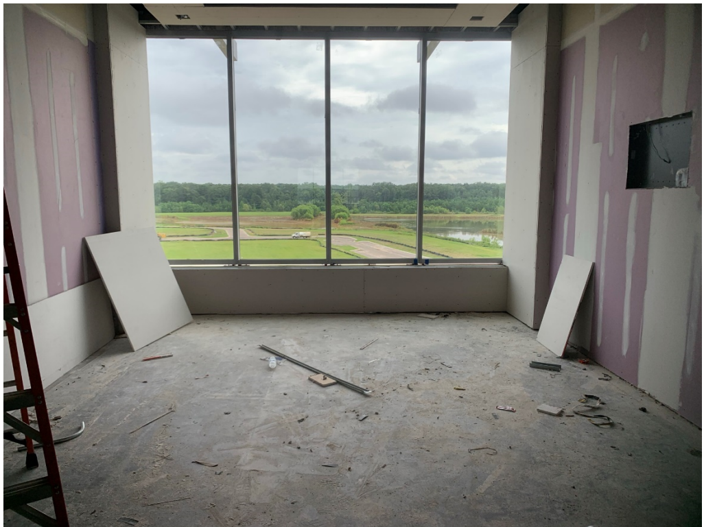
Figure 10 – Drywall & Framing Progress where Glass Is Installed
