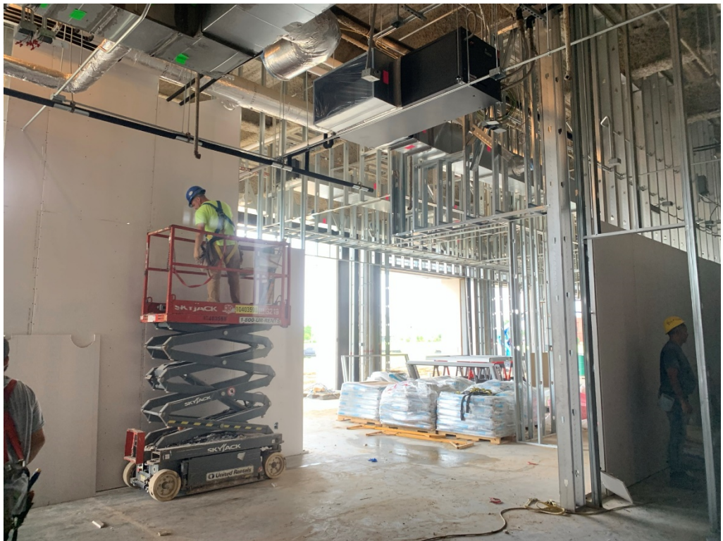
Figure 4 – Drywall Started at the 1 st Floor
