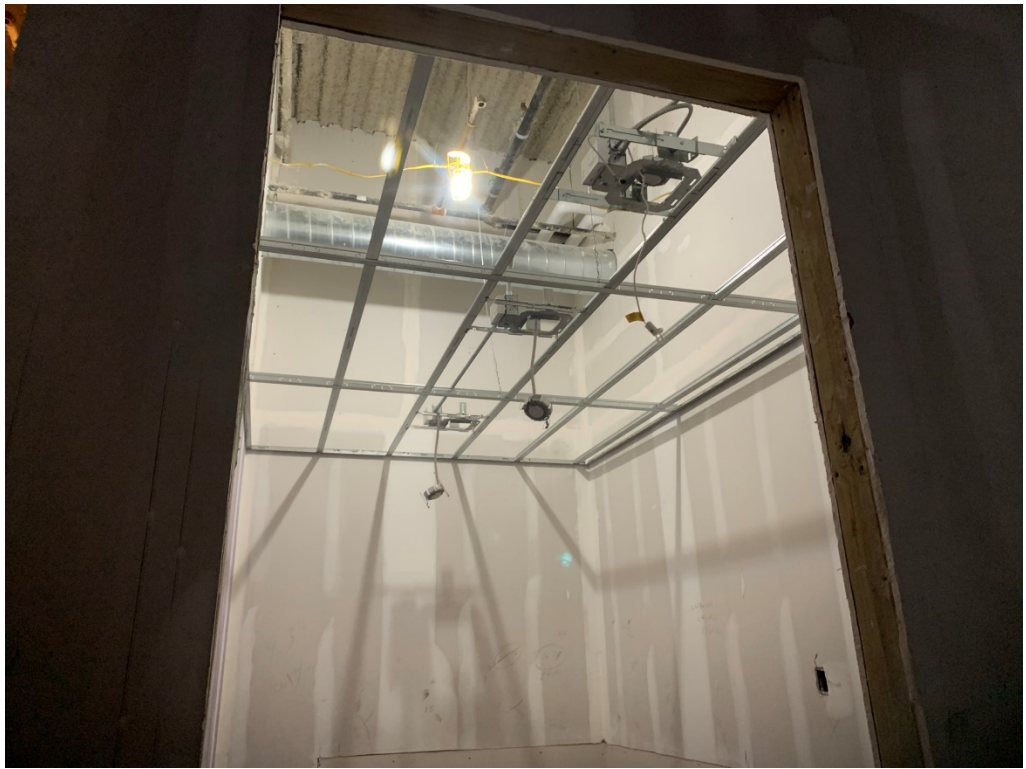
Figure 9 – Ceiling progress on 4 th Floor
