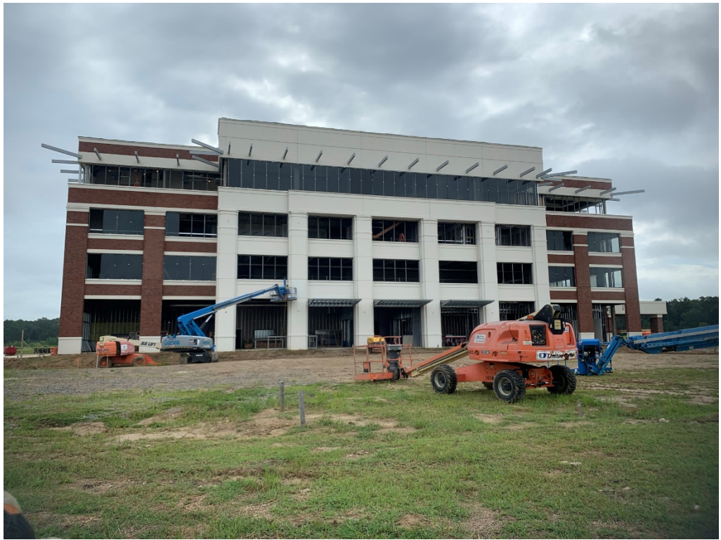
Figure 1 – West Façade Progress
