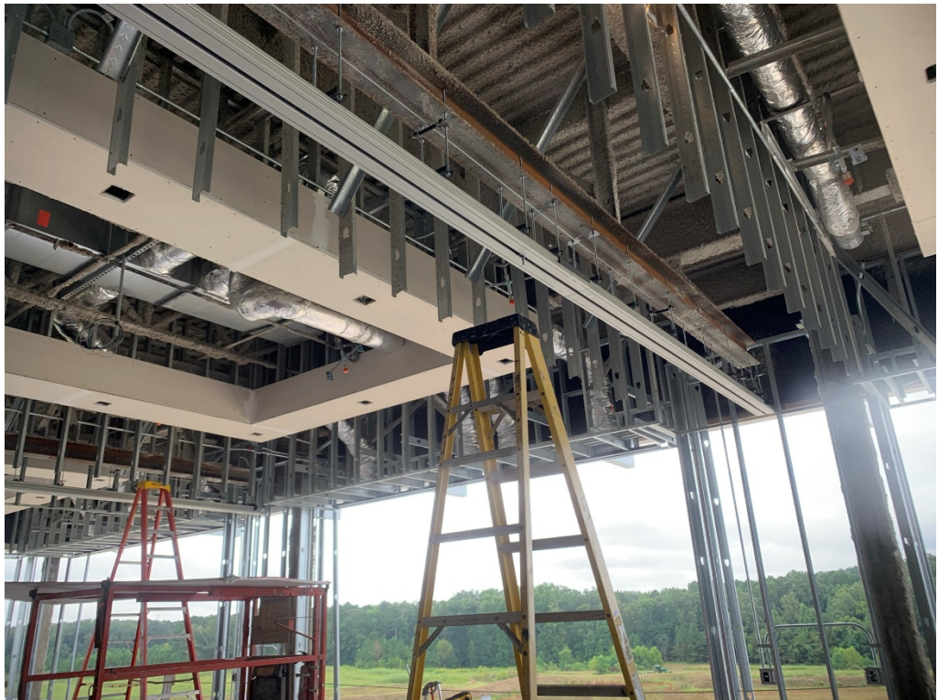
Figure 12 – Sliding Tracks Installed
