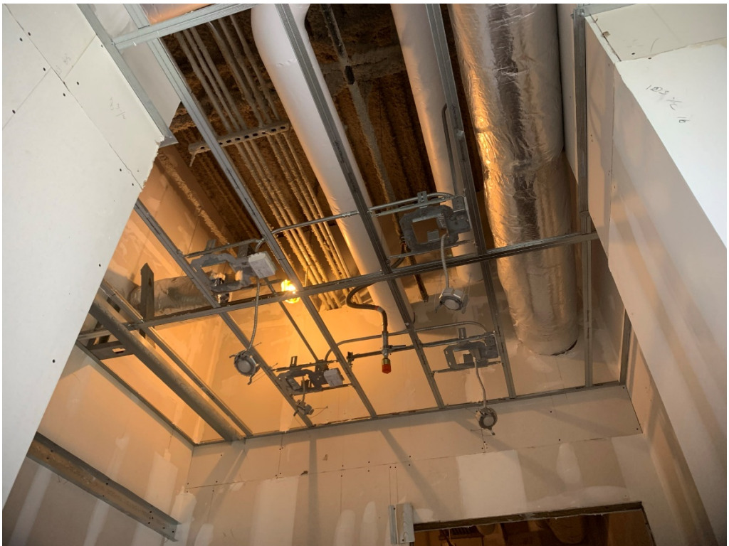
Figure 8 – Ceiling progress on 4 th Floor
