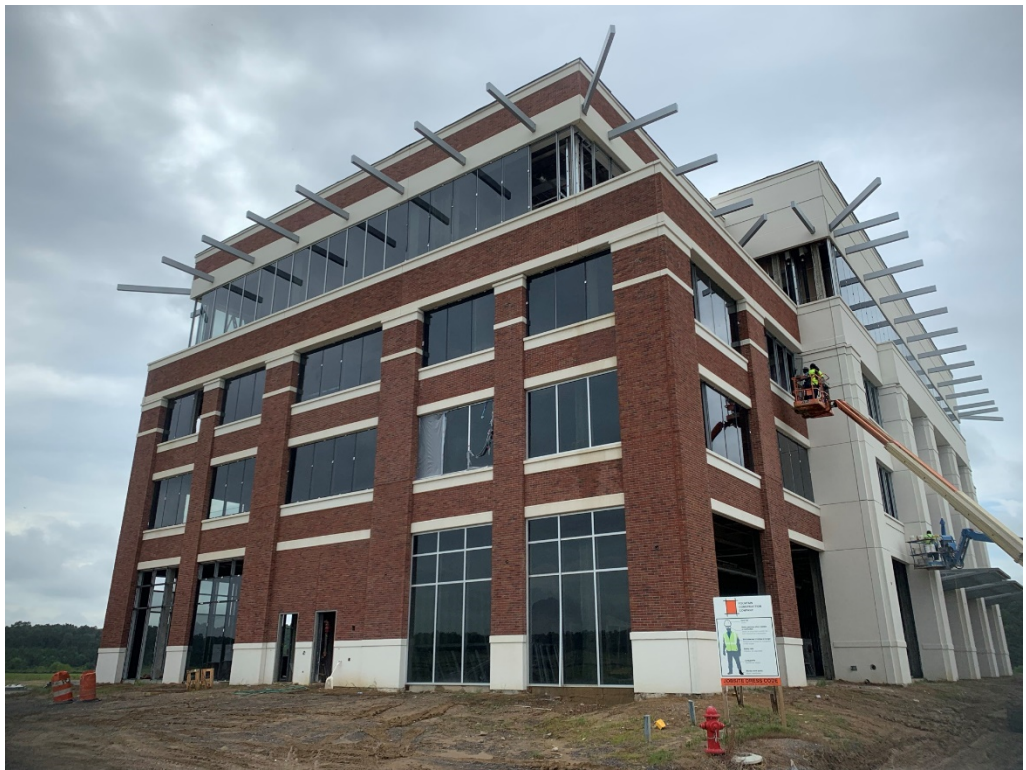
Figure 2 – North Façade Progress
