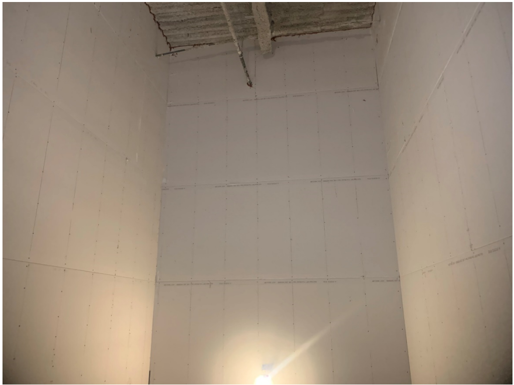
Figure 15 – South Stairwell Sheetrock Fully Installed
