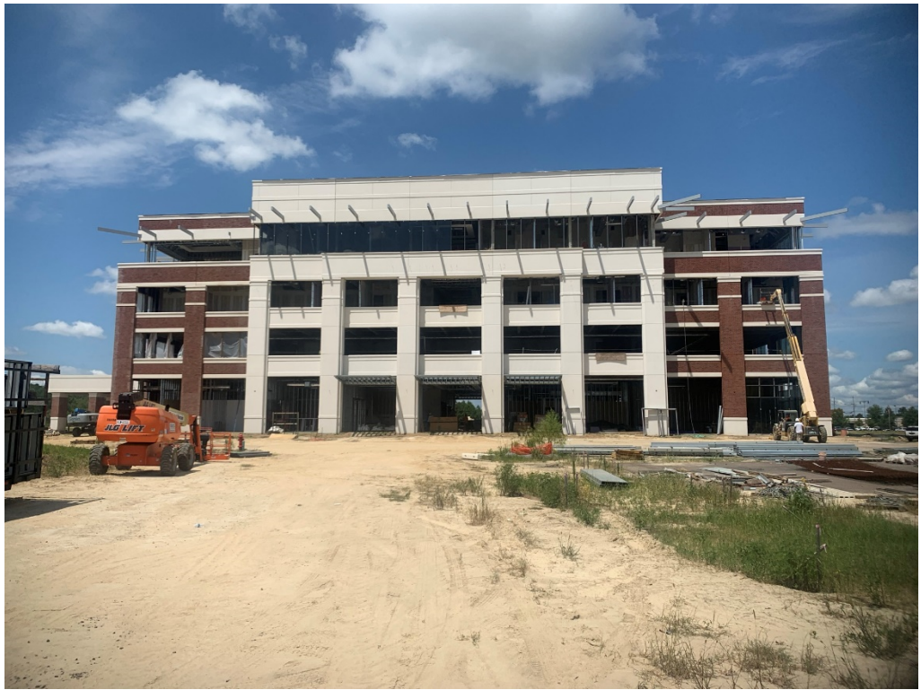
Figure 3 – East Façade Progress
