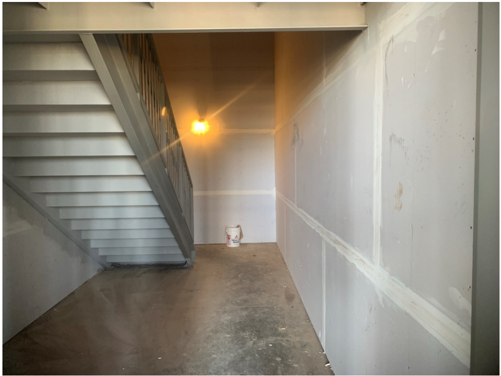
Figure 7 – South Stair Sheetrock Installed
