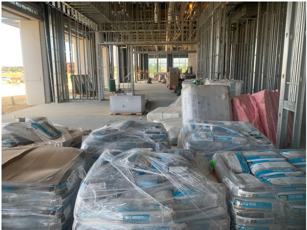
Figure 6 – Staged Mortar & Grout
