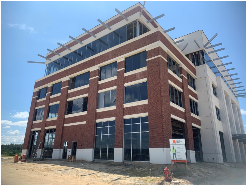
Figure 2 – North Façade Progress
