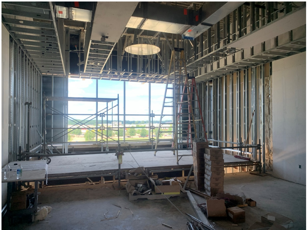
Figure 12 – Ongoing Ceiling work at 4 th Floor Monumental Stair
