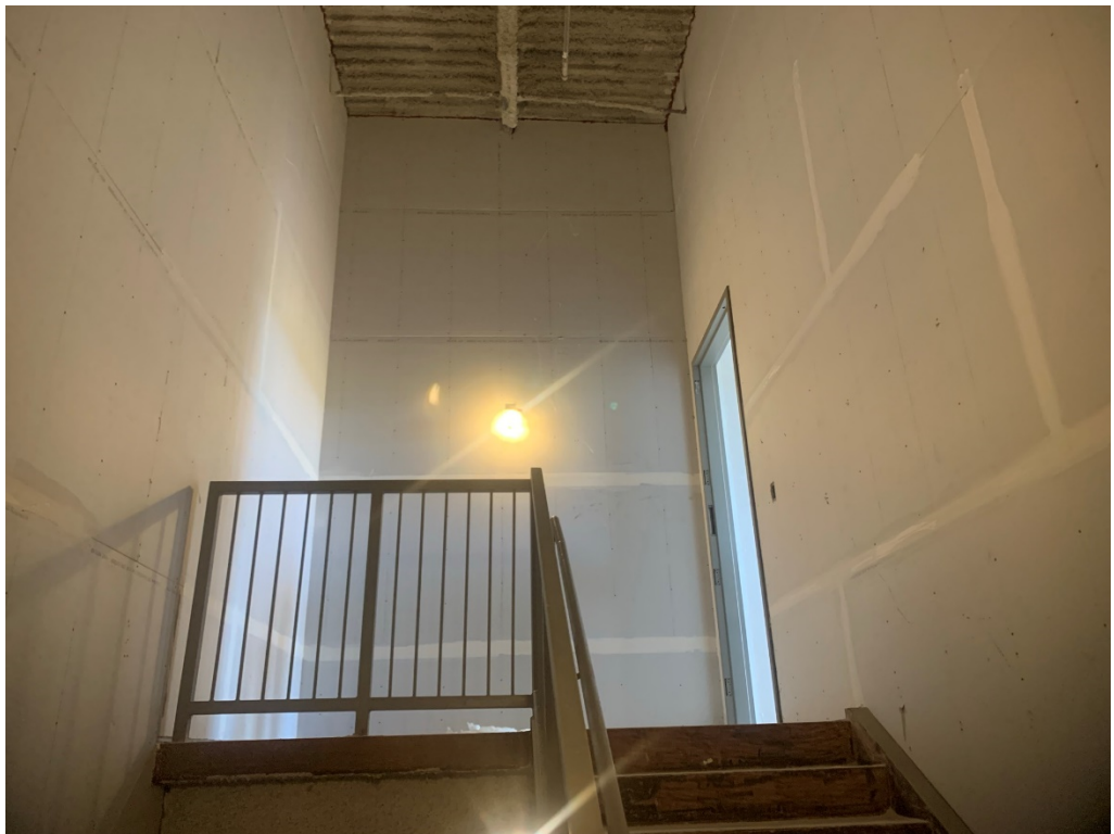
Figure 16 – South Stairwell Sheetrock Fully Installed
