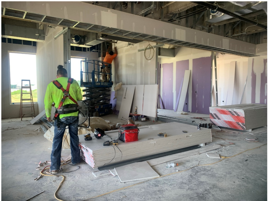
Figure 8 – Gypsum Install is Ongoing
