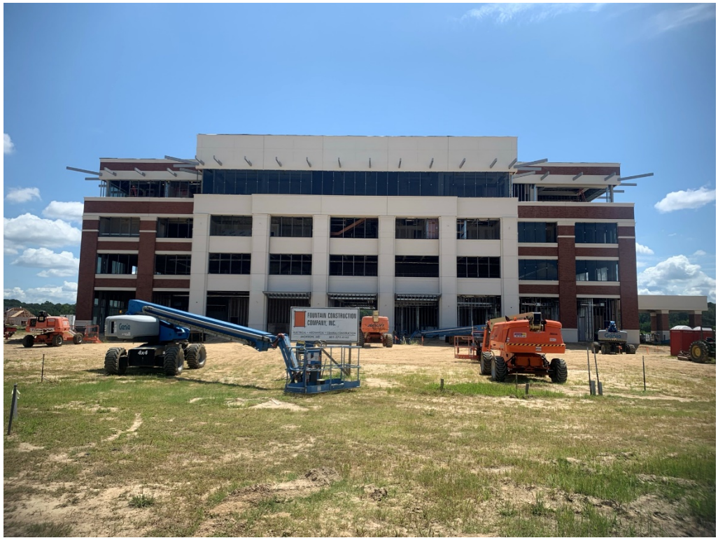
Figure 1 – West Façade Progress
