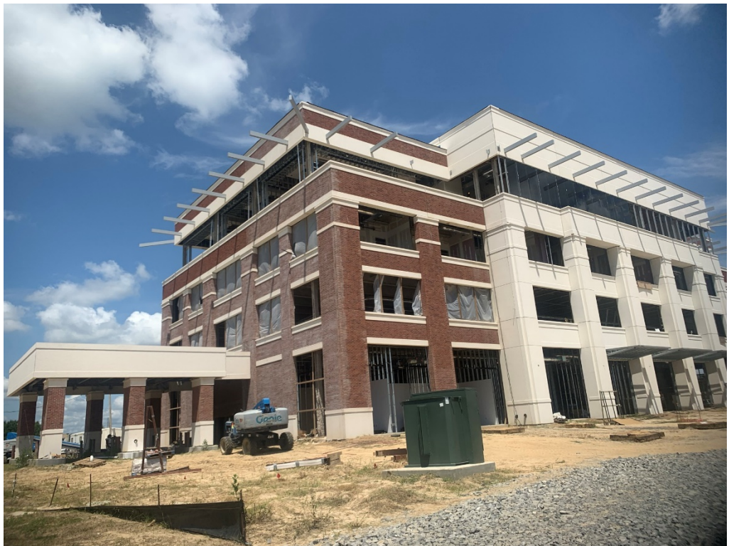
Figure 4 – South Façade Progress
