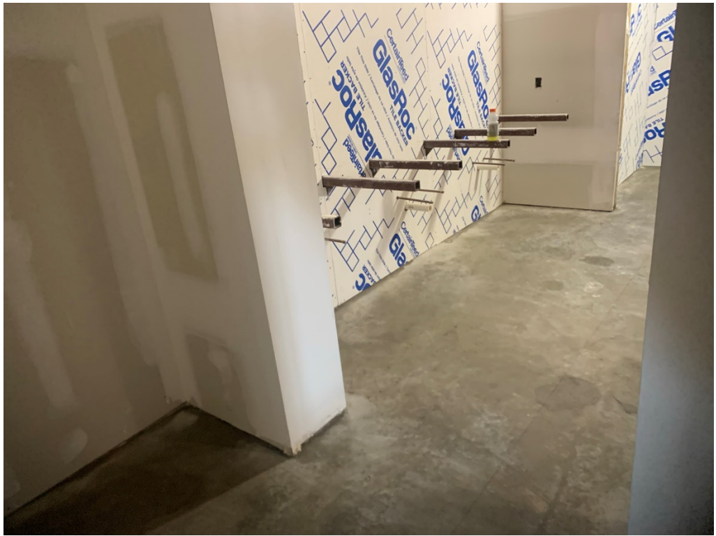
Figure 13 – Cleaned and Prepped 4 th Floor Bathroom 4005; ready for tile install
