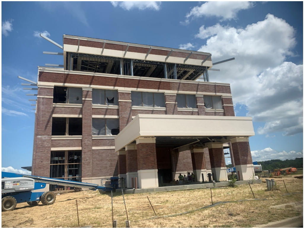
Figure 5 – South Façade Progress
