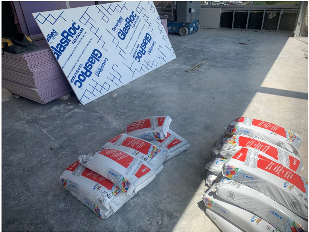
Figure 9 – Mortar Lifted to 4 th Floor for Tile Install
