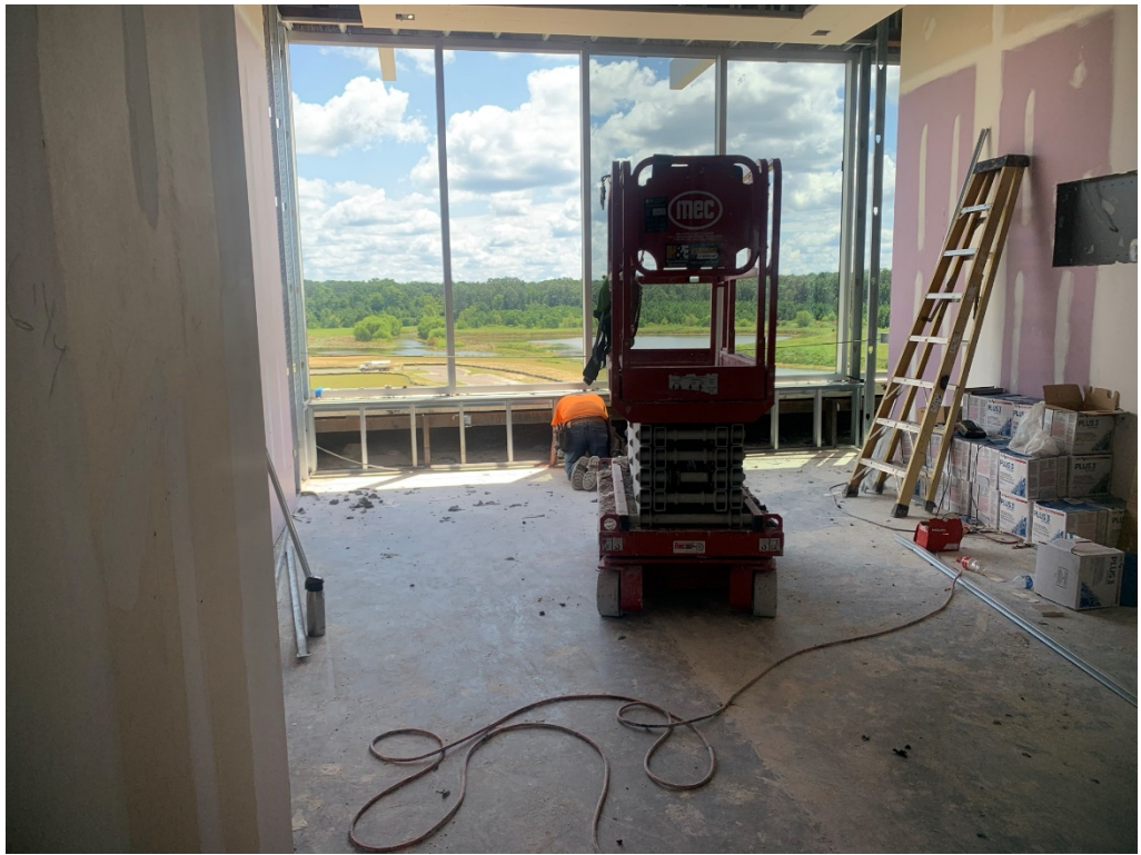
Figure 11 – Framing is Ongoing Throughout
