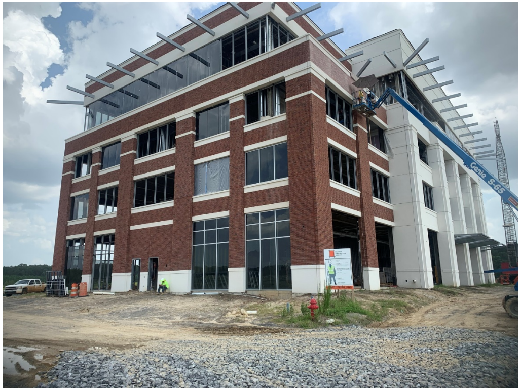
Figure 1 – Northwest Corner Progress
