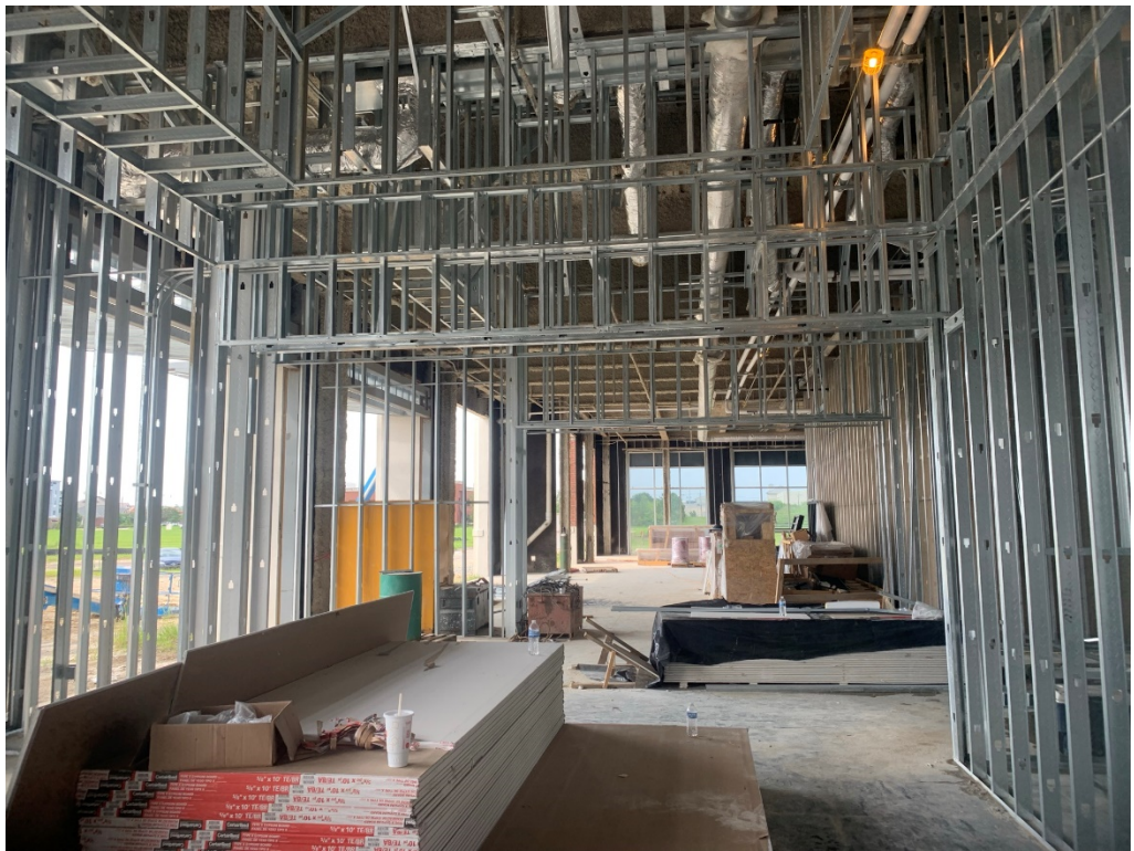
Figure 6 – Ceiling Framing @ 1 st Floor
