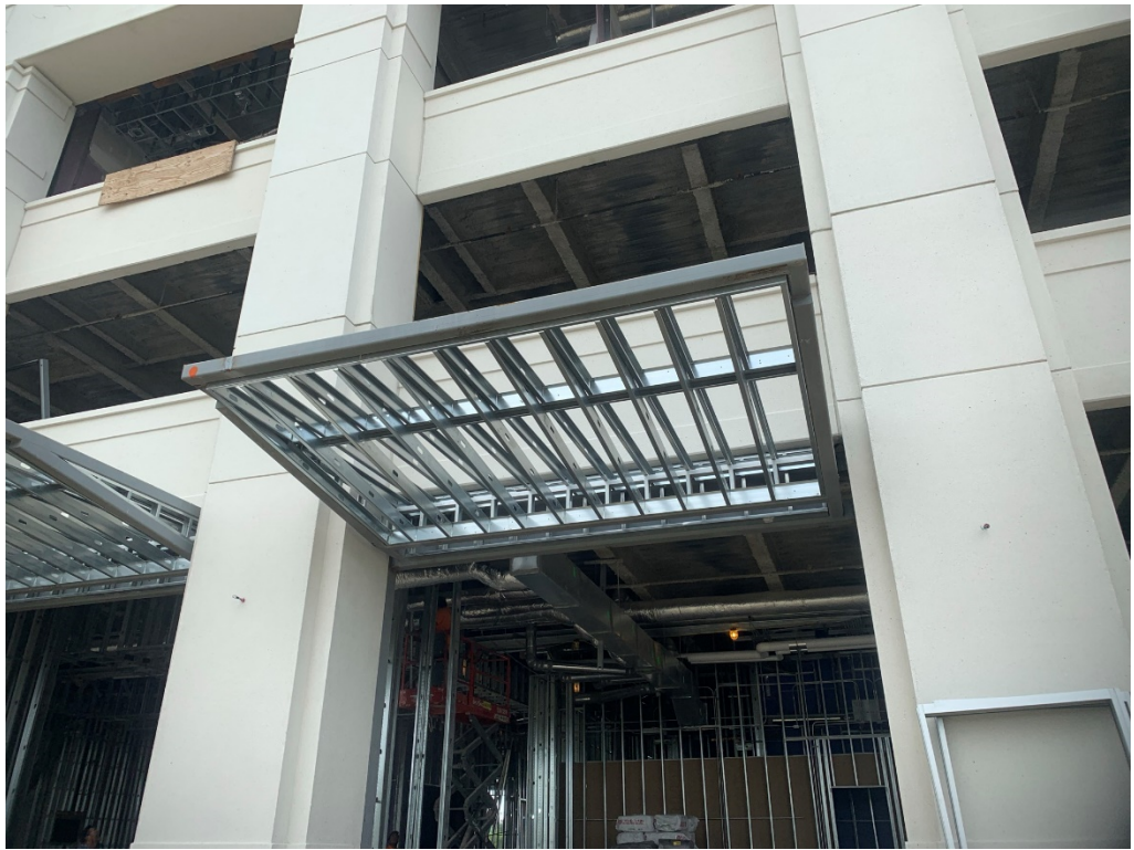
Figure 3 – Framing at Awnings
