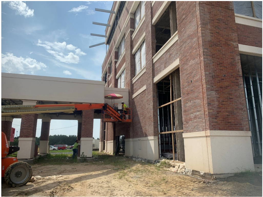
Figure 5 – Masonry is Ongoing
