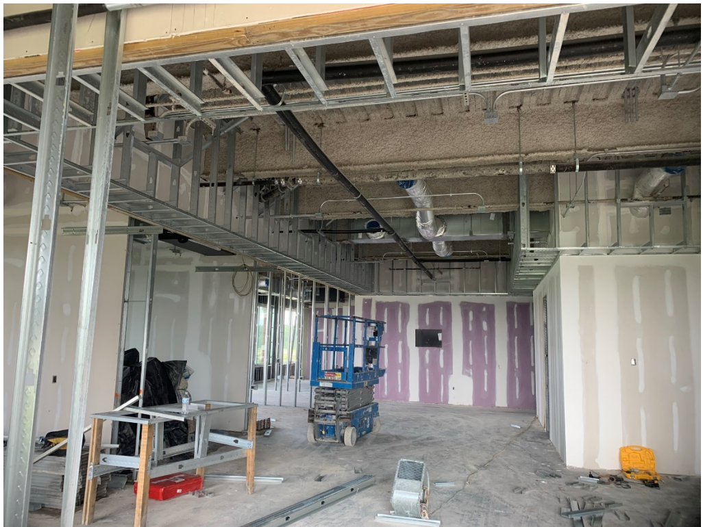
Figure 10 – Ceiling Framing @ 4 th Floor
