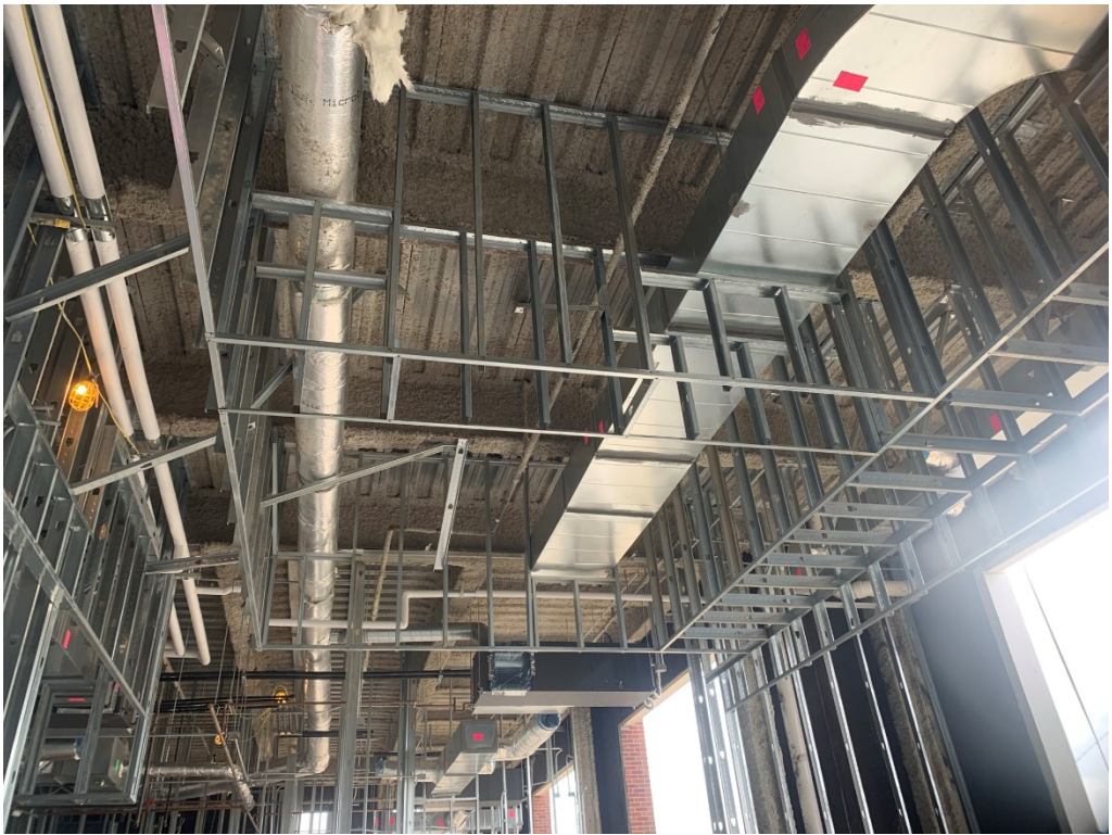
Figure 7 – Ceiling Framing @ 1 st Floor
