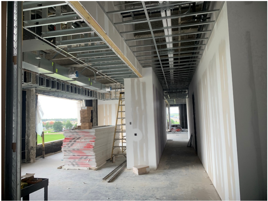
Figure 9 – Ceiling Framing @ 4 th Floor
