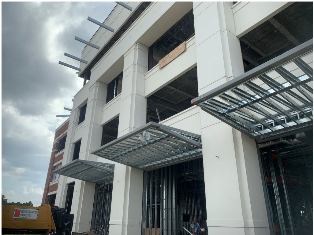
Figure 4 – Framing at Awnings
