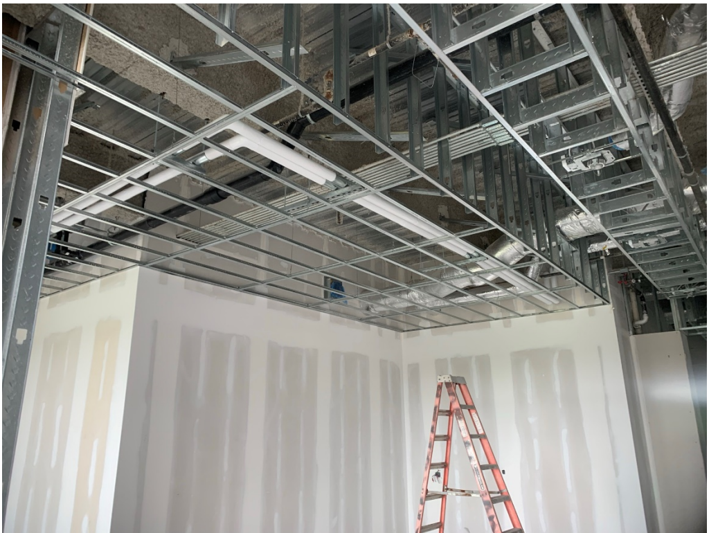
Figure 8 – Ceiling Framing @ 4 th Floor
