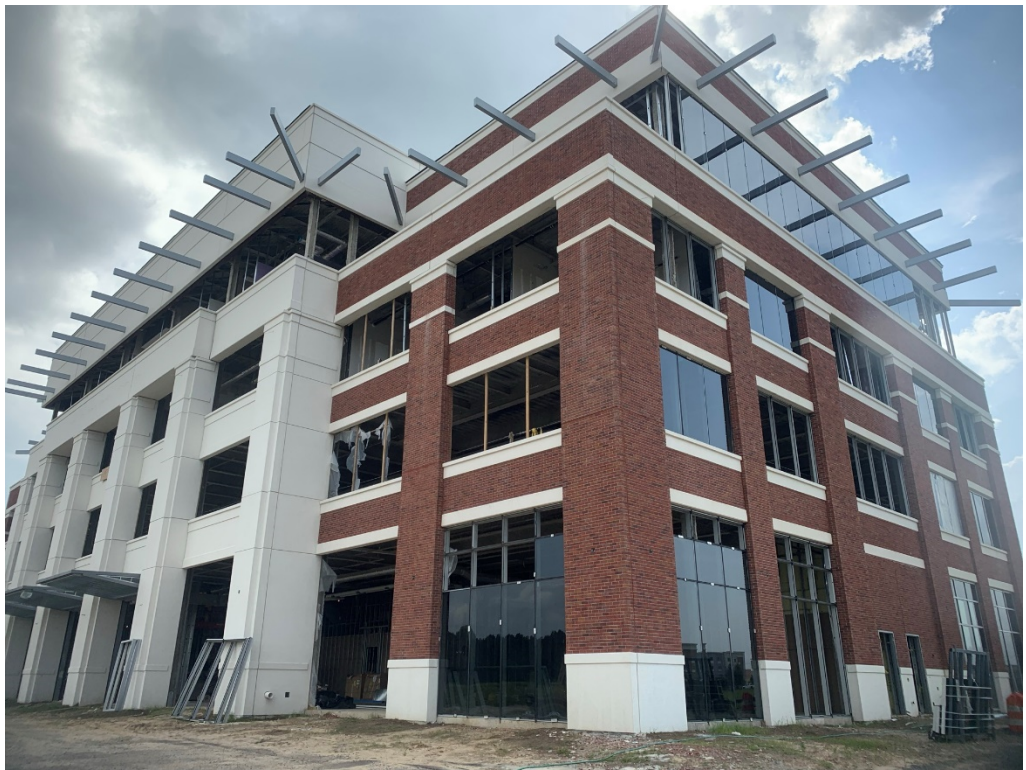
Figure 2 – Northeast Corner Progress
