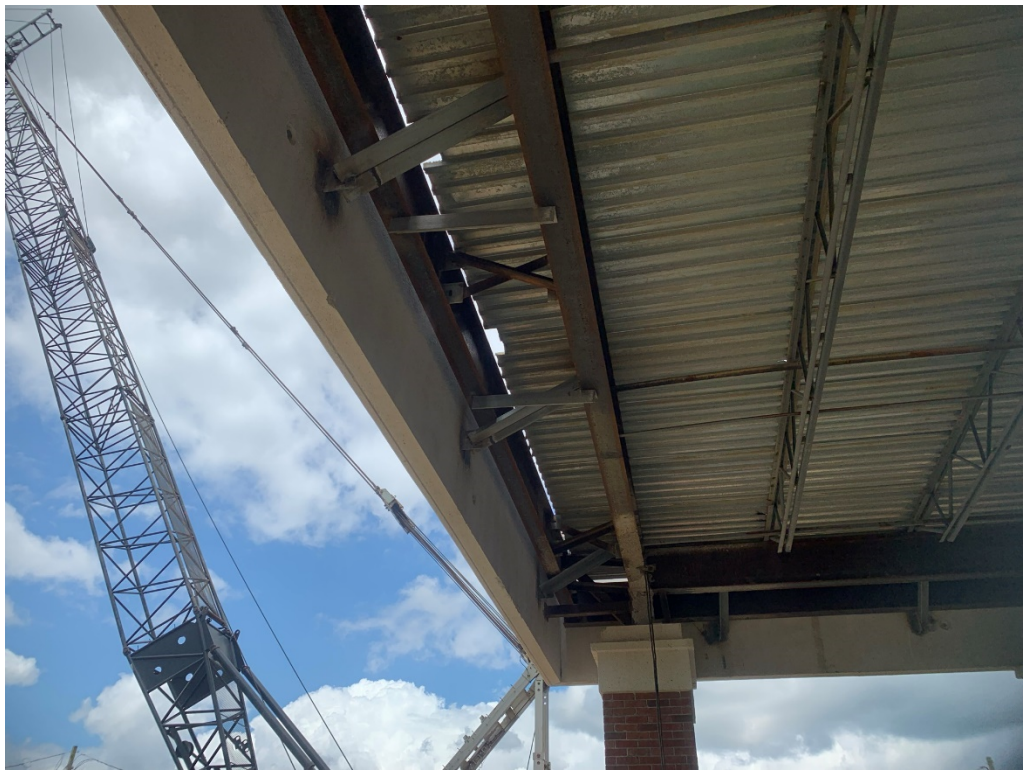
Figure 6 – Bracing at Drive Thru Canopy
