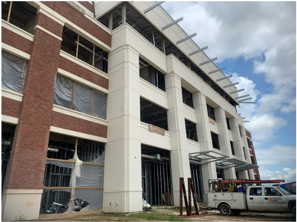
Figure 9 – East Façade Progress
