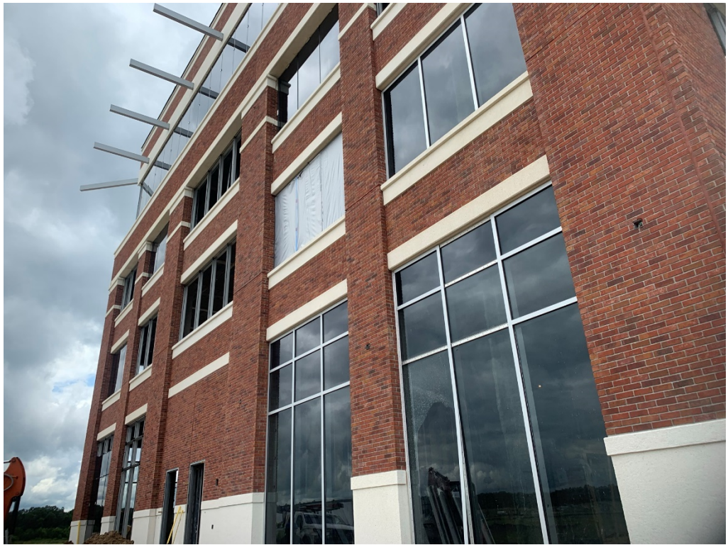
Figure 13 – North Façade Progress
