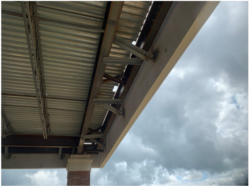
Figure 5 – Bracing at Drive Thru Canopy
