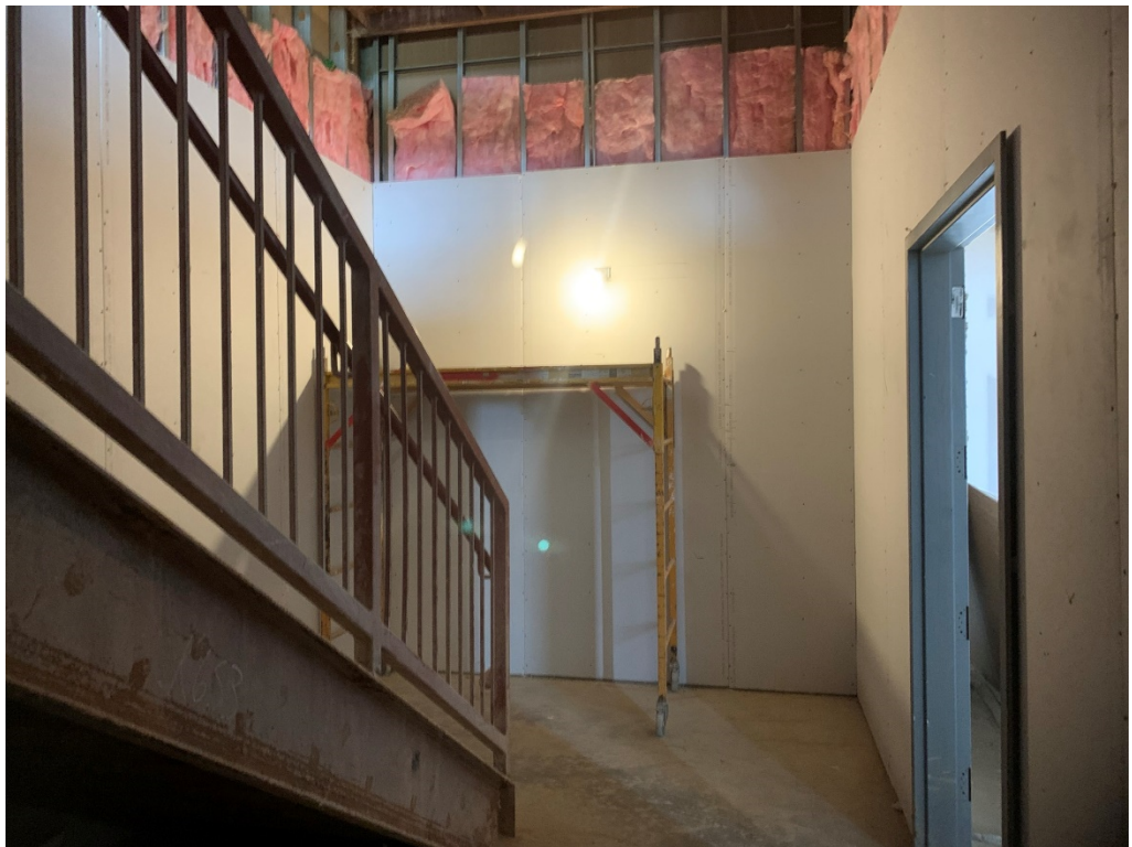
Figure 10 – Drywall Installation at North Stairwell
