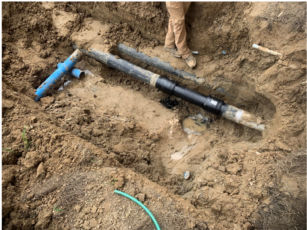
Figure 14 – Below Ground Work at North Facade
