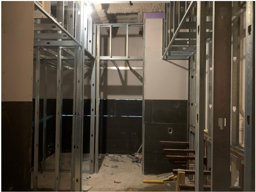
Figure 11 – 2 nd Floor Bathroom
