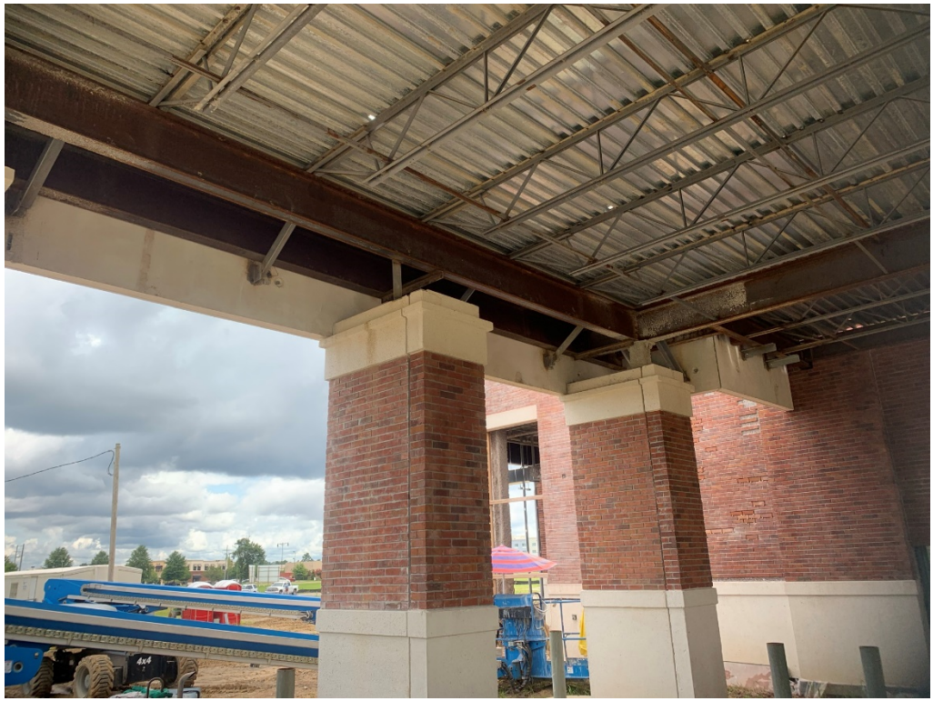
Figure 7 – Bracing at Drive Thru Canopy
