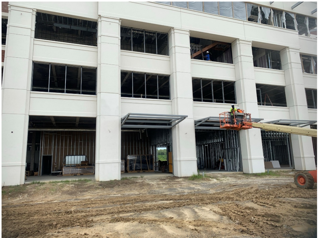
Figure 2 – West Curtainwall Installation is Ongoing
