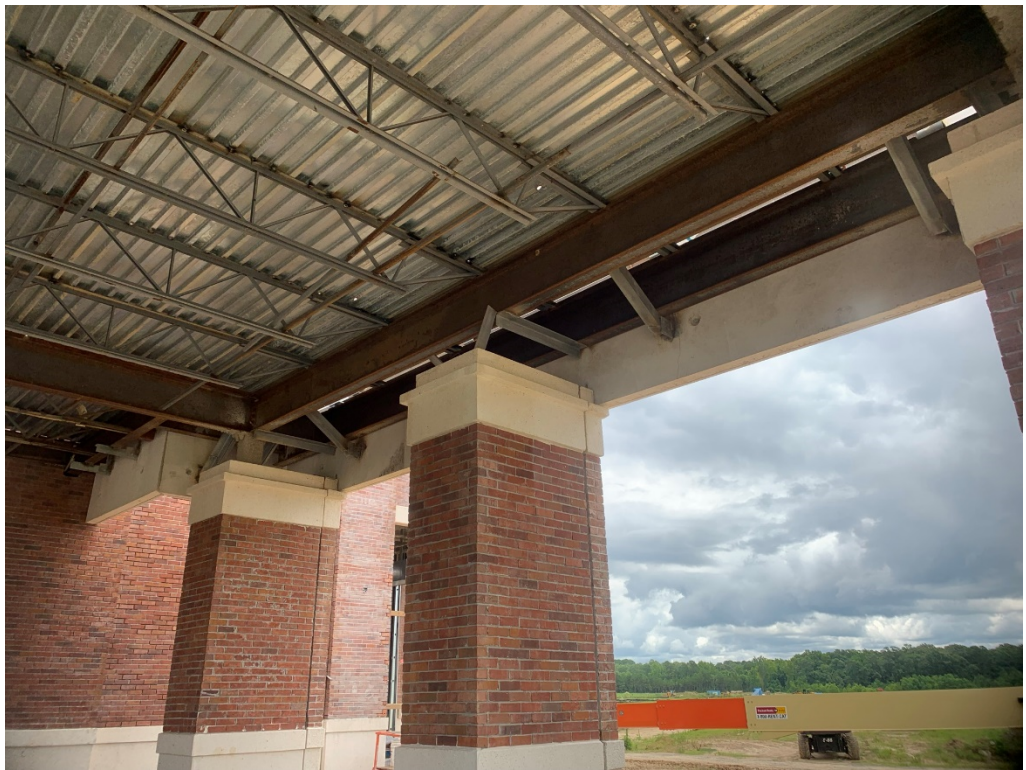
Figure 8 – Bracing at Drive Thru Canopy
