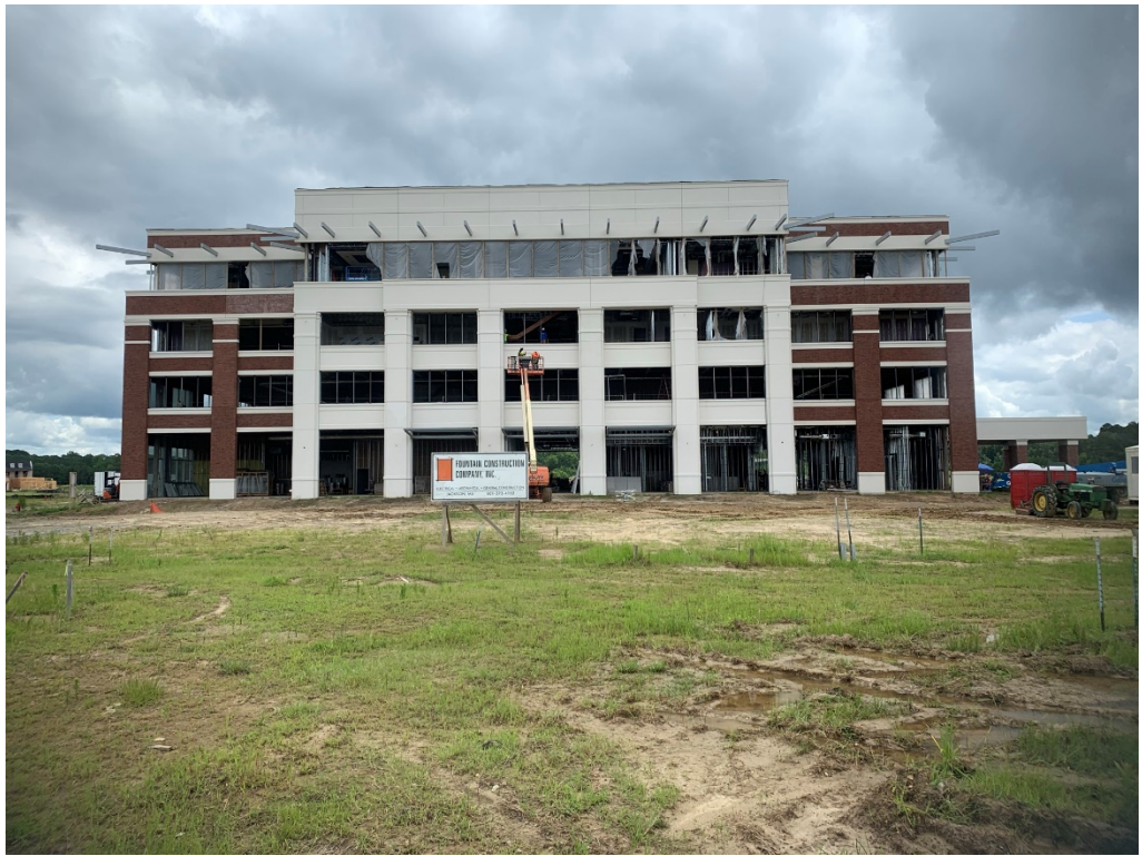
Figure 1 – Front Façade Progress
