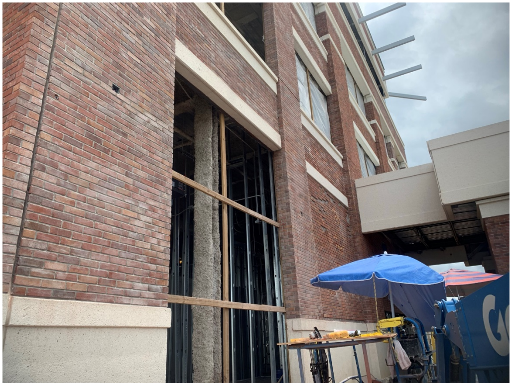
Figure 4 – South Façade Masonry is Ongoing
