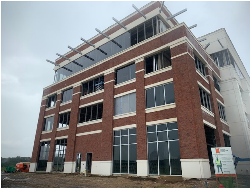
Figure 2 – Glazing Progress at North Facade
