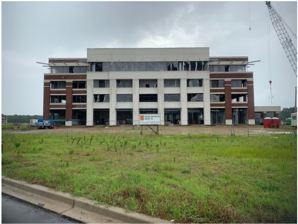
Figure 1 – Front Façade Progress
