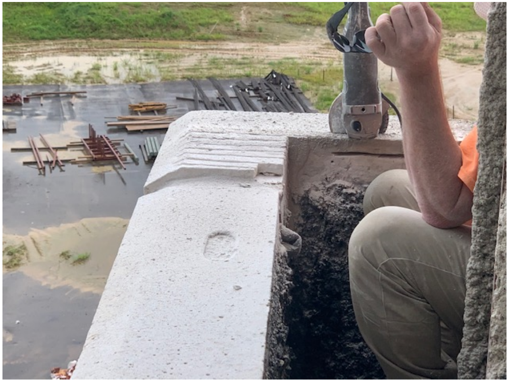
Figure 19 – Stone Worker Repairing Panel In place
