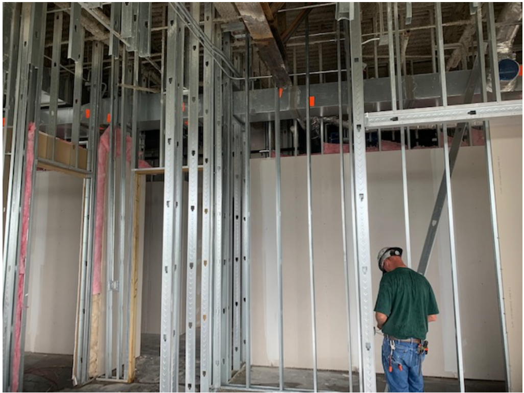
Figure 13 – Framing at Banquet Room
