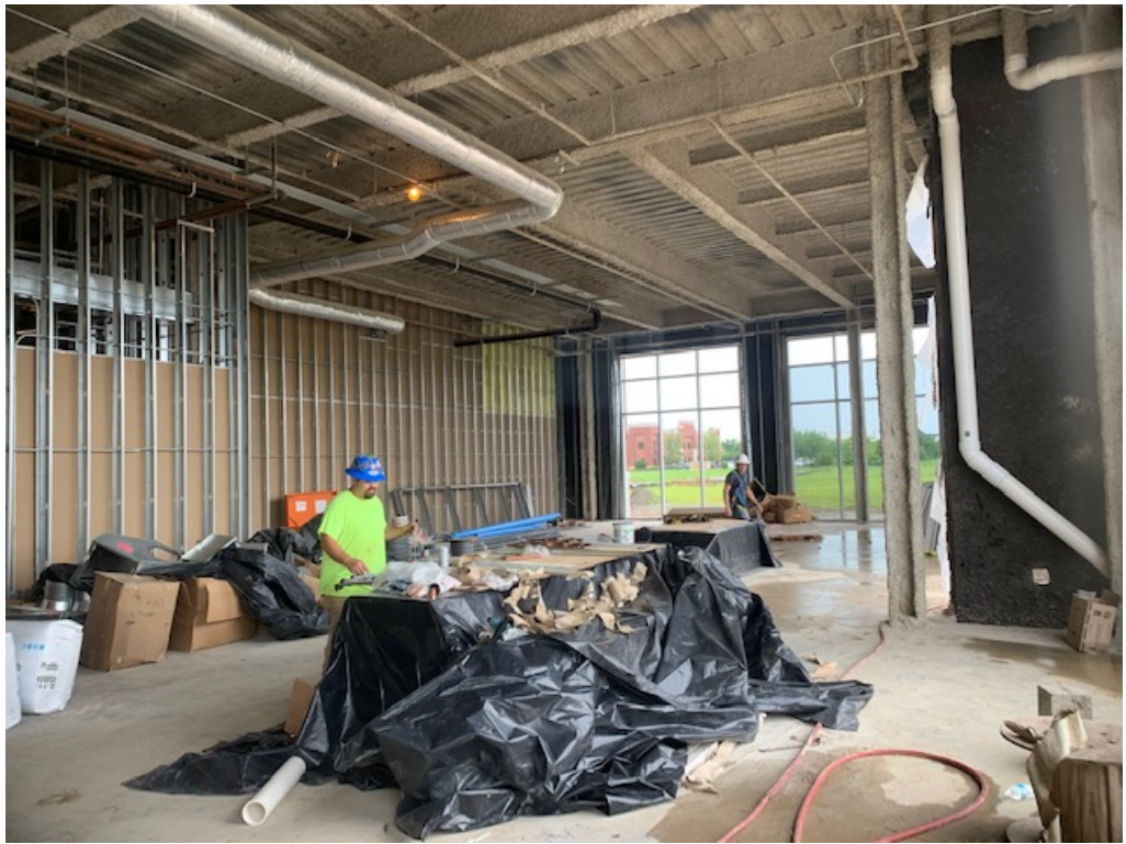
Figure 5 – 1 st Floor Staging Area
