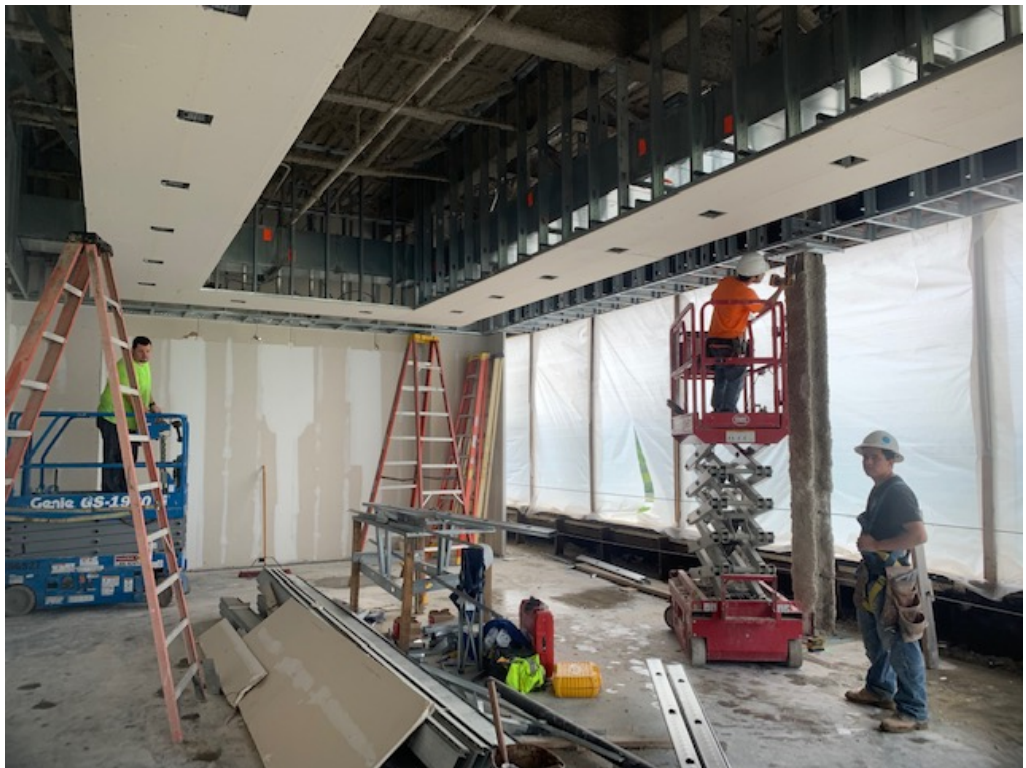
Figure 16 – Framing & Electrical at the Board Room
