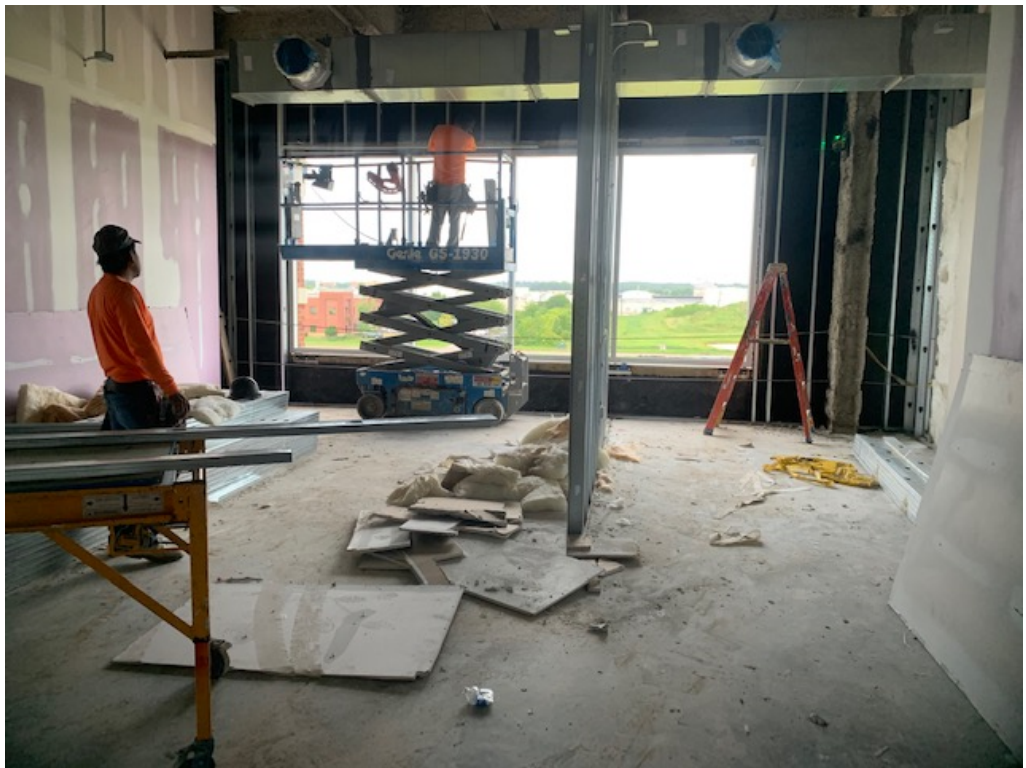
Figure 12 – Framing at 3 rd Floor North Section
