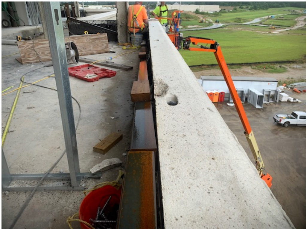
Figure 20 – Stone Worker Repairing Panel In place
