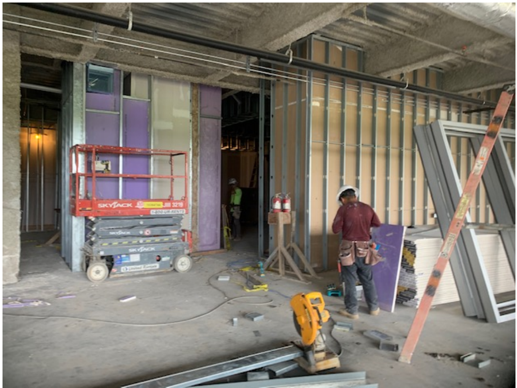
Figure 8 – Electrical Work at 2 nd Floor Elevators
