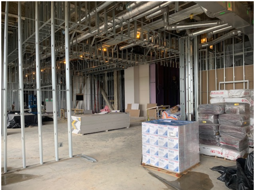
Figure 4 – 1 st Floor Staging Area
