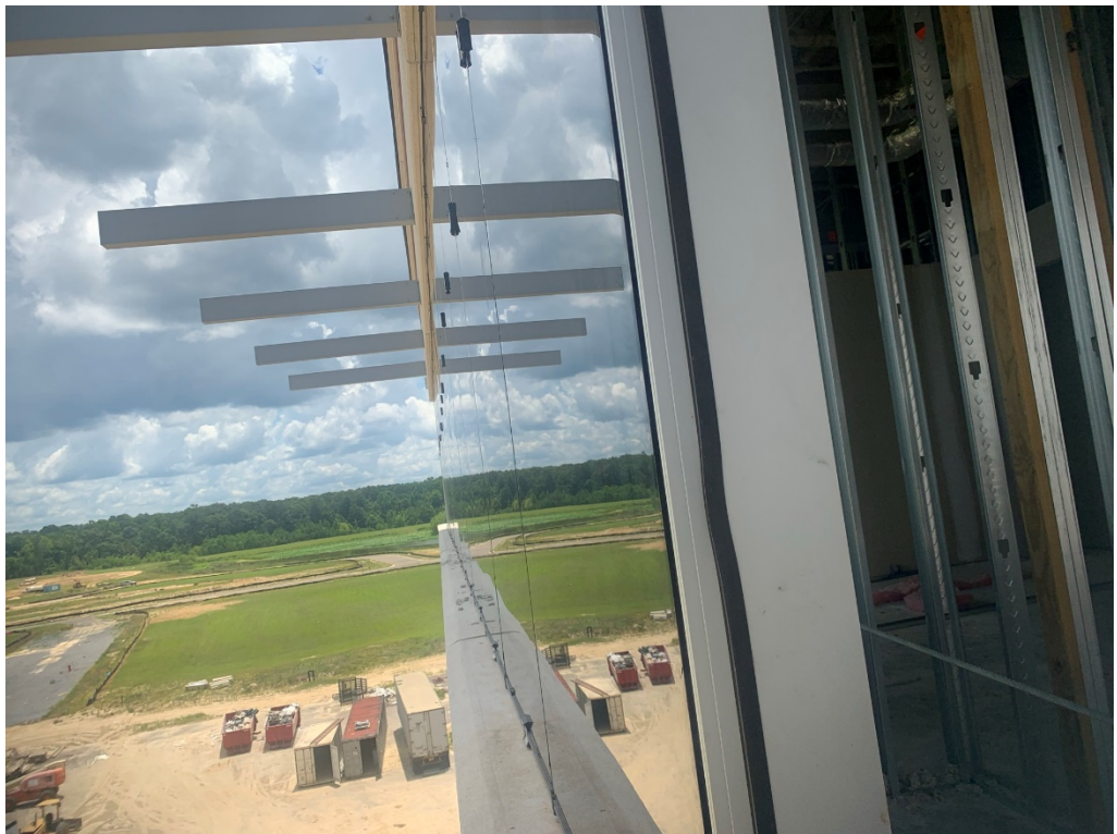
Figure 16 – Additional Glass Installed Since Monday
