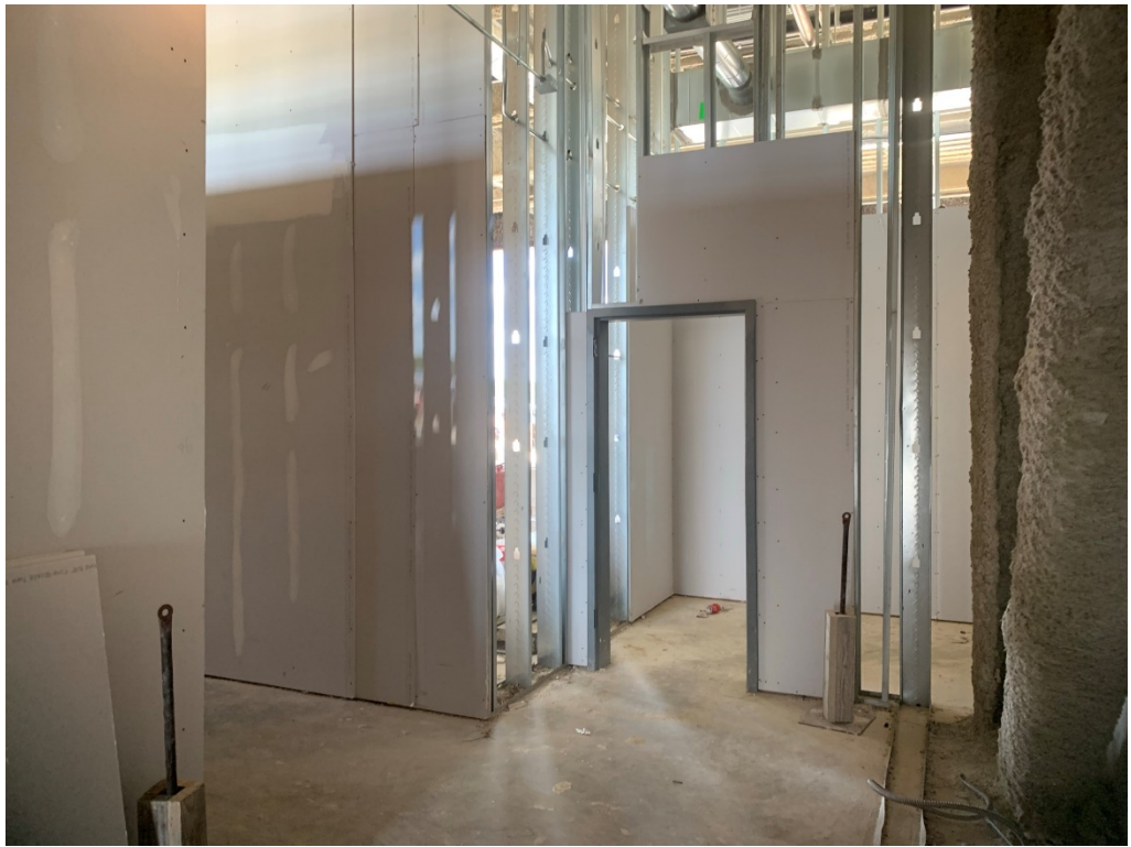
Figure 7 – Drywall Installation is Ongoing at the 4 th Floor
