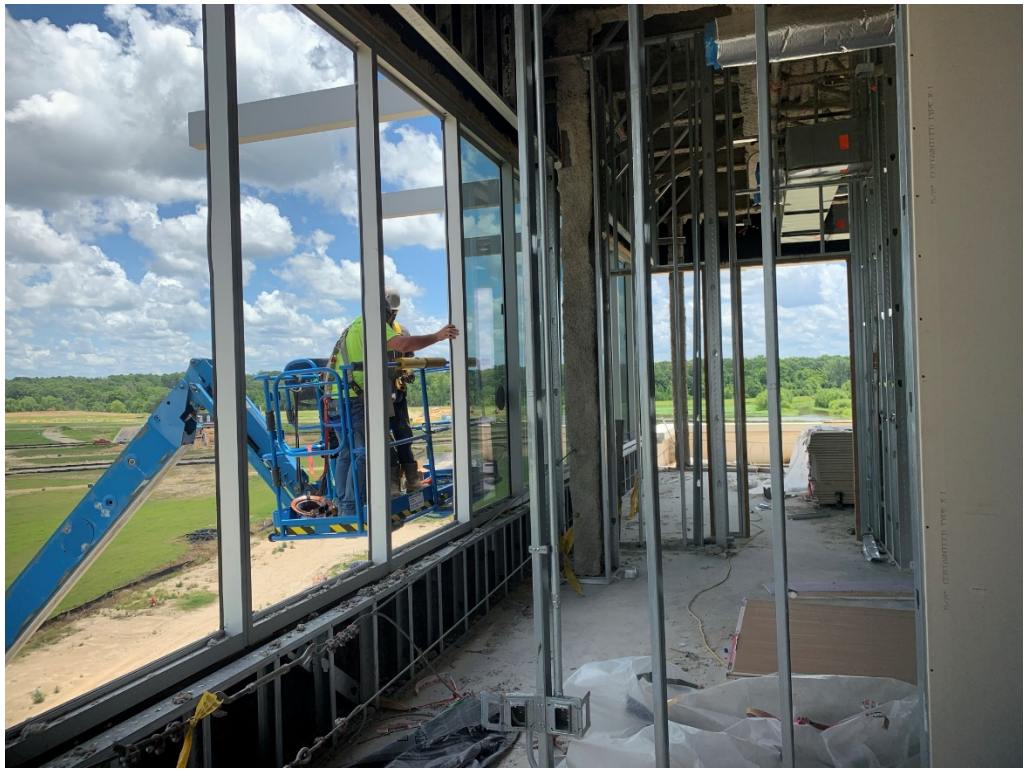
Figure 11 – Glazing Installation at 4 th Floor
