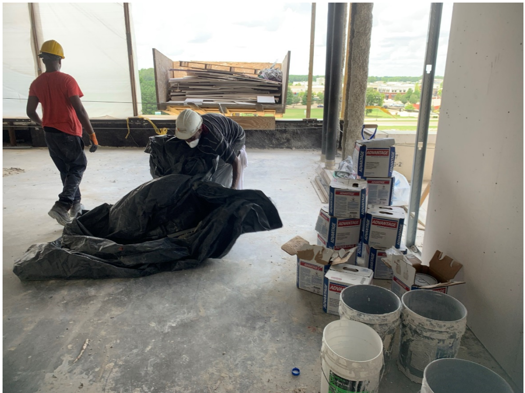
Figure 10 – Continued Debris Removal at 4 th Floor
