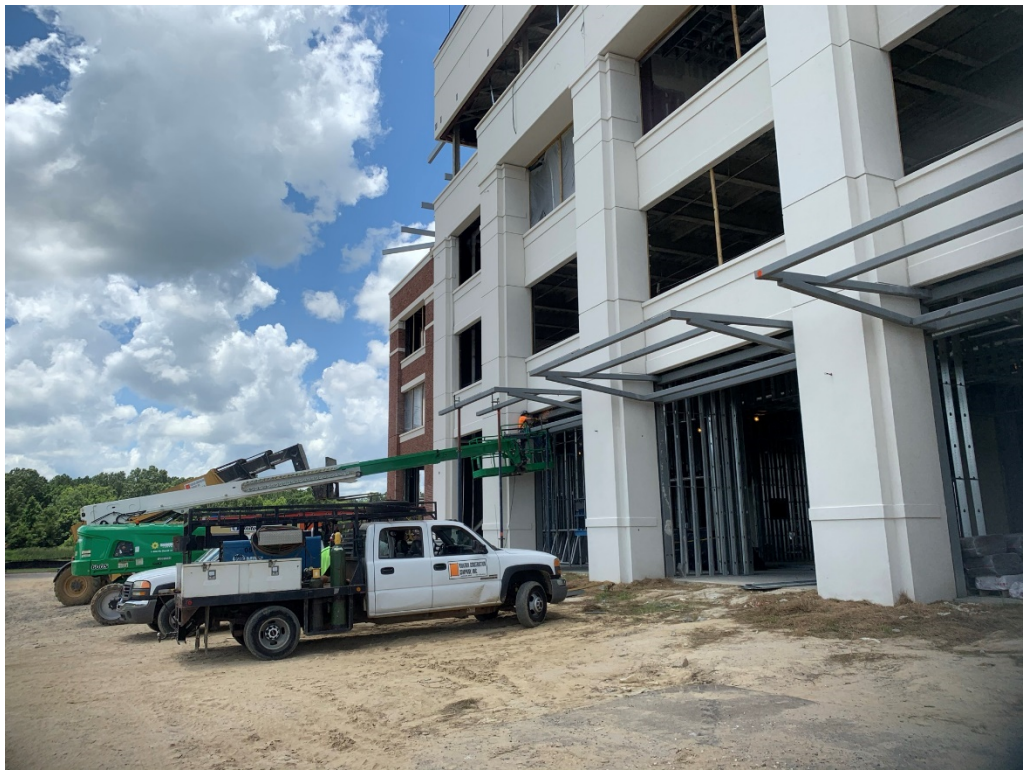
Figure 4 – Canopy Steel Rework
