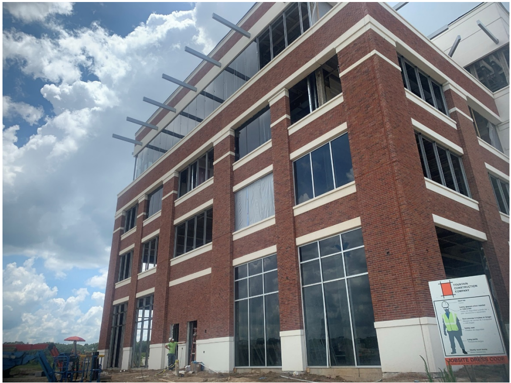
Figure 13 – Glazing Progress at North Facade
