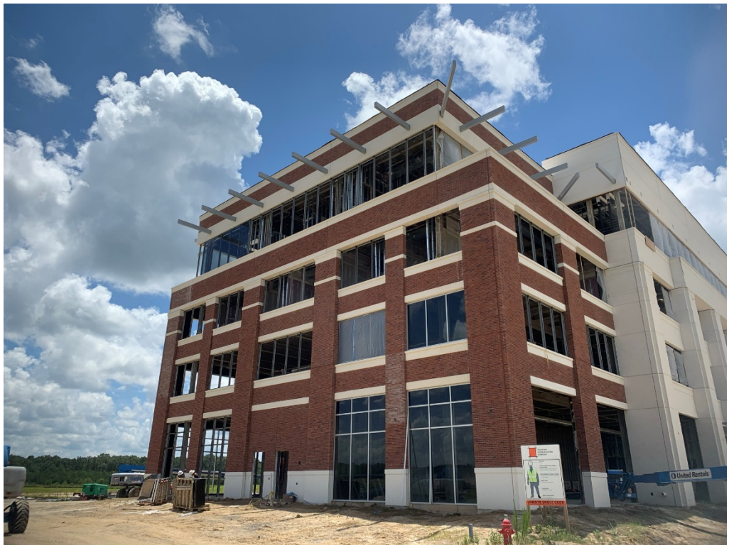
Figure 2 – North Façade Progress
