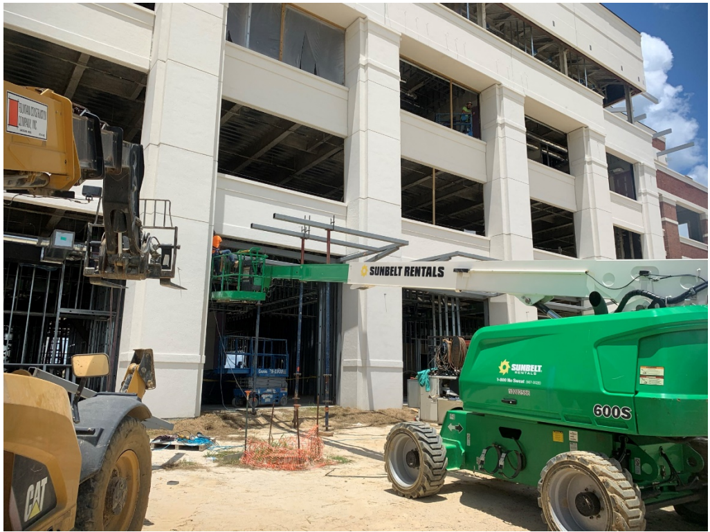
Figure 5 – Canopy Steel Rework
