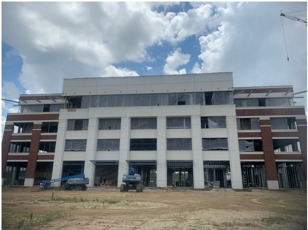
Figure 12 – Progress at Front Façade on the 1 st
