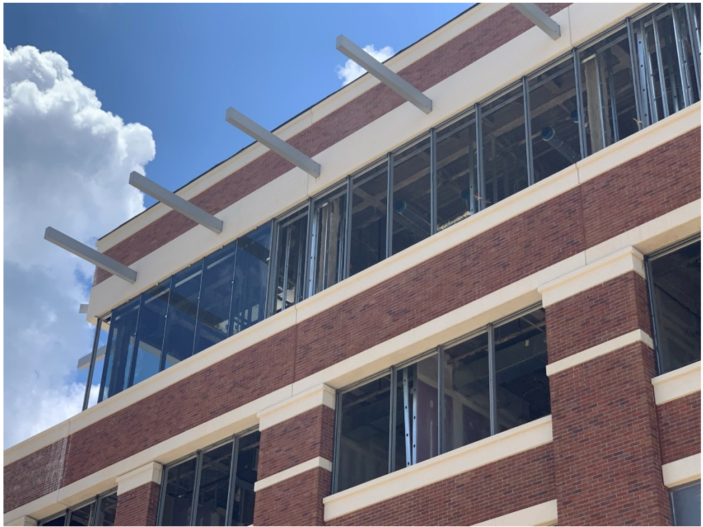
Figure 3 – Glazing Installation at 4 th Floor
