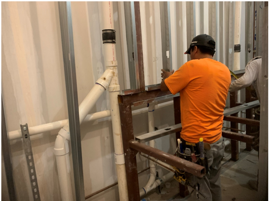
Figure 8 – Framing Work Behind Carriers at 4005
