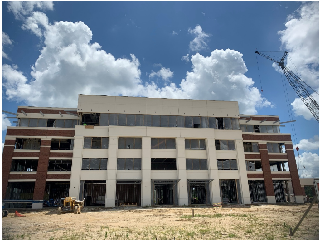
Figure 1 – Front Façade Progress on the 28 th
