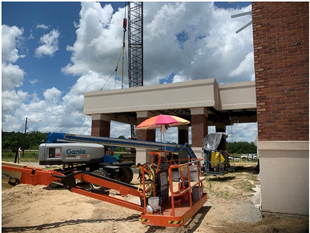
Figure 6 – Drive Thru Progress
