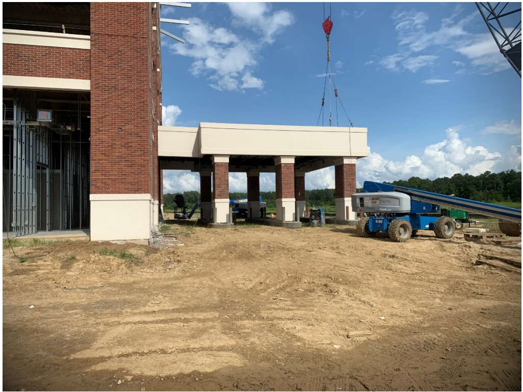
Figure 1 – Drive Thru Progress
