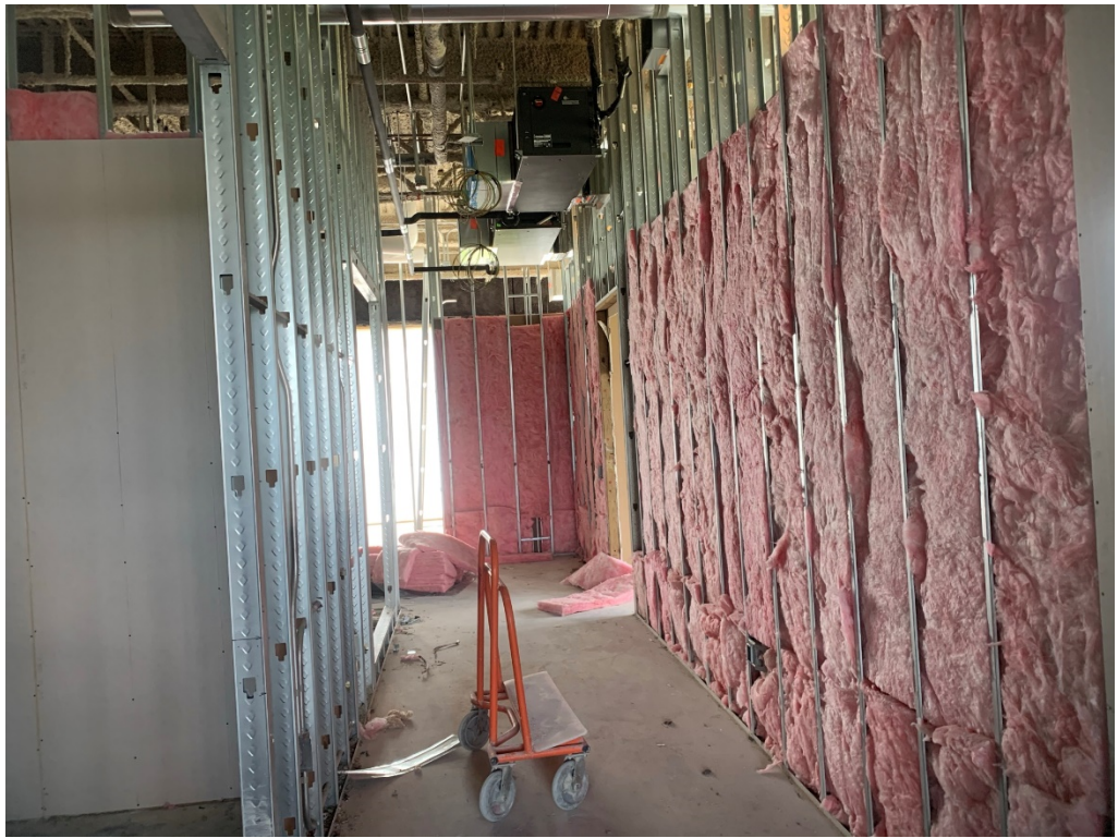
Figure 9 – Framing, Insulation, & Drywall Ongoing at the 4 th Floor
