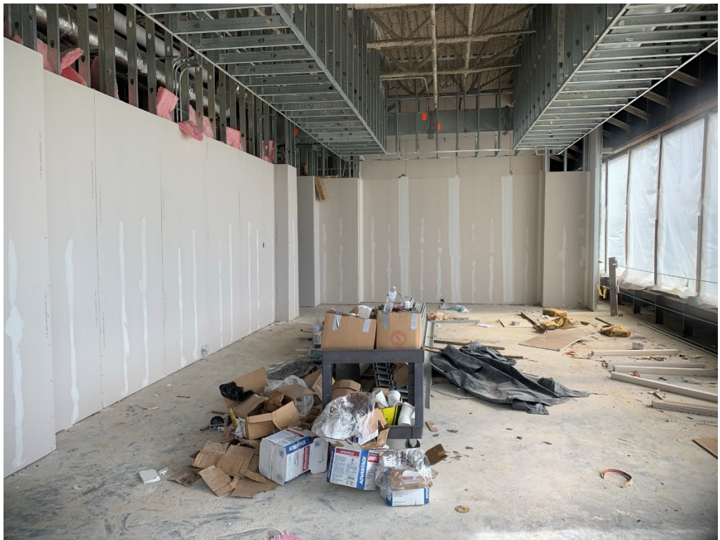
Figure 10 – Drywall Progress at 4 th Floor
