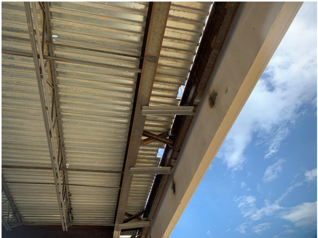
Figure 2 – Bracing at Drive Thru Panel
