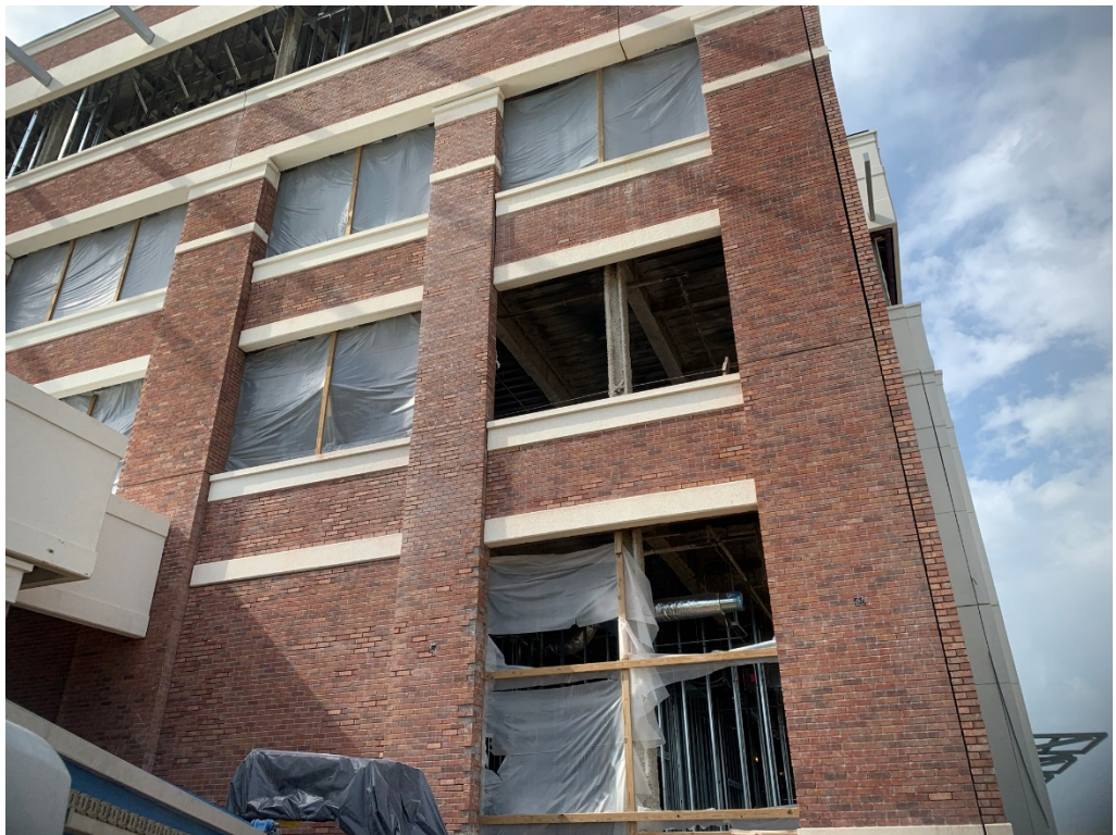
Figure 4 – Masonry work at the South Elevation is Ongoing
