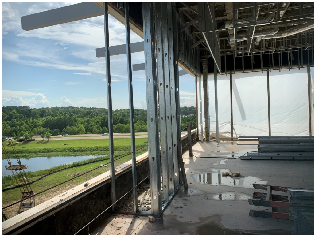
Figure 6 – Framing at the 4 th Floor
