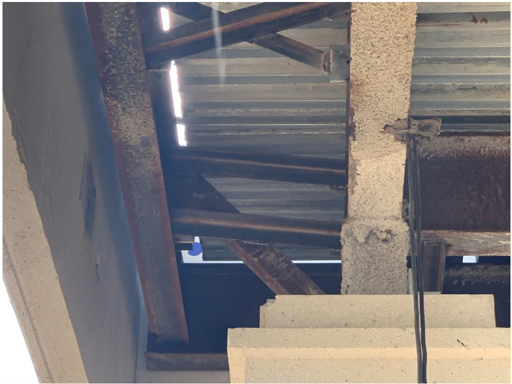
Figure 3 – Bracing at Drive Thru Panel
