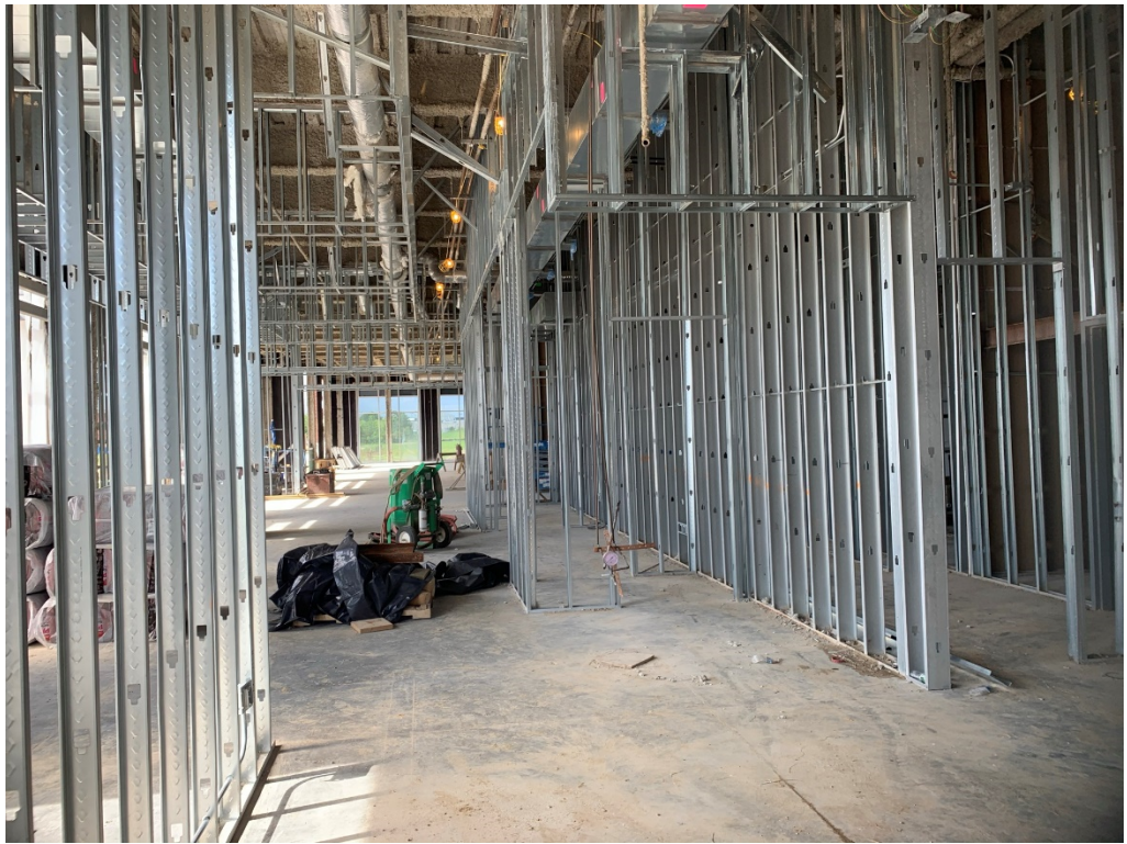
Figure 5 – Framing Progress at the First Floor
