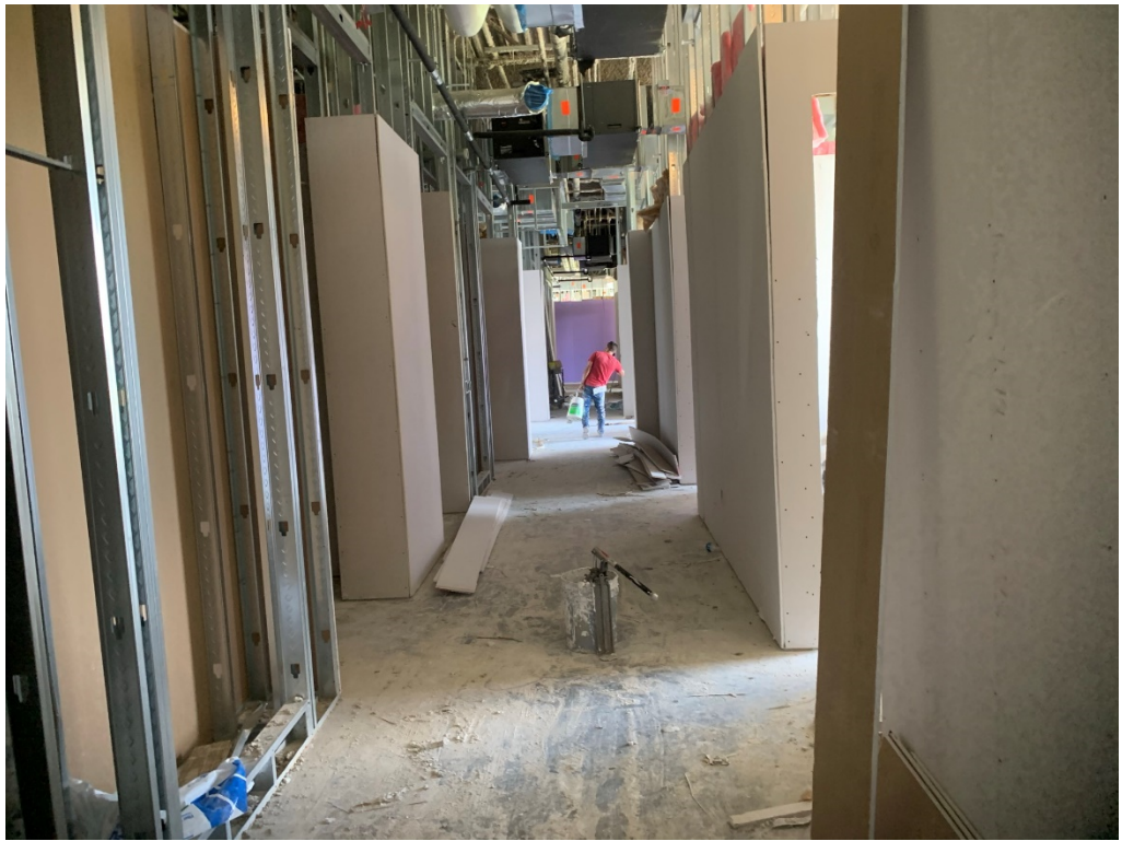
Figure 7 – Framing, Insulation, & Drywall Ongoing at the 4 th Floor
