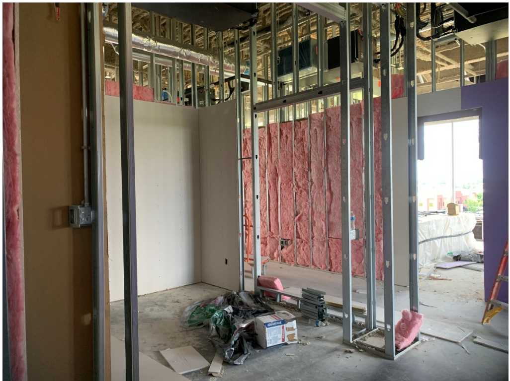
Figure 8 – Framing, Insulation, & Drywall Ongoing at the 4 th Floor
