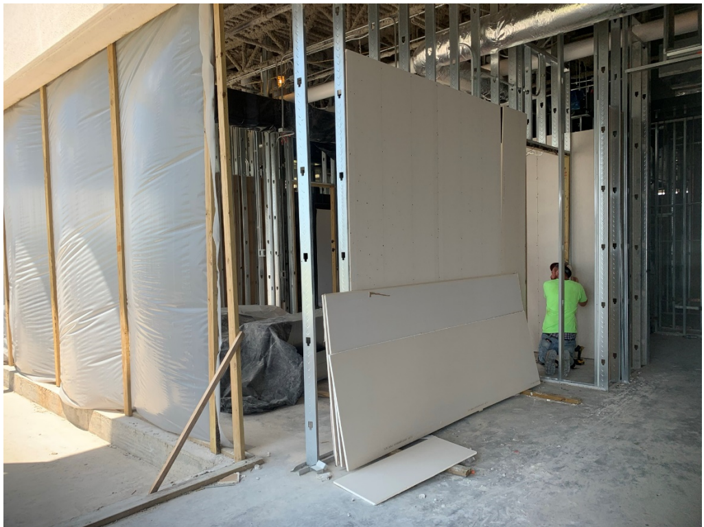
Figure 8 – Drywall Installers at 4 th Floor
