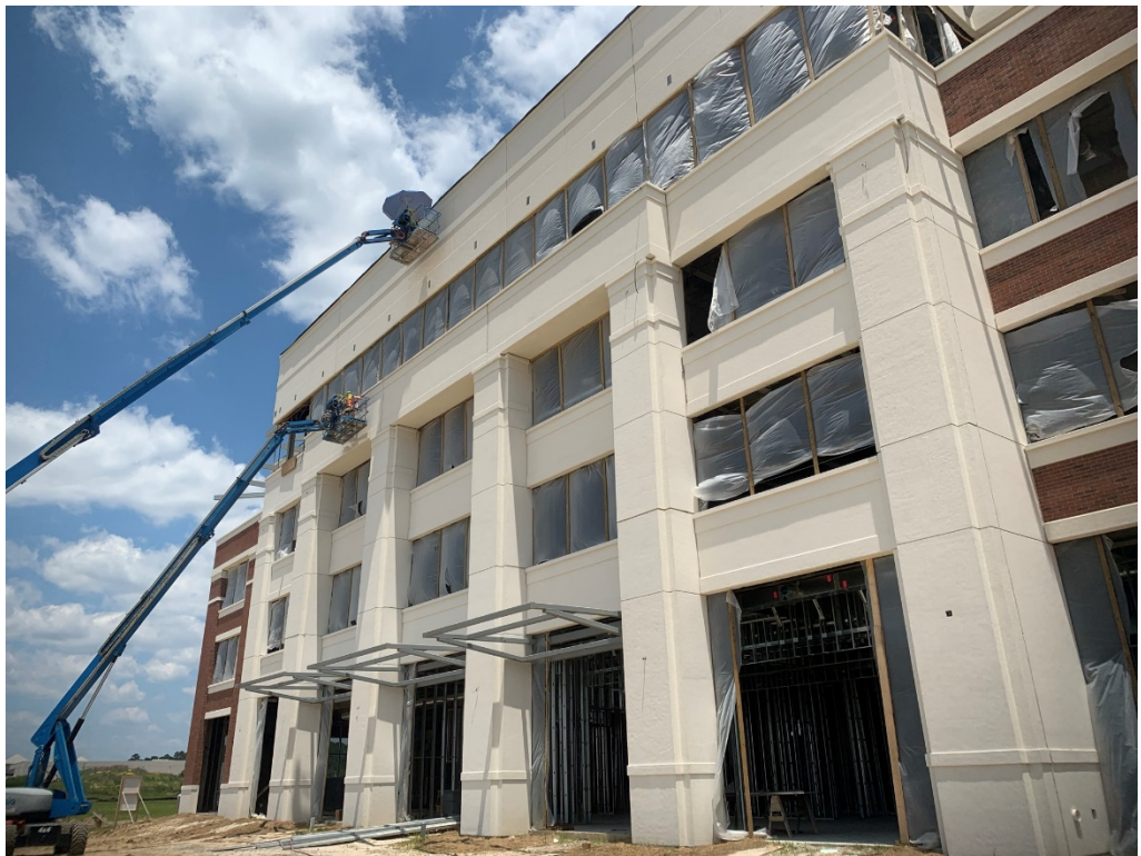
Figure 2 – Sealant Work is Ongoing
