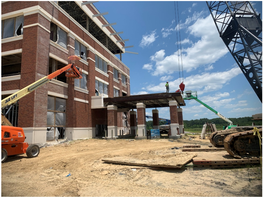
Figure 1 – Drive Thru Progress
