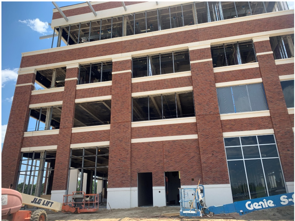
Figure 4 – North Façade Progress
