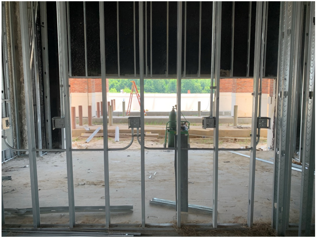
Figure 5 – Bank Window Room Progress
