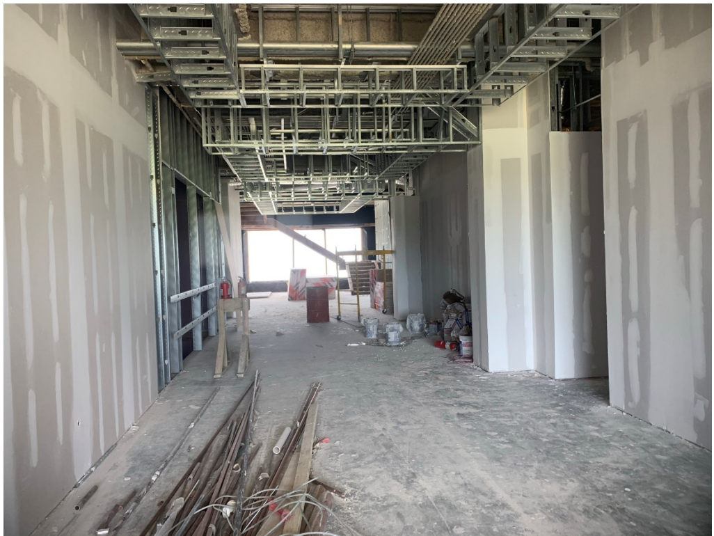
Figure 6 – Progress at 3 rd Floor
