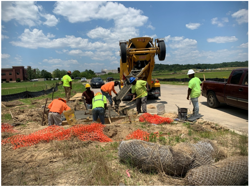
Figure 3 – Concrete Work at Site
