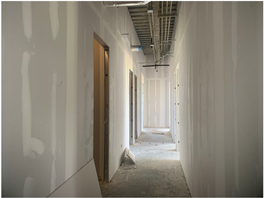
Figure 9 – 3 rd Floor Progress
