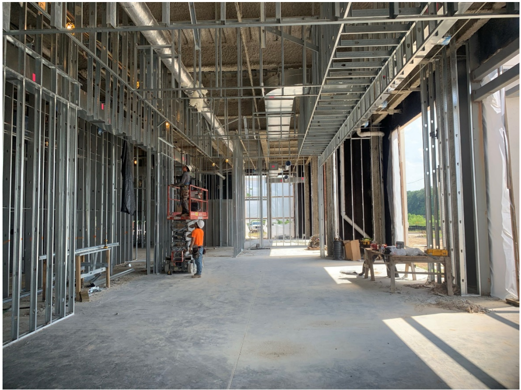
Figure 7 – 1 st Floor Progress
