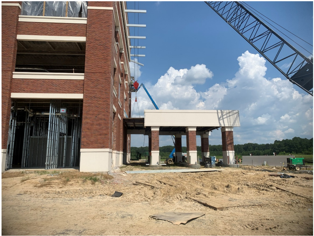
Figure 1 – Panel Install at Drive-Thru
