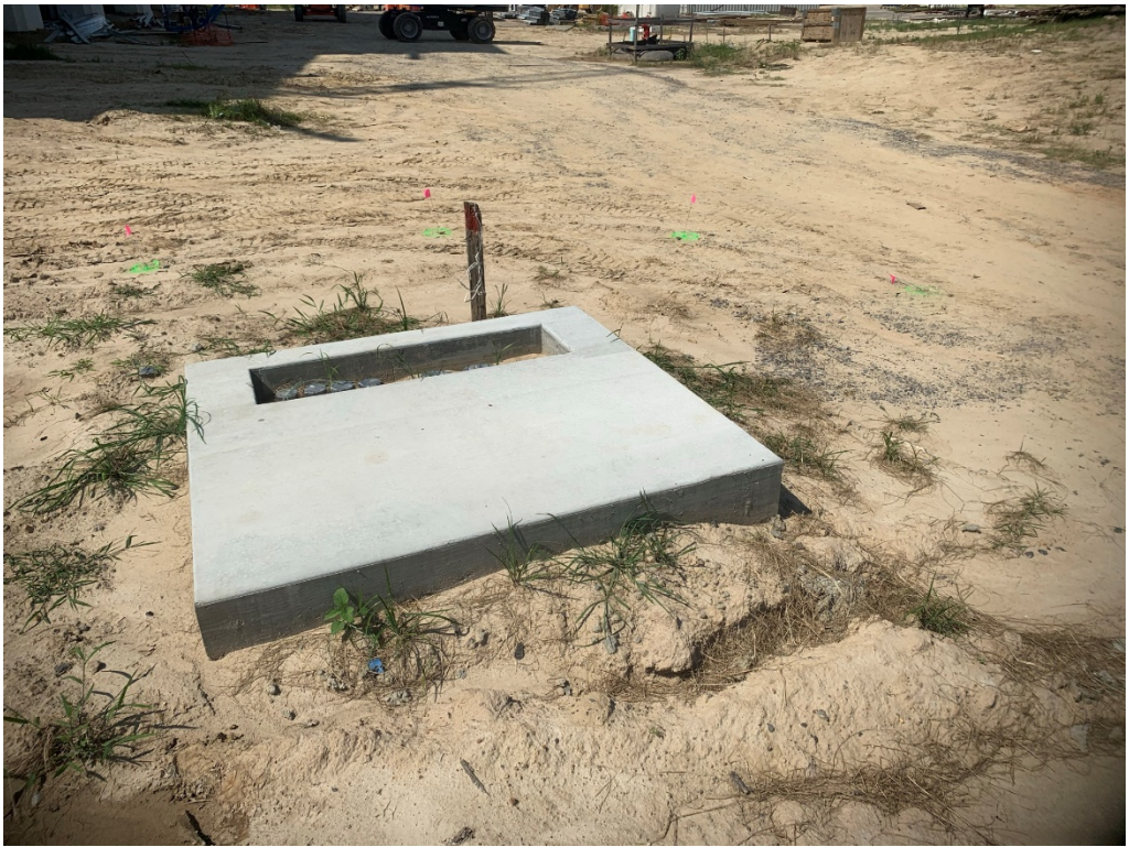
Figure 3 – Curb Marked Appears correct distance from Transformer Slab
