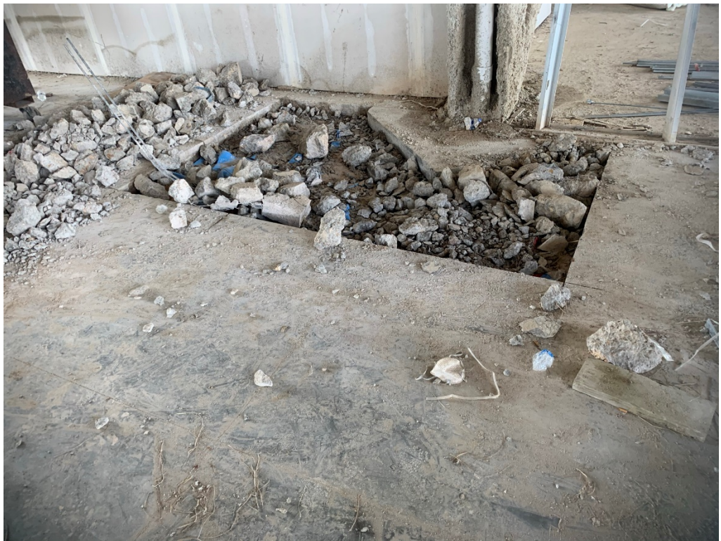
Figure 8 – Excavation at Employee Lounge
