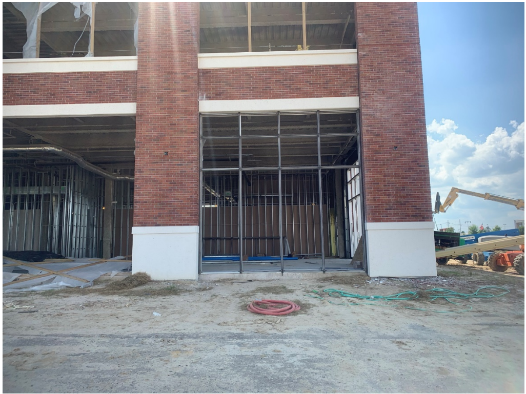
Figure 5 – Curtain Wall Install Ongoing
