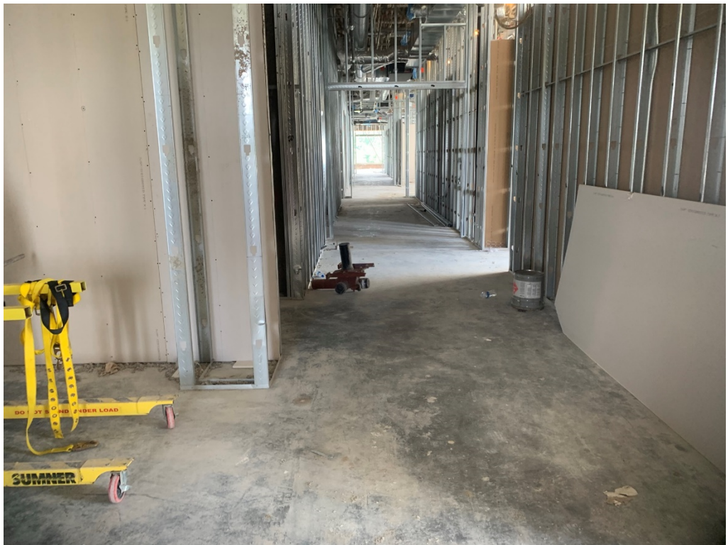
Figure 10 – 4 th Floor Progress
