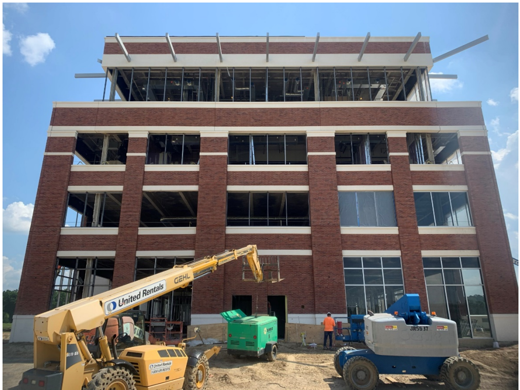
Figure 6 – North Elevation Progress
