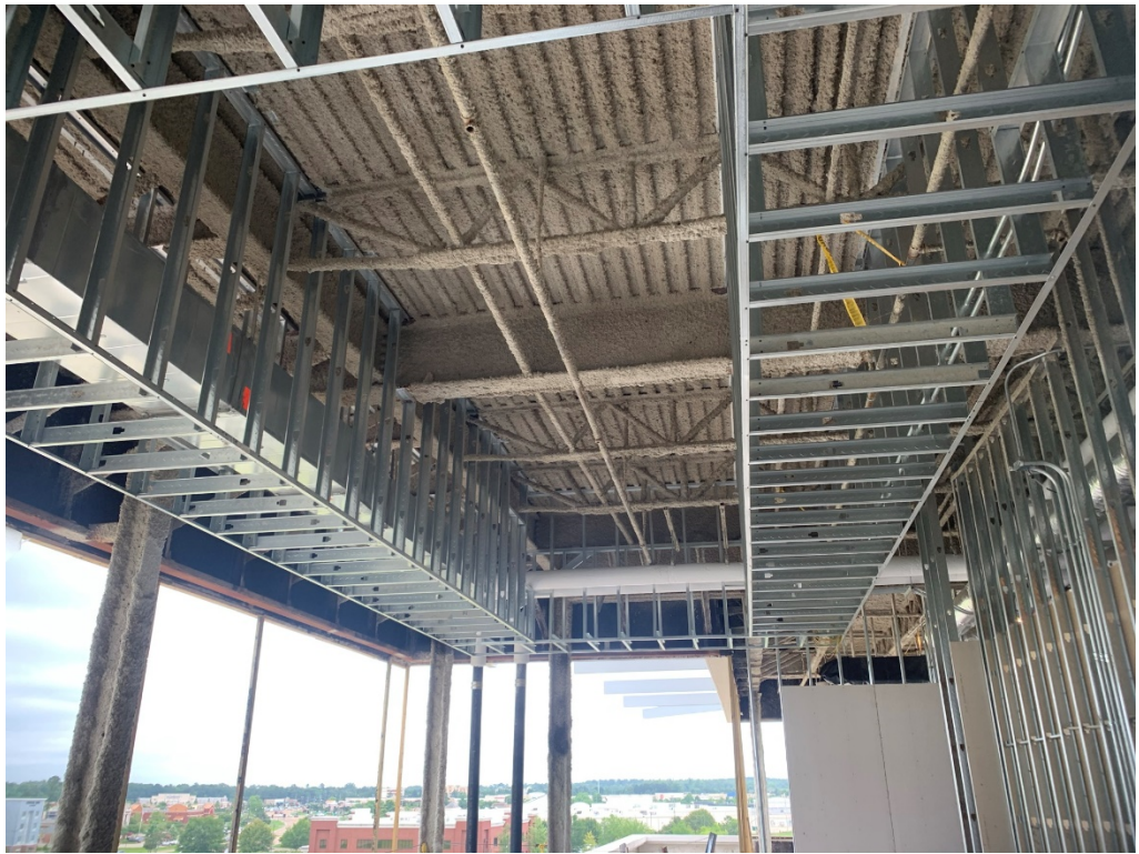
Figure 13 – Board Room Ceiling Framing
