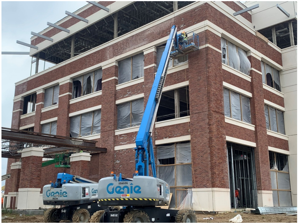
Figure 3 – South Façade Work is Ongoing
