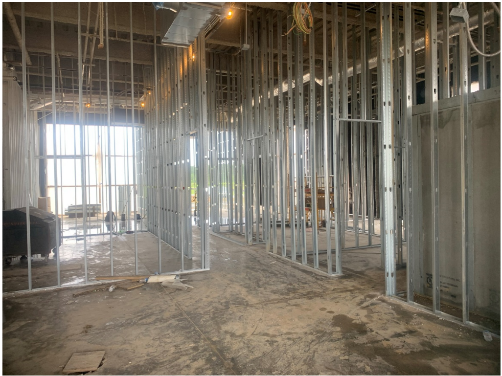
Figure 11 – 1 st Floor Bank Area Framing Progress
