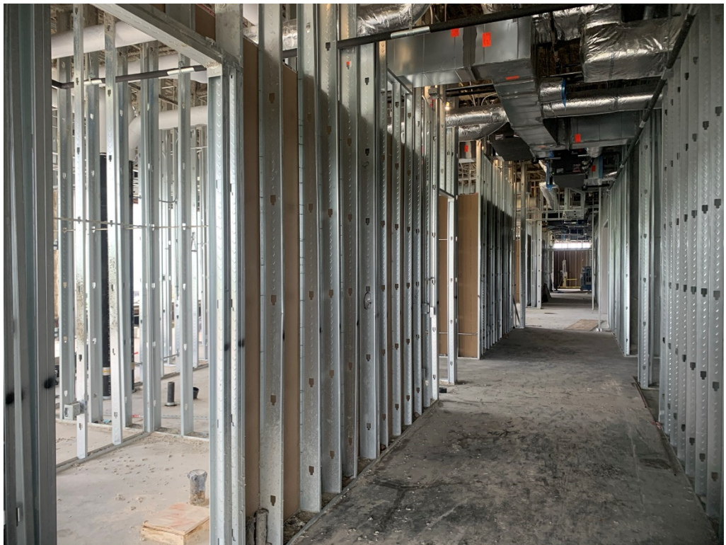
Figure 14 – Top Floor Progress
