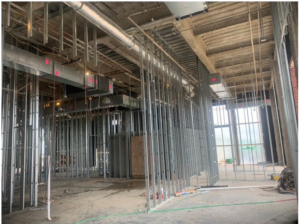
Figure 10 – 1 st Floor Bank Area Framing Progress
