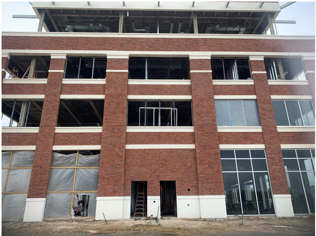
Figure 4 – North Façade Progress
