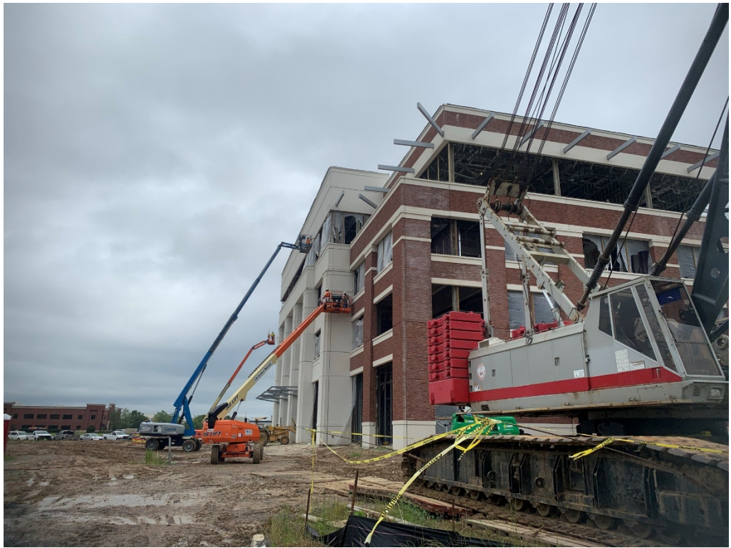
Figure 1 – Continued work on West Elevation
