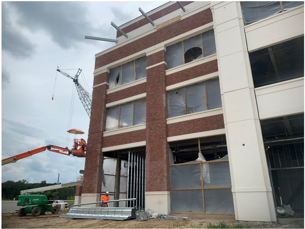
Figure 5 – Masonry is Ongoing
