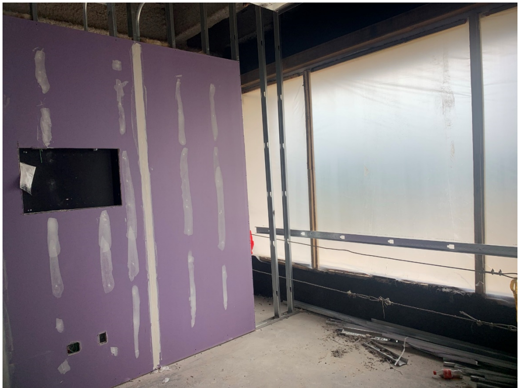
Figure 10 – Typical Recess of Finished Framing (pending storefront installation)
