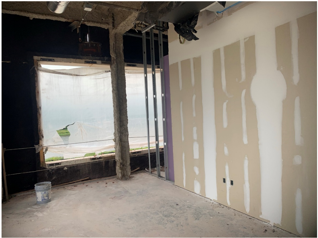
Figure 11 – Typical Recess of Finished Framing (pending storefront installation)
