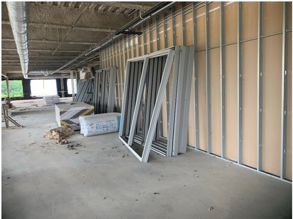
Figure 8 – Storefront Frames Stored on 2 nd Floor
