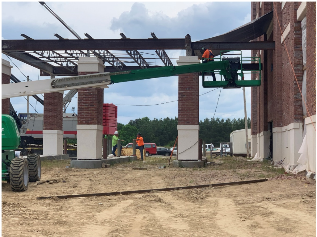
Figure 6 – Panel Install at Drive Thru
