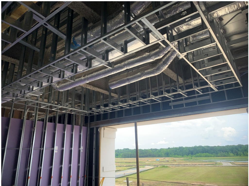
Figure 12 – 3 rd Floor Ceiling Framing @ Conference
