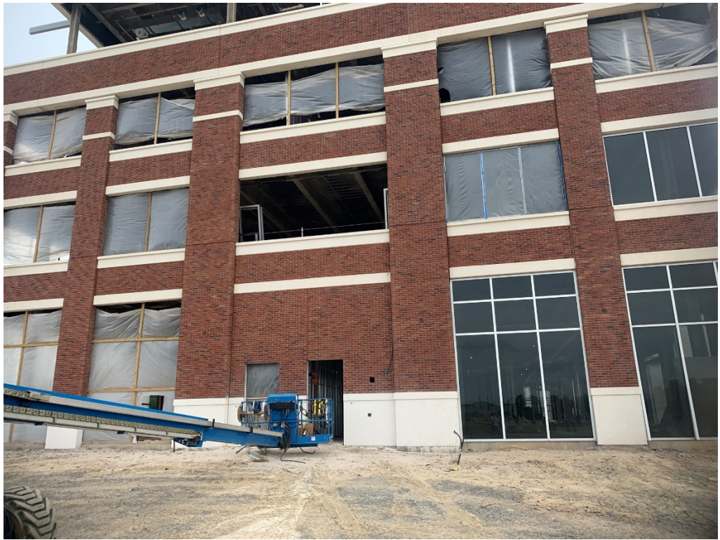
Figure 1 – Continued work on North elevation
