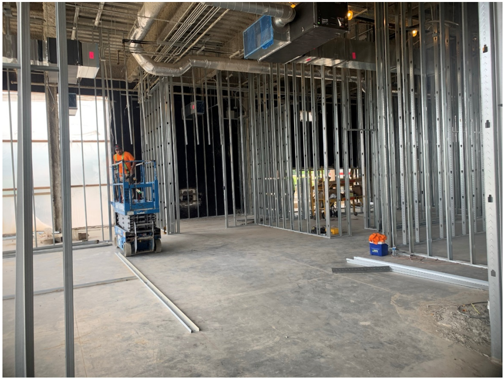
Figure 7 – Framing at 1 st Floor
