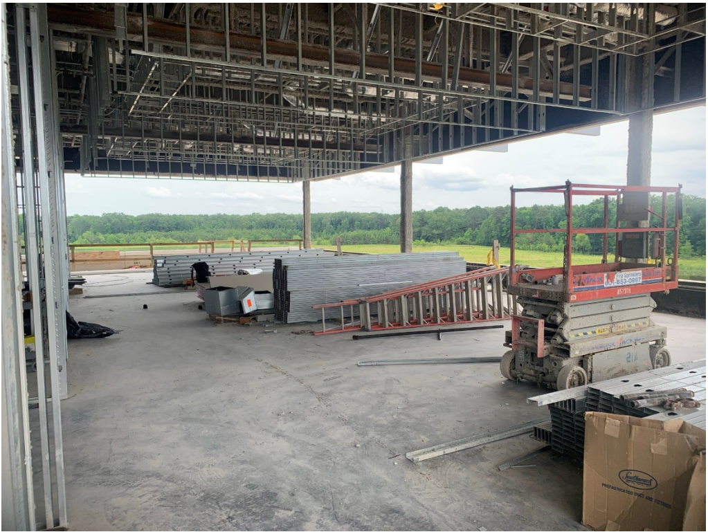
Figure 17 – 4 th Floor Banquet Progress
