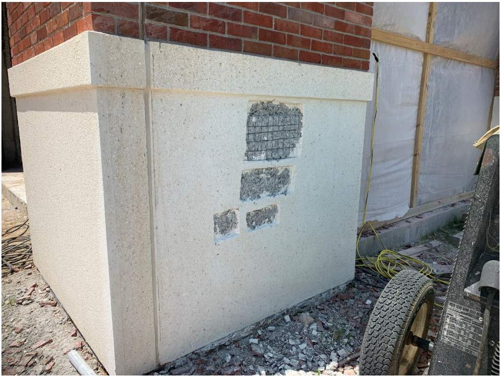
Figure 3 – Work at Precast Panel NE Corner
