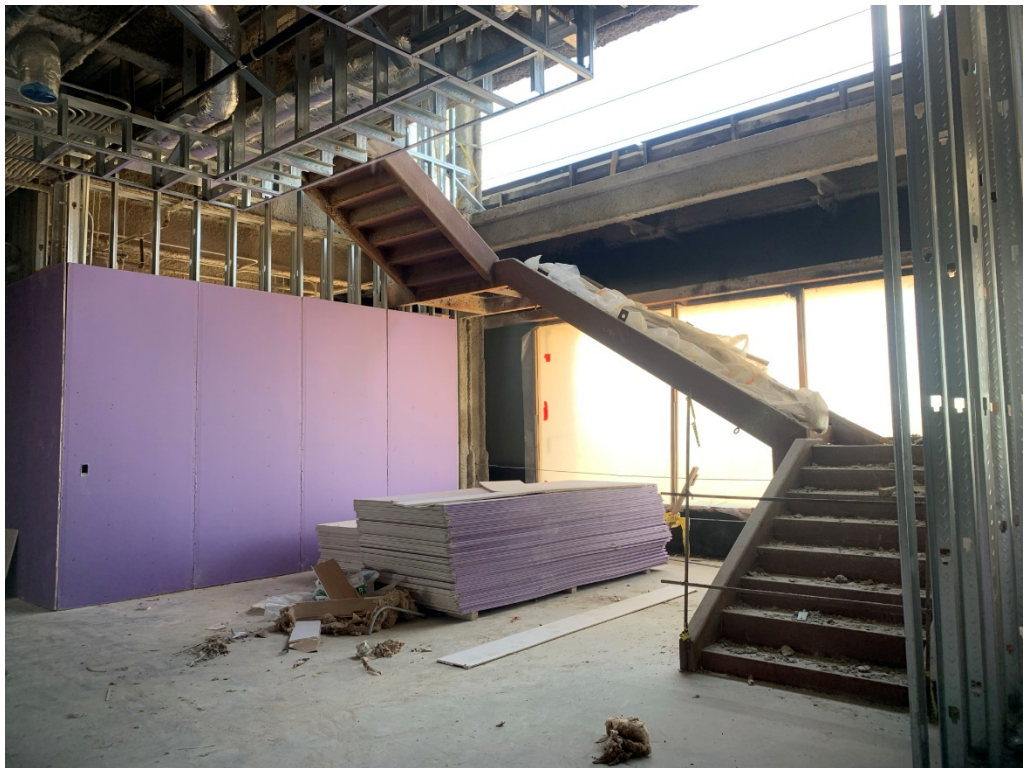
Figure 6 – Double Height Stair Space is Shaping Up
