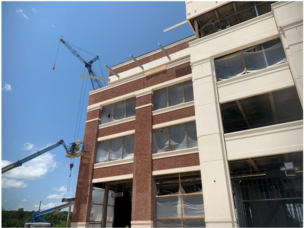
Figure 5 – SE Brick work at Corner
