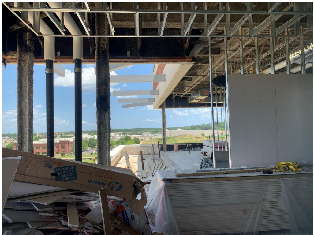
Figure 8 – Upper Floor Progress
