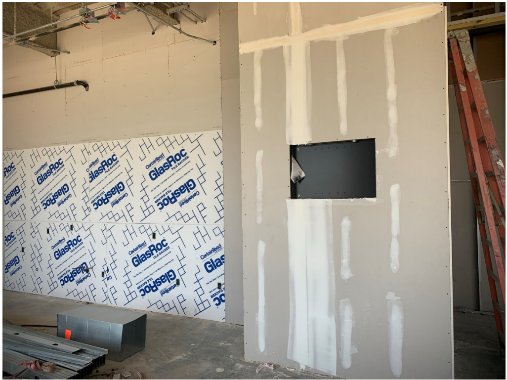
Figure 7 – 3 rd Floor Break Room; GlasRoc installed at cabinet wall
