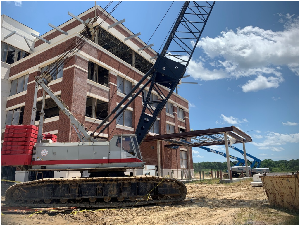
Figure 1 – Continued work on south elevation
