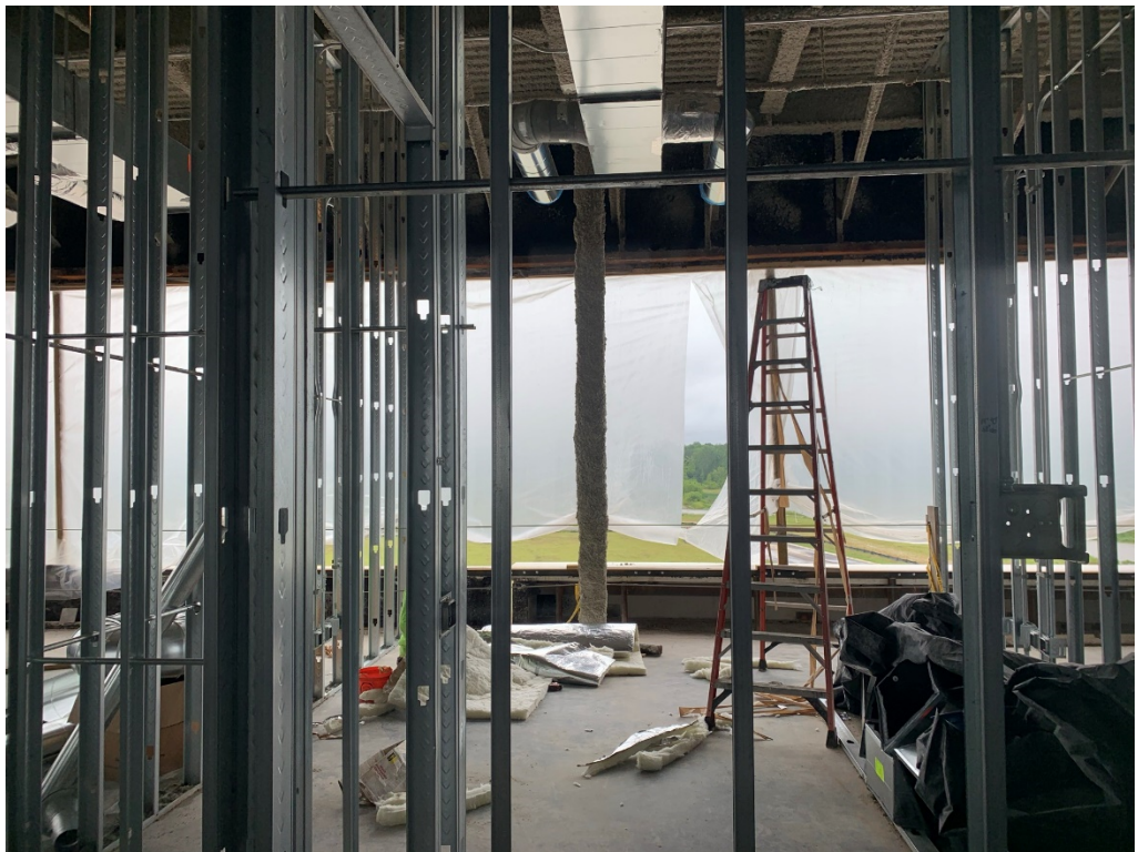
Figure 10 – Duct Insulation is Ongoing
