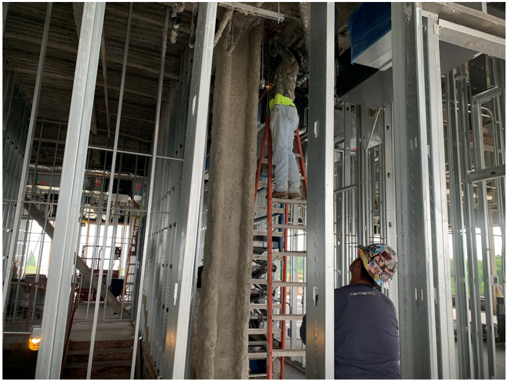
Figure 9 – Plumbers Installing Copper Pipe
