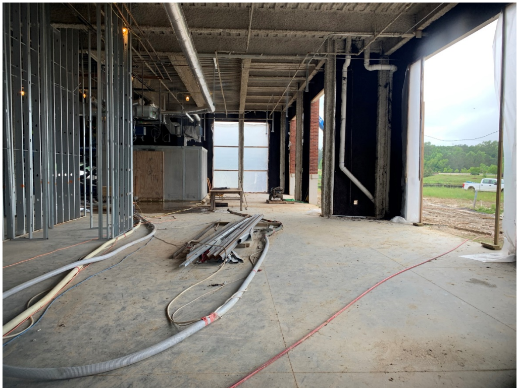
Figure 4 – 1 st Floor Space
