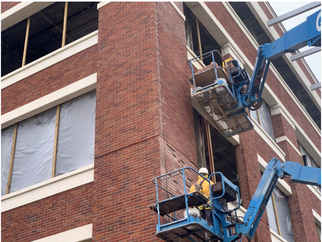
Figure 2 – Brick Repair at Cast Panels is Ongoing
