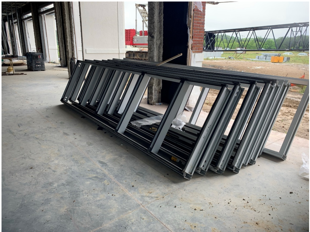
Figure 8 – Curtain Wall Stored at First Floor
