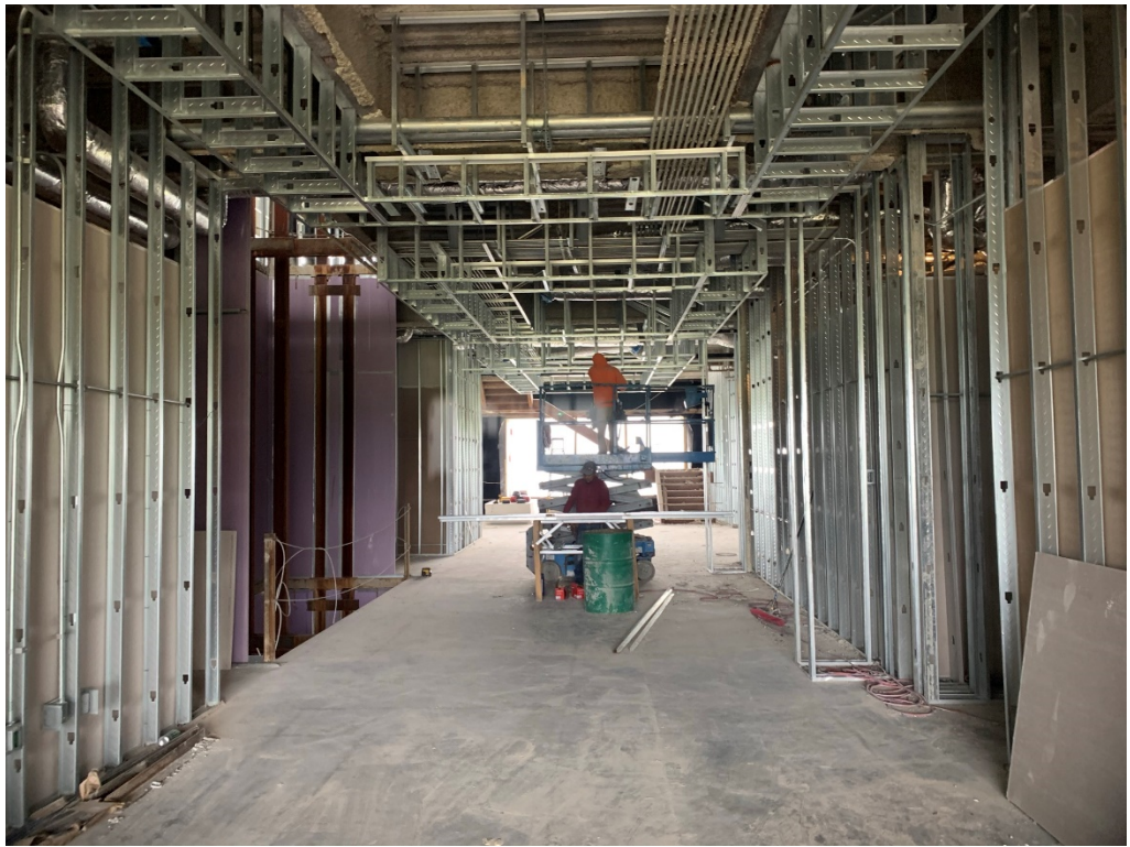
Figure 7 – 3 rd Floor Ceiling Framing is Ongoing
