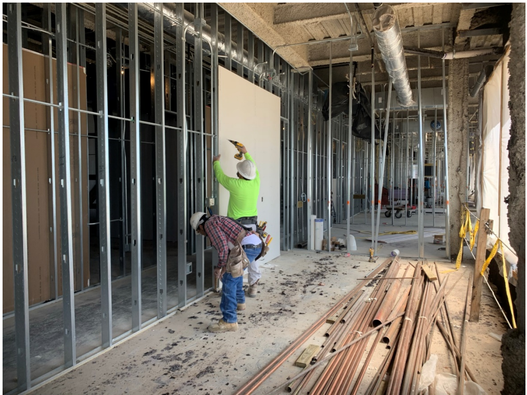
Figure 6 – Drywall at 3 rd Floor
