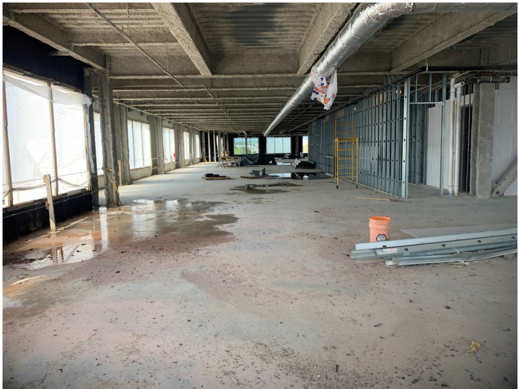
Figure 14 – 2 nd Floor Progress
