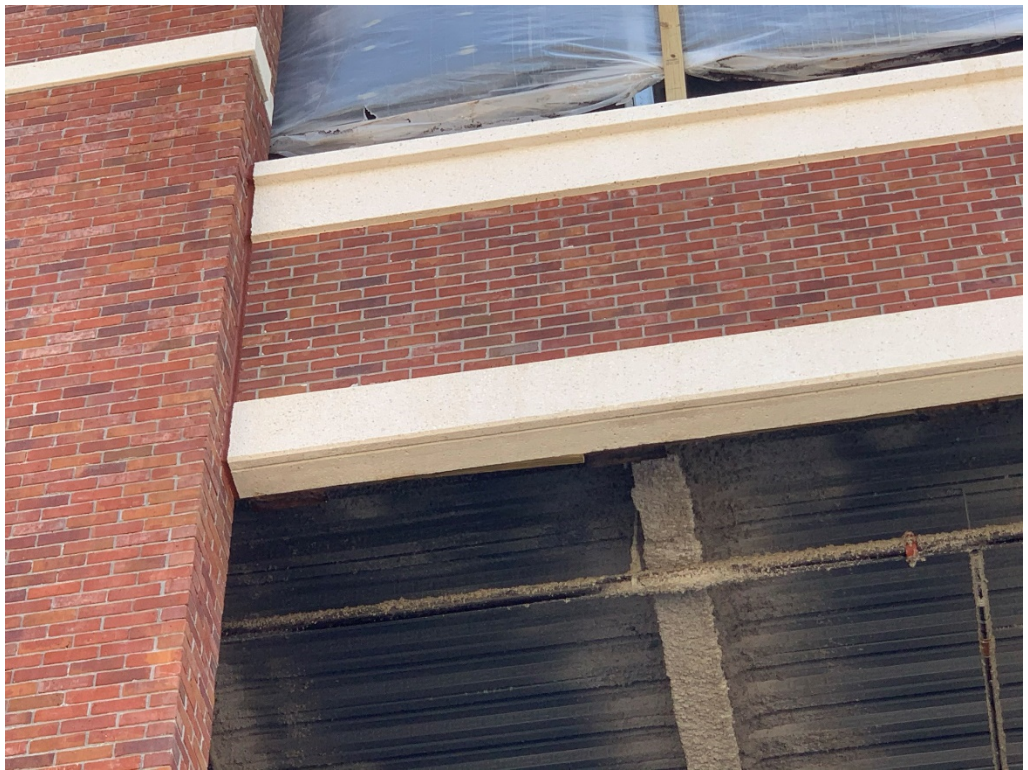
Figure 4 – Example of Red Sealant at Panels Looks Good
