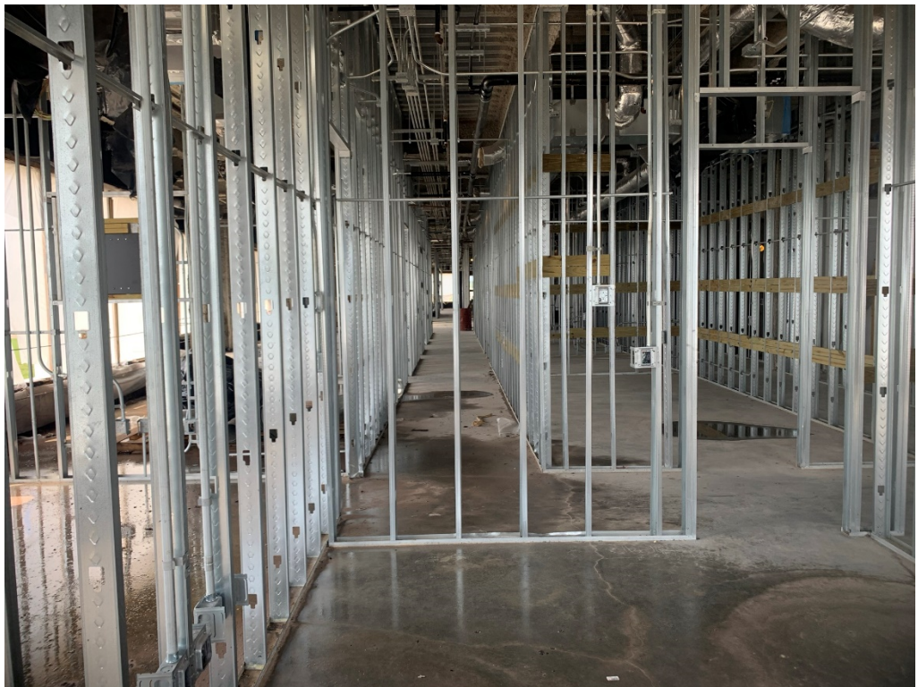
Figure 16 – 3 rd Floor Framing Progress
