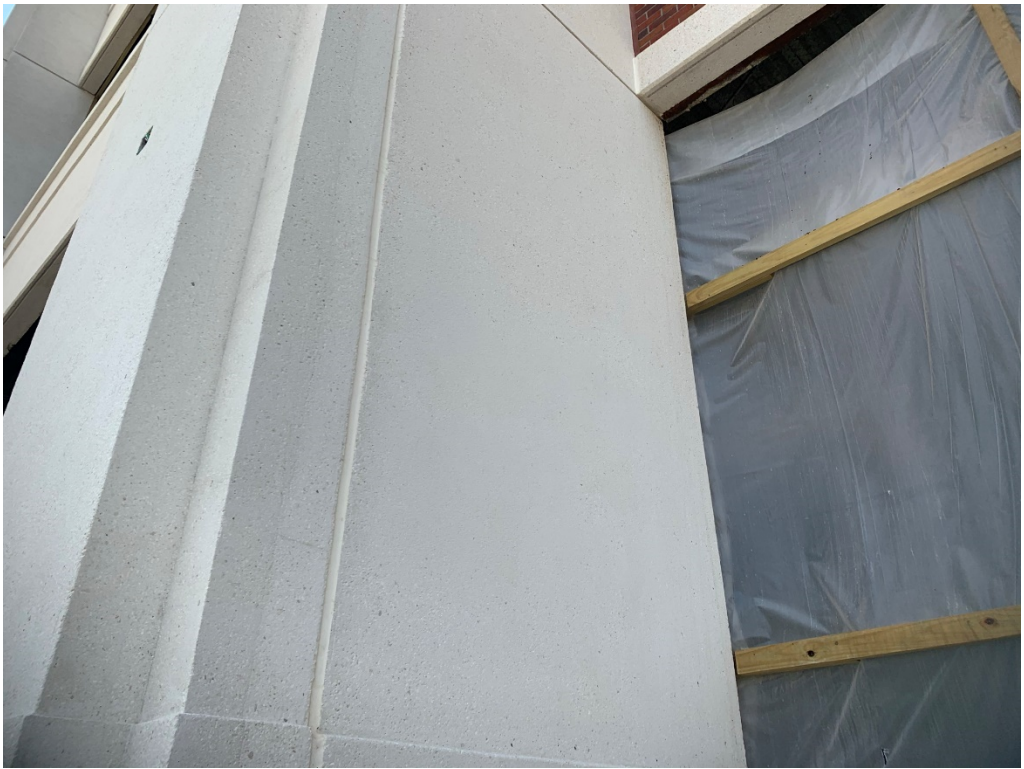
Figure 5 – Sealant Progress
