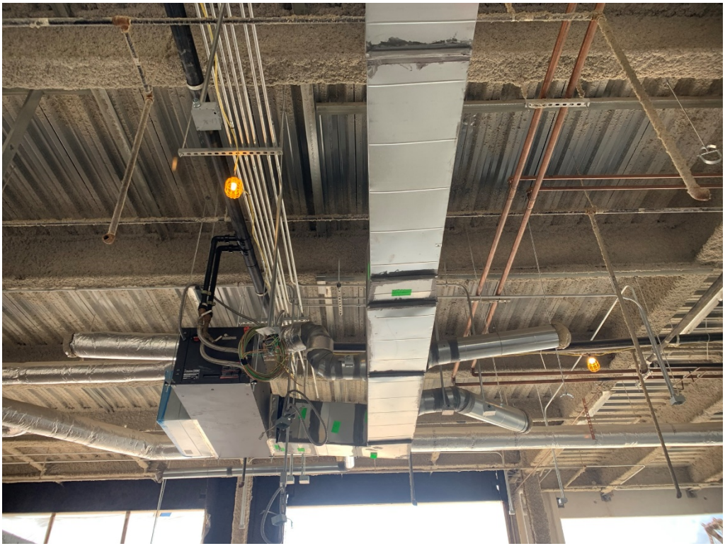
Figure 9 – Mechanical Work is Ongoing
