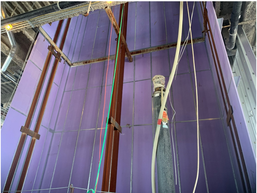
Figure 10 – Drywall at Shafts
