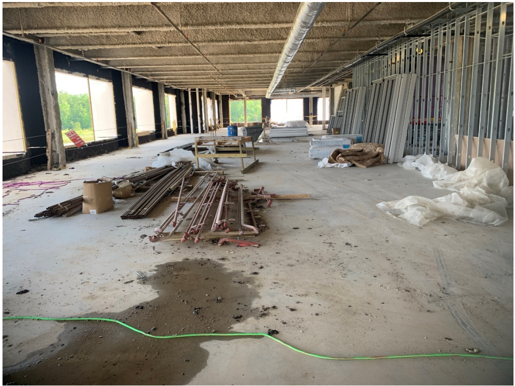
Figure 13 – 2 nd Floor Progress
