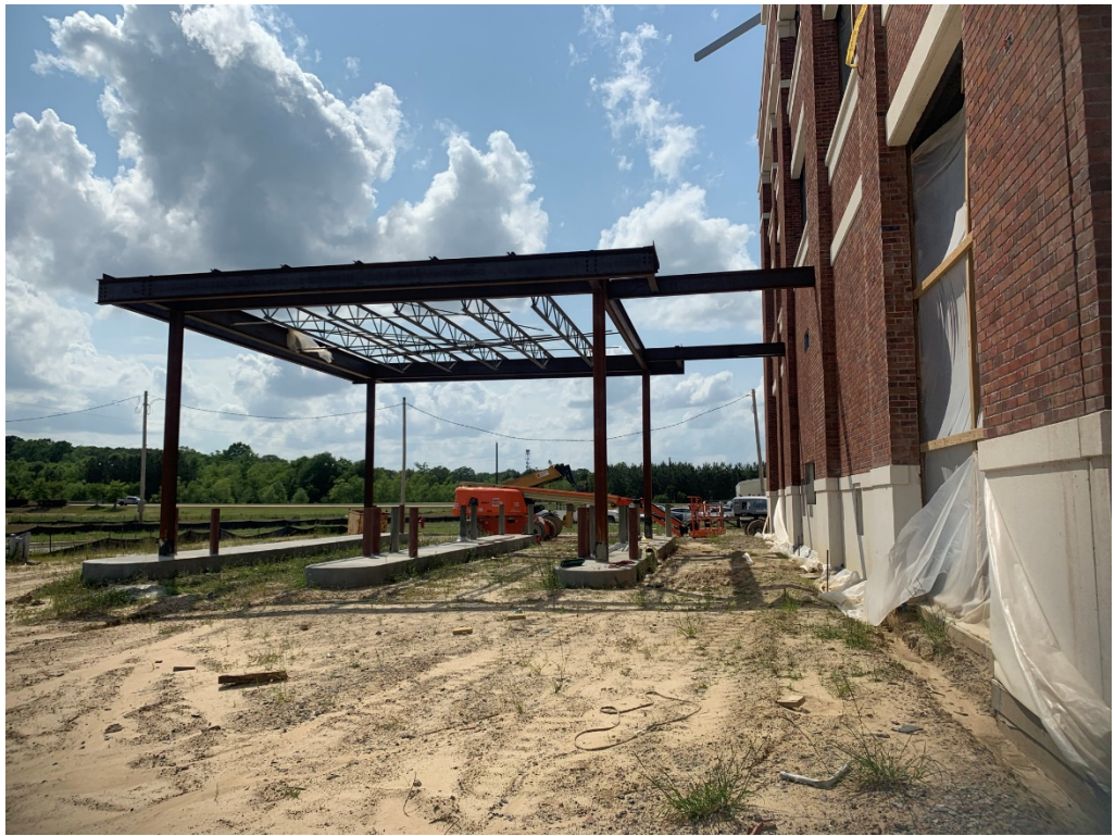
Figure 7 – Drive Thru Progress
