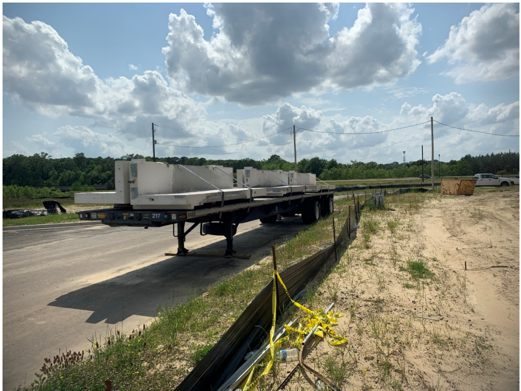
Figure 8 – Precast on Site Ready to Install
