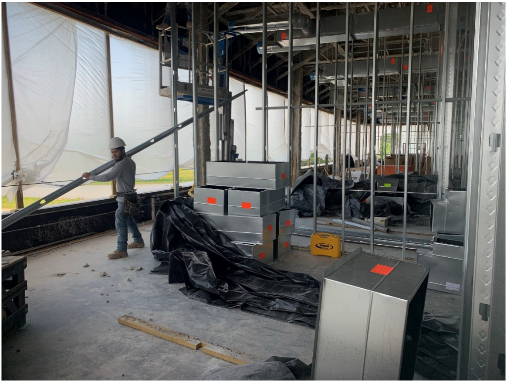
Figure 17 – Fourth Floor Framing is Ongoing
