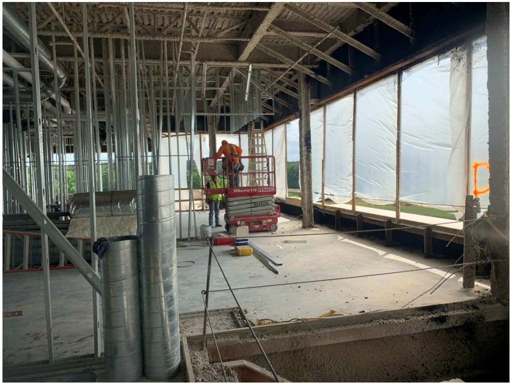
Figure 15 – Fourth Floor Framing is Ongoing
