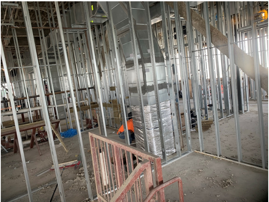
Figure 18 – Duct Insulation is Ongoing
