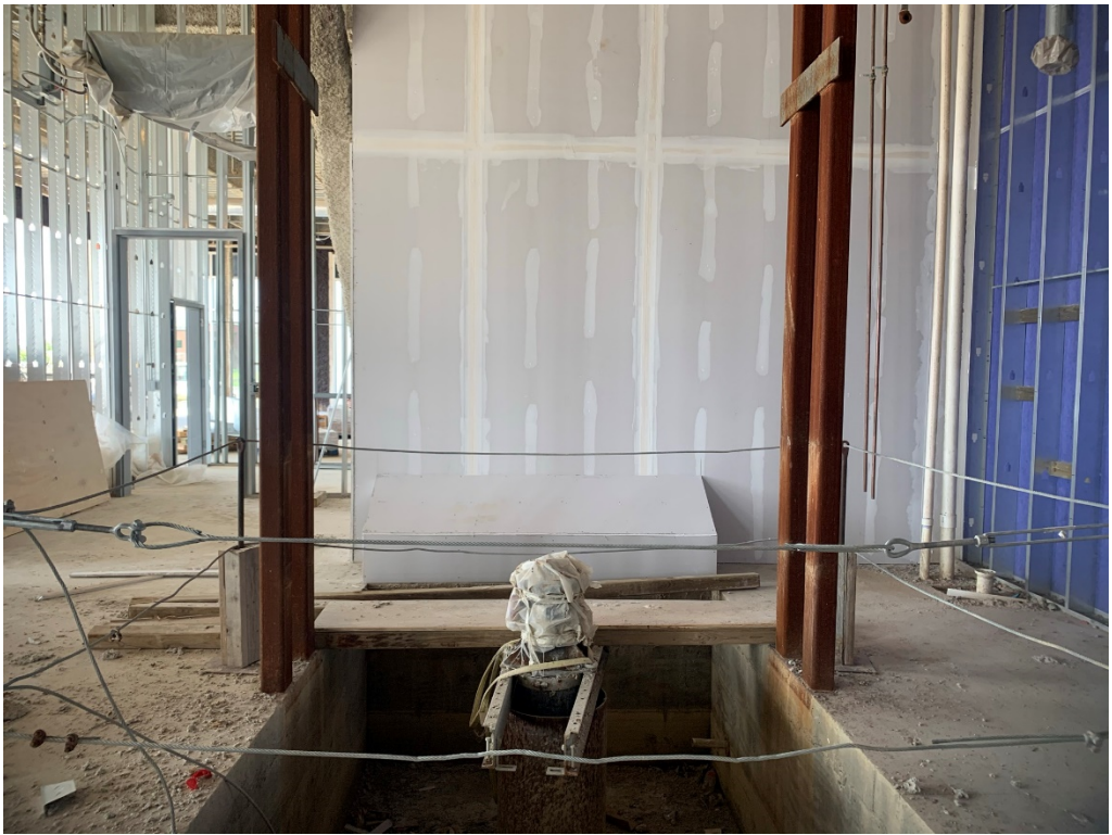
Figure 11 – Drywall at Shafts
