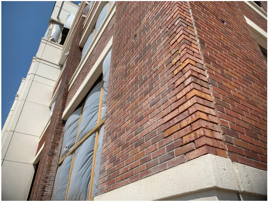
Figure 1 – SW Corner Brick Progress
