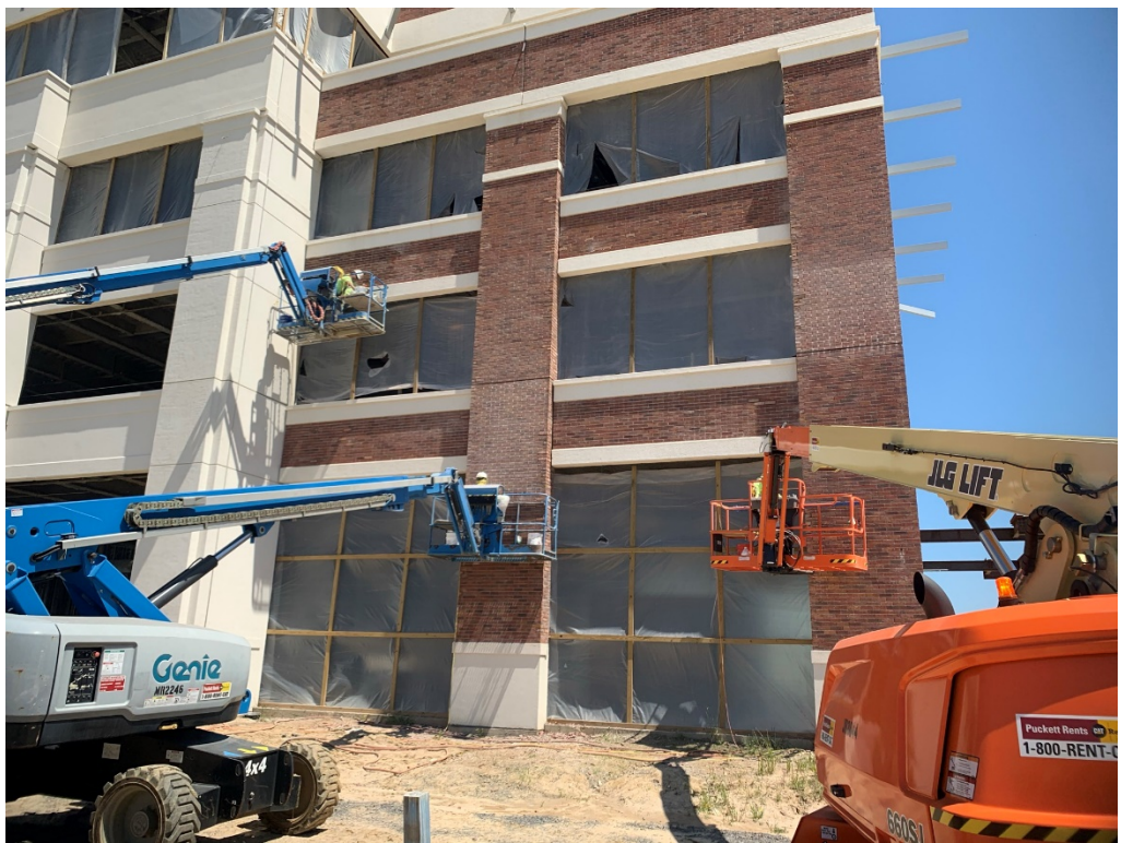
Figure 2 – Masons Reworking Brick
