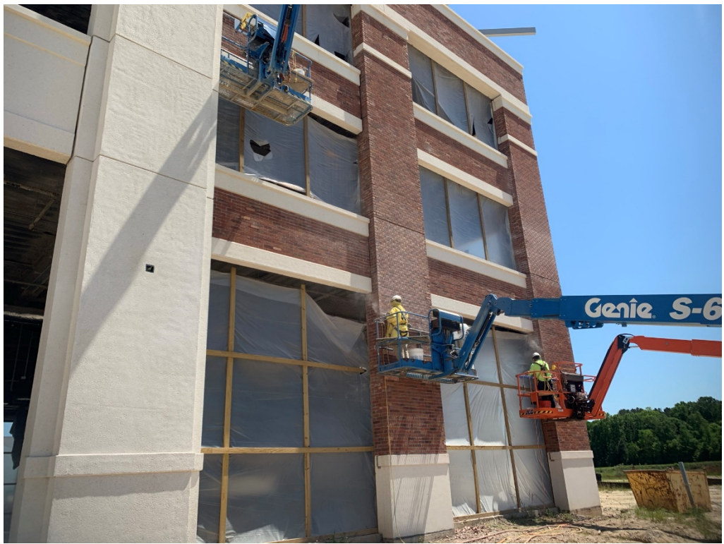
Figure 1 – Masons Reworking Brick
