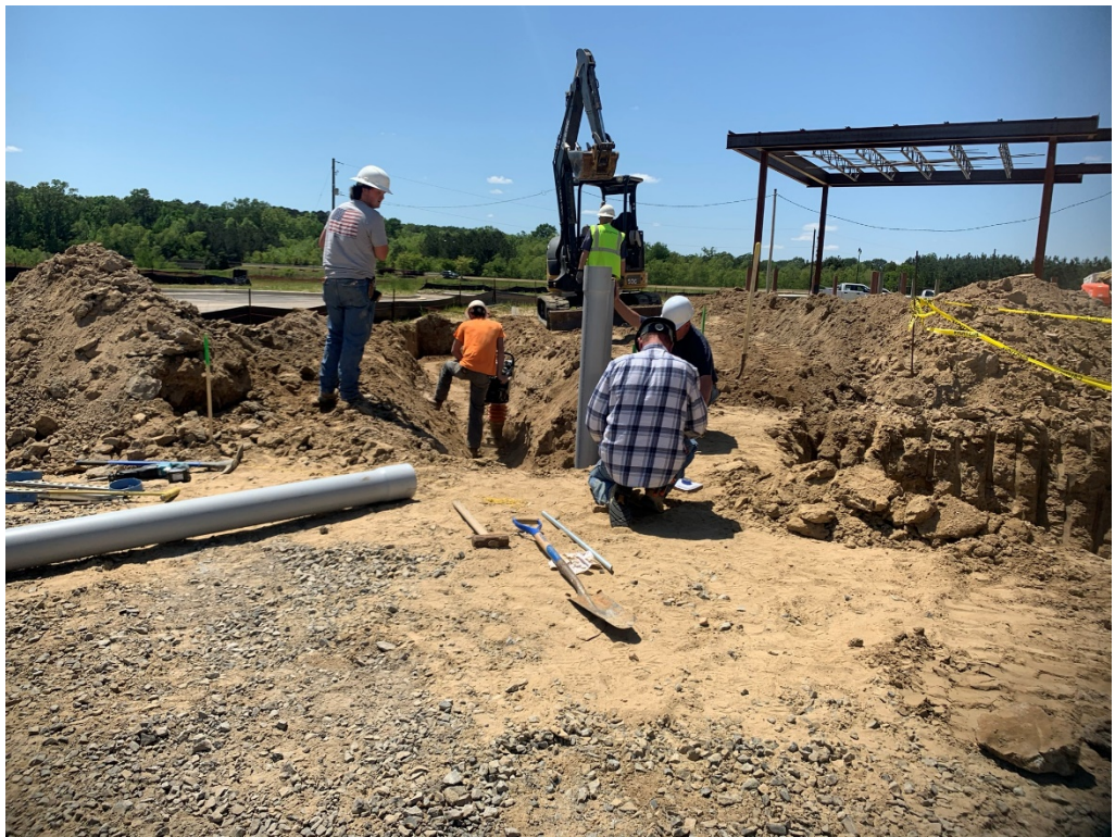
Figure 4 – Underground Electrical Work
