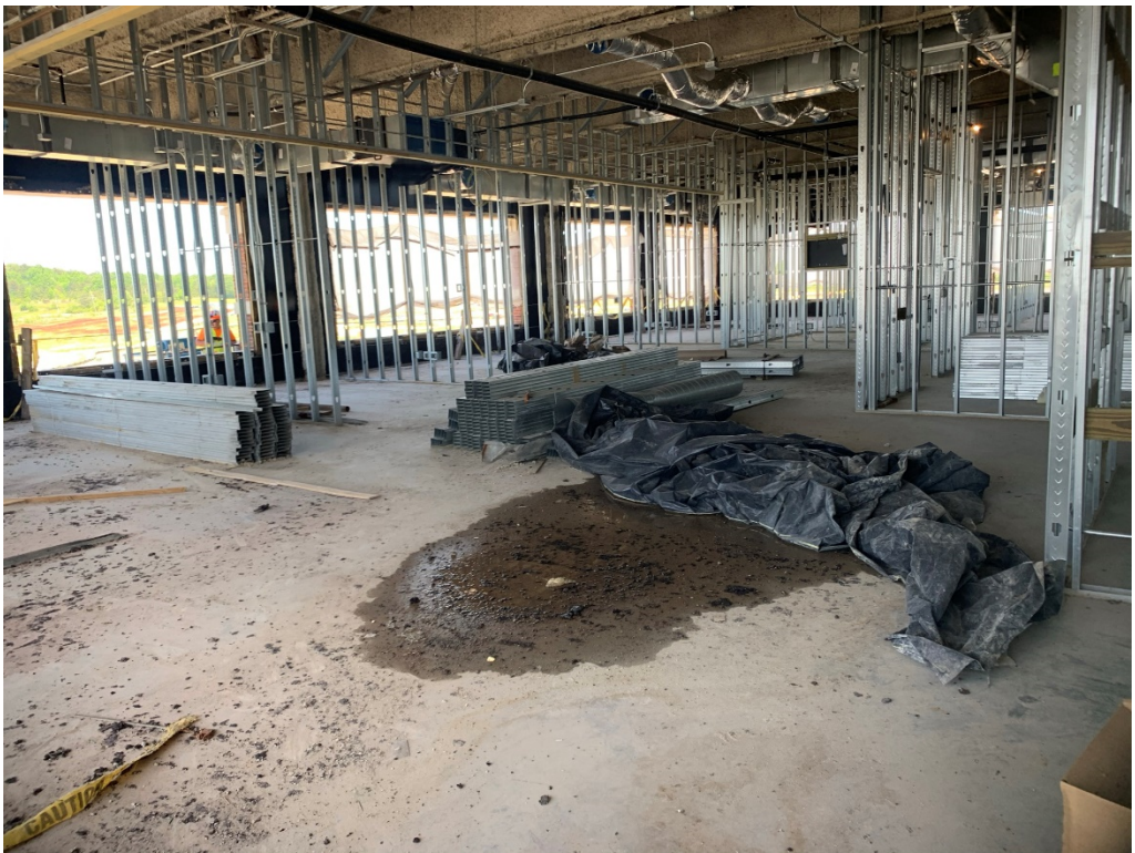
Figure 6 – 3 rd Floor Progress
