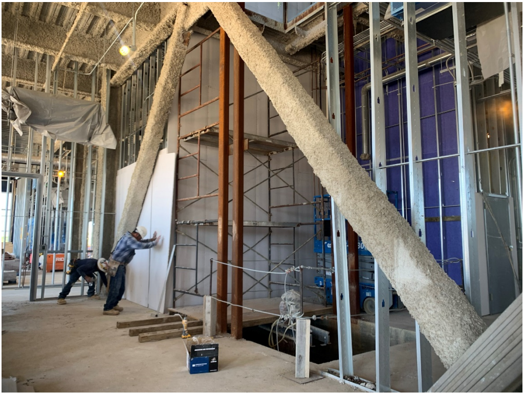
Figure 5 – First Floor Drywall Install at Elevator Shaft
