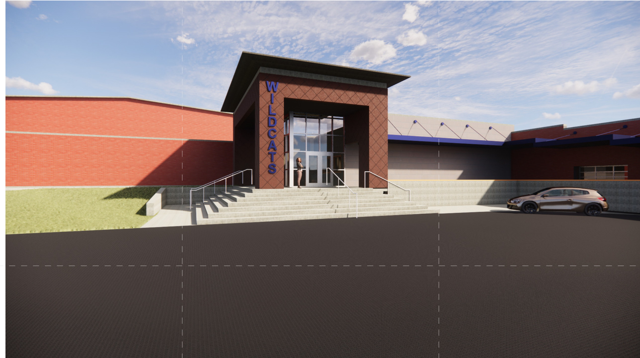
Car Drop Off & Gym Entry
