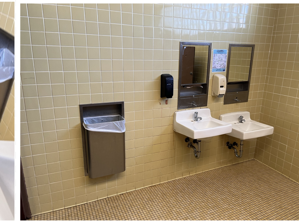
Typical Toilet Lav Wall
