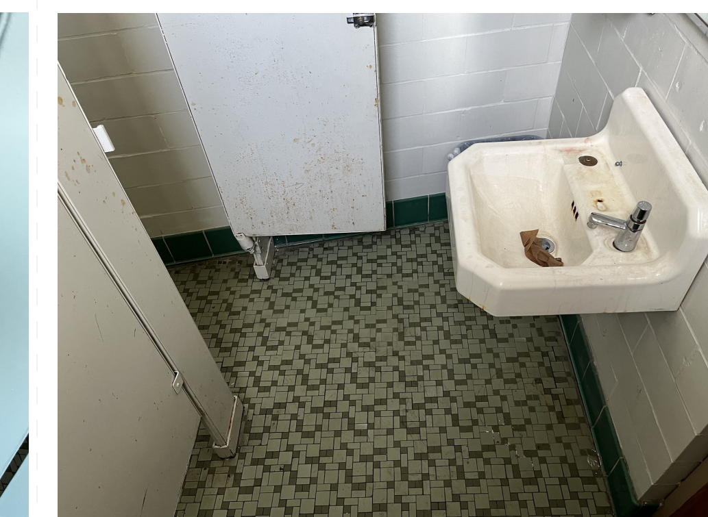
Typical Lav to Replace
