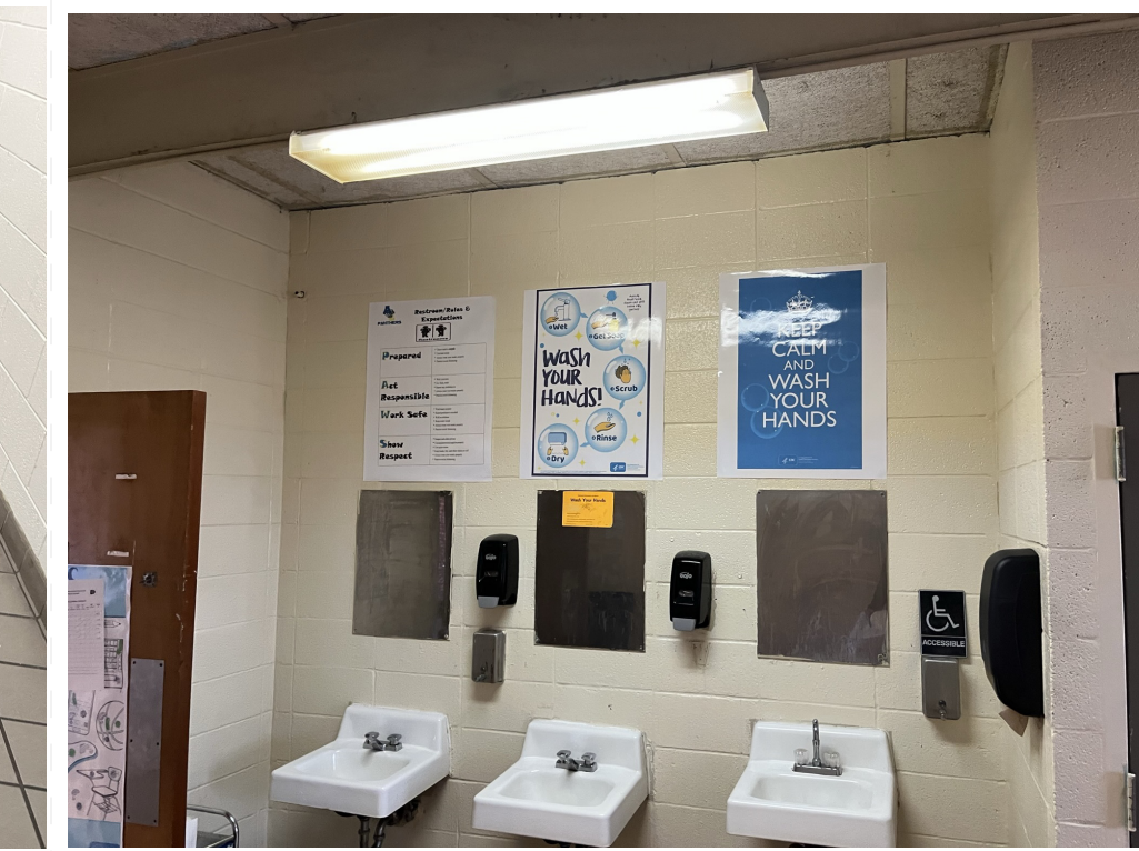
Typical Toilet Lav Wall
