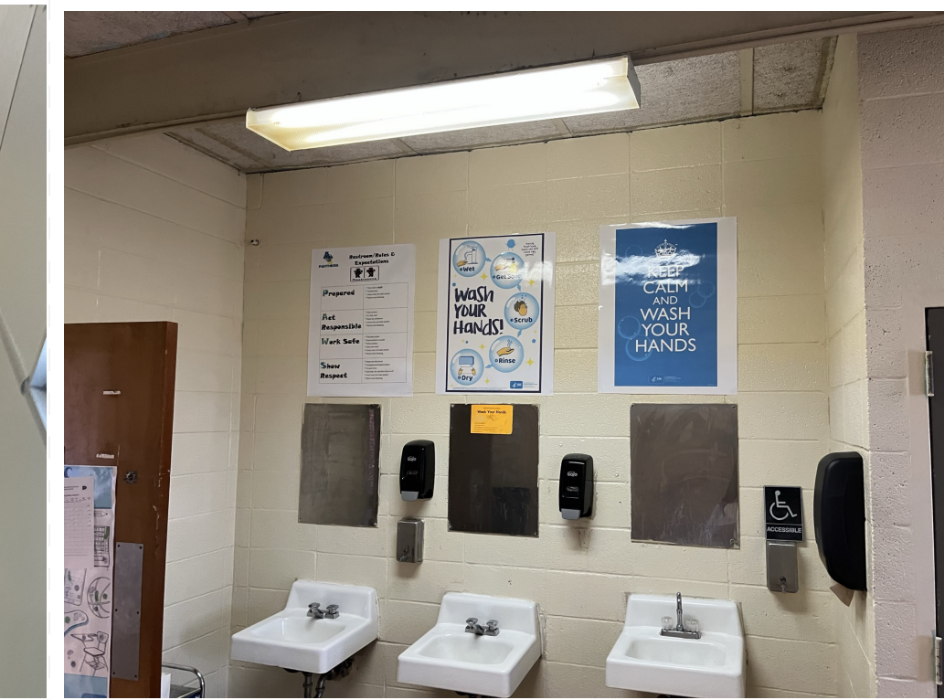
Typical Toilet Lav Wall
