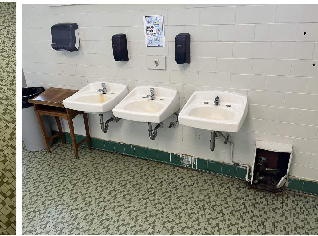
Typical Toilet Lav Wall
