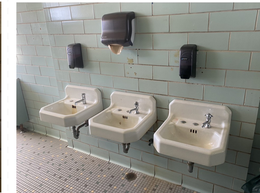
Typical Toilet Lav Wall
