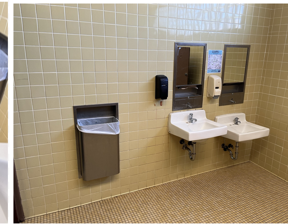
Typical Toilet Lav Wall
