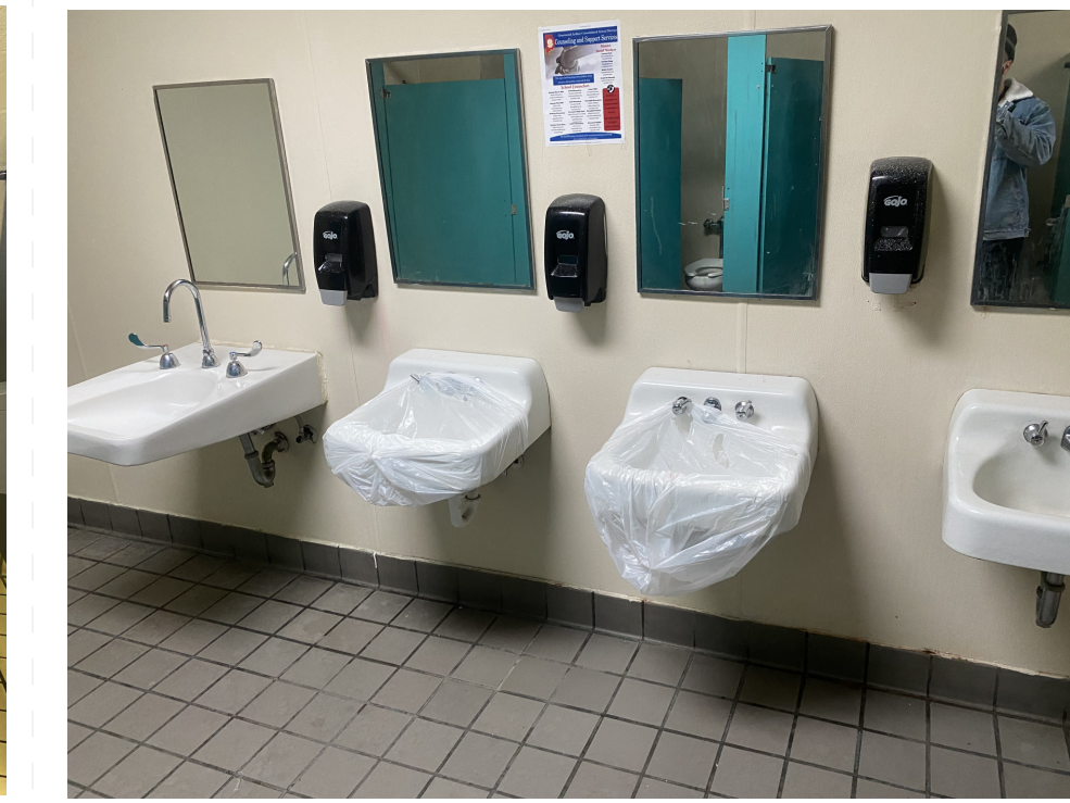
Typical Toilet Lav Wall
