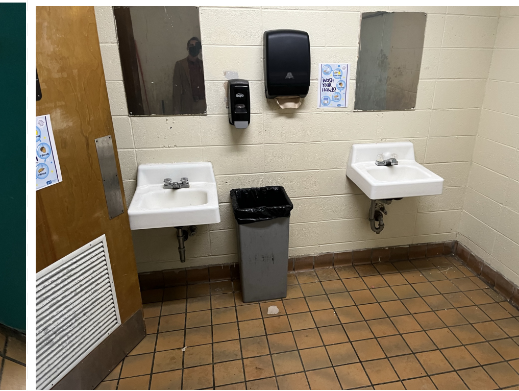
Typical Toilet Lav Wall
