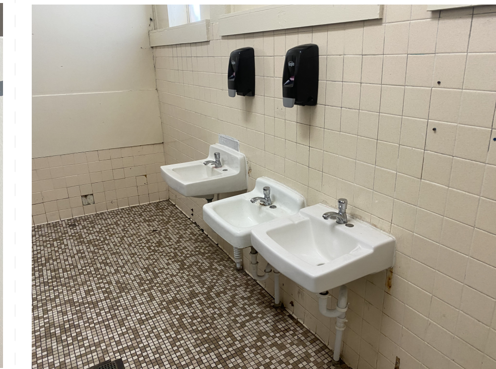
Typical Toilet Lav Wall
