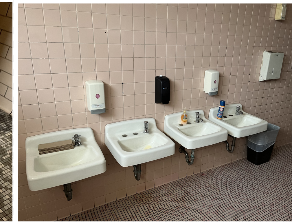
Typical Toilet Lav Wall
