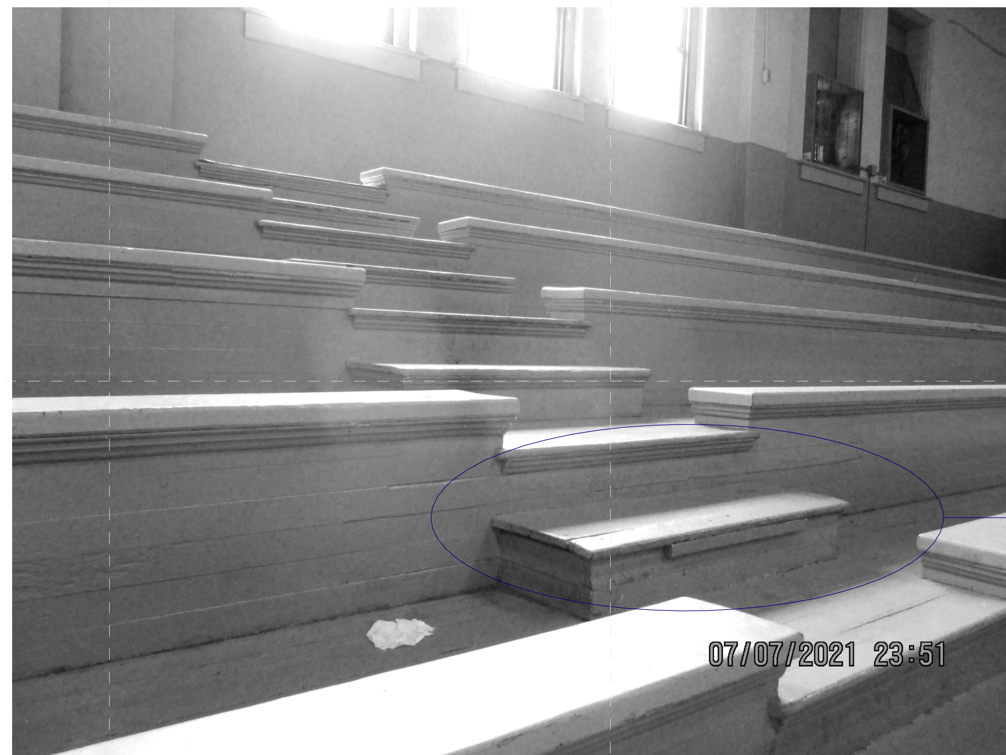
Example of Typical Repair
